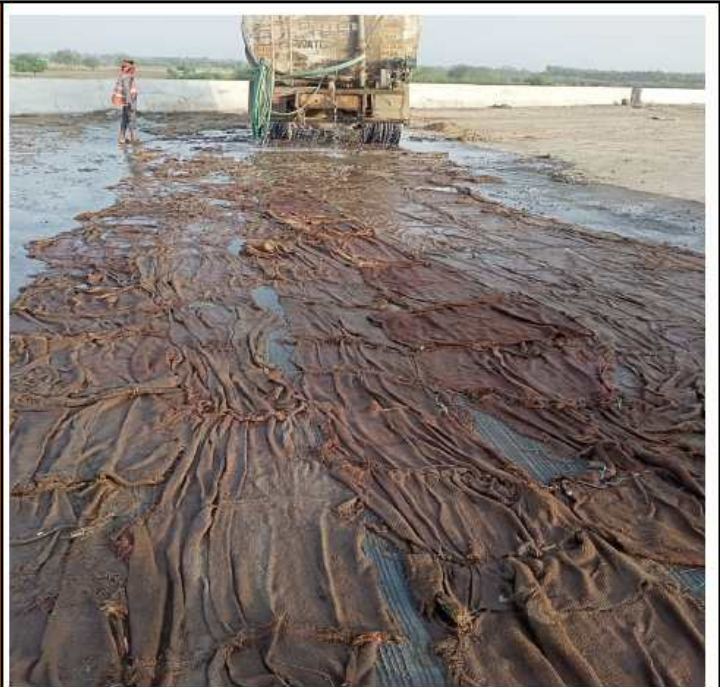
Ch- 313+809 A1&A2 approach slab wearing coat curing RHS
