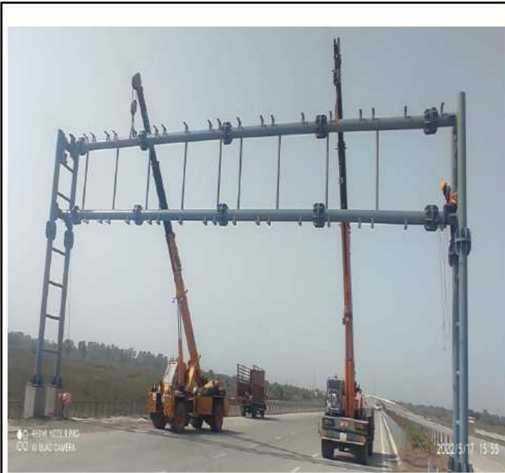
CH-321+900 Overhead gantry erection work in progress LHS
