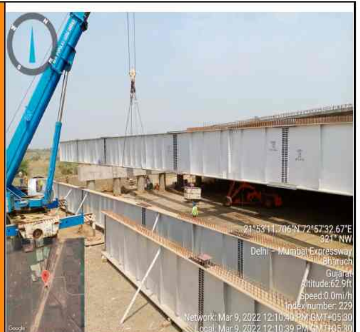
CH-309+074 MNB Steel girder launching work in progress LHS G1 to G6 of S1
