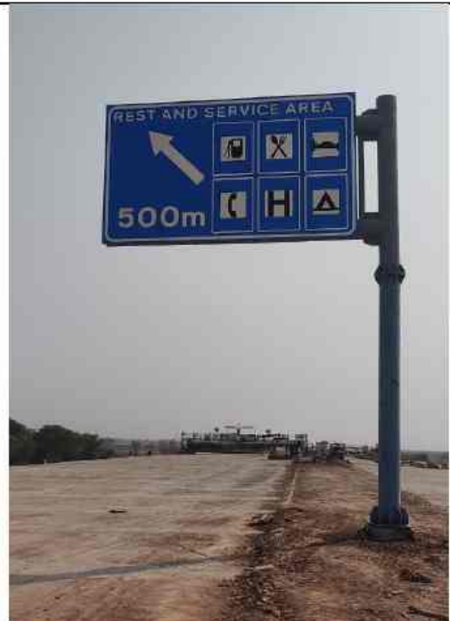
500m way side amenities sign board gantry erection completed.
