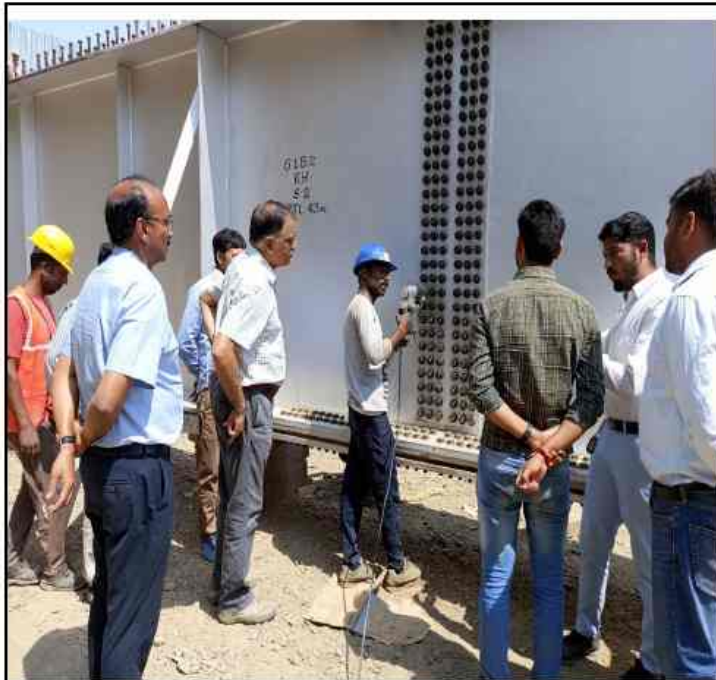
CH-309+074 MNB Steel girders bolts torque checking by IE team at
