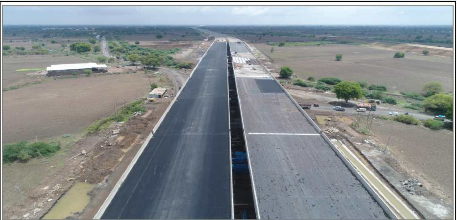
ROB at 293+014 LHS Completed, RHS last Slab Reinforcement in Progress
