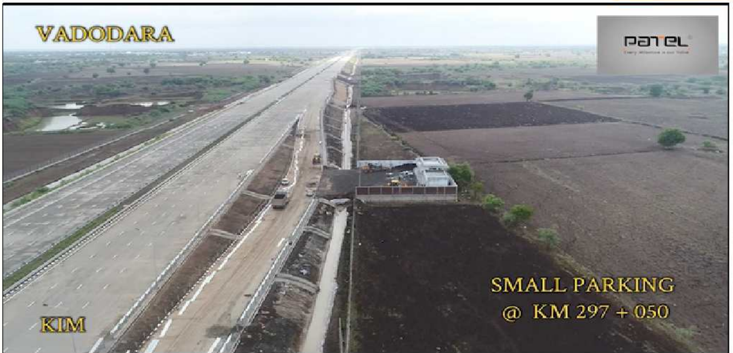
Small Parking at Ch.297+050 and its Ramp
