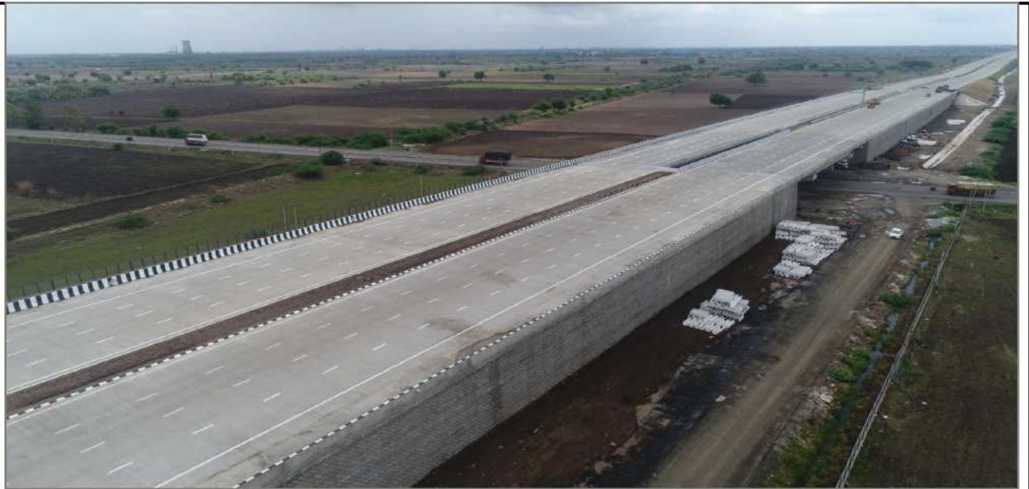
Ch 299 +354 Flyover Completed
