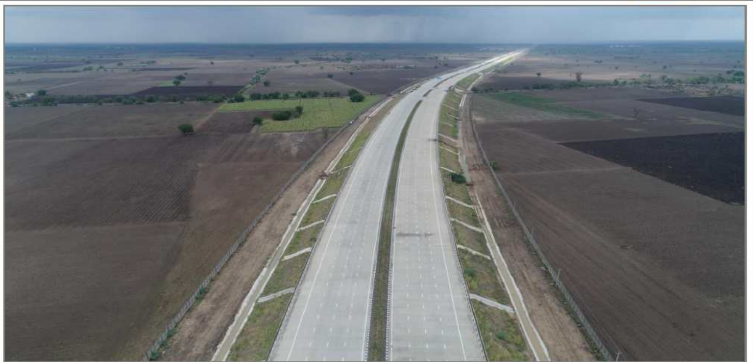
Ch 303+800 with all finishing works of Highway completed
