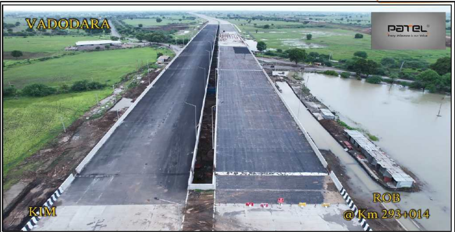
ROB at CH 293+014 BC Work in Progress
