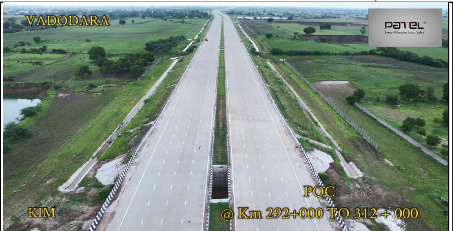
Highway works completed Ch 292+000 to Ch 312+000
