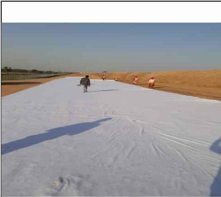
Ch-323+075 Re wall A1 side closing wall 3 (segment-11A , length-15.20m) 4th layer geogrid laying
