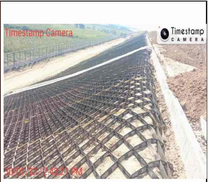
318+610 to 318+750 Geocell laying in progress RHS
