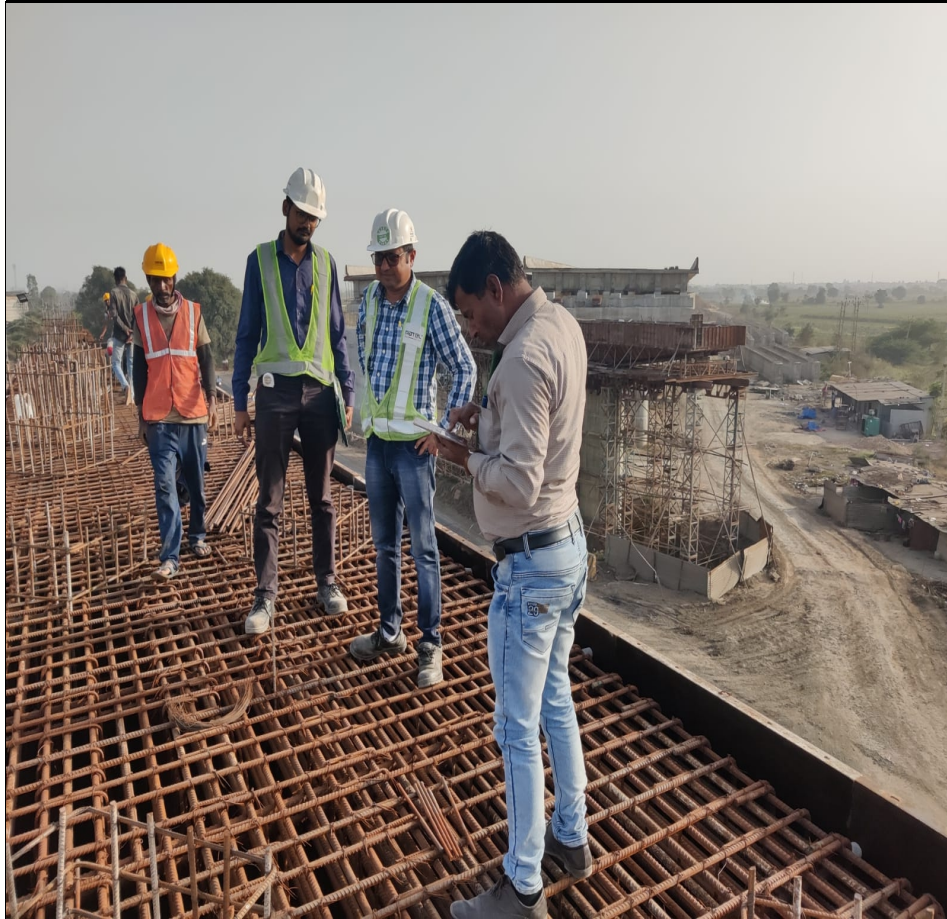
CH-293+014 P8 pier cap checking with railway official LHS
