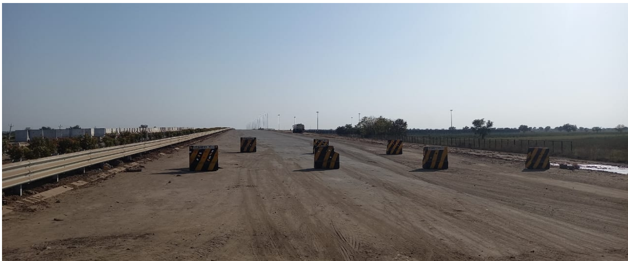
Installed NJ barrier
