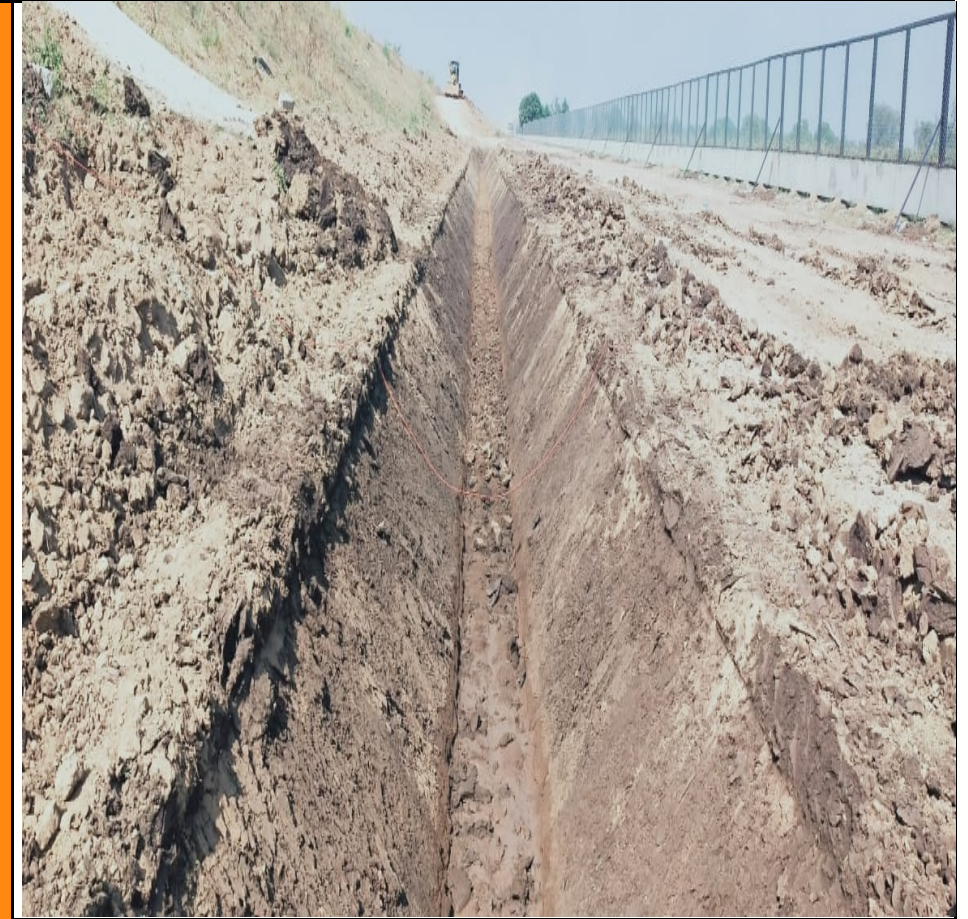
ch-317+050 to 317+180 toe drain excavation. RHS
