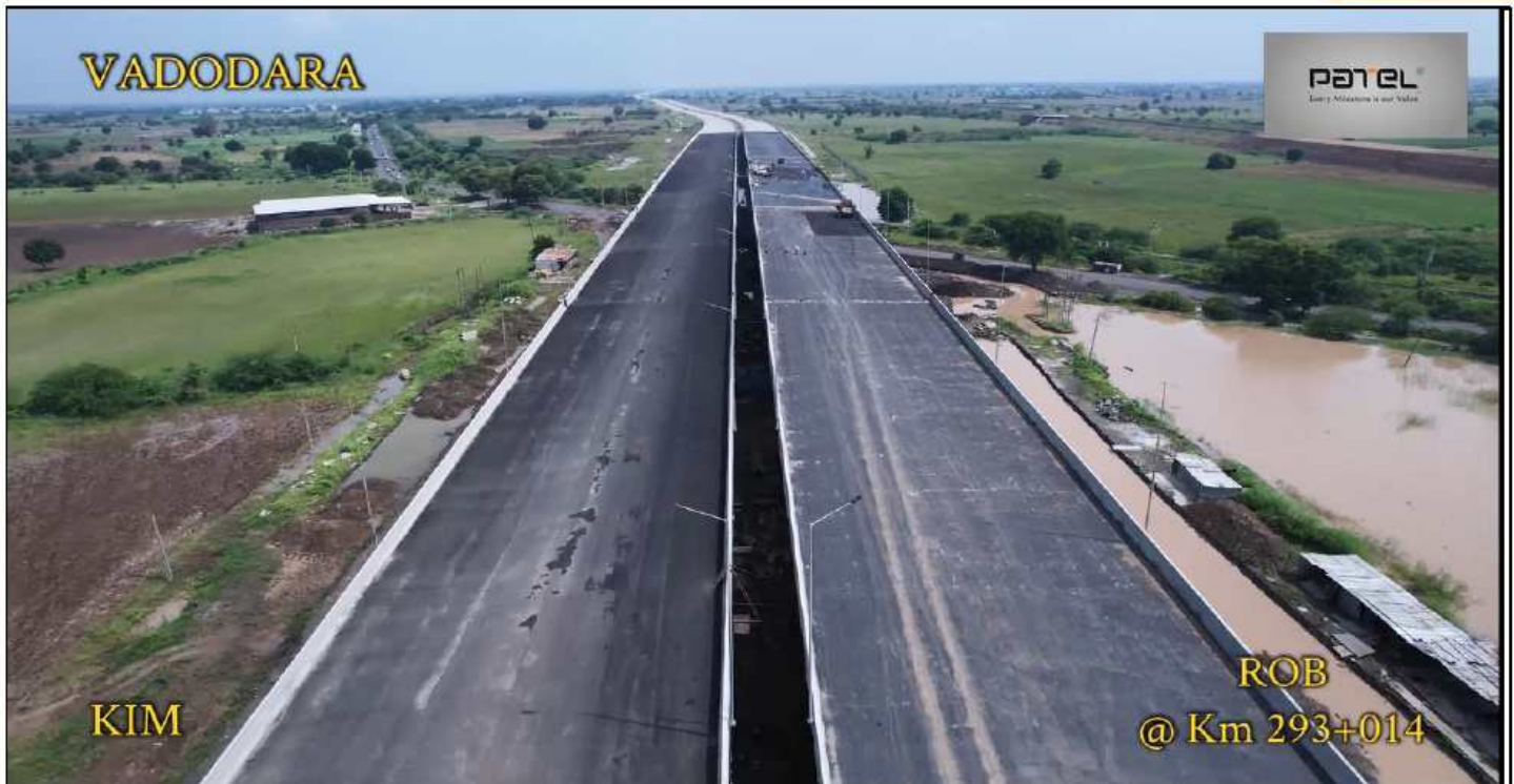
ROB @ Ch. 293+014 All Slabs completed, BC Work in Progress
