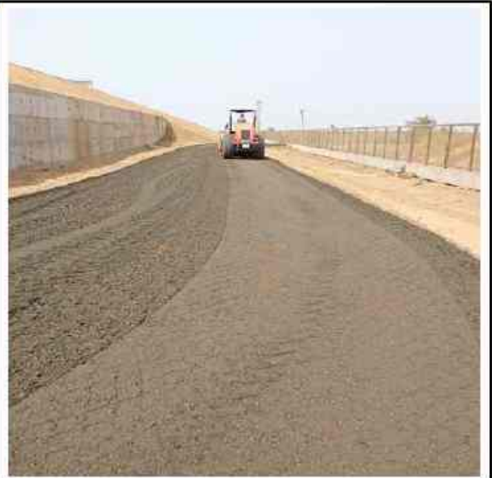
Ch- 318+890 to 318+975 Connectivity road WMM 1st layer Rolling RHS
