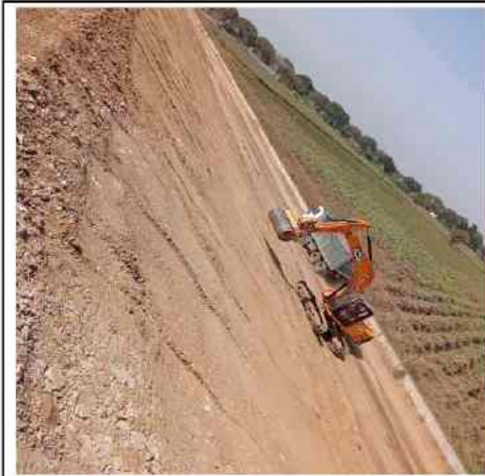
Ch- 319+100 to 319+200 Slope Rolling LHS
