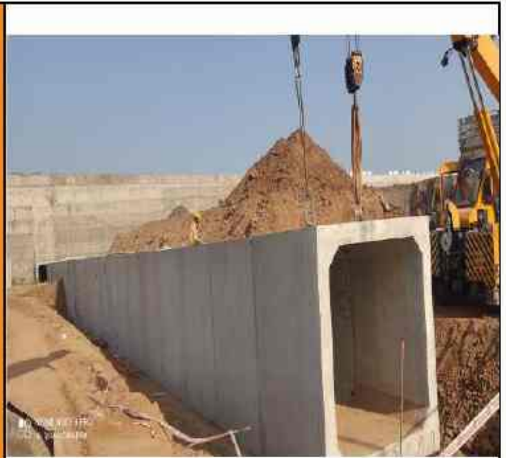
Ch- 0+460 ramp-1 precast box (52.00 m) erection work completed LHS
