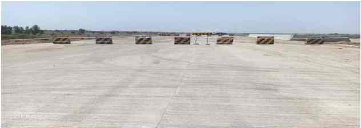
NJ barrier installed
