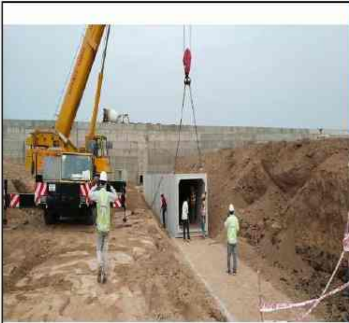
Ch- 0+460 Precast Box segment erection work in progress LHS
