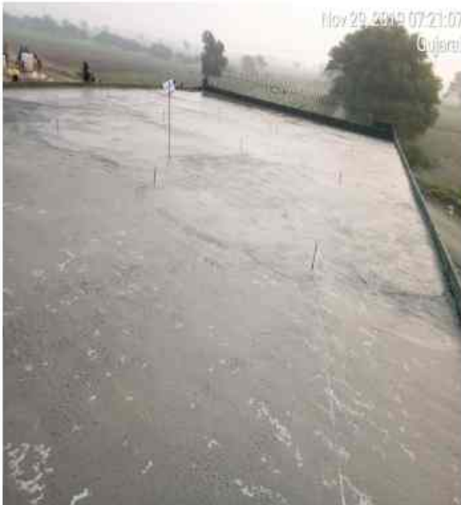
At Chainage no 311+047 LVUP RHS top slab
