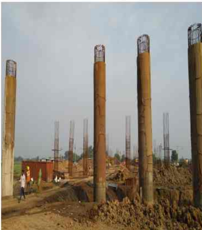
Pier Shaft Curing at ROB
