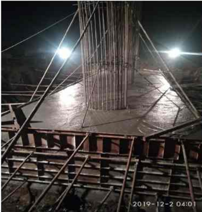
CH 293+014 ROB P10 LHS pile cap complete
