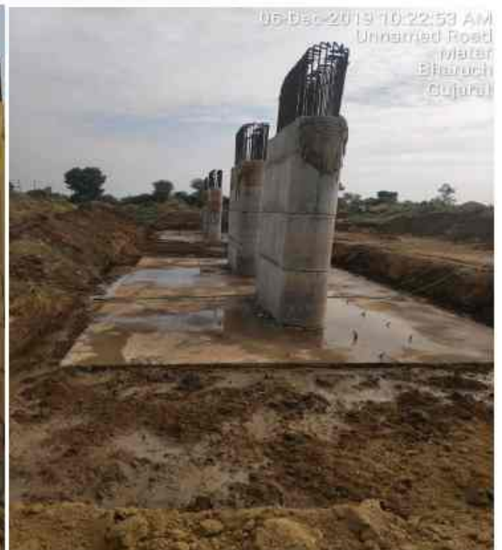
Mjb CH 321+253 P1 BHS Pier Shaft
