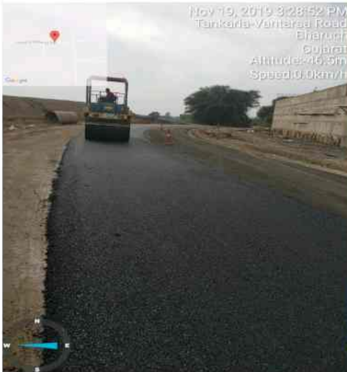
DBM laying in progress - Ch - 311+040 Diversion
