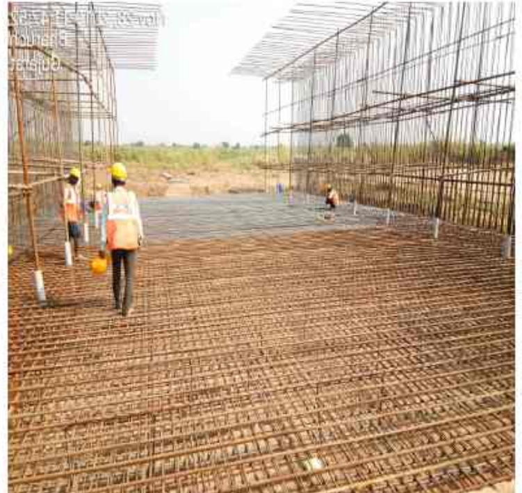
Ch. 309+550 PUP LHS Raft top reinforcement binding .
