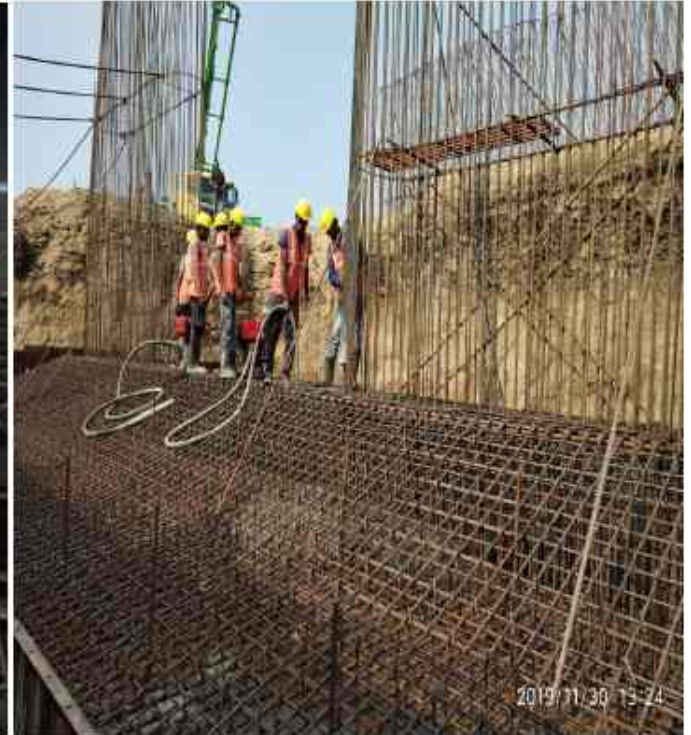
CH 318+870 MJB LHS P2 RAFT Concreting
