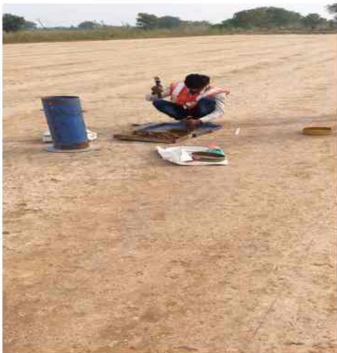
Chainage 304+500 to 304+660 RHS side Embankment TOP
