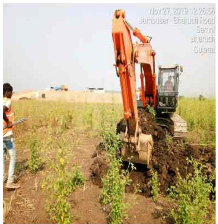
Toe wall excavation from Ch. 308+420 to Ch. 308+540 .
