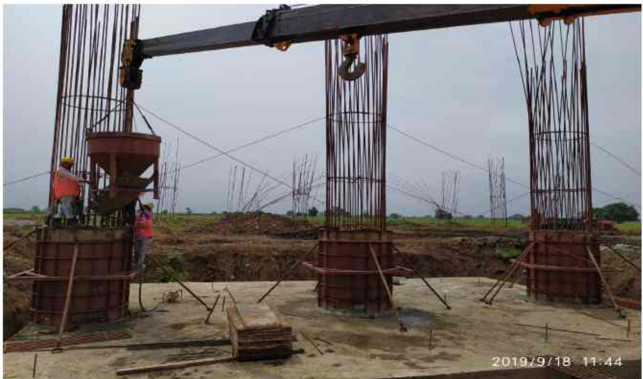
ROB P1 shaft concreting
