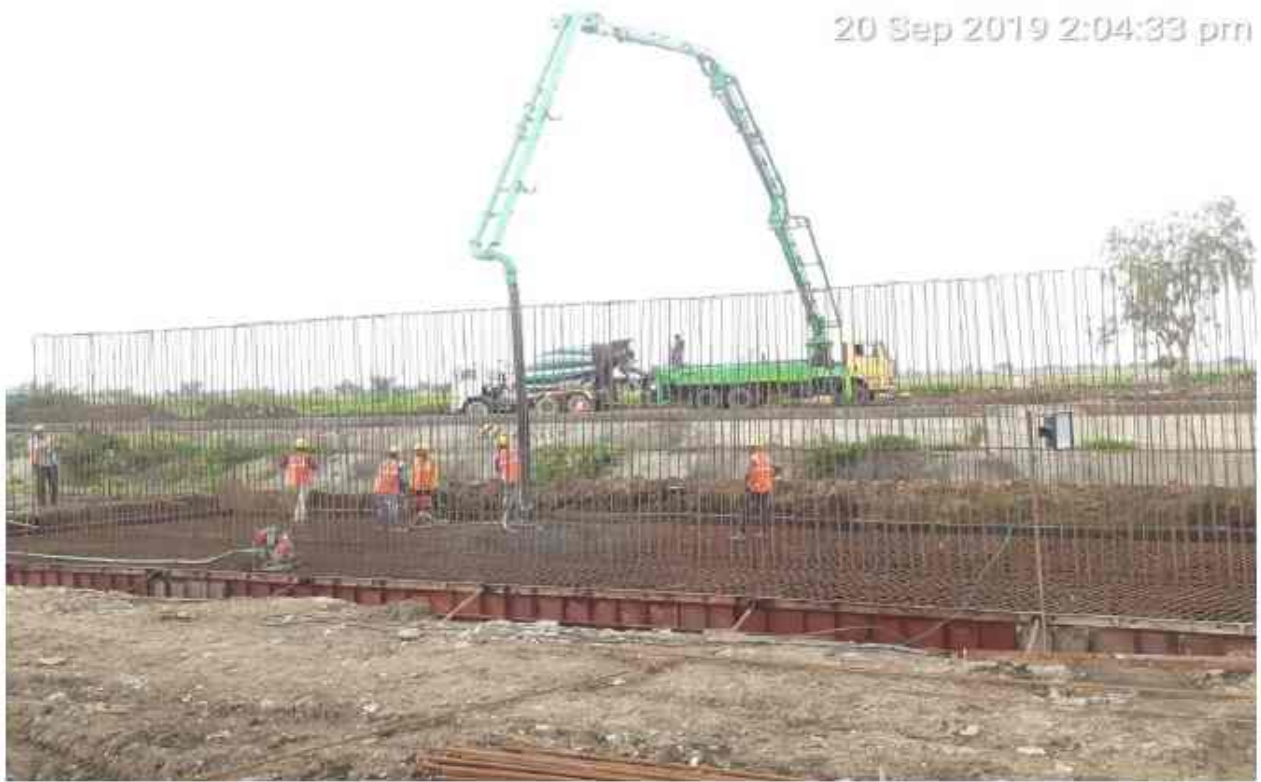
307+733 MNB pile cap Concreting
