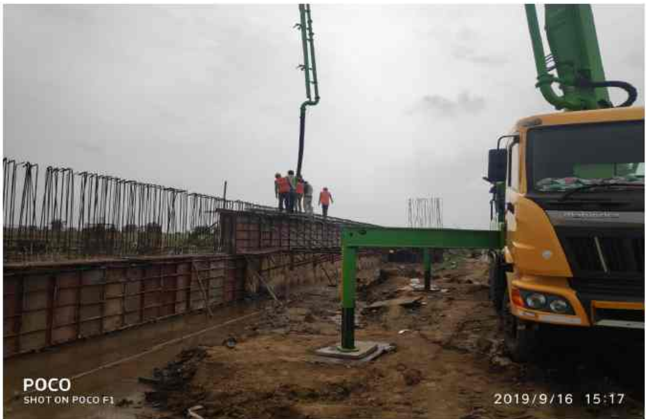
321+253 MJB Abutment concreting
