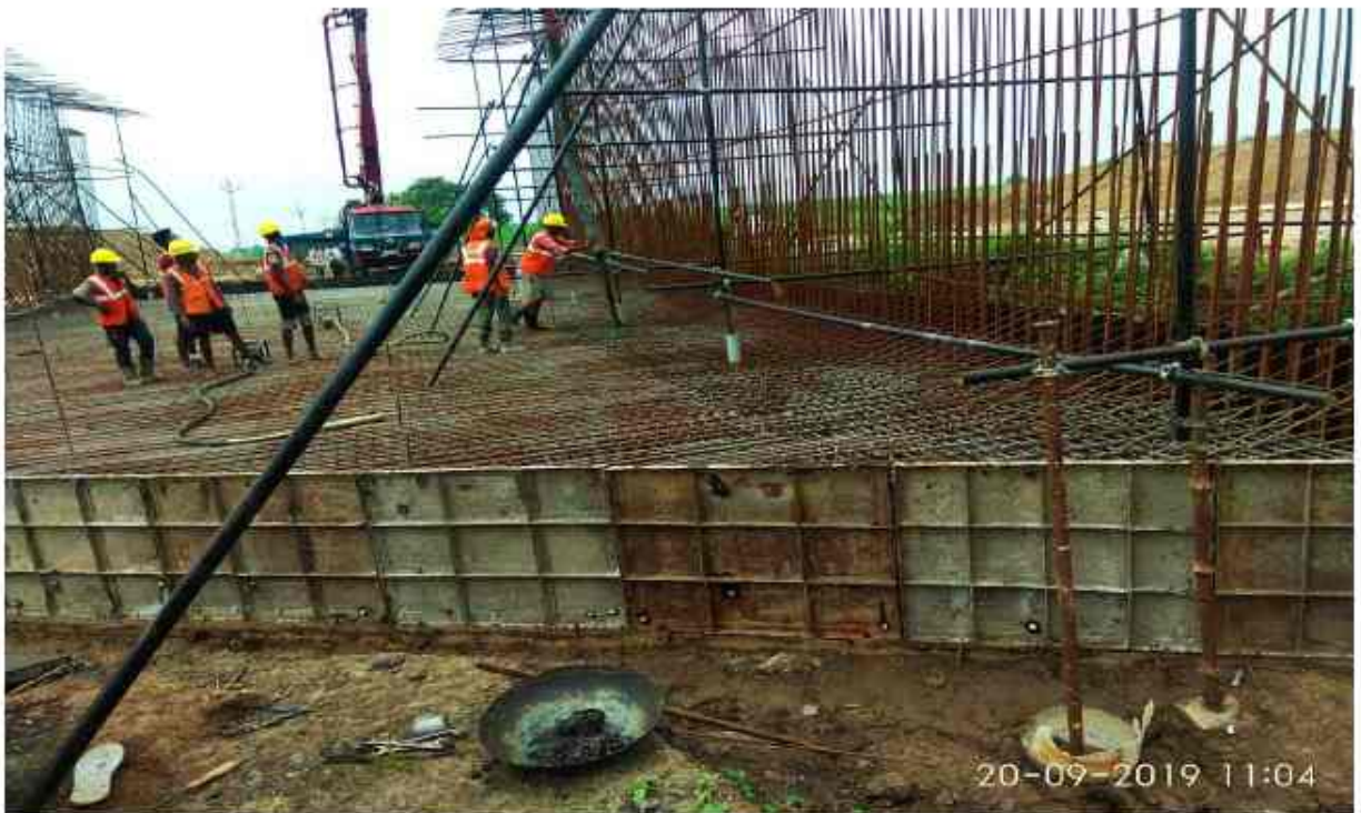
311+047 LVUP raft Concreting
