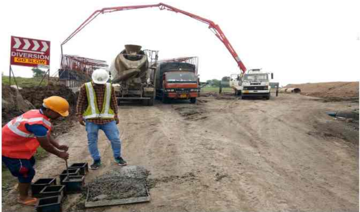
on site Cub casting at 311+047 LVUP
