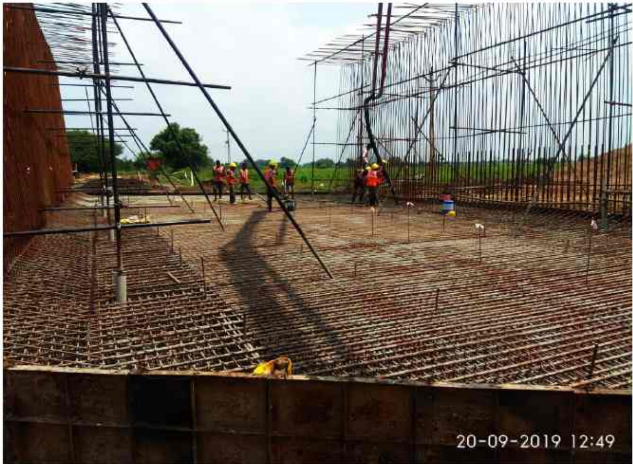
VUP ch 303+808 raft concrete work
