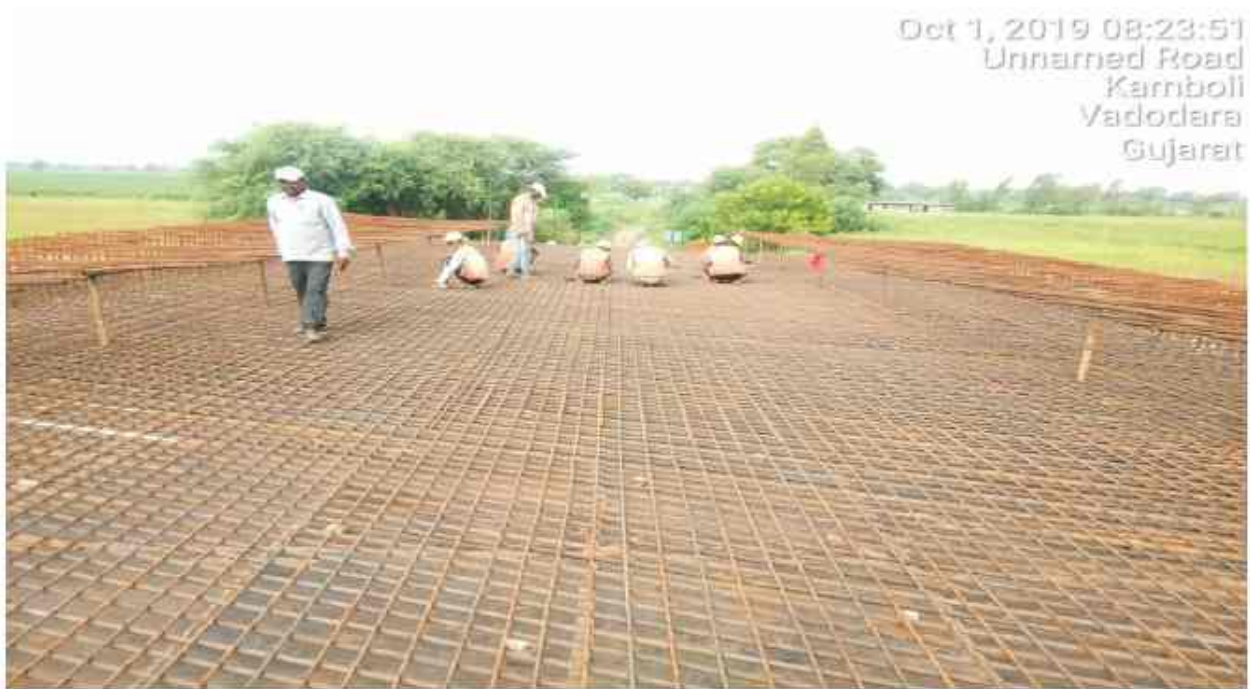
311+047 LVUP slab Reinforcement
