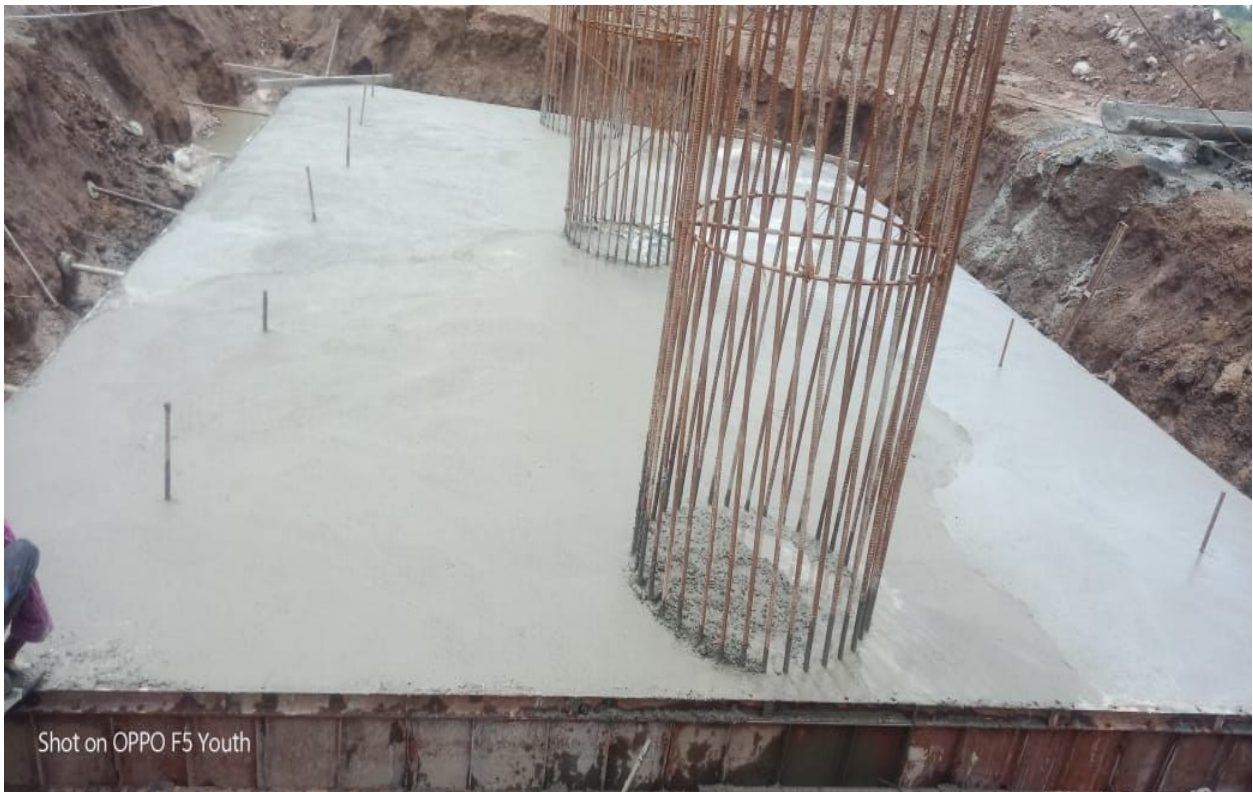
Pile Cap Concrete done at ROB Km293+014 P2 RHS
