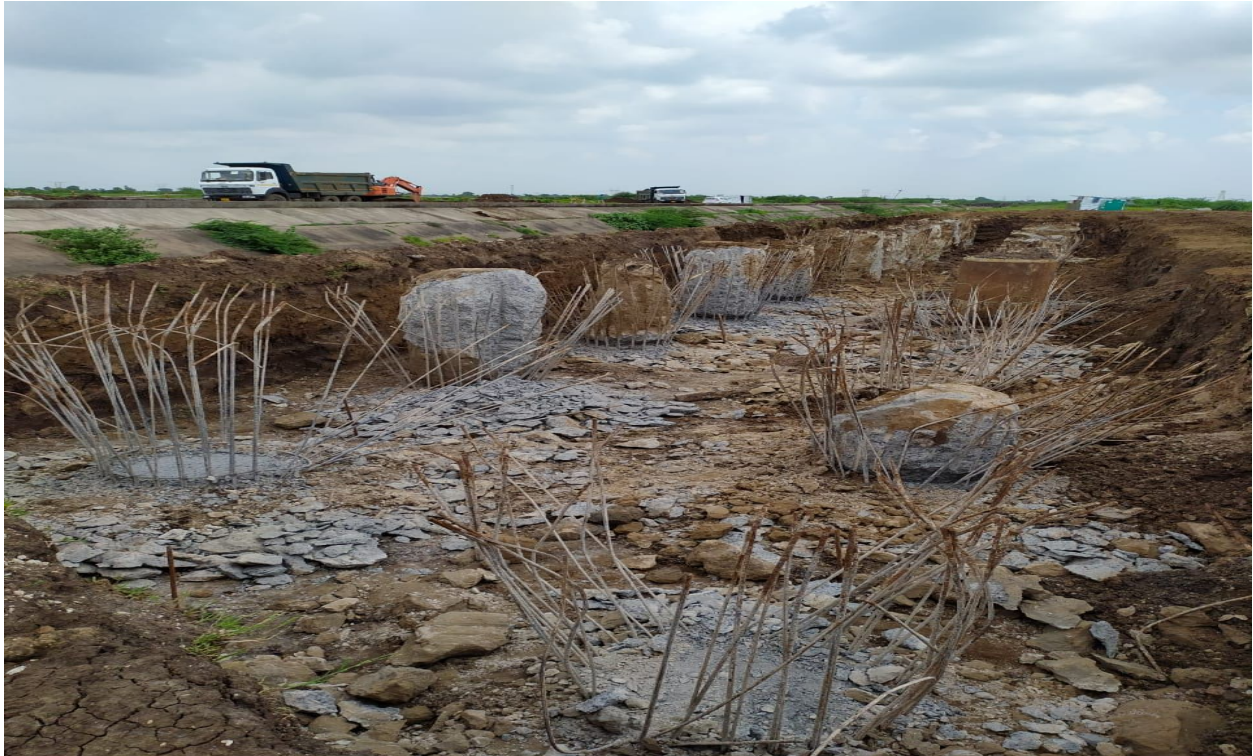
Pile Chipping at 307 +733 MNB A1 side
