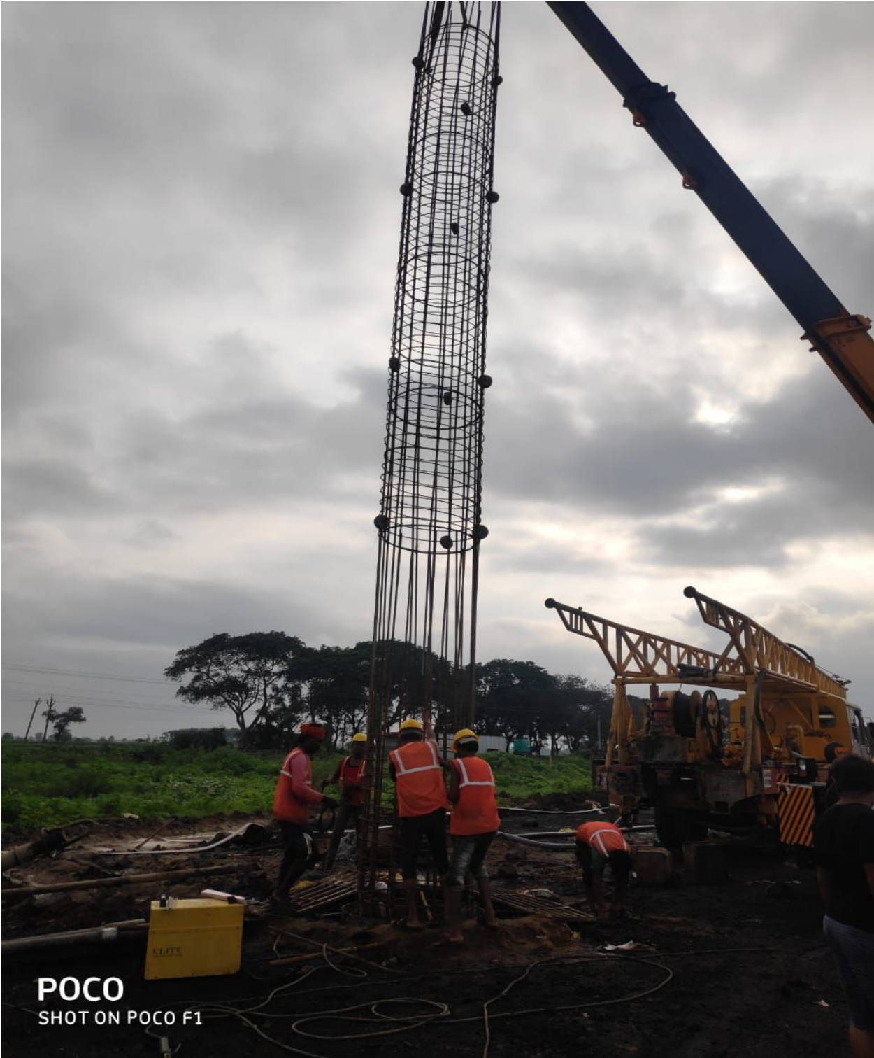
Km 318+870 MJB pile cage lowering in progress at A2 abutment
