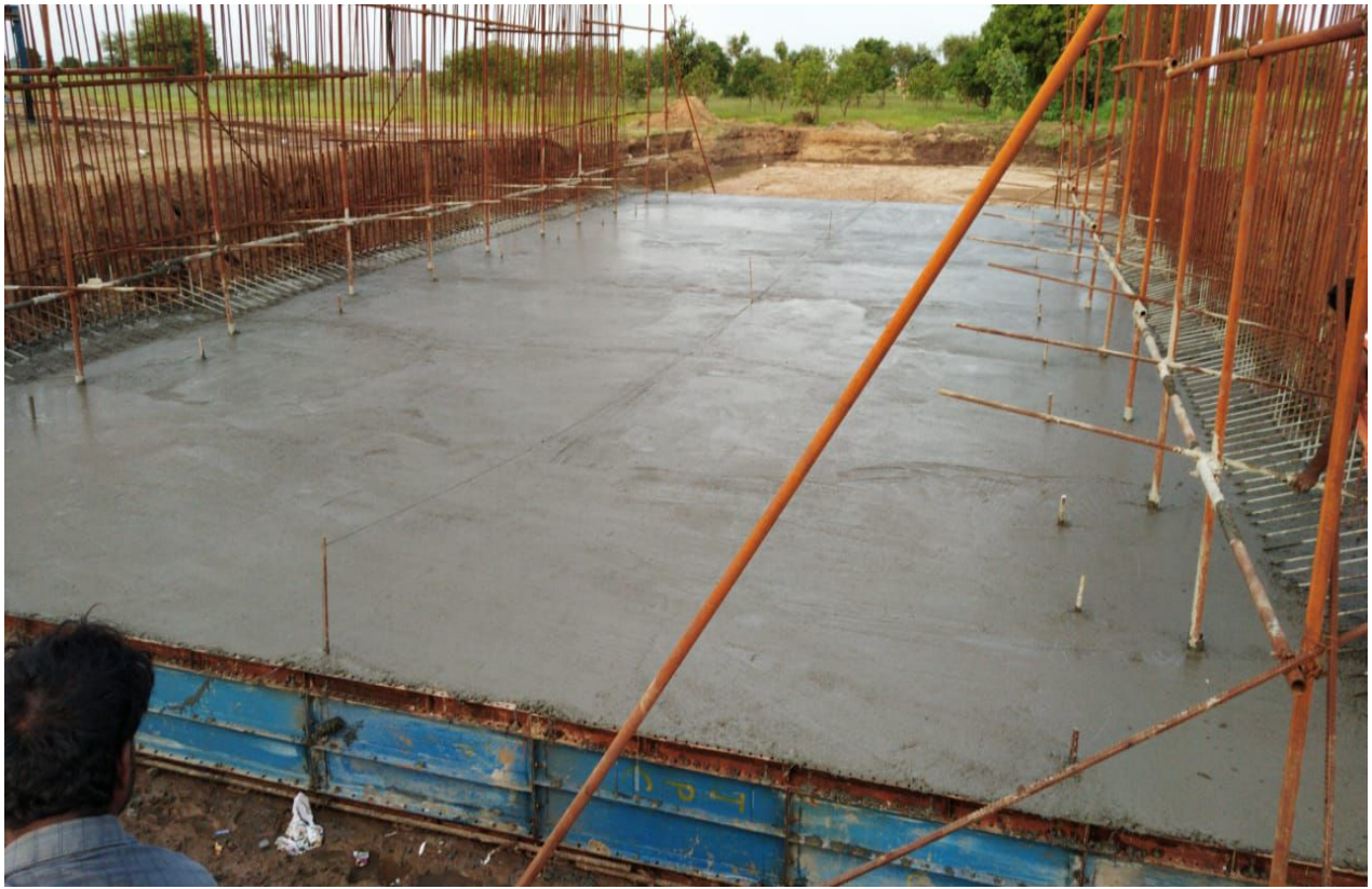
PUP Raft Completed @295+151 LHS
