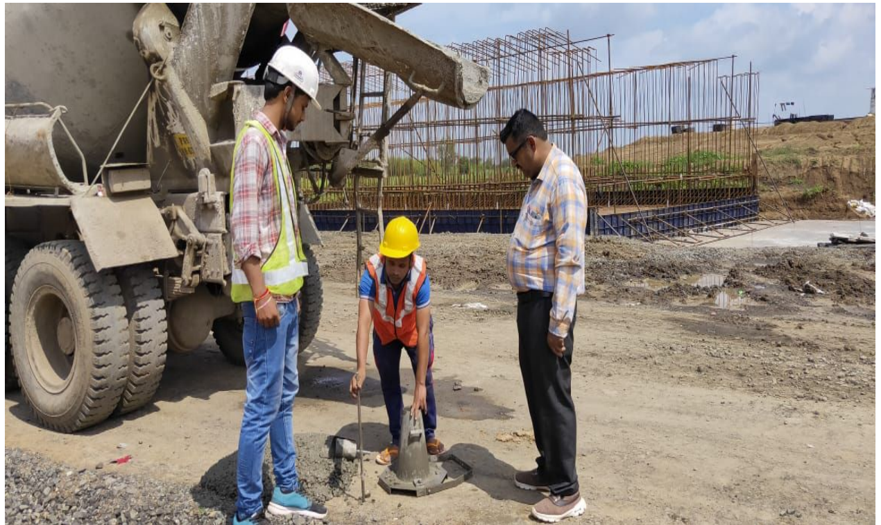
Slump Testing at Site
