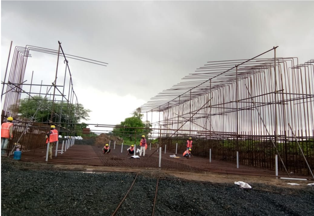
Concreting for Raft-LHS @311+047 LVUP
