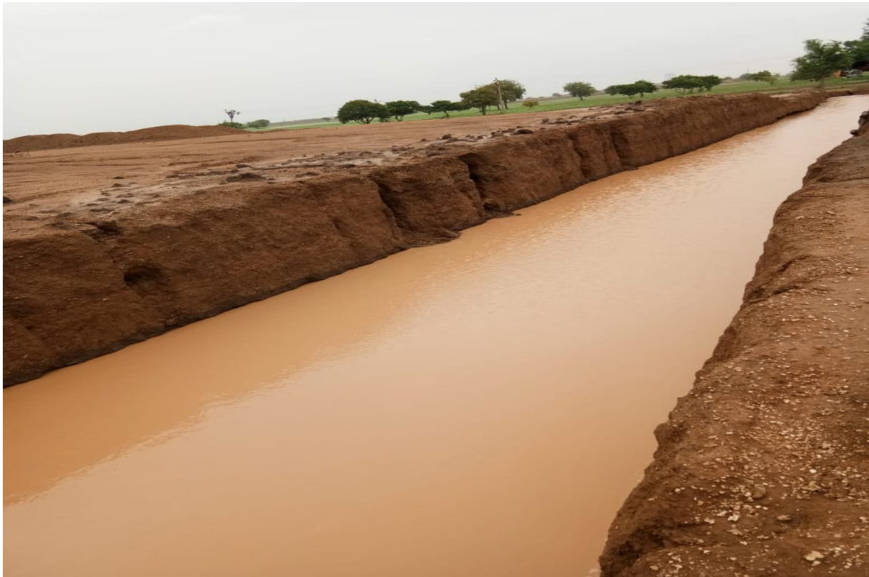
CH.295+585 Box Culvert Dewatering
