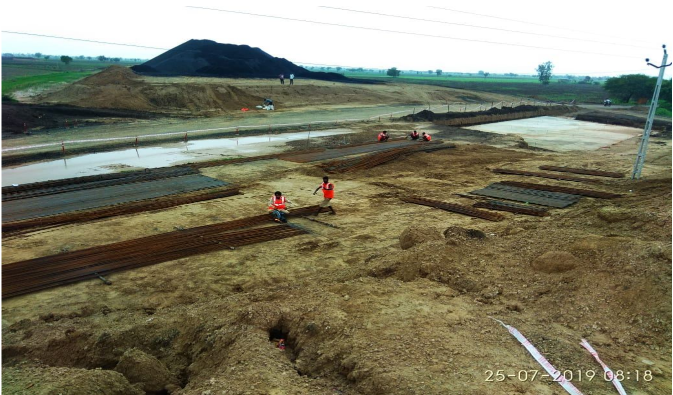
ROB Pile Cap Reinforcement work
