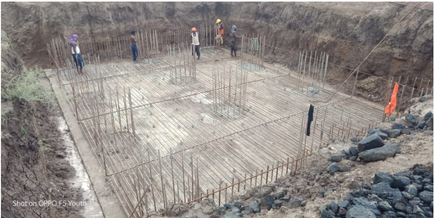
ROB Pile Cap Reinforcement work
