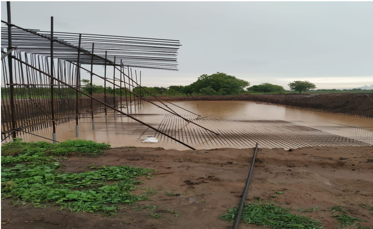
CH.295+151 PUP Reinforcement work
