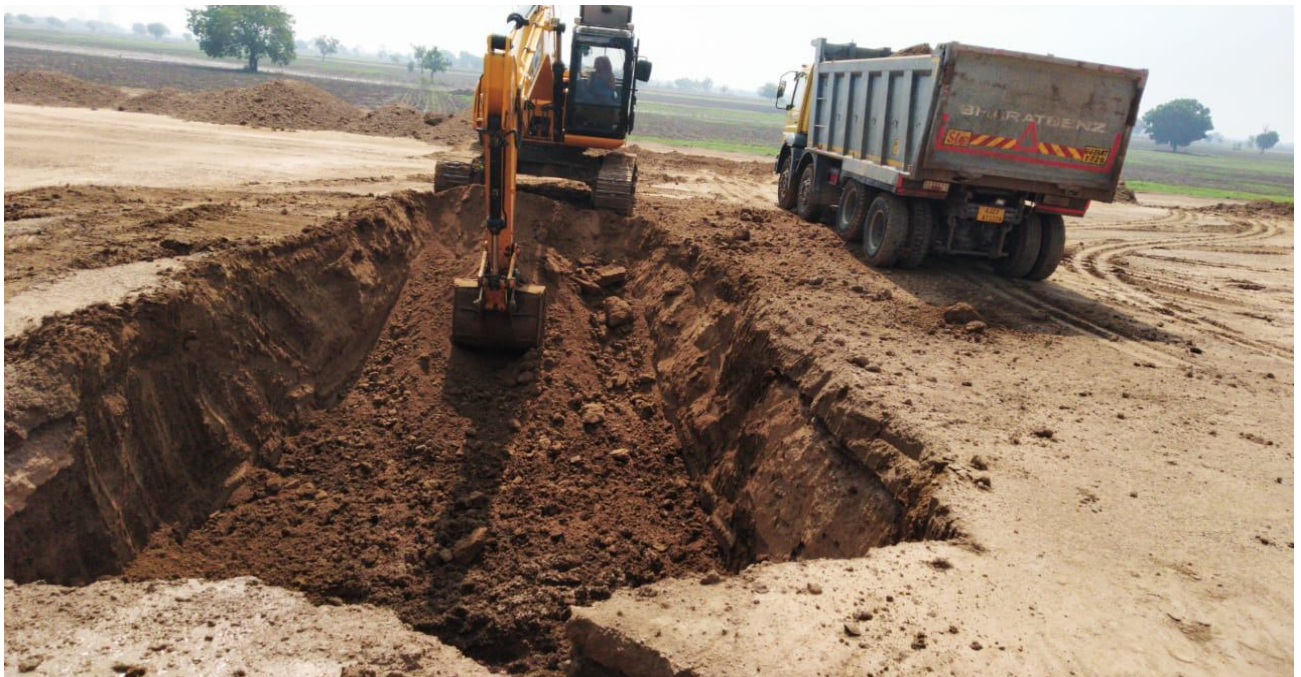
CH.294+520 PUP Excavation work
