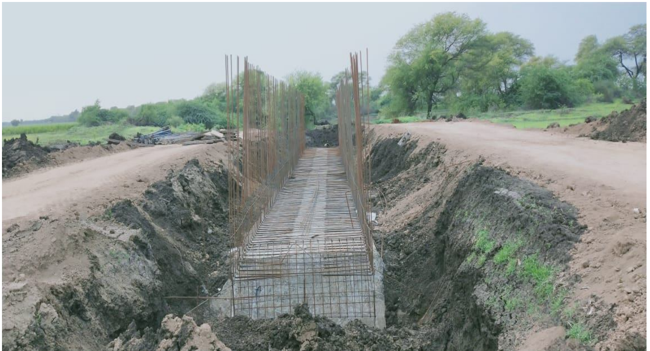
Ch. 316+420Box Culvert Reinforcement work
