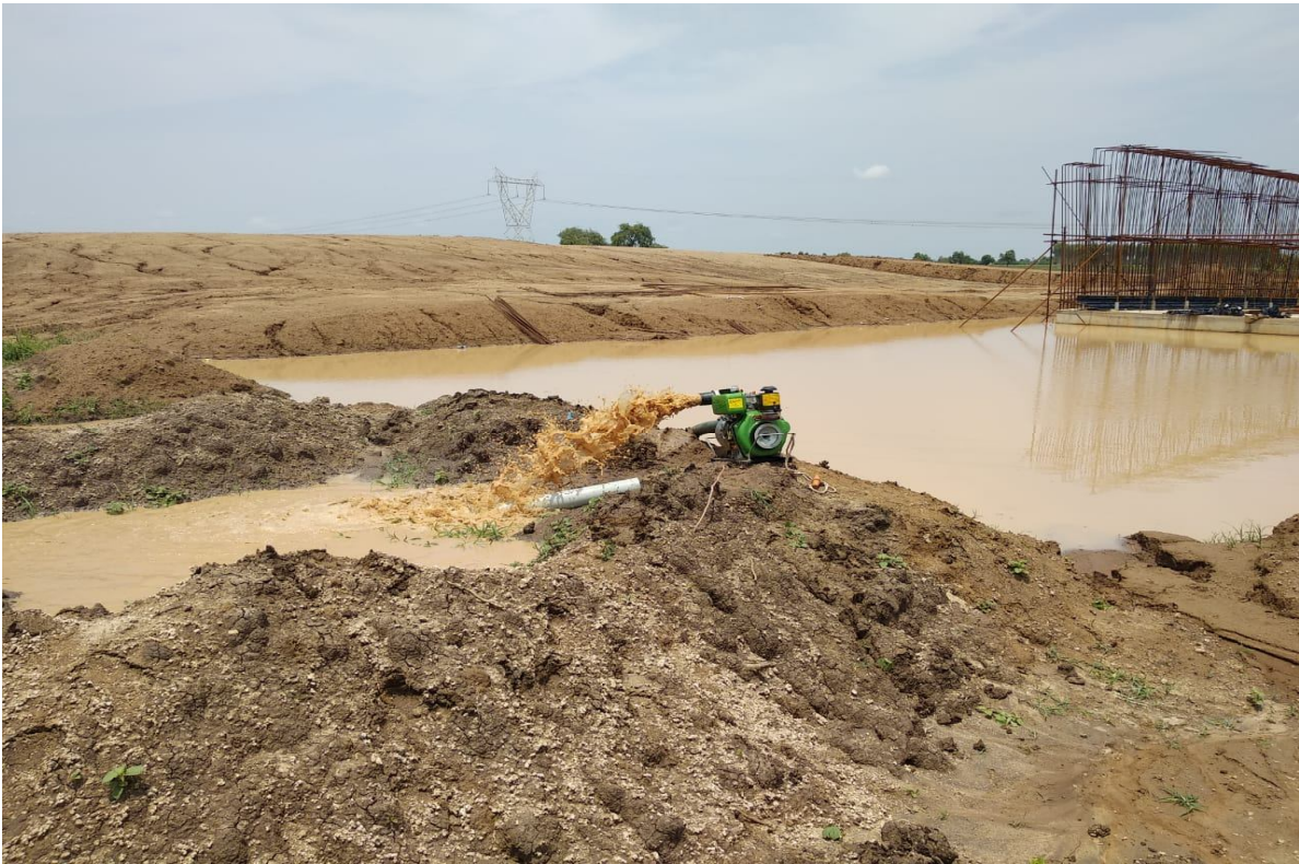
CH.303+220 PUP Dewatering
