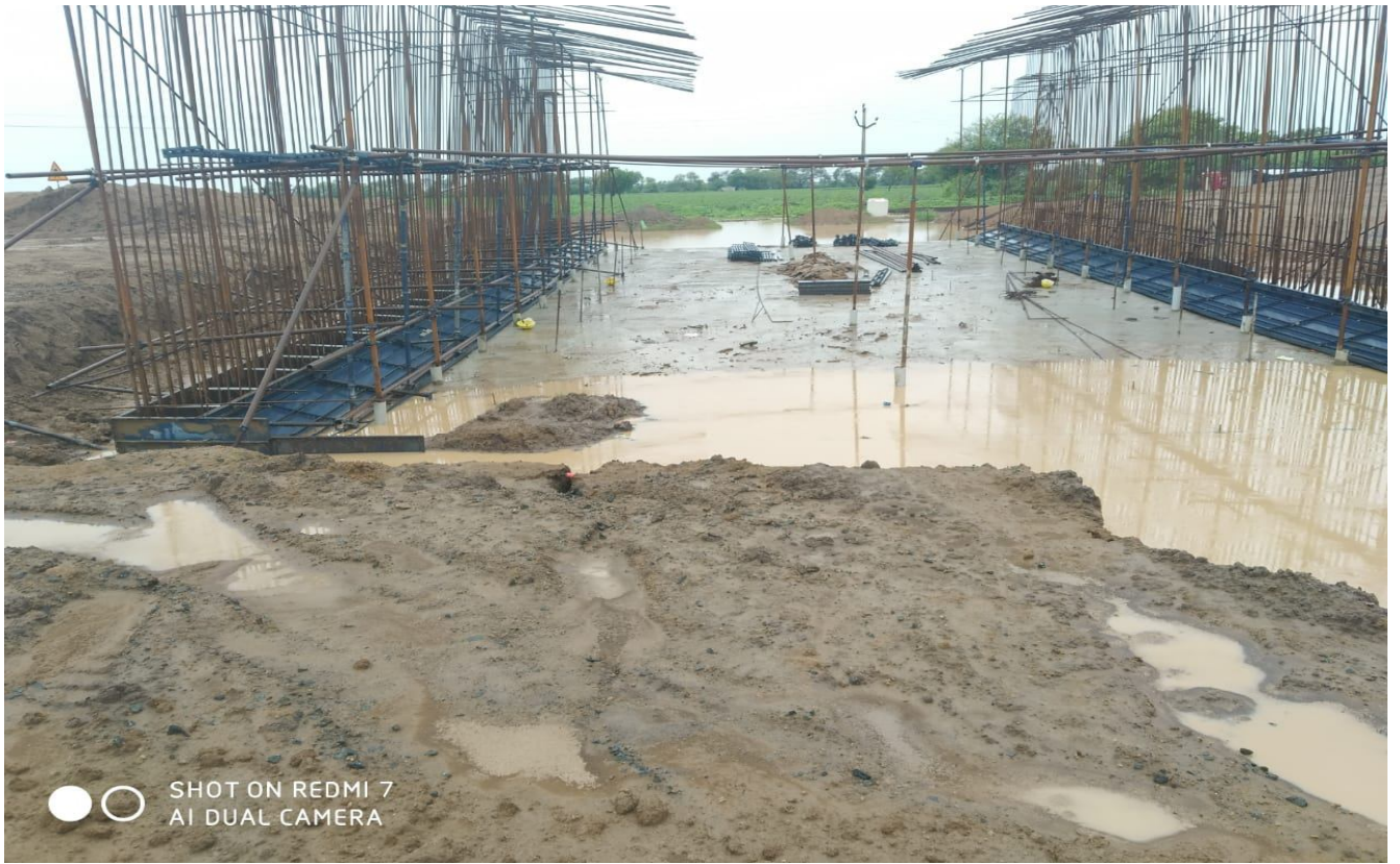
CH.311+650 PUP wall reinforcement
