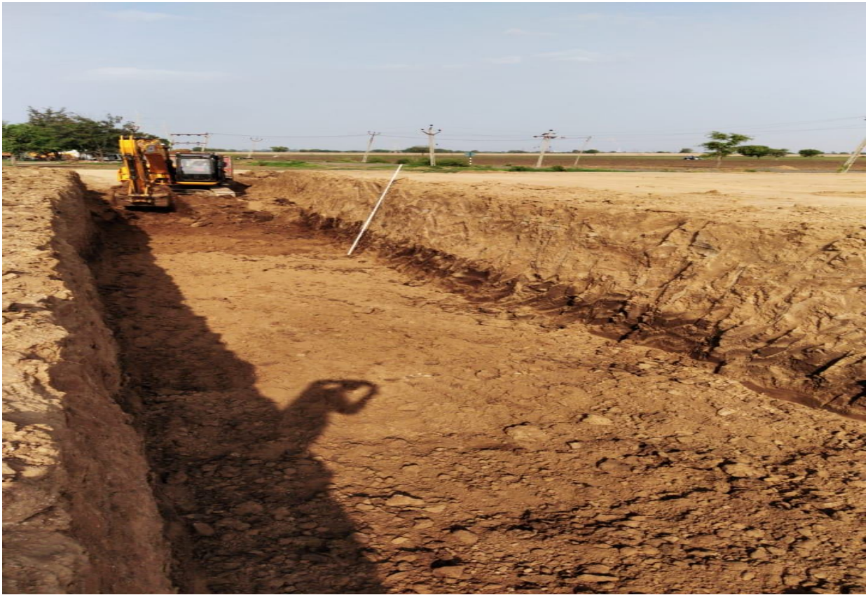
CH.295+585 Box Culvert Excavation work In Progress
