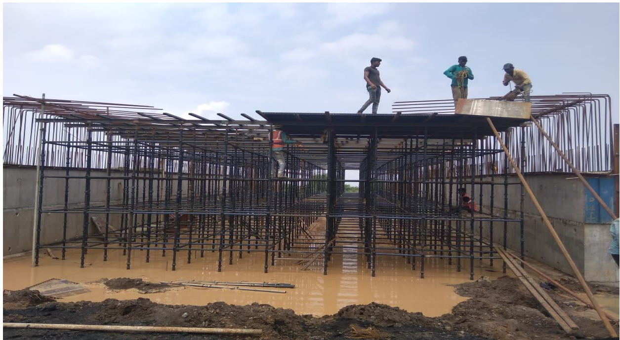
CH298+380 PUP Slab reinforcement work in progress
