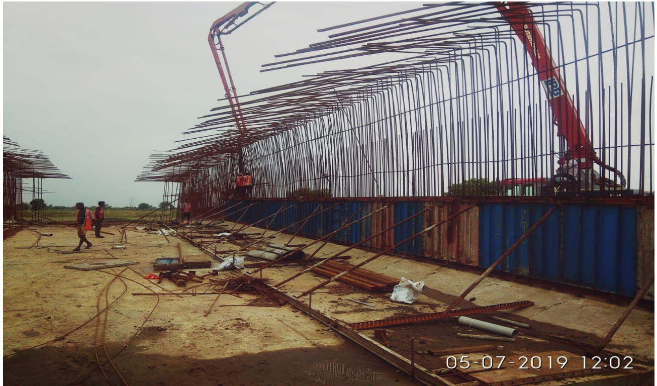
CH.297+900 PUP Wall Concreting
