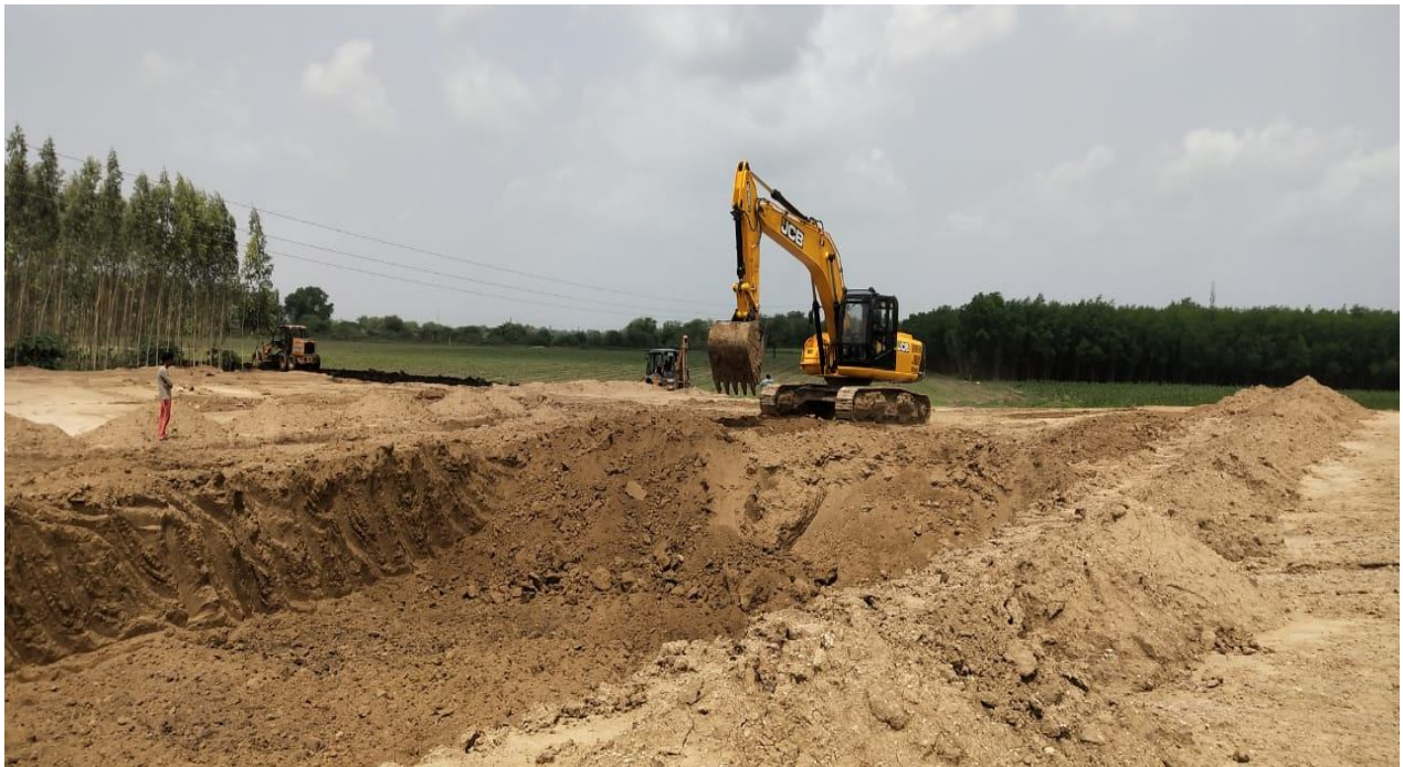
CH.310+480 PUP Excavation
