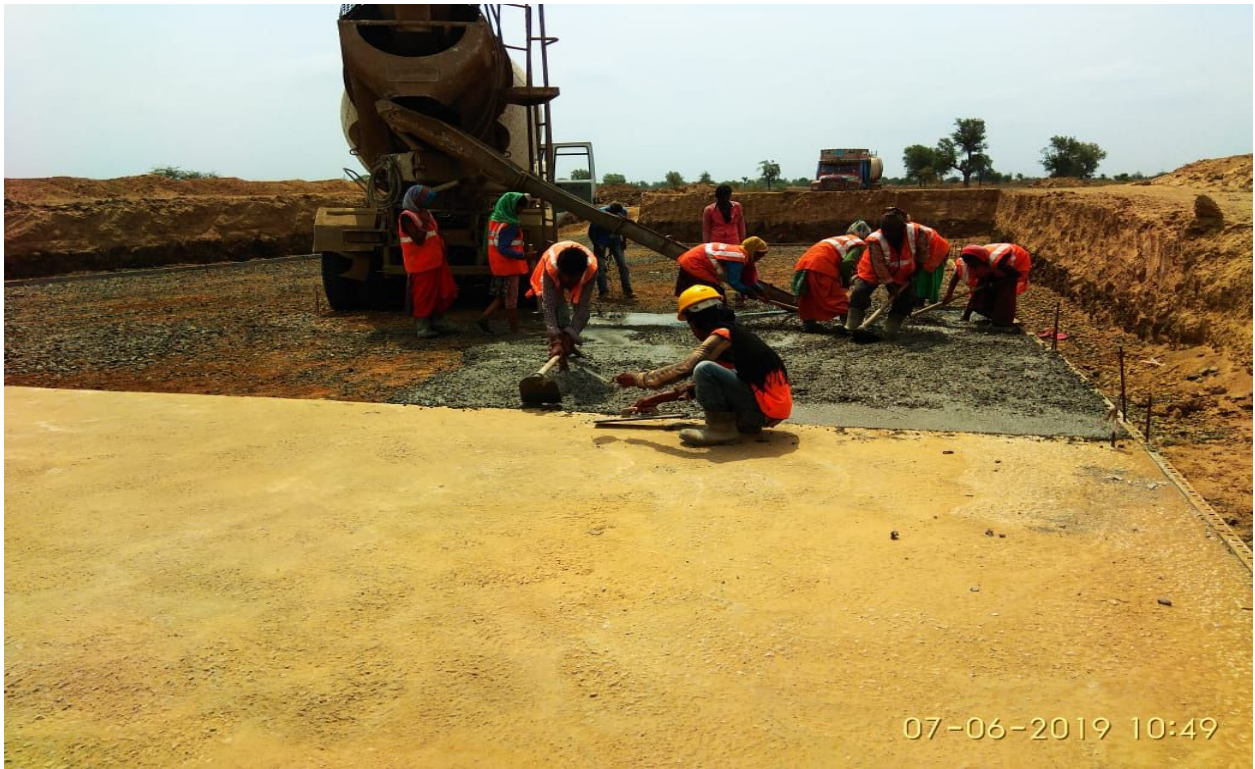
CH.305+850 PUP PCC Laying (RHS)
