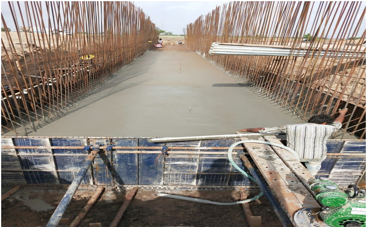
CH.300+148 Box Culvert Raft Concreting
