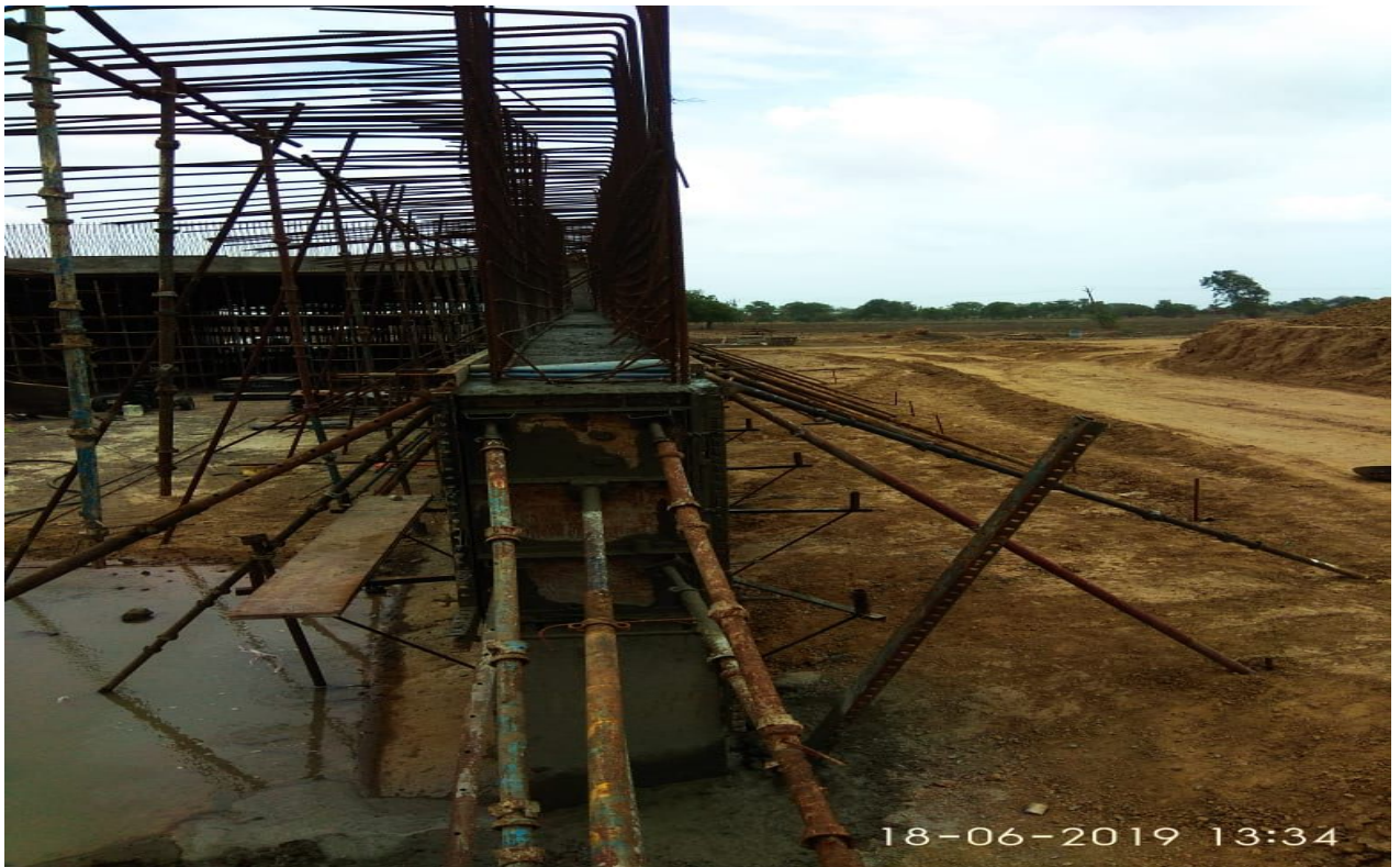
CH.305+058 PUP Wall Concreting
