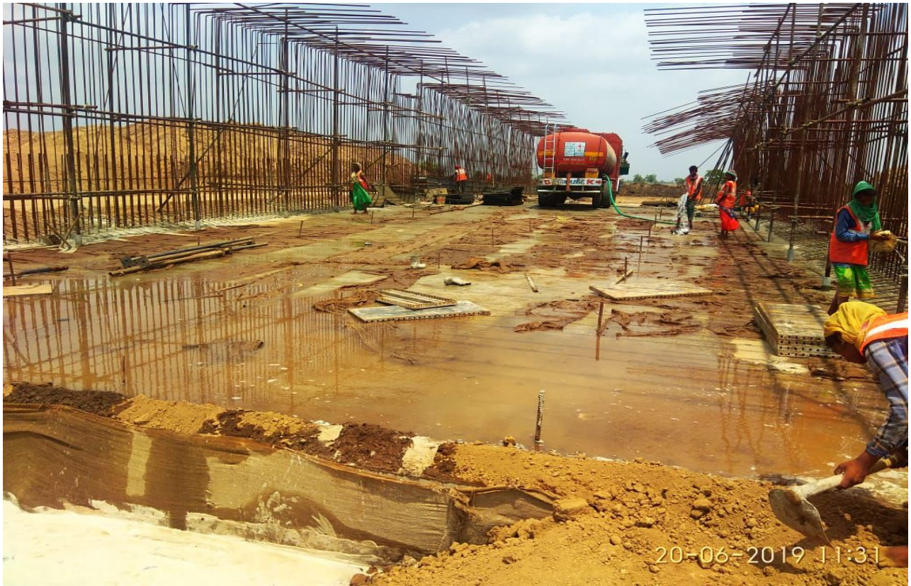
CH.305+058 Raft Curing
