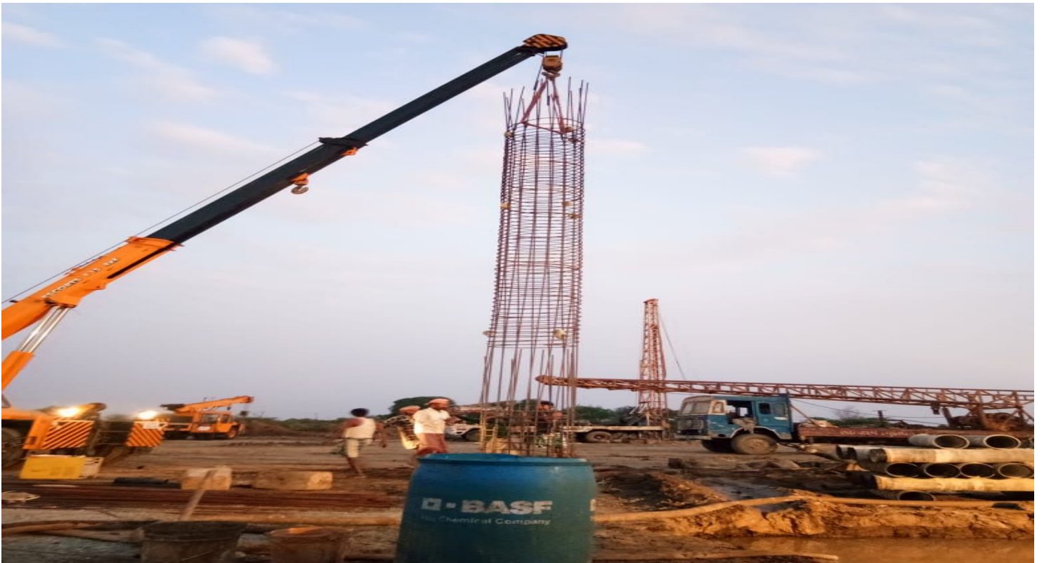
■ ROB Piling Work
