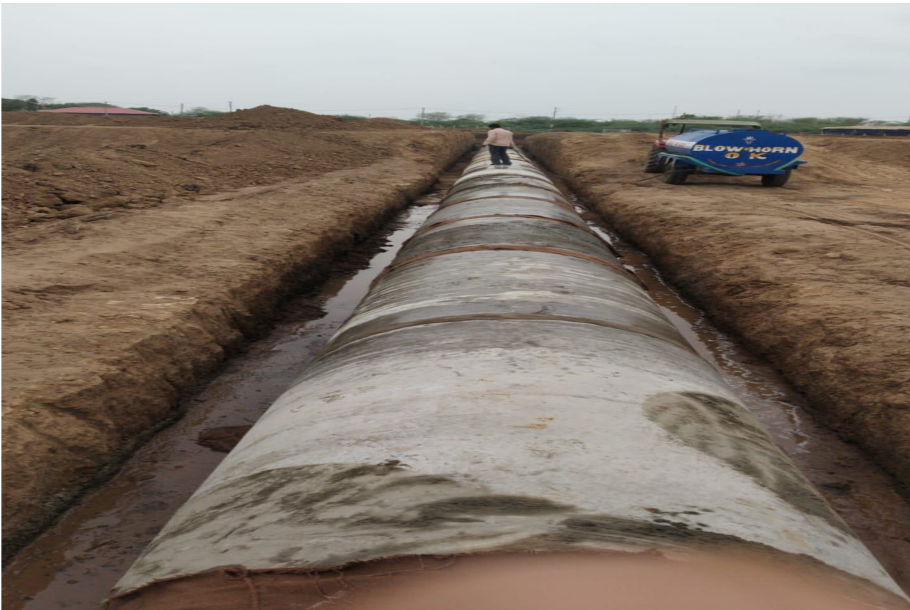
CH.296+720 Pipe Laying
