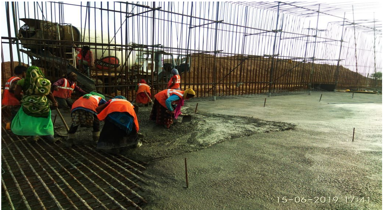
CH.305+058 PUP Raft Concreting
