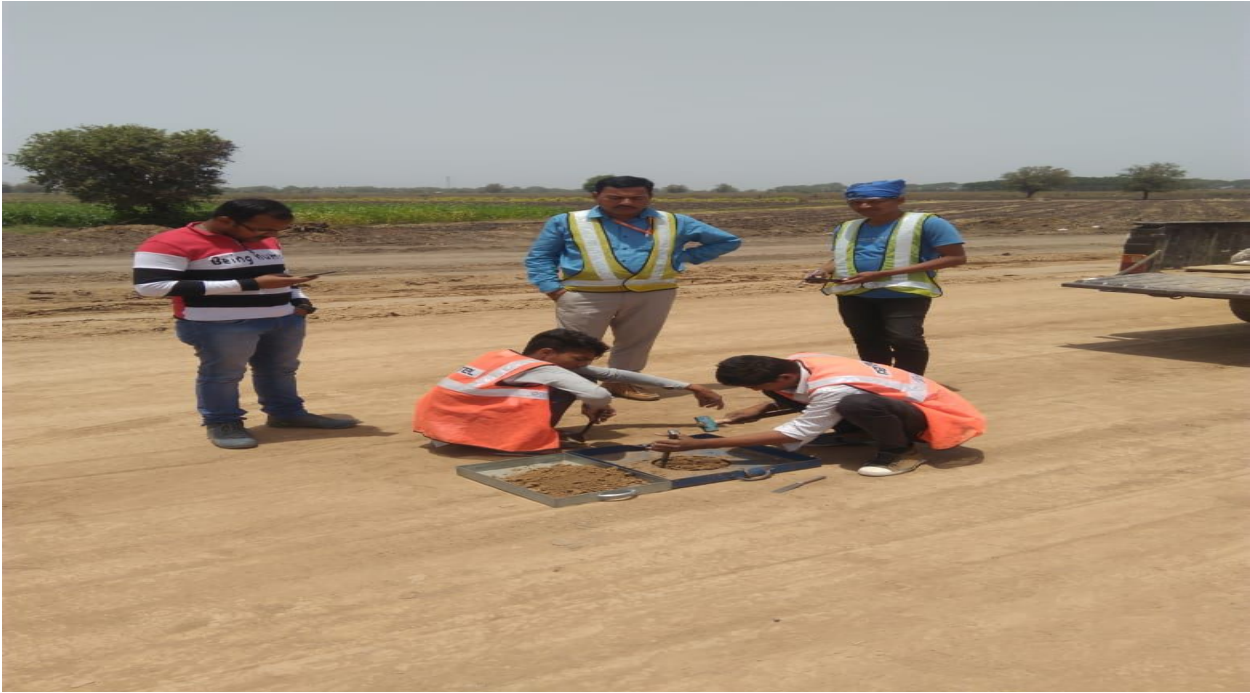
Checking of FDD of Embankment 11 th Layer @ CH.311+070
