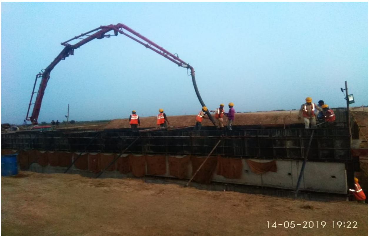
Slab Concreting of Box Culvert @ CH.305+437
