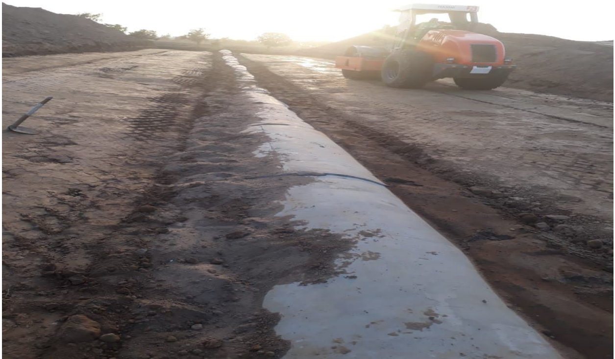
Backfilling of Pipe Culvert @ CH.298+819
