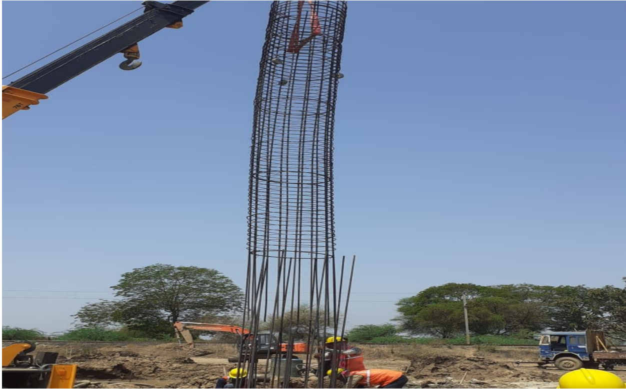
Piling Work of MJB @ CH.302+713
