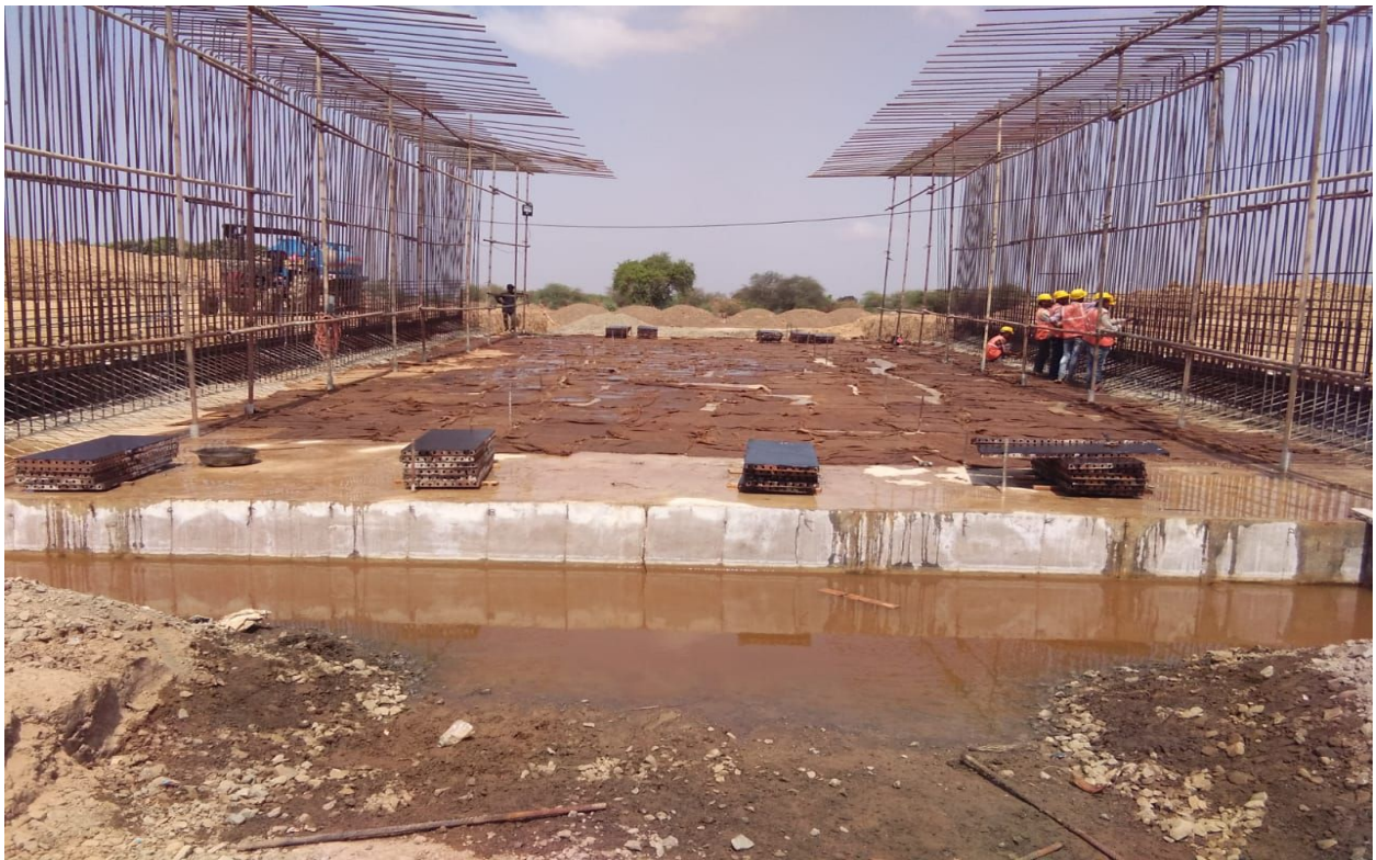
Curing of Raft of PUP @ CH.304+170
