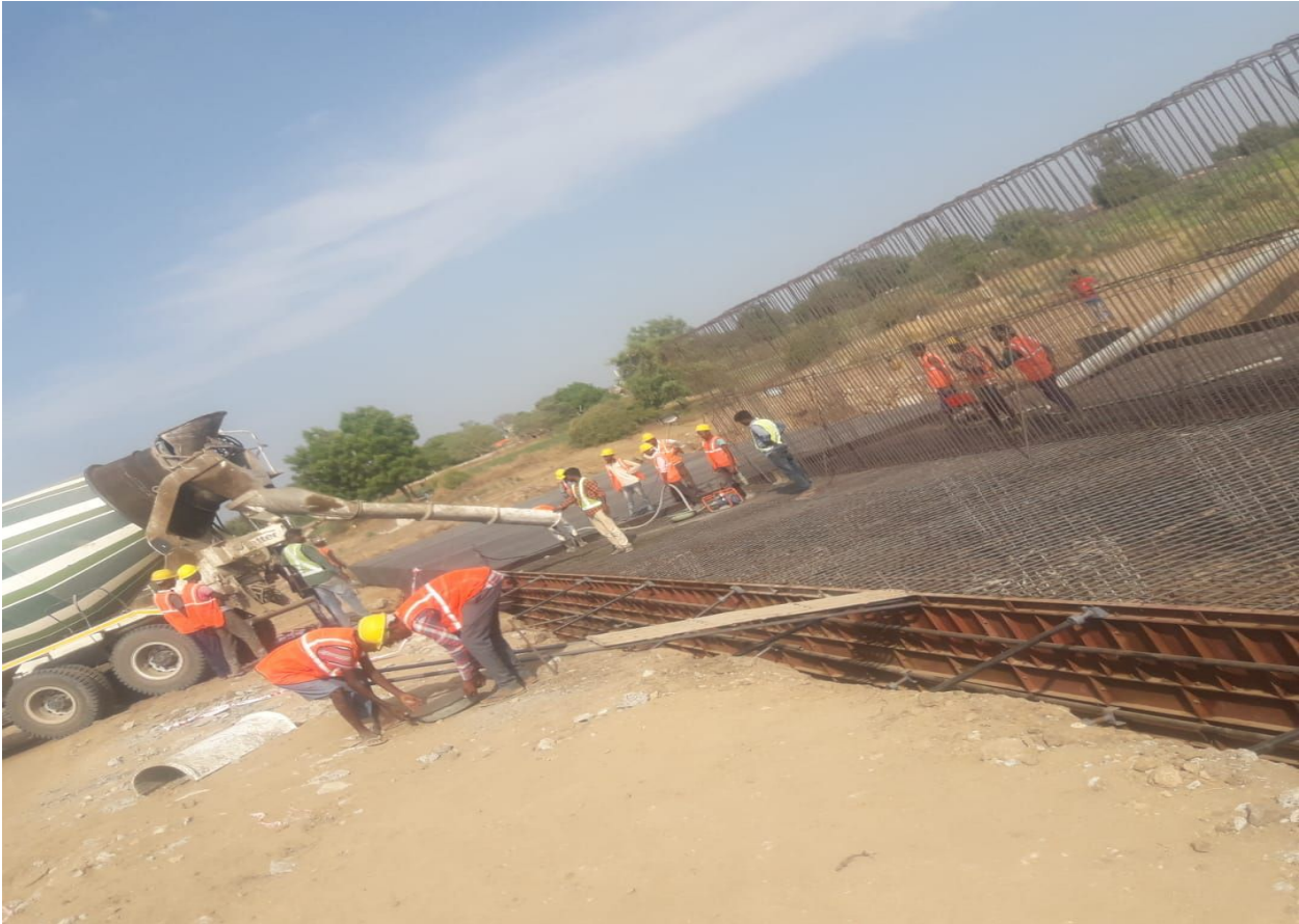
Raft Concreting of PUP @ CH.304+170
