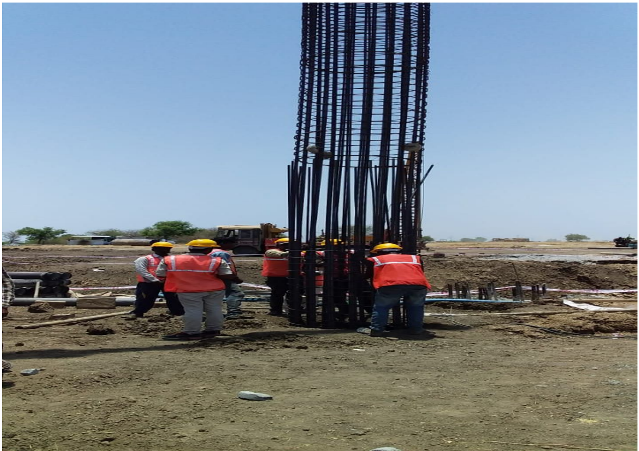
Piling Work of ROB @ CH.293+014
