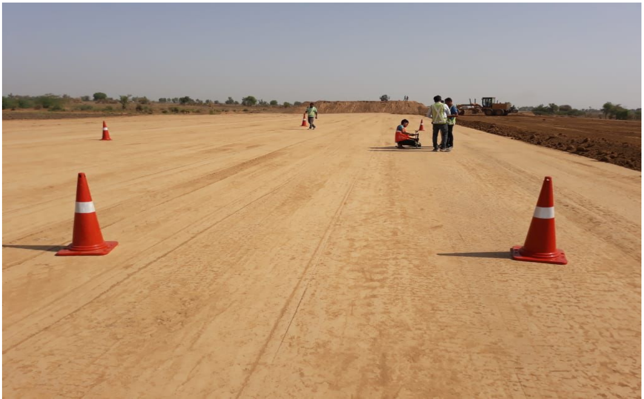
Checking of FDD of Embankment 9 th Layer @ CH.303+225
