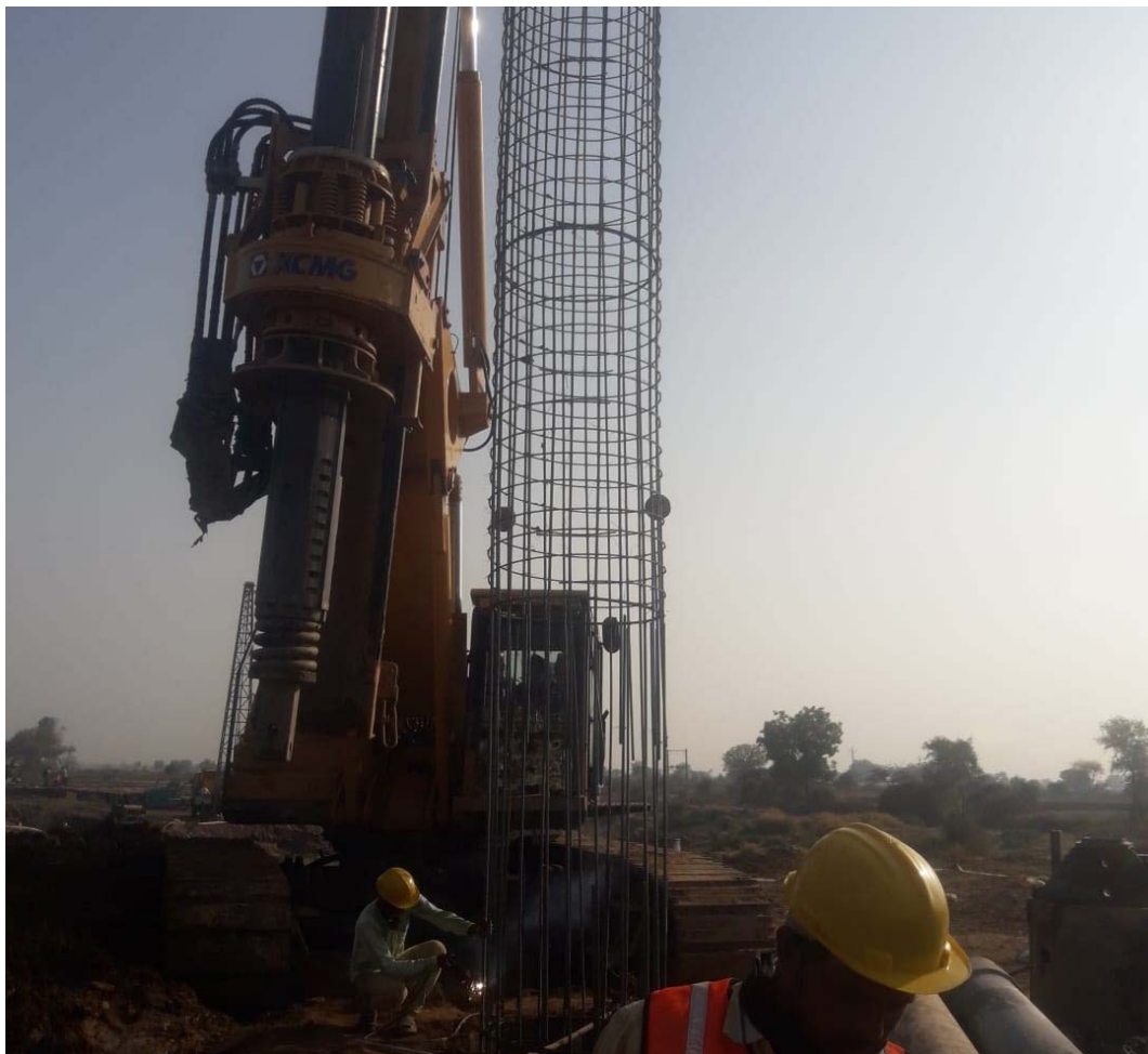
Cage lowering of Pile at Minor Bridge 307+731
