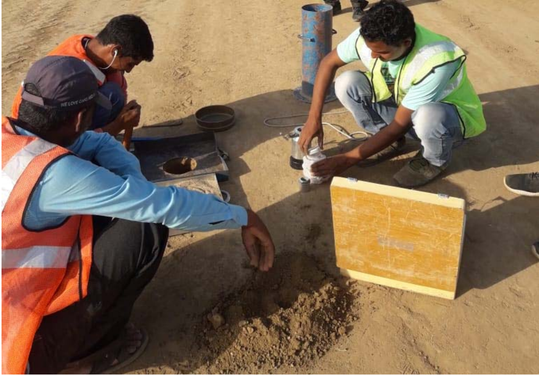
Embankment FDD Checking at 297+000 LHS.
