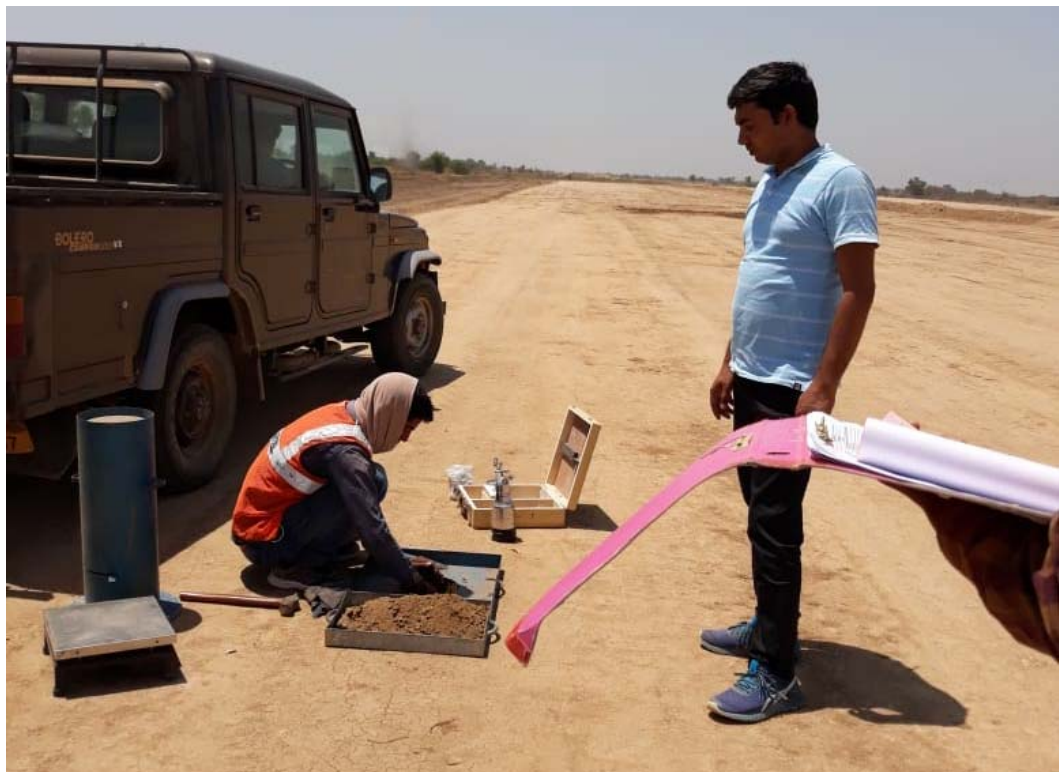
Embankment FDD Checking at 306+700 RHS.
