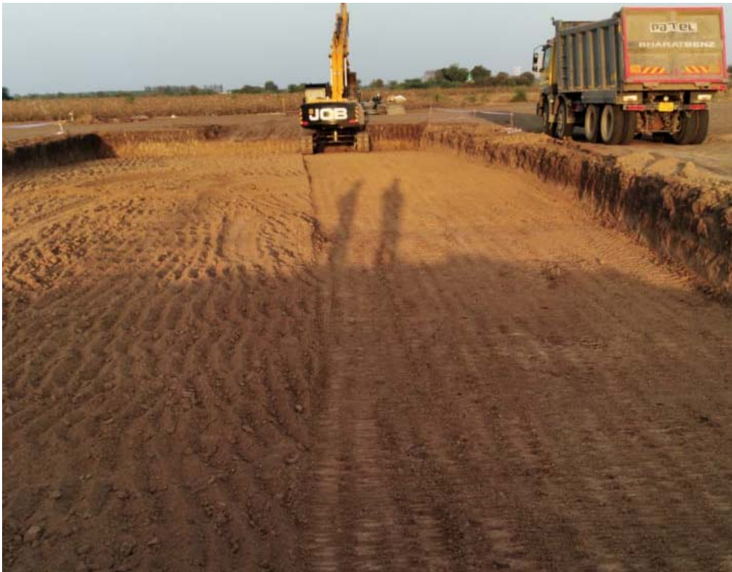
Excavation of PUP at 297+900
