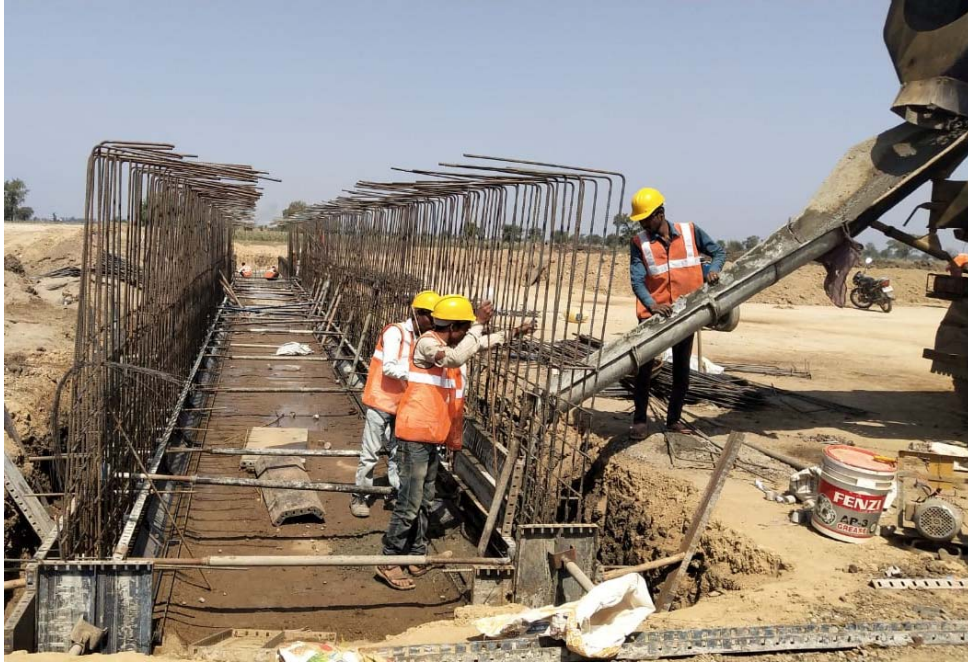
Concrete work of Haunch Box culvert at 305+437
