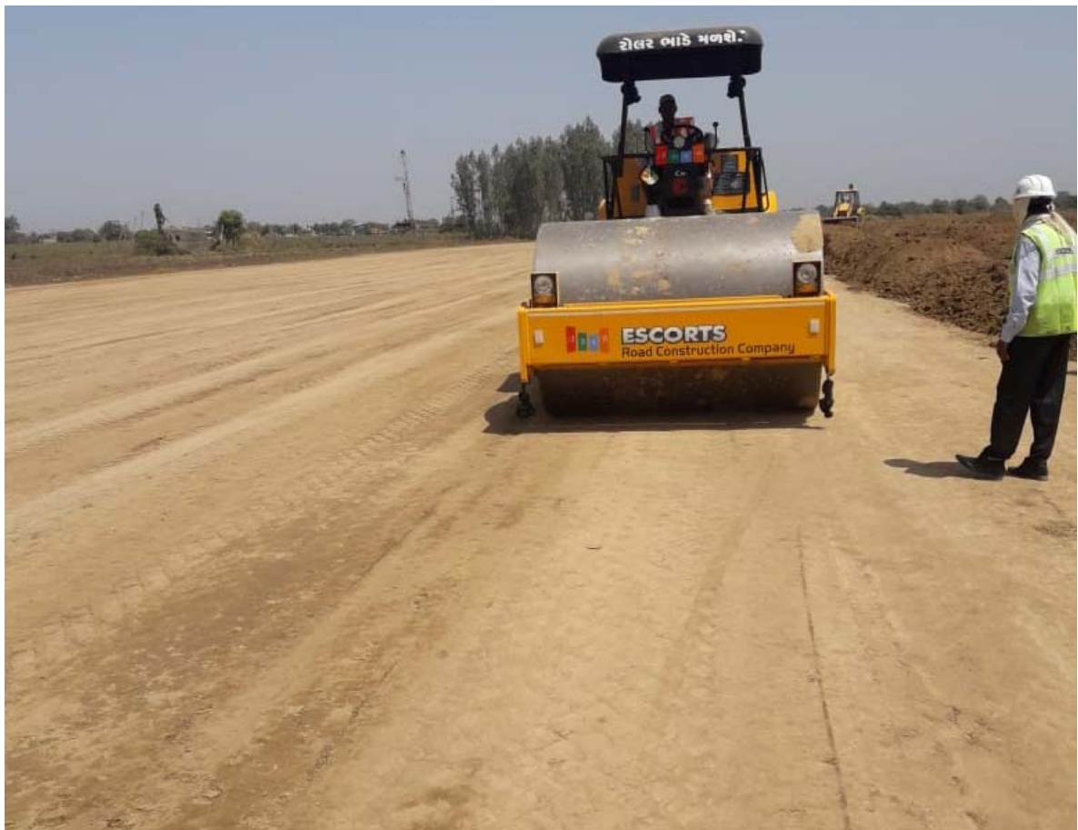
Embankment Preparation at 309+140
