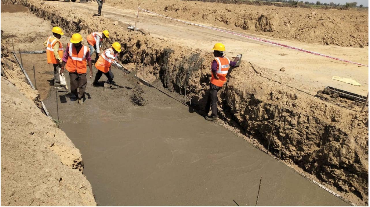
PCC work of Box Culvert at 304+170
