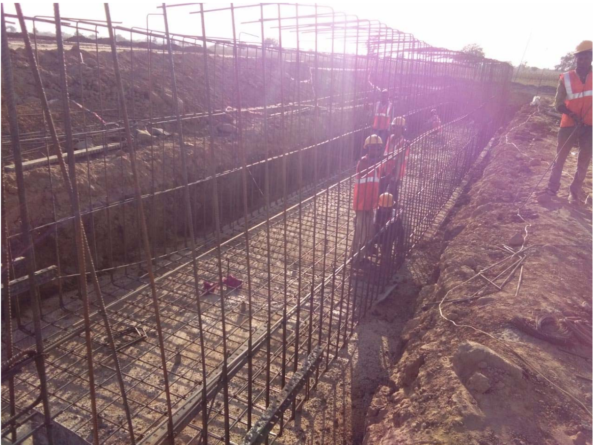
Concrete work of raft PUP at 304+170
