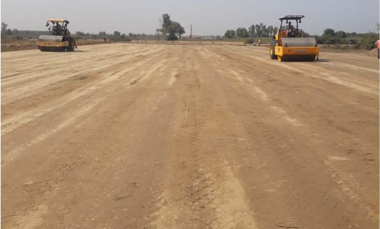
Embankment Preparation at 296+300
