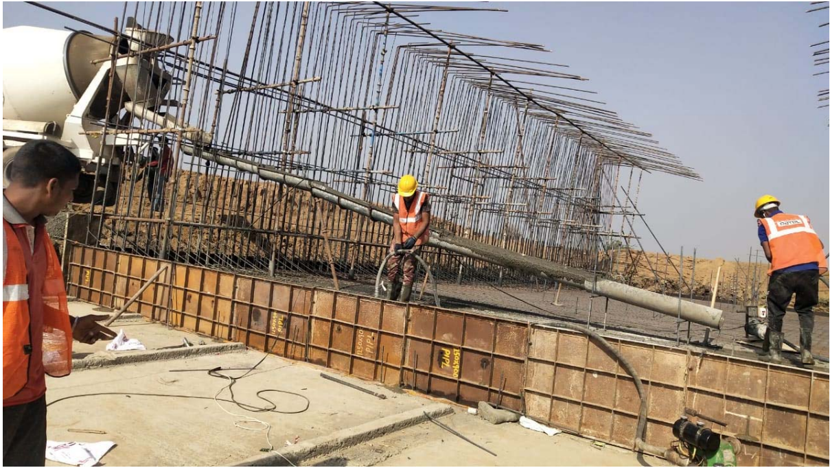
Concrete work of raft PUP at 304+170
