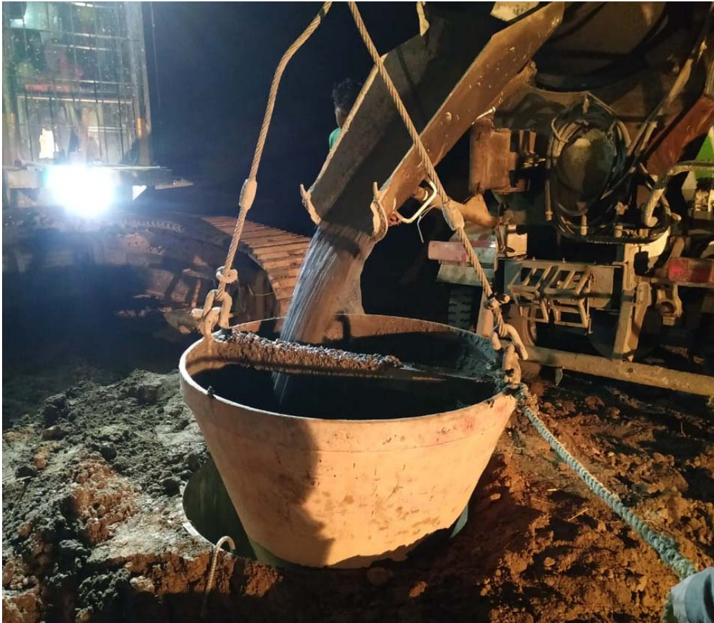
Concrete pouring of Pile at Major Bridge 321+253
