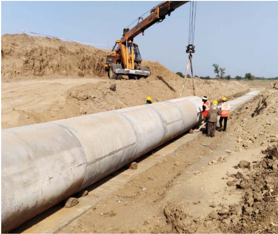
Pipe Laying of HPC at 303+608
