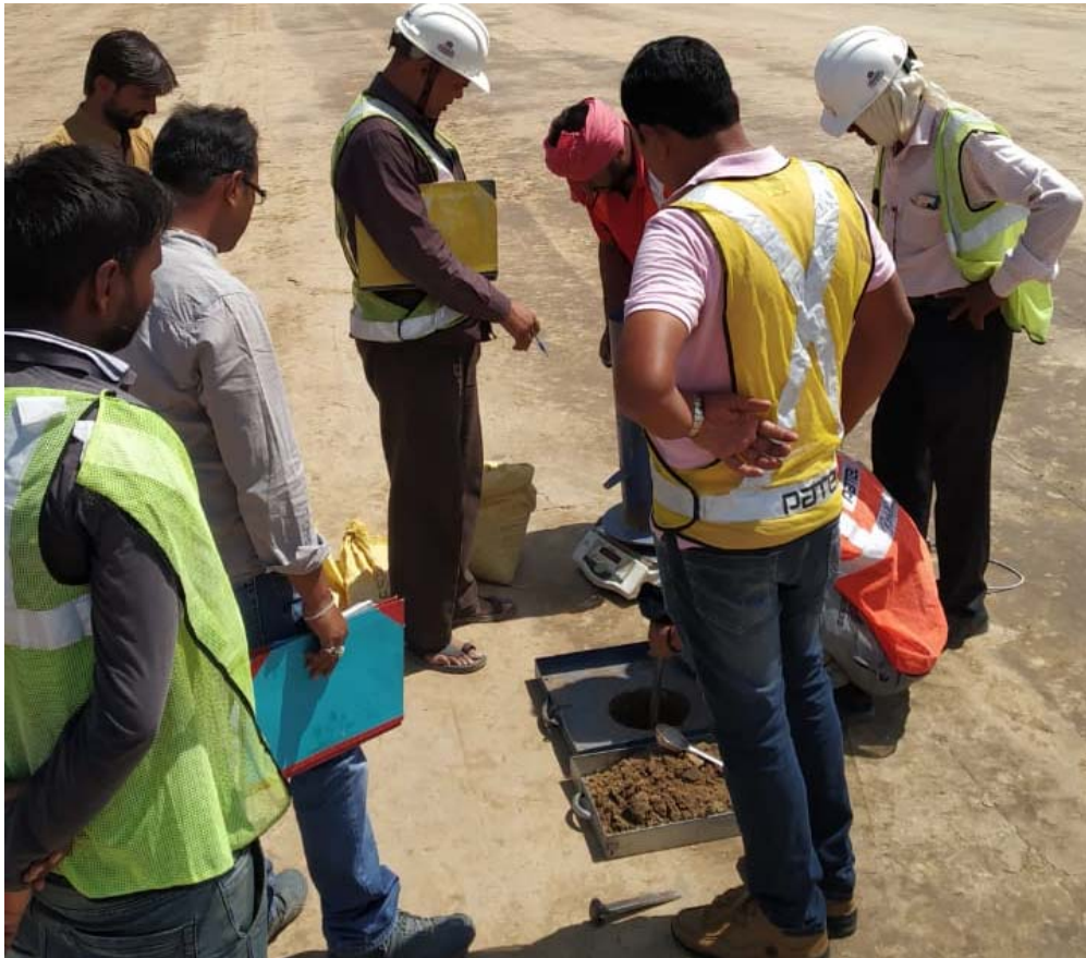
Embankment FDD Checking at 322+100 RHS.
