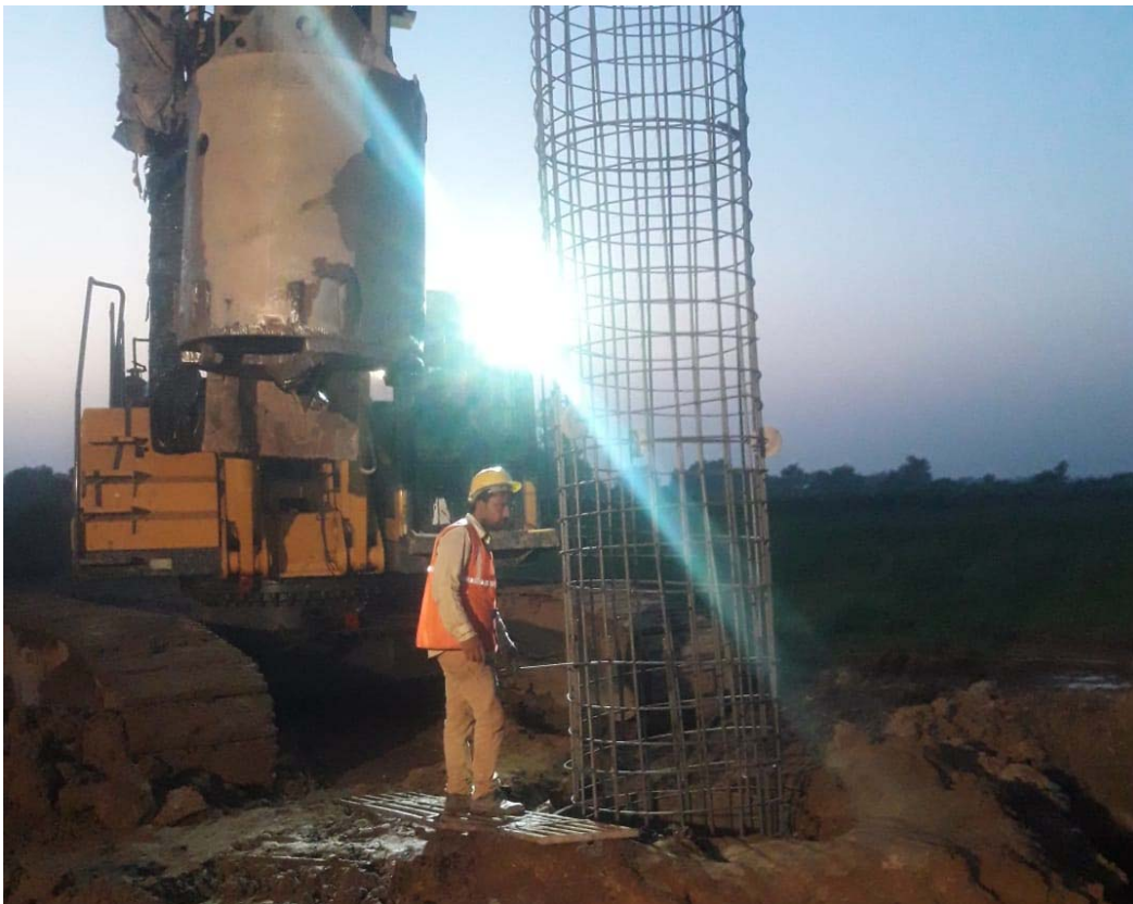
Cage lowering of Pile at Major Bridge 321+253
