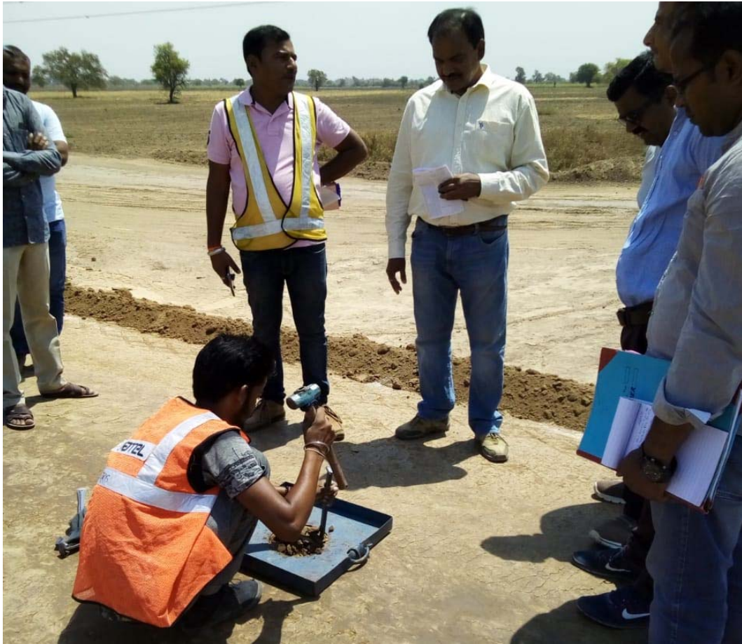
Embankment FDD Checking at 311+670 RHS.
