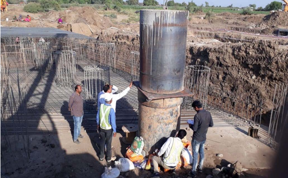
Dynamic Pile Load Test at Major Bridge 321+253
