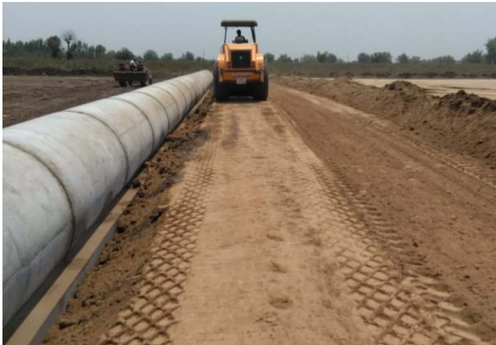
Back filling of HPC at 311+329
