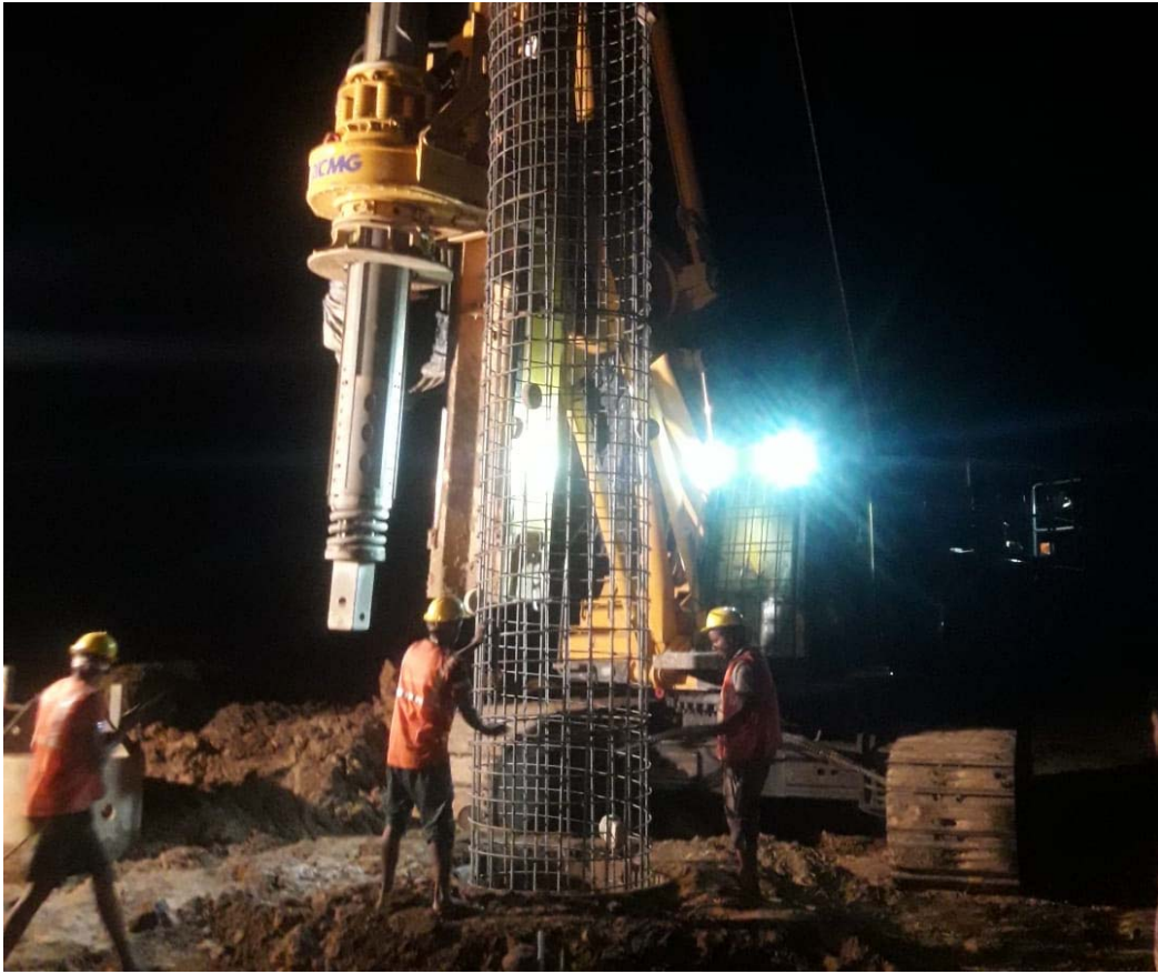
Cage lowering of Pile at Major Bridge 302+713
