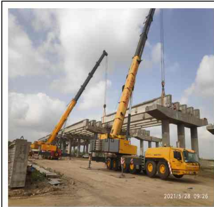
CH 293+014 Girder launching work in progress
