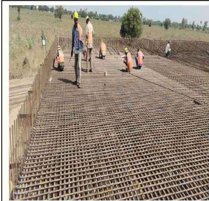
CH 310+717 MNB TOP slab reinforcement work in progress
