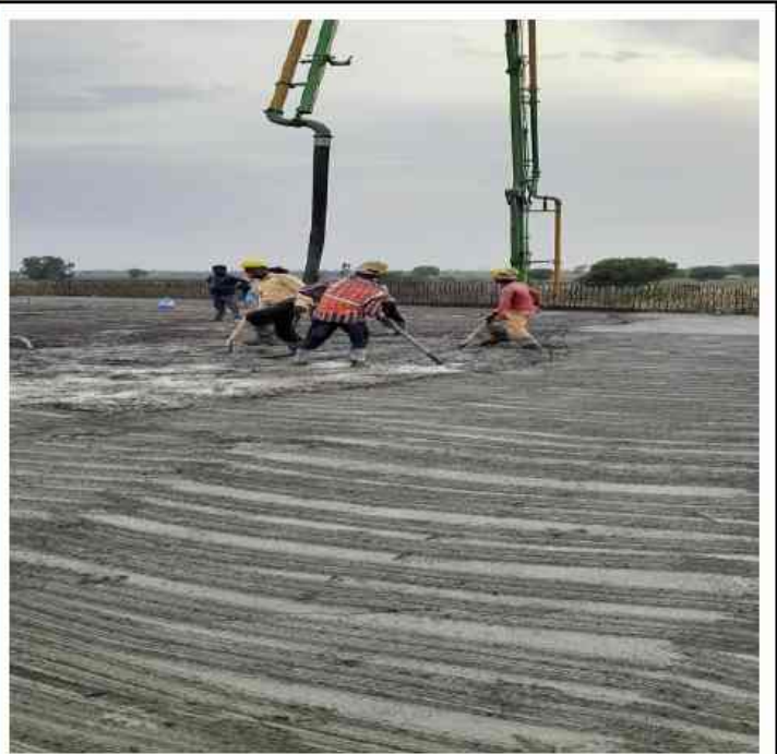
CH 321+253 MJB A1P1 Deck slab pouring work in progress
