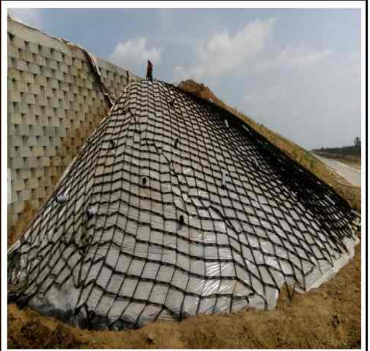
CH 305+058 A1-A2 – Quarter conning slope protection concrete work in progress
