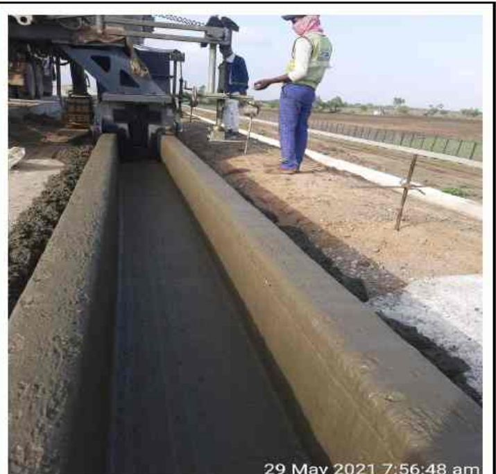
CH 311+300 U drain work in progress
