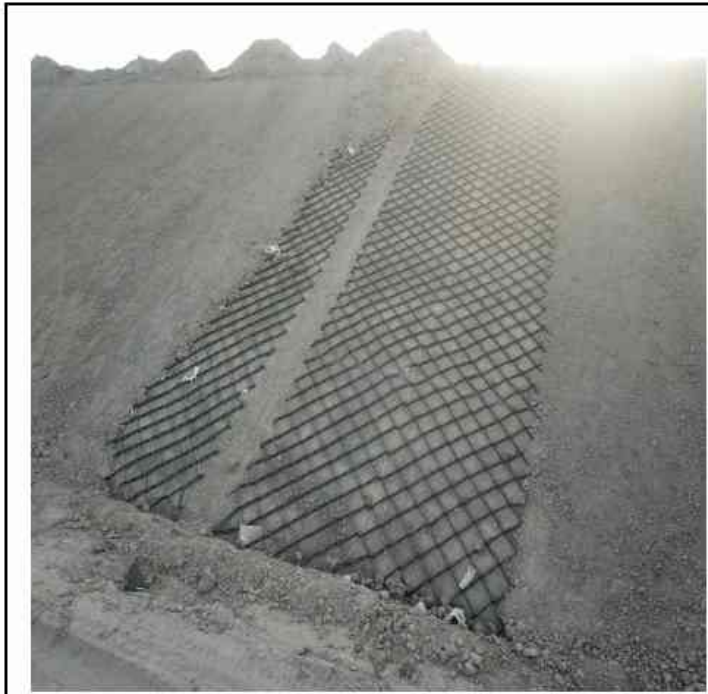
Slope Protection with Geocell & Vetiver grass (Embankment height > 6m)
