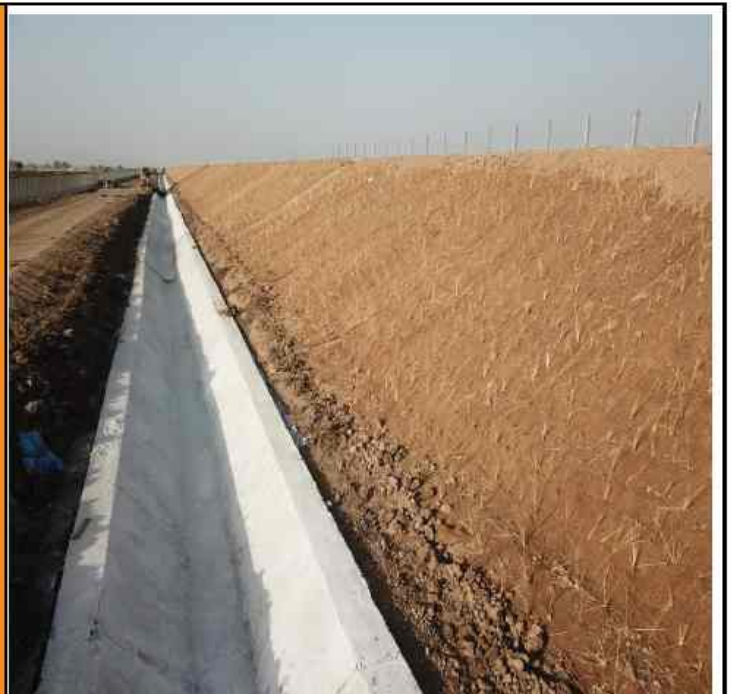
Slope Protection with Coir Mat & Vetiver grass (Embankment height < 6m)
