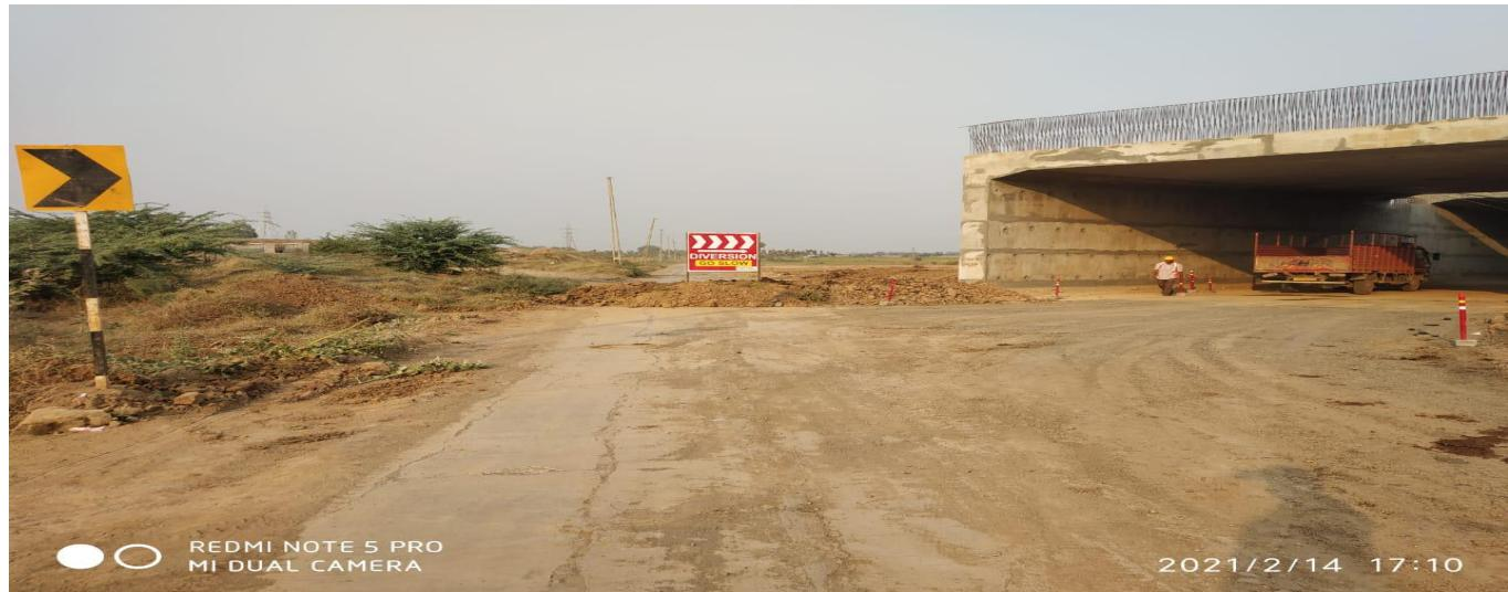
**Provided Safety barricading at excavation area**
