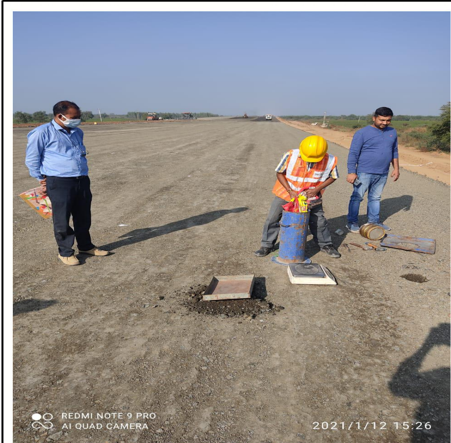
CH 313+310 FDD Checking of GSB top by IE RHS
