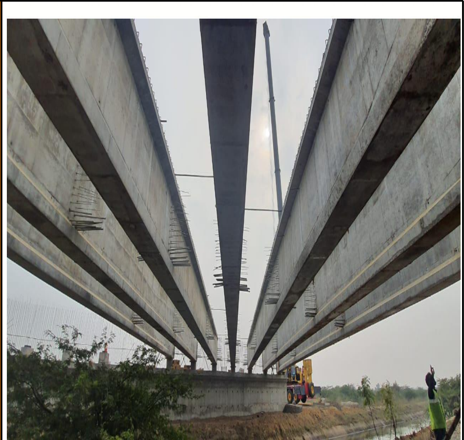
CH 307+733 MNB Girders launched
