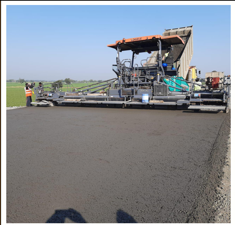
CH 302+990 TO 303+170 DLC laying work in progress
