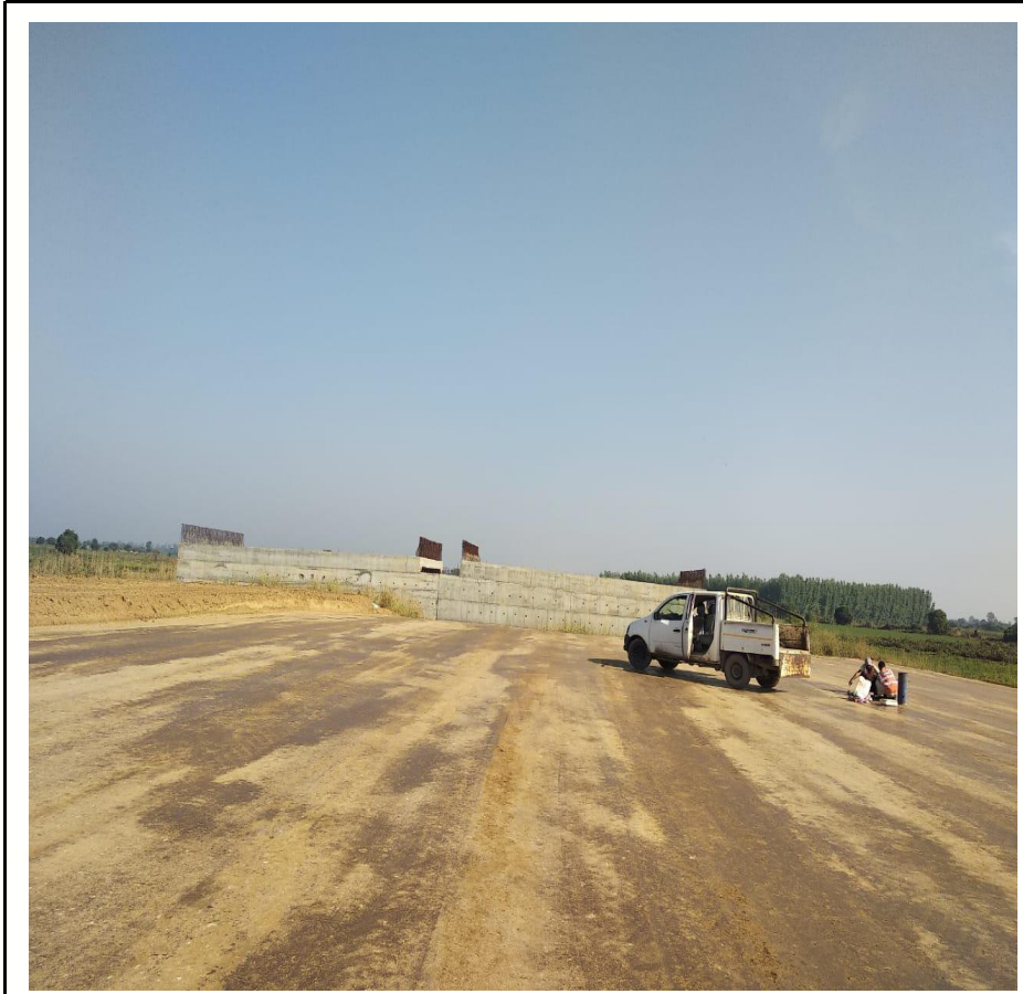
CH 319+500 TO 319+550 FDD checking of EMB 12 th layer
