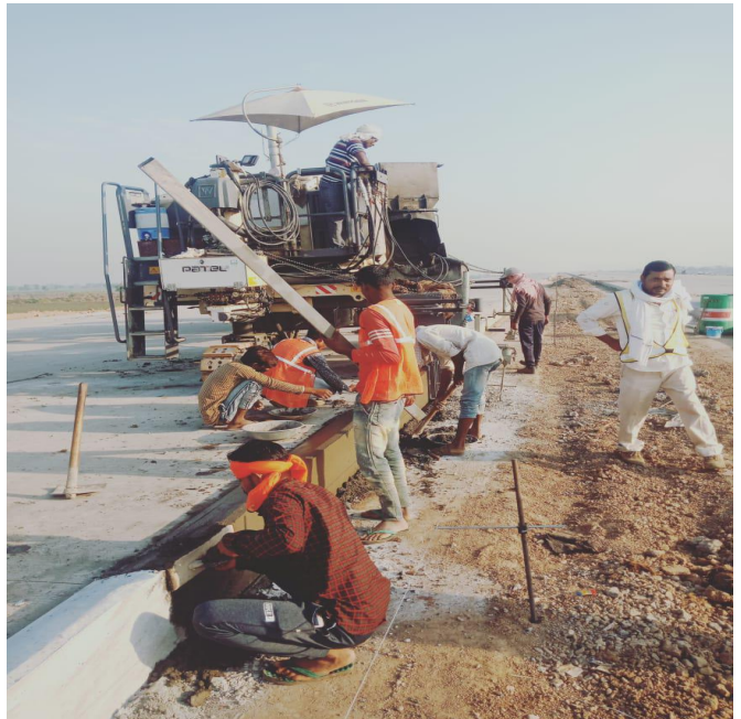
Retaining wall shuttering work CH 322+610 Ch-318+870 MJB (RHS)
