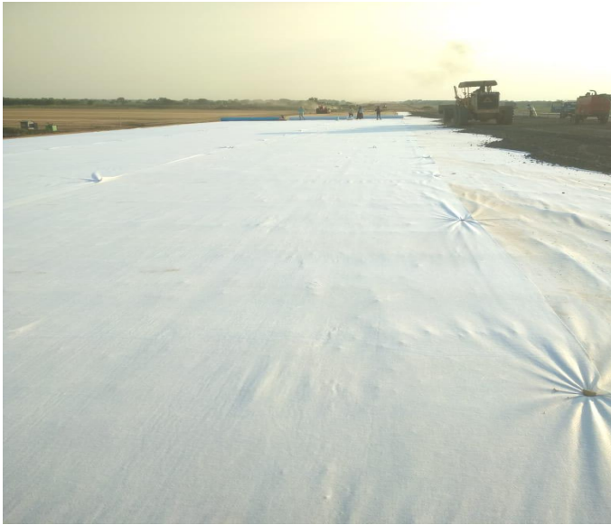
Geo textiles laying work in progress CH 318+140 - 318+340(RHS)
