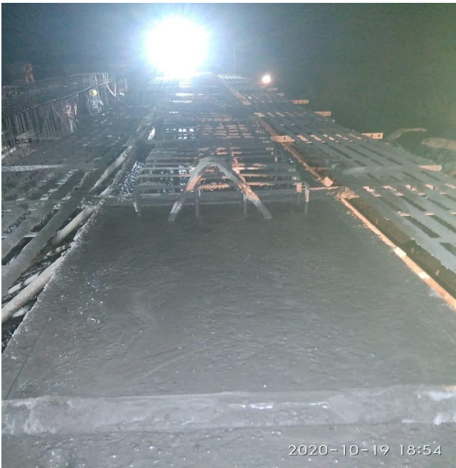
P3-P4 PSC Girder no. 7 concreting work in progress CH 293+014 ROB
