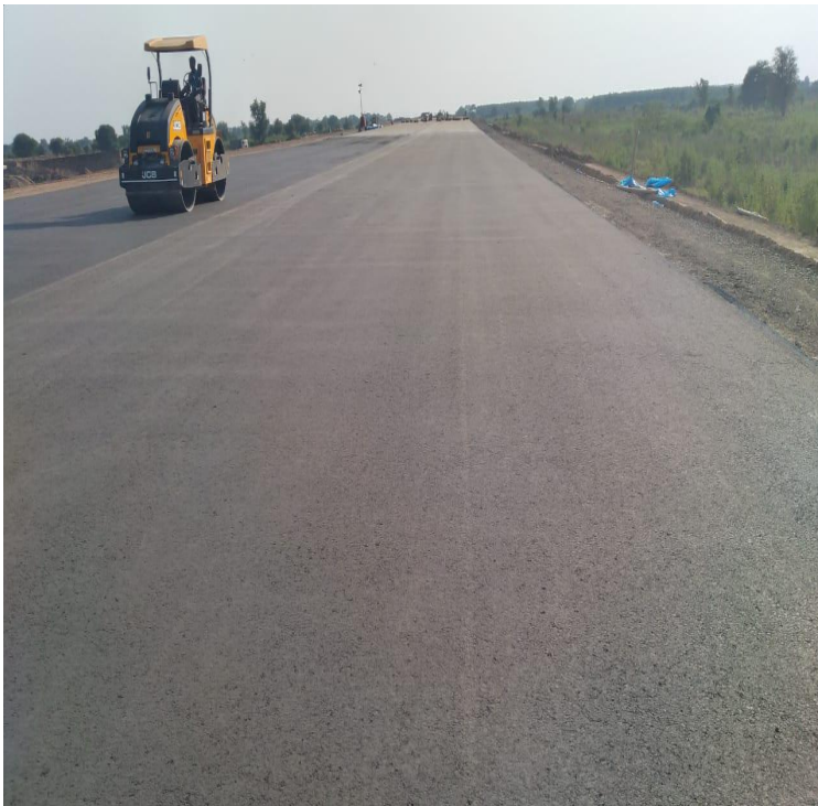
DLC laying work in progress 317+855 - 318+000 (LHS)
