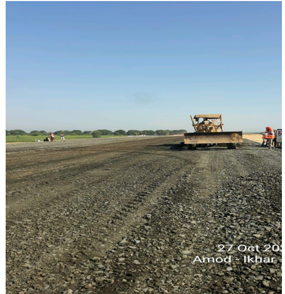
GSB top work in progress CH 318+200 - 318+330(LHS)
