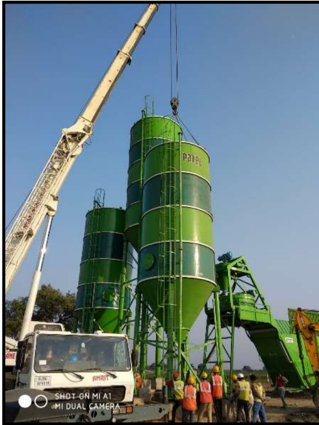
Concrete Batching Plant Setup at Camp (60,120 CUM/Hr. Capacity)
