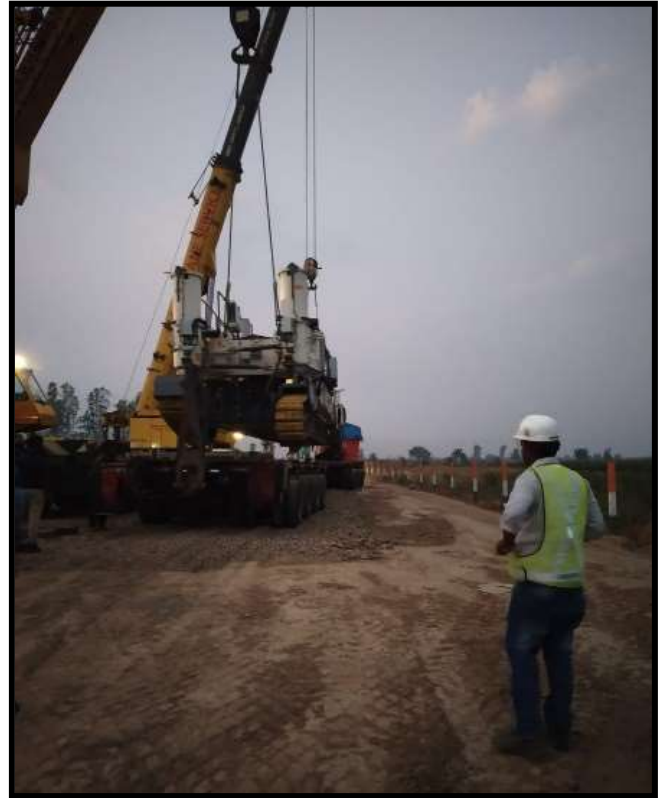
Paver Unloading at camp
