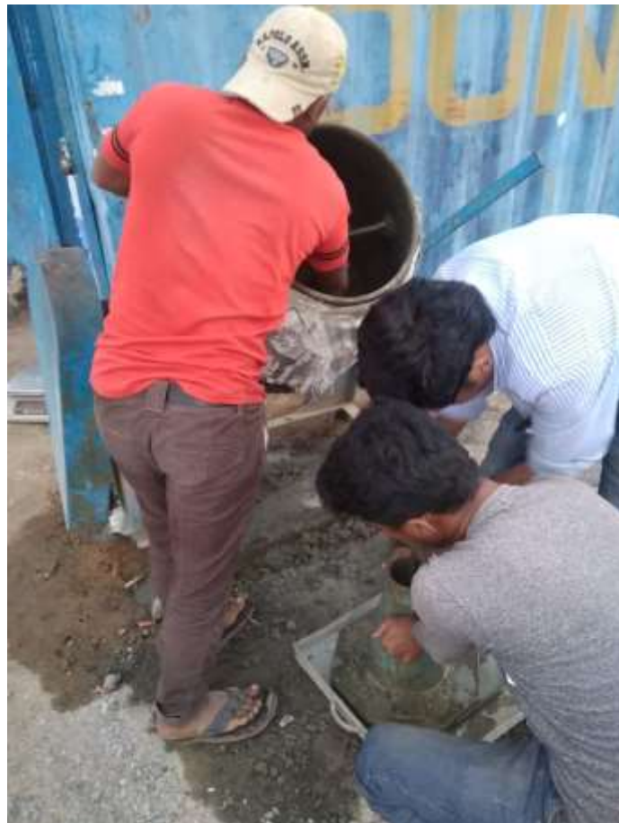
Slum test for trail mix design of M-35 Pile
