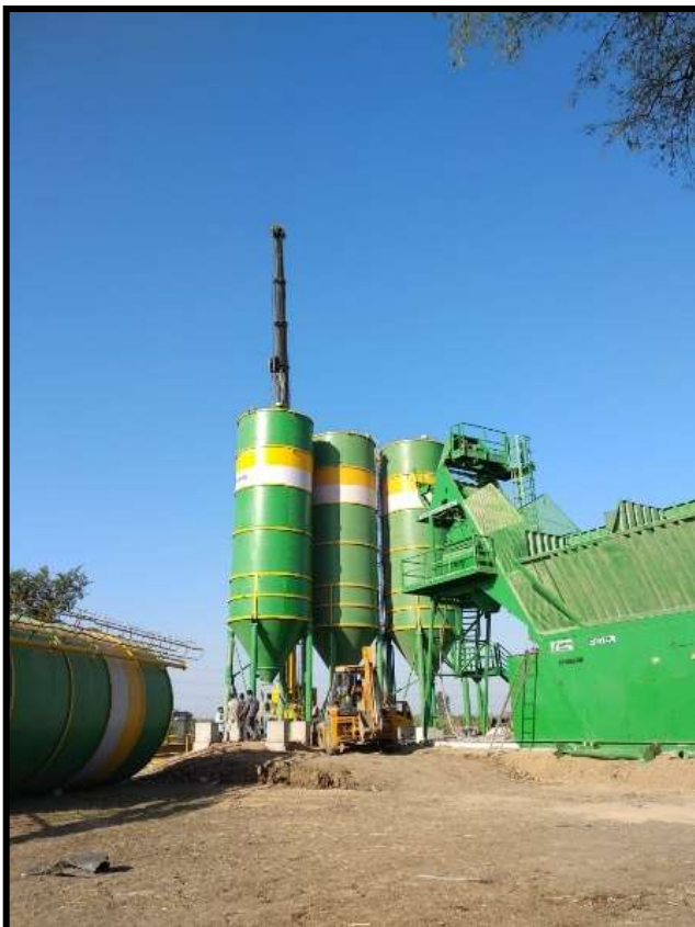
Concrete Batching Plant Setup at Camp (60,120 CUM/Hr. Capacity)
