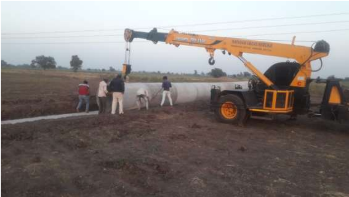
Pipe laying in progress for HPC at ch_311 +969
