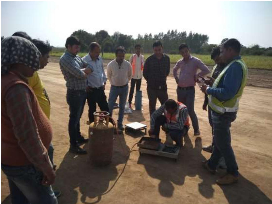
FDD checking Emb 2nd layer Ch. - 294+080 to 294+200 lhs with client
