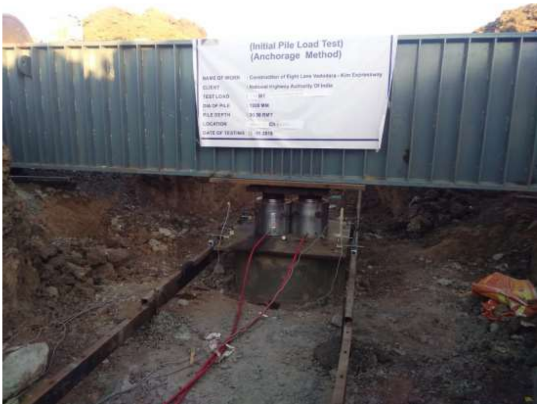
Pile load test @ 321+253 MJB in progress
