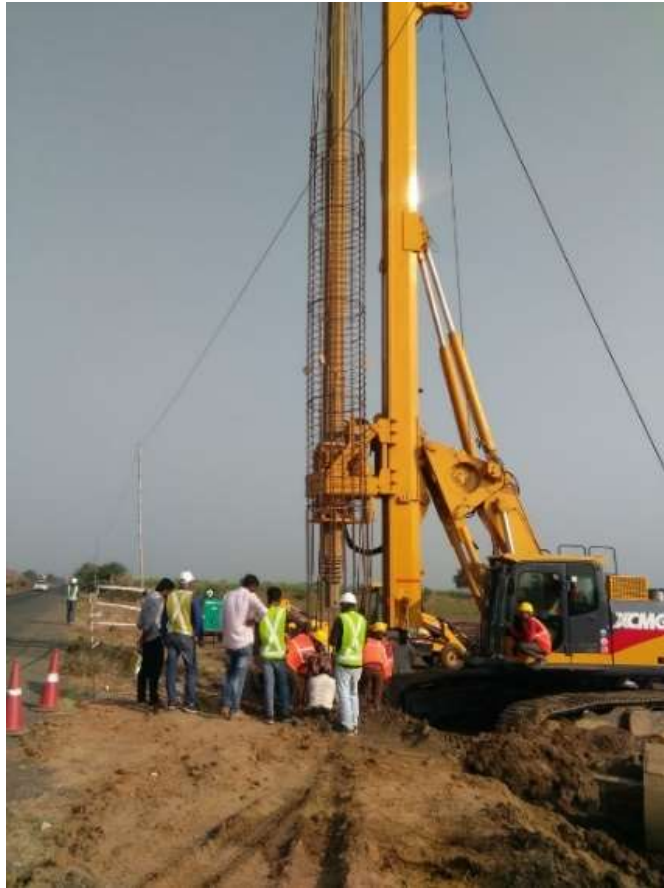
Test pile cage lowering at 299 flyover
