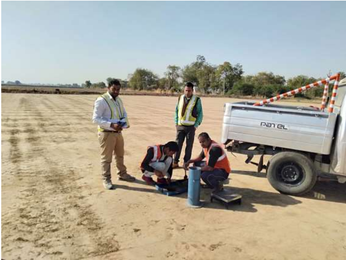
FDD checking Emb 1 st layer Ch. – 314+120 to 314+400 lhs
