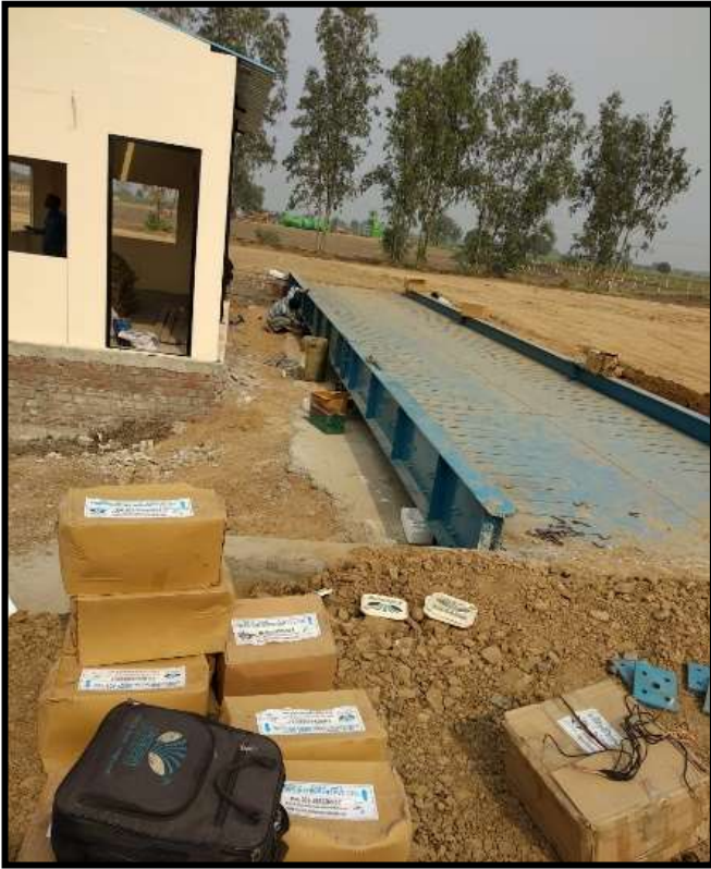
Weighbridge establishment at camp
