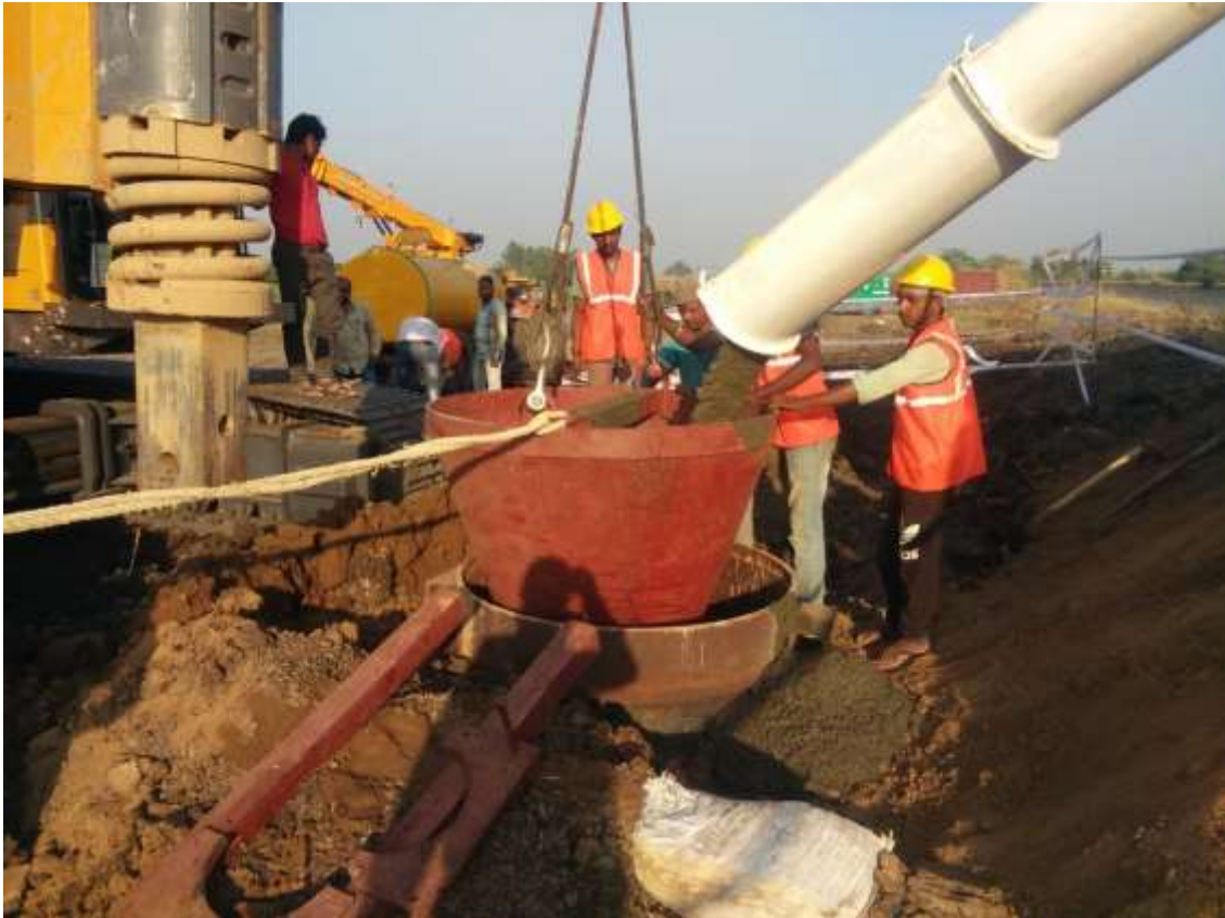
Test pile concreting at 302+ MJB
