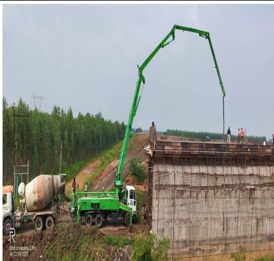
CH 308+550 LVUP Top slab concrete pouring work in progress LVUP LHS
