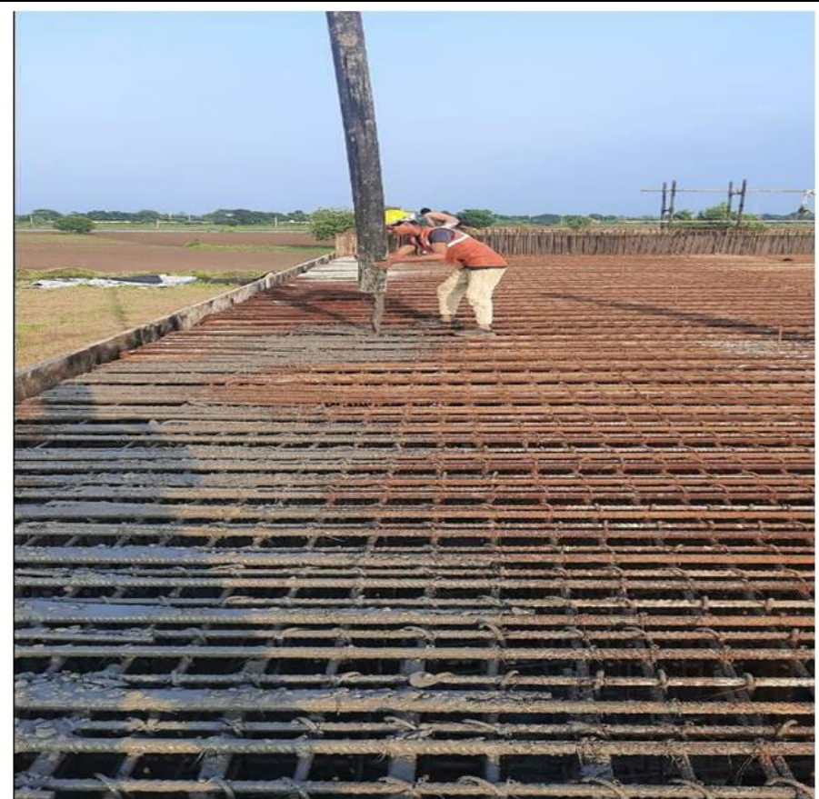
CH 316+960 PUP Top slab concreting work in progress PUP LHS
