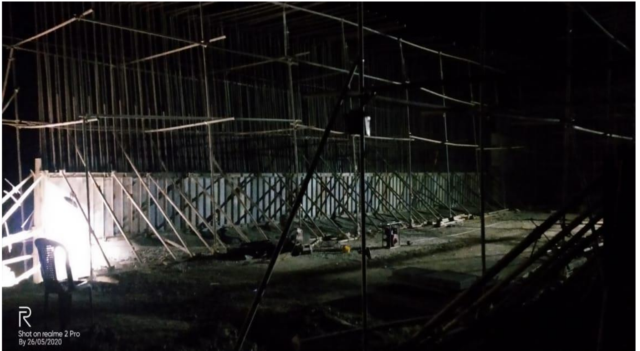
Ch-322+550 pup lhs A1 and A2 first lift casting completed
