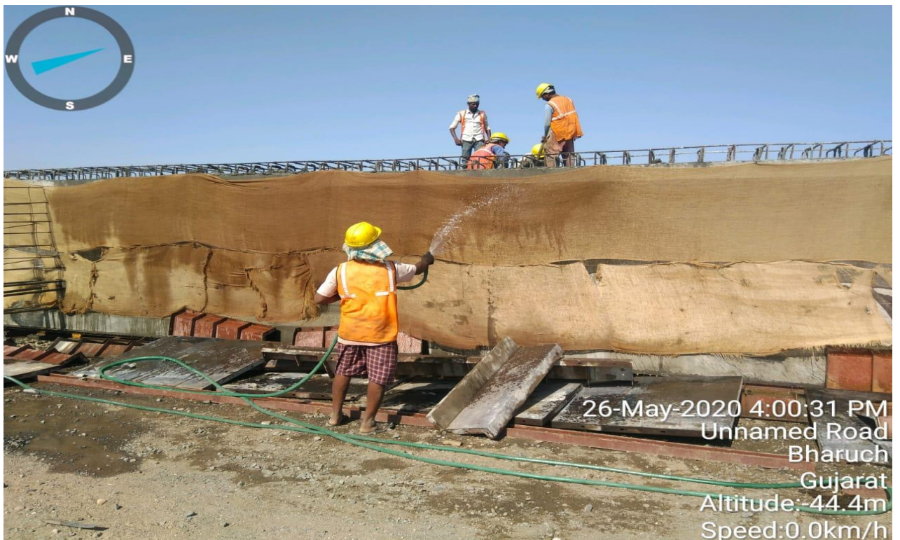
BC slab concrete work in progress LHS ch 294+985
