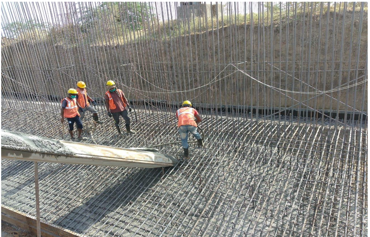
Concrete in progress at ch-313+809 MNB LHS A1 Raft
