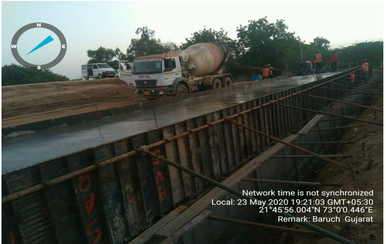
BC slab concrete work in progress LHS ch 294+985
