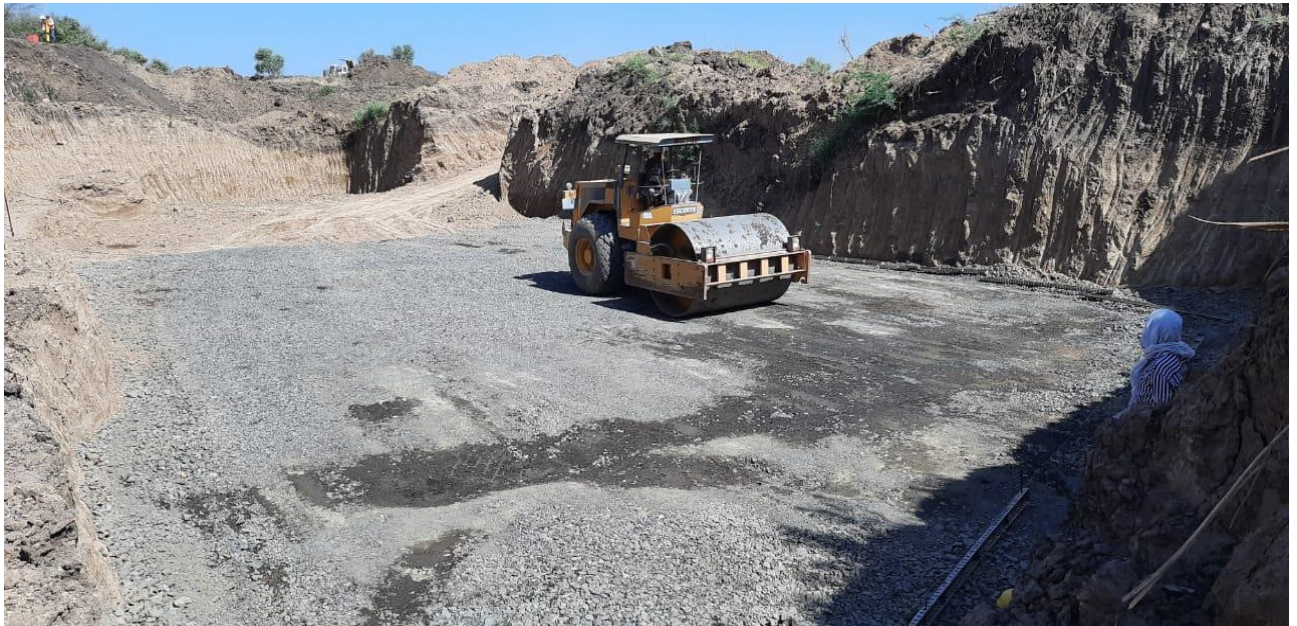
297+472 MNB LHS A1 rolling work in progress
