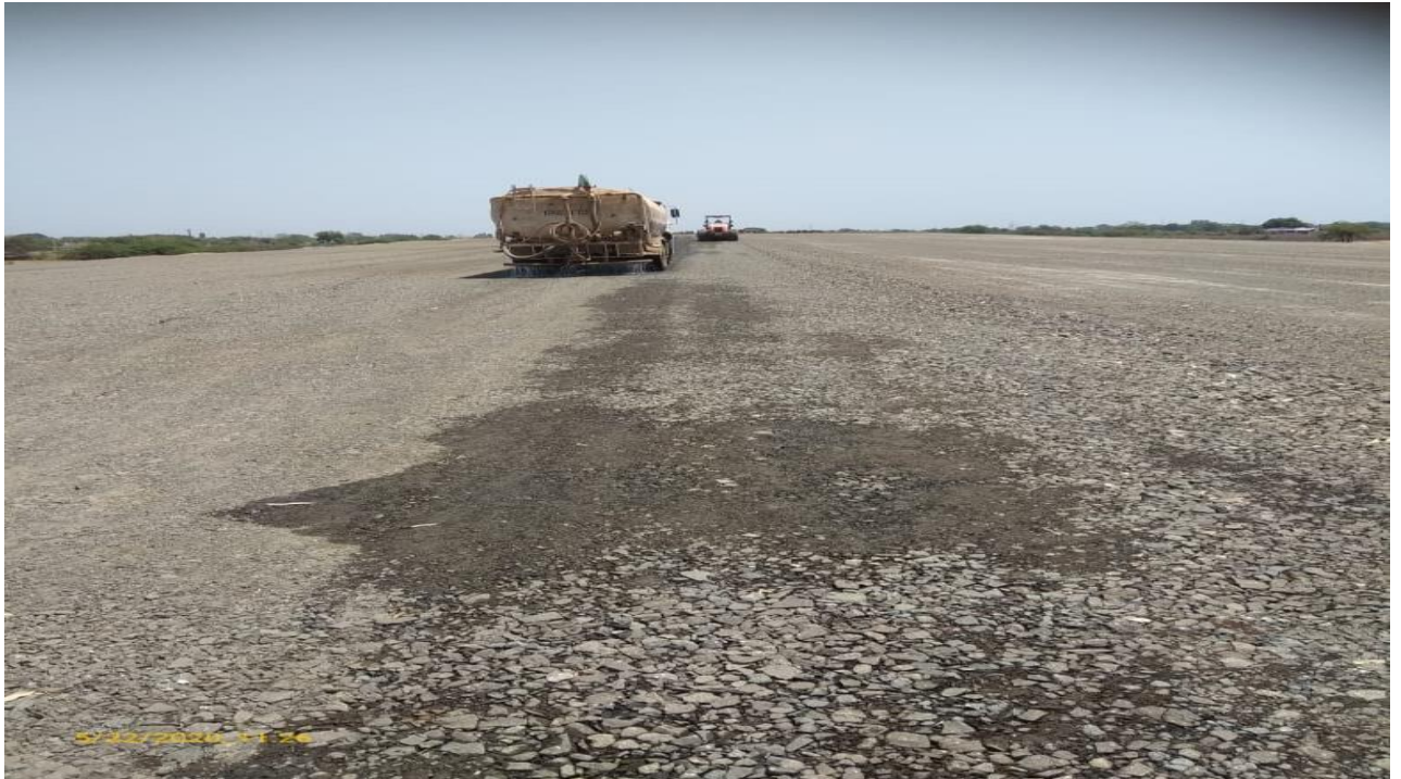
GSB watering and rolling Ch. 322+200 to 322+370 BHS
