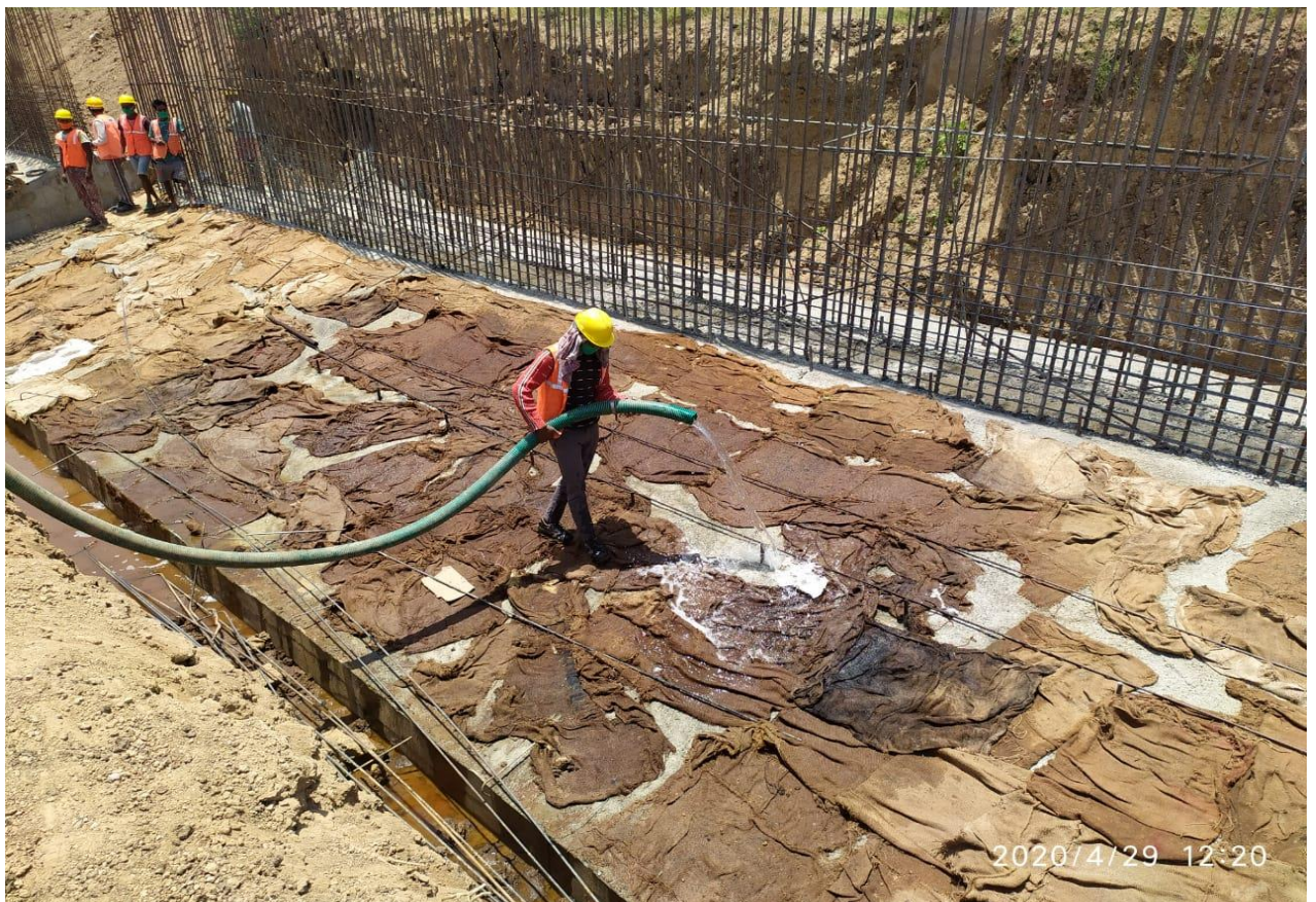
Ch.313+808 MNB A2 LHS Raft Curing Work in Progress
