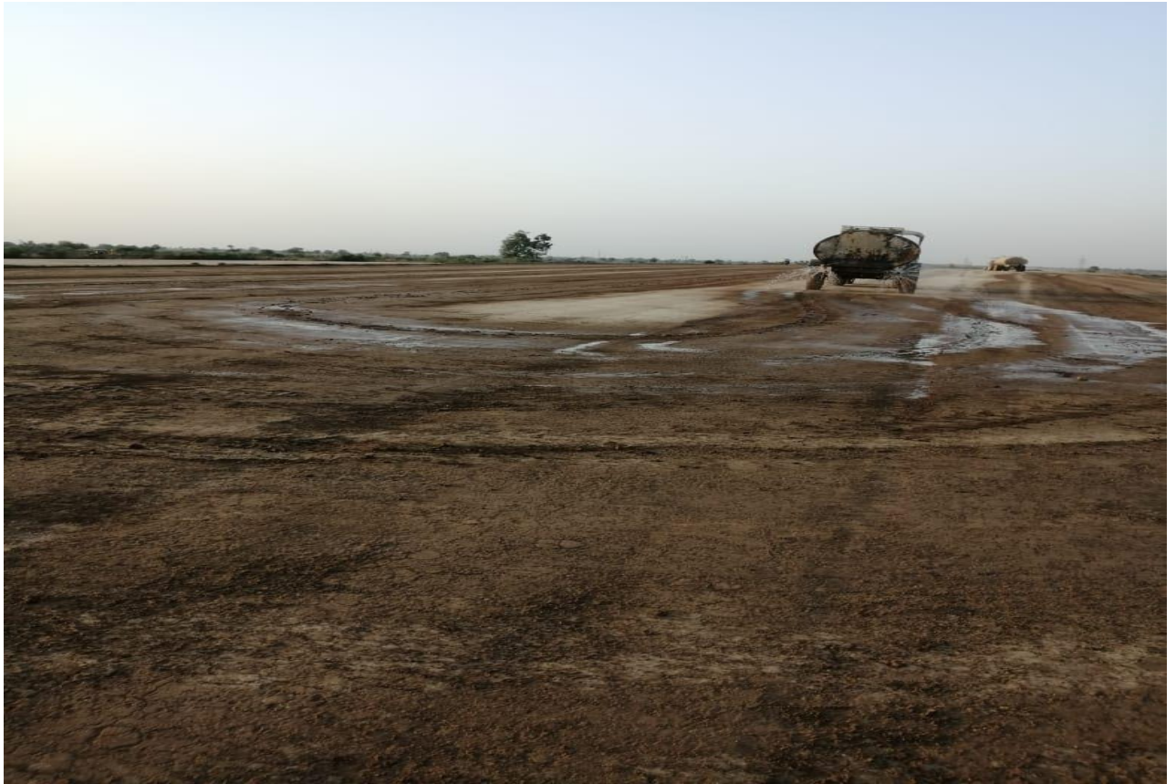
Ch.307+400 to 307+500 RHS Earthwork in Progress
