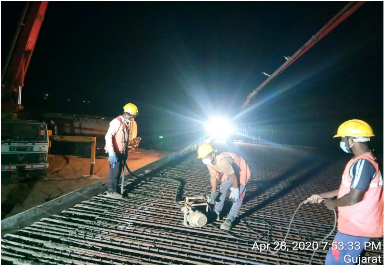
Ch.317+460 PUP LHS TOP Slab Concrete Work in Progress
