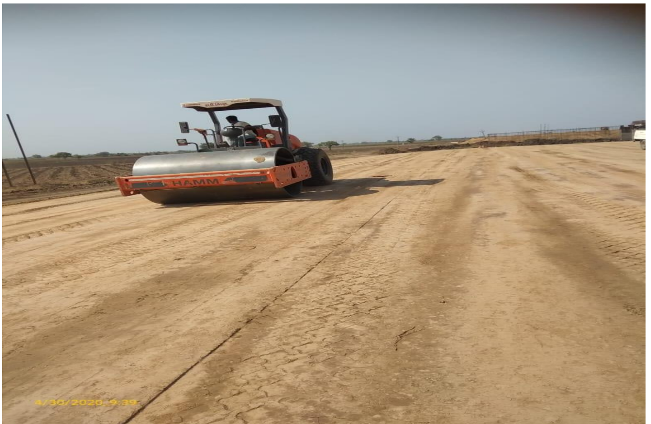
317+500 to 317+760 SG 1 st rolling in progress
