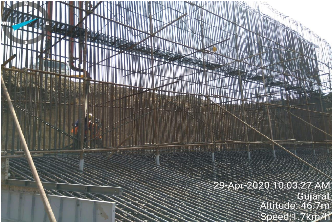
Ch.297+472 MNB A2 RHS Raft Concrete Work in Progress
