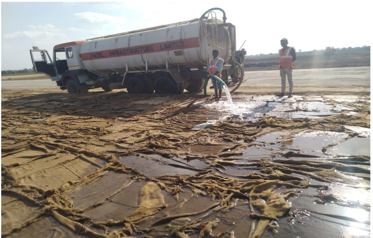
Dt. 10.03.2020 PQC curing work in progress at CH-305+400 LHS
