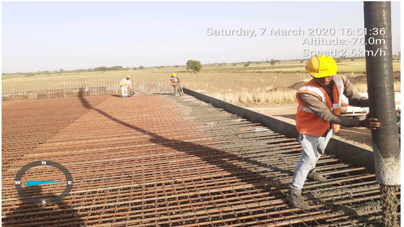
Dt. 07.03.2020 Slab concrete work in progress at ch 300+725
