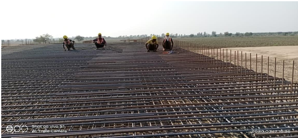
Dt. 17.03.2020 PUP slab( RHS) reinforcement in progress at ch 306+820
