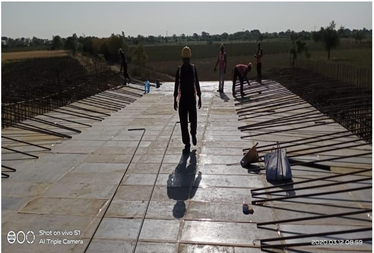
Dt. 12.03.2020 Shuttering for PUP slab (RHS) in process at ch-306+820
