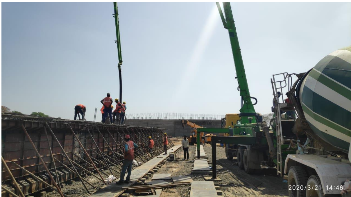
Dt. 21.03.2020 321+253.mjb.lha.a1-p1.G-1 psc girder concrete in progress.
