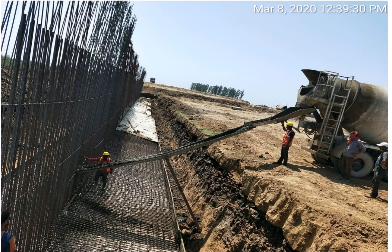
Dt. 08.03.2020 Ch-322+510 to -322+530 rhs retaining wall footing work in progress
