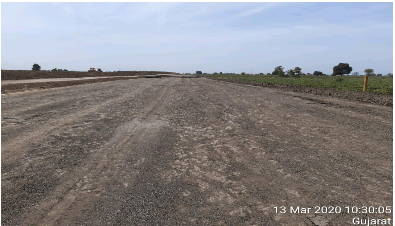
Dt. 13.03.2020 C&G done for small trucks parking at 292+030 to 292+320 lhs
