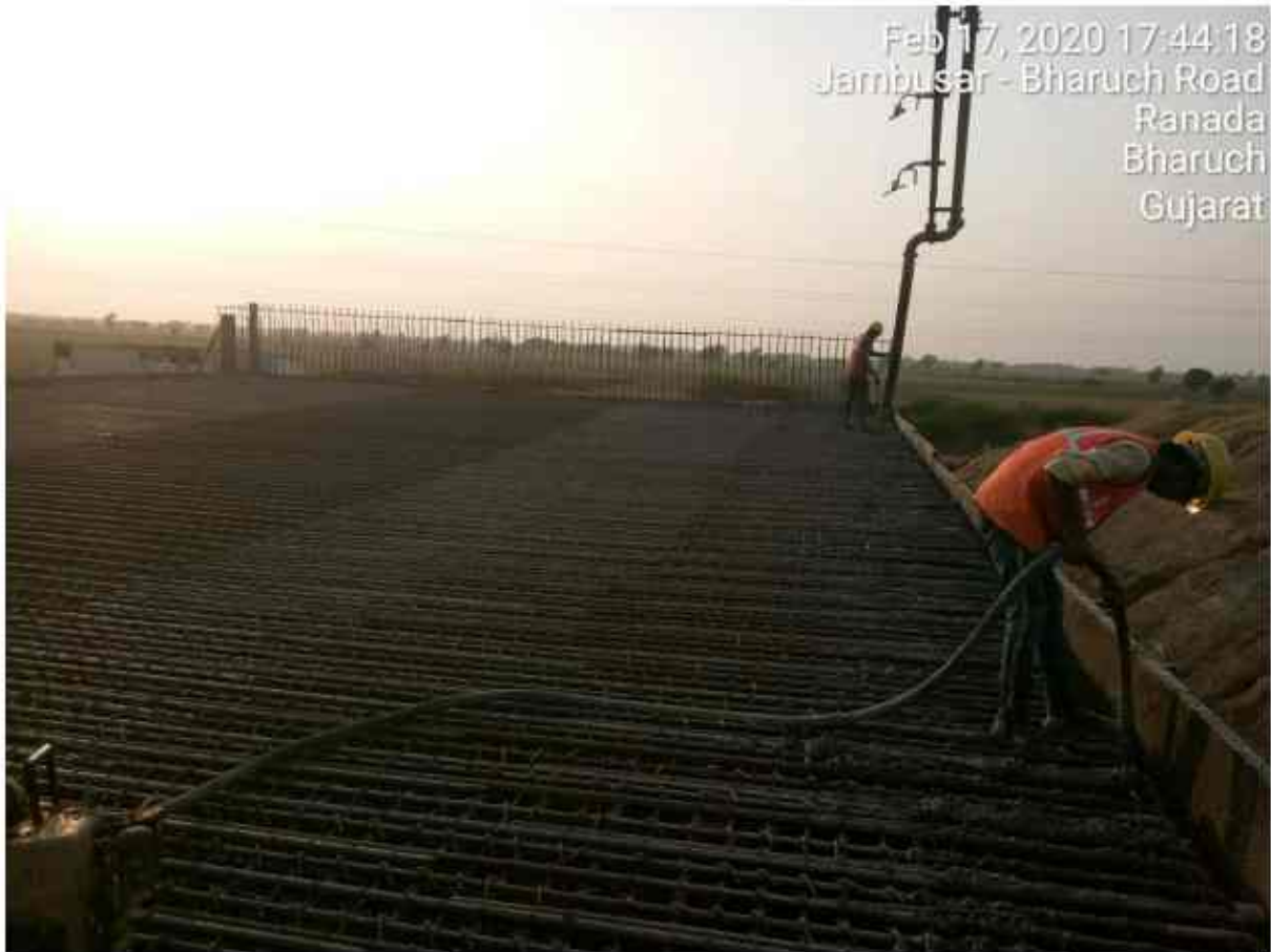
Chainage no 308+550 LVUP RHSTop slab's concreting.
