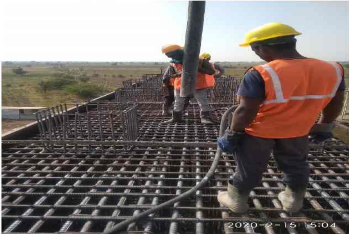
CH 293+014 ROBLP4 Pier cap concrete Pouring start
