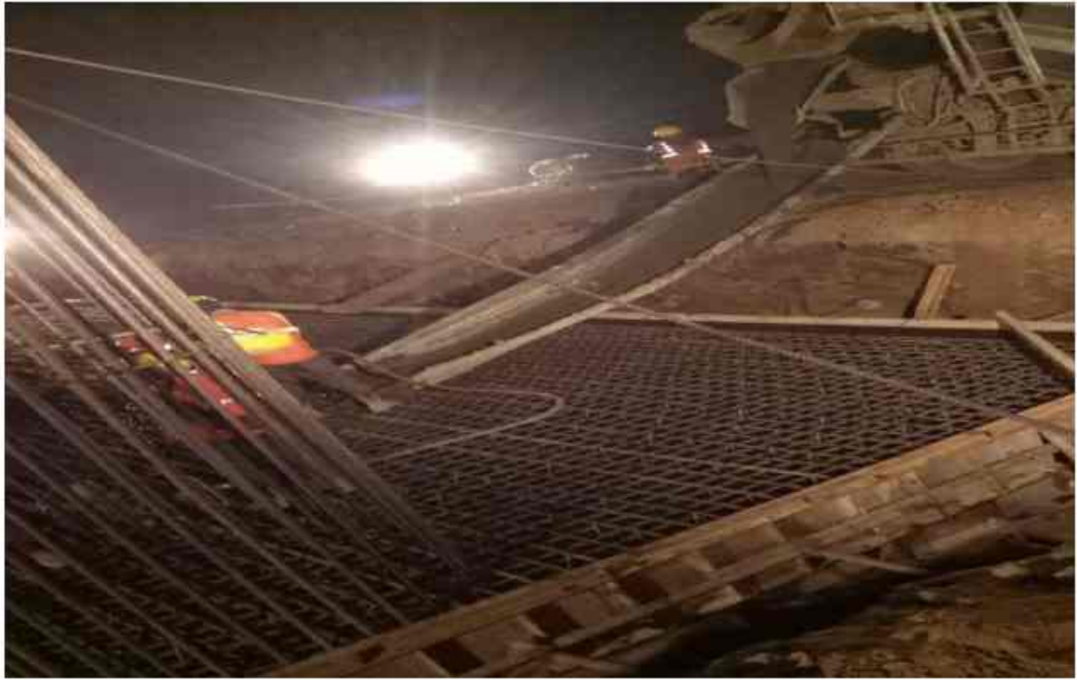
293+014 ROB pile cap RP15 concrete start
