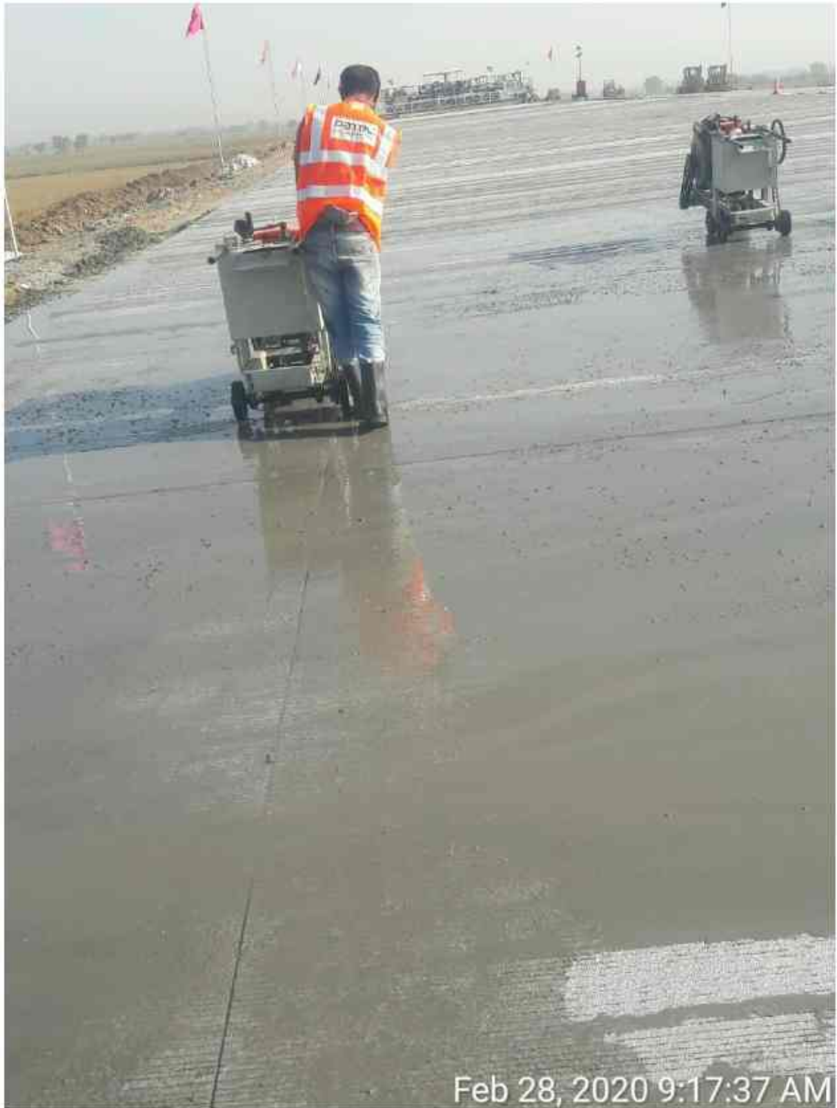
First cutting in progress
