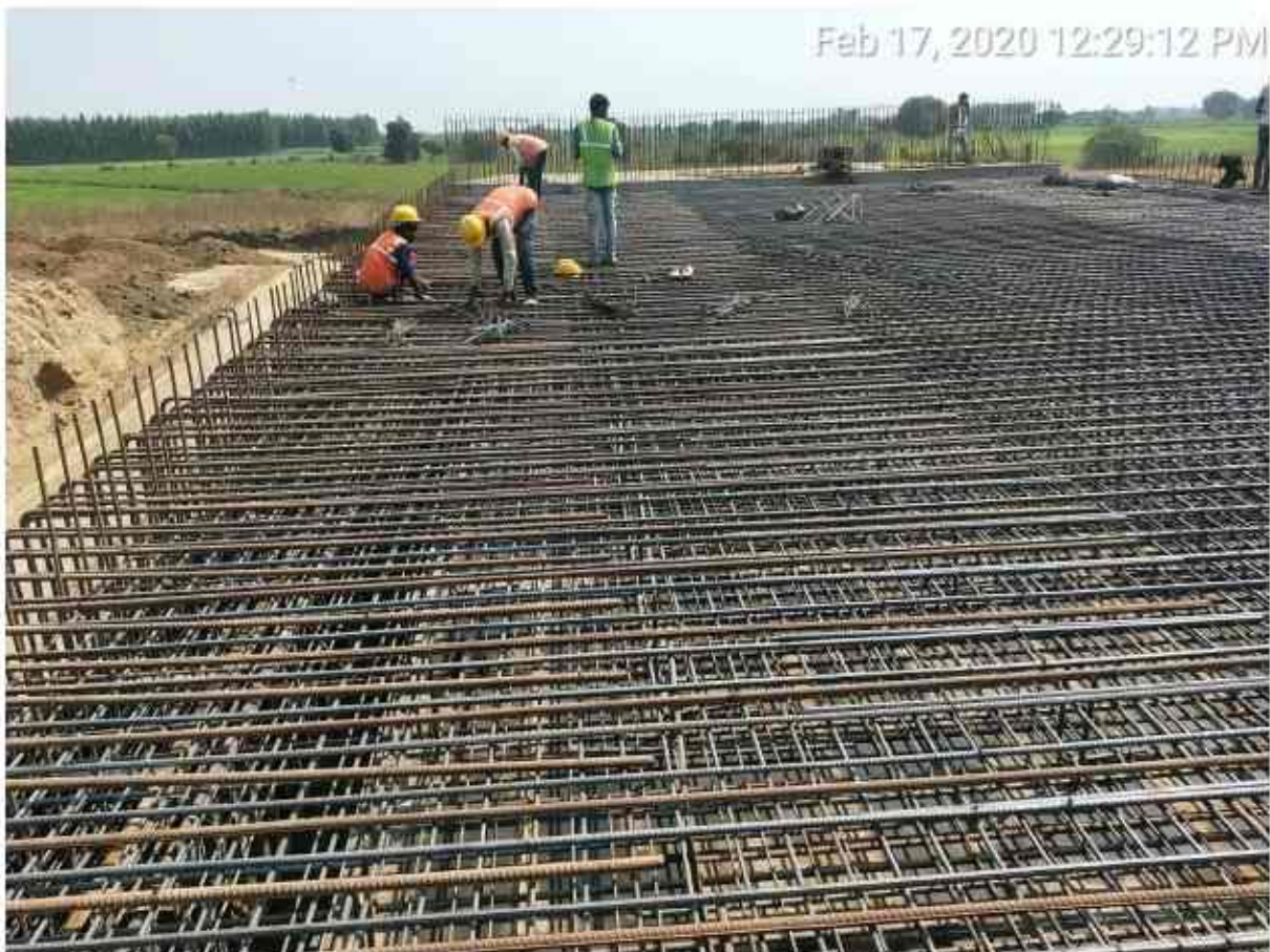
Ch-320+330 pup lhstop slab reinforcement work in progress
