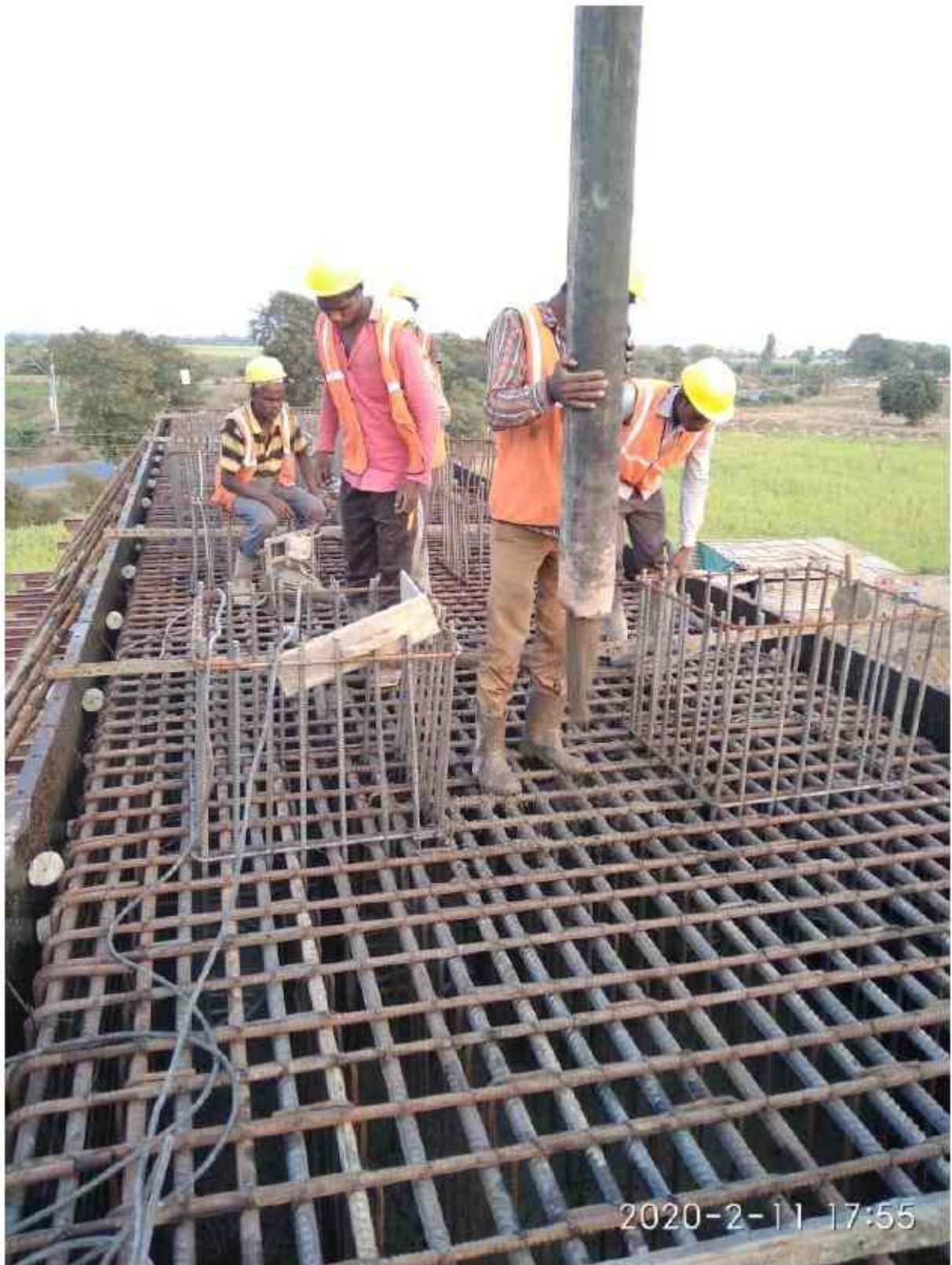
CH 293+014 ROB RP4 Pier cap concrete Pouring start
