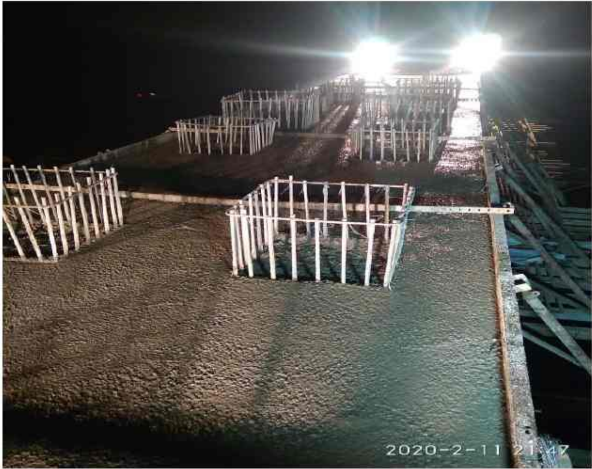
CH 293+014 ROB RP4 Pier cap complete.
