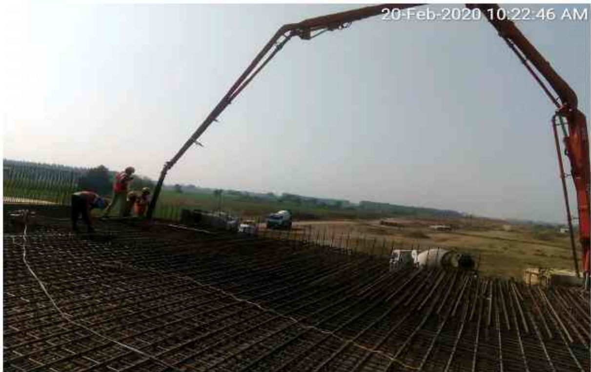
Ch-320+825,FUP, 3rd lift,LHS,concrete Pouring Progress.
