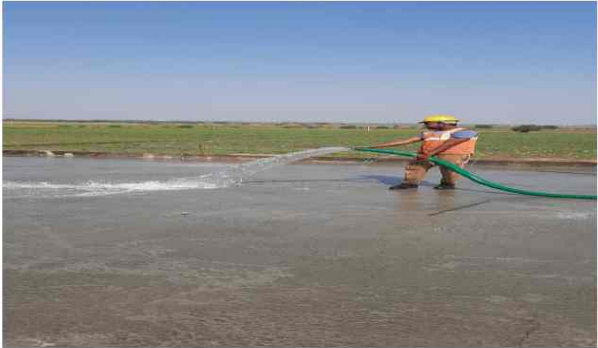
At ch 303+808 vu.pl.h.s slab curing in progress
