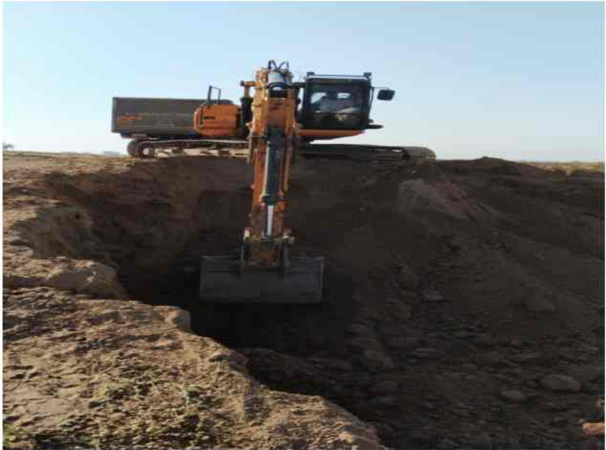
Ch 309+007 box culvert expression in progress
