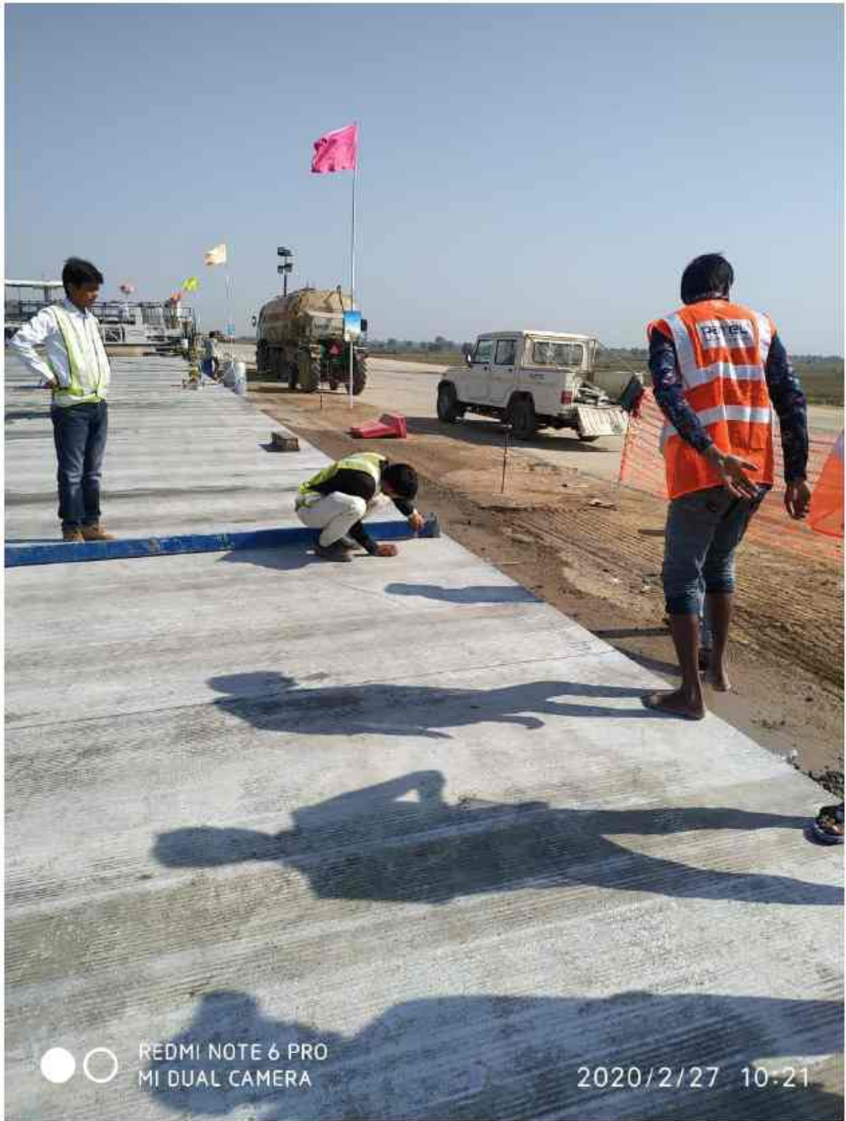
Surface regularity test is in progress at 304+725 (2)
