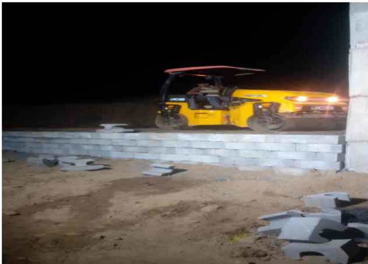
Block Erection Wall 2 sand filing 306+060
