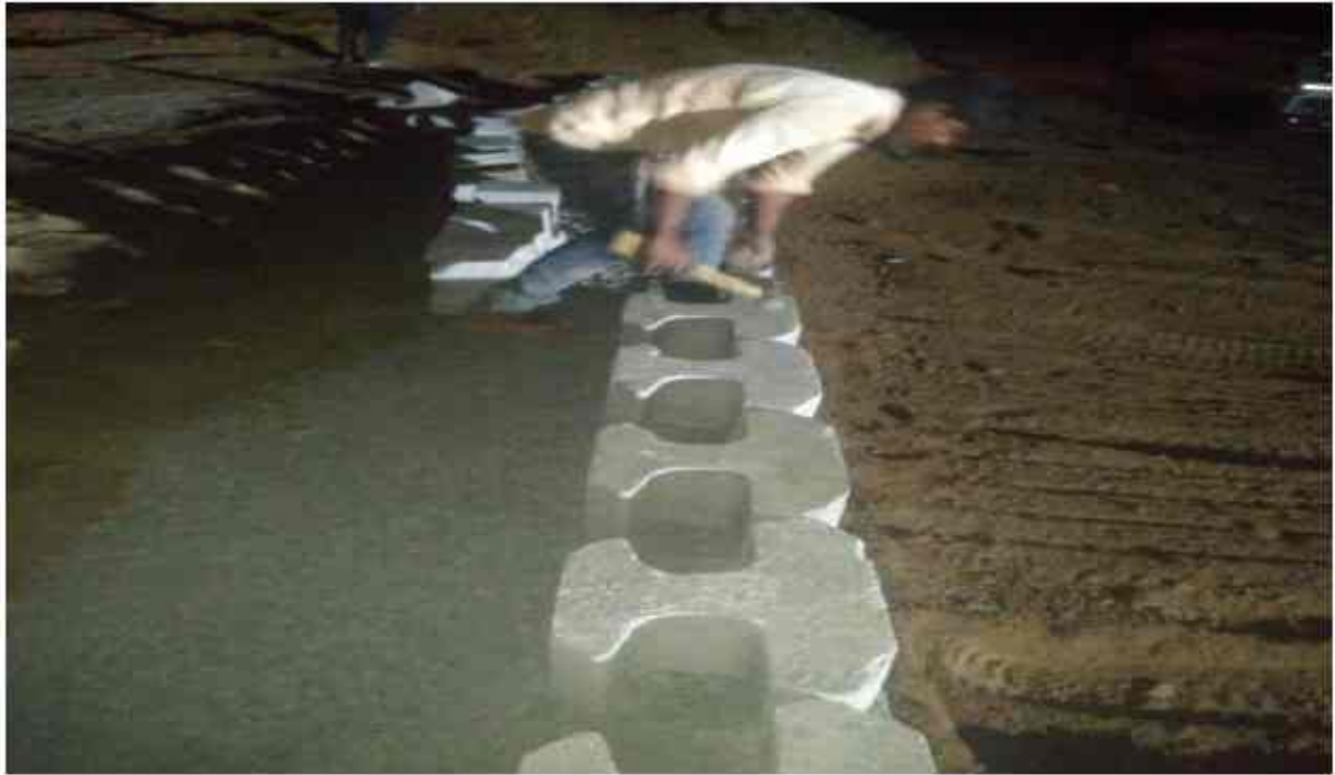
Block Erection wall-2 19th layer
