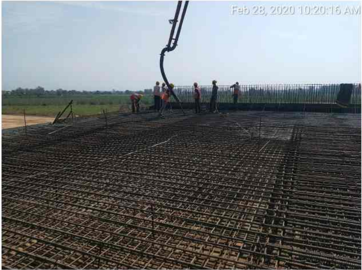
Ch-320+825 lhs pup top slab casting (w.p)
