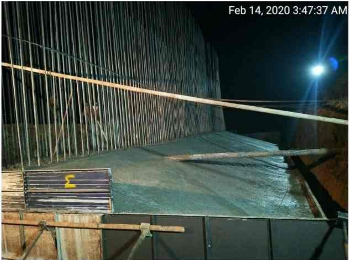
Ch-322+750 to-322+770 rhs retaining wall footing completed
