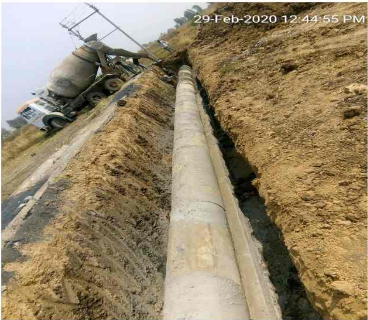
Ch-299+400, R H S, Utility cradle, in progress.
