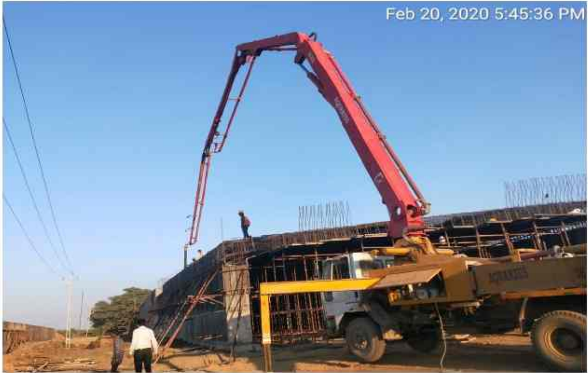
Ch-316+536 lvuplhsA2 final lift casting w.i.p
