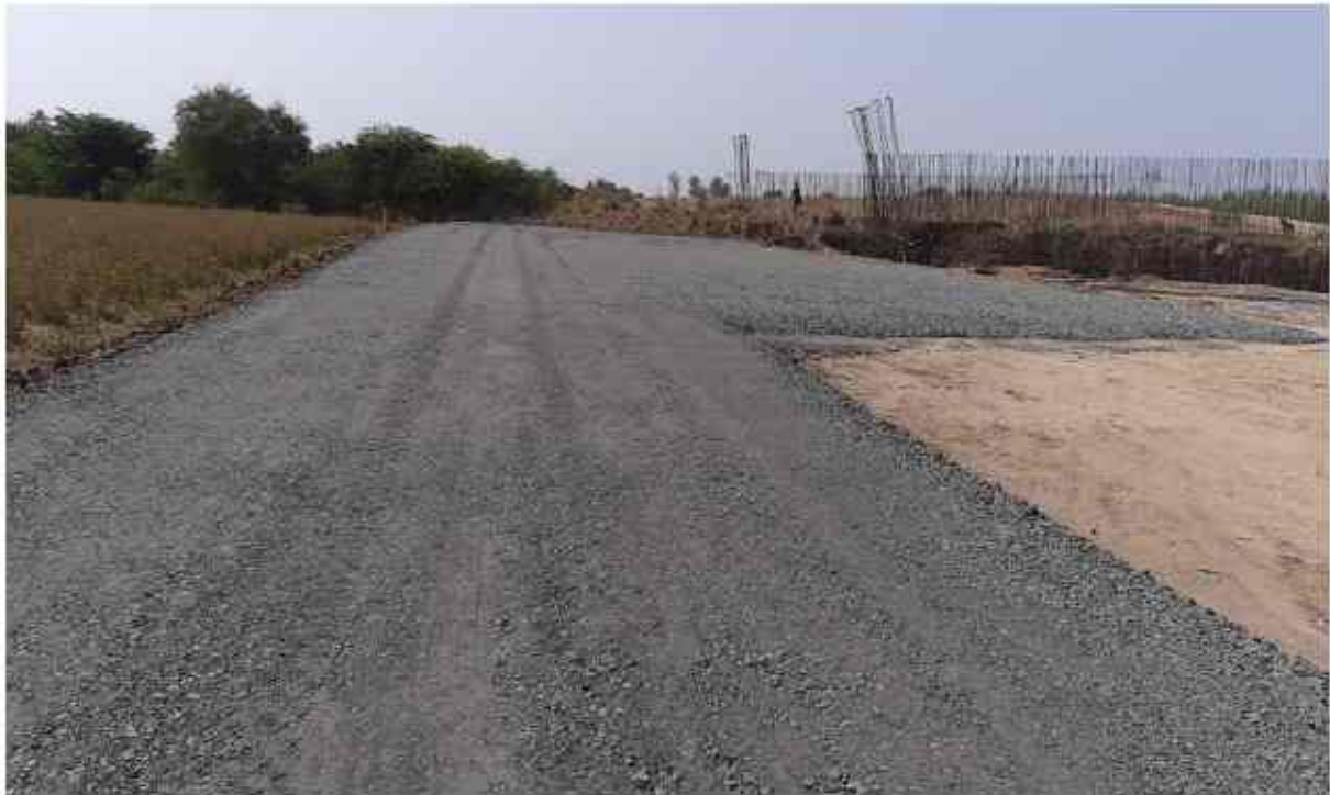
Girdersbed ready uptogsb level at ch 313+808
