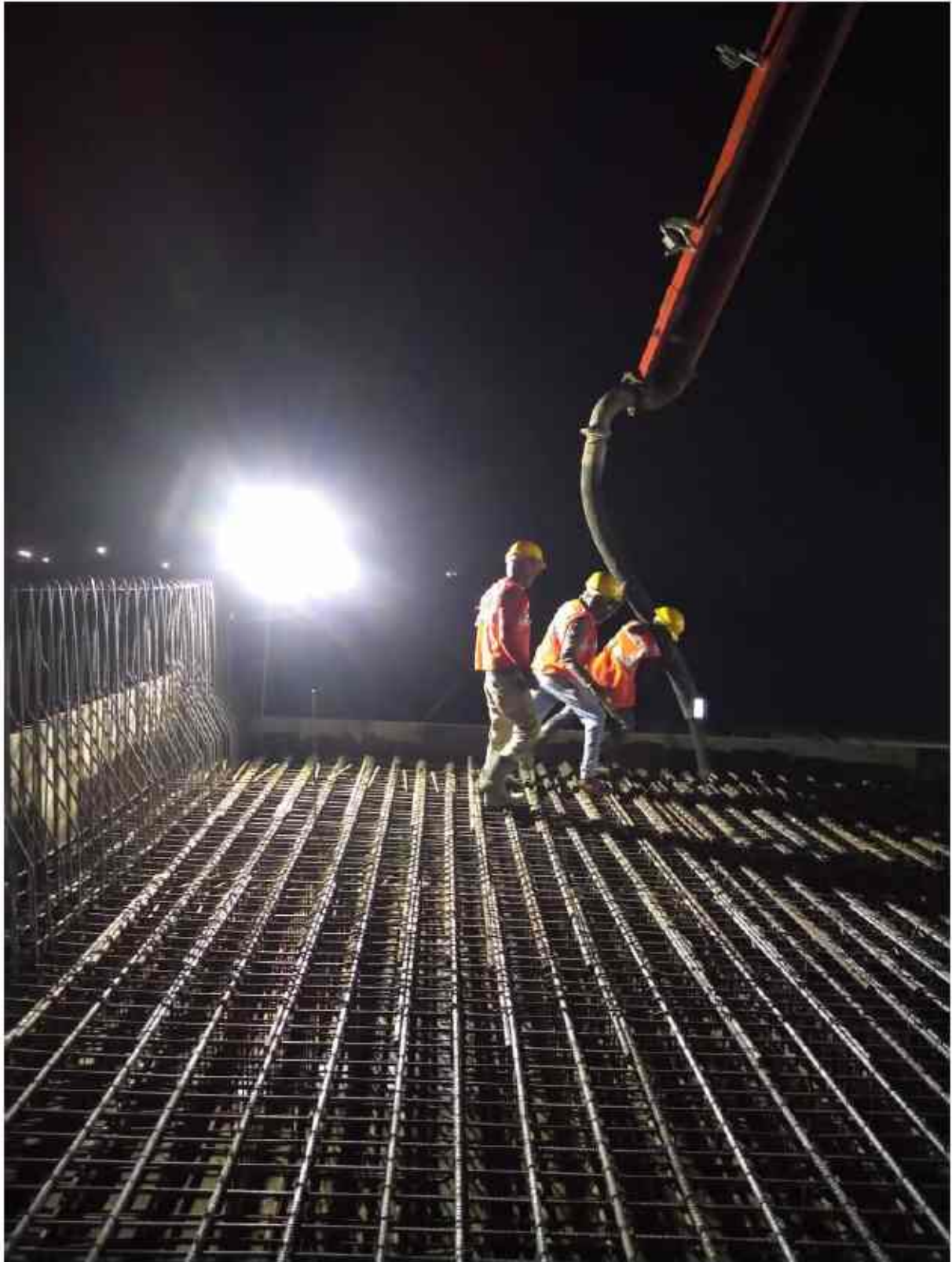
300+725 pup LHS slab concrete start
