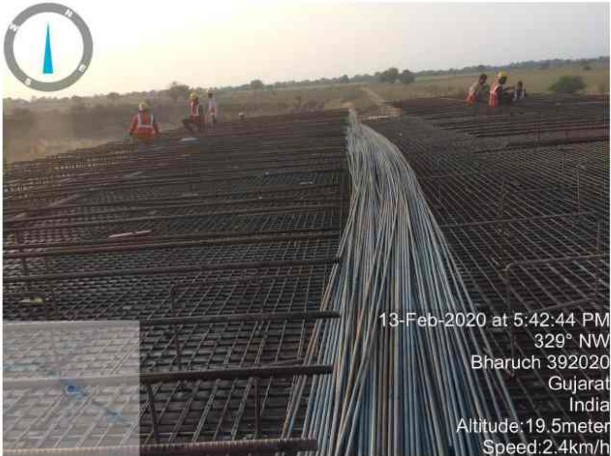
Ch-301+214 lvup LHS slab top main bar reinforcement work in progress.
