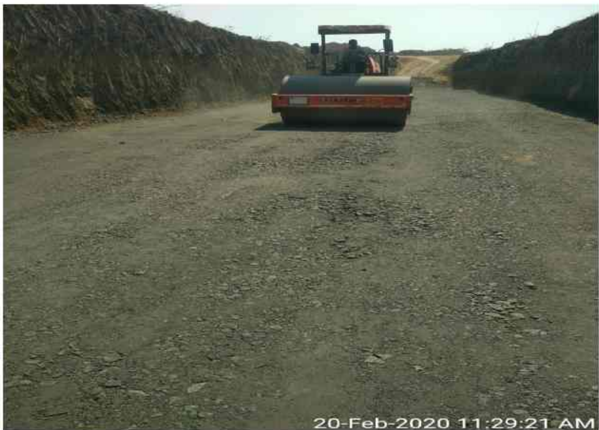
Rolling in progress at ch-309+840,MNB A2 ground improvement second layer
