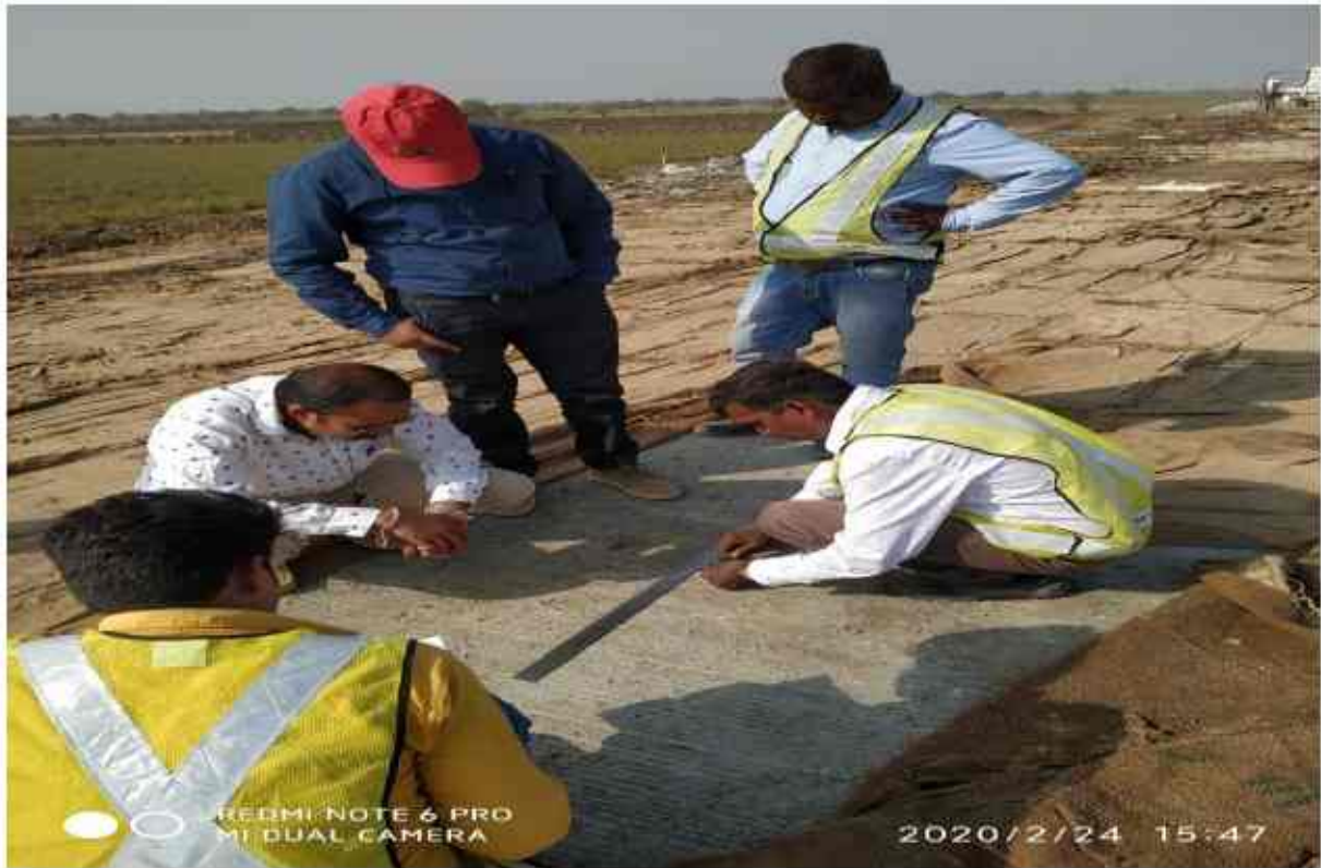
Texture test of PQC pavement (1)
