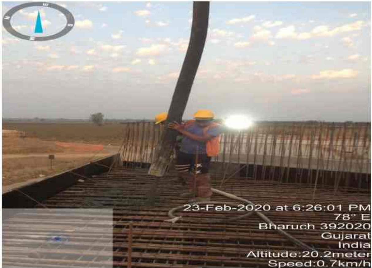
Ch-303+808 Vup LHStop slab pouring work start
