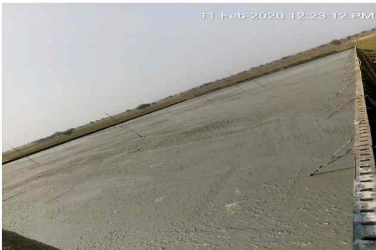
Completed, Top slab concrete, 306+060, PUP, LHS.
