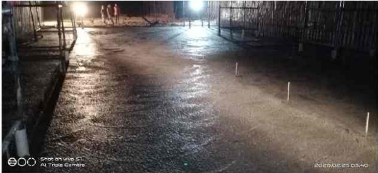
306+820 FUP raft LHS Concrete pouring completed
