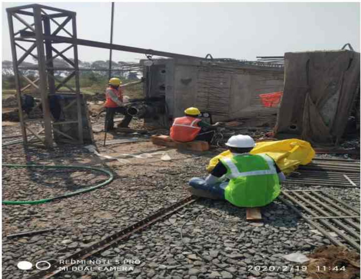
Stressing work in progress girder G1 321+253 A1P1 RHS
