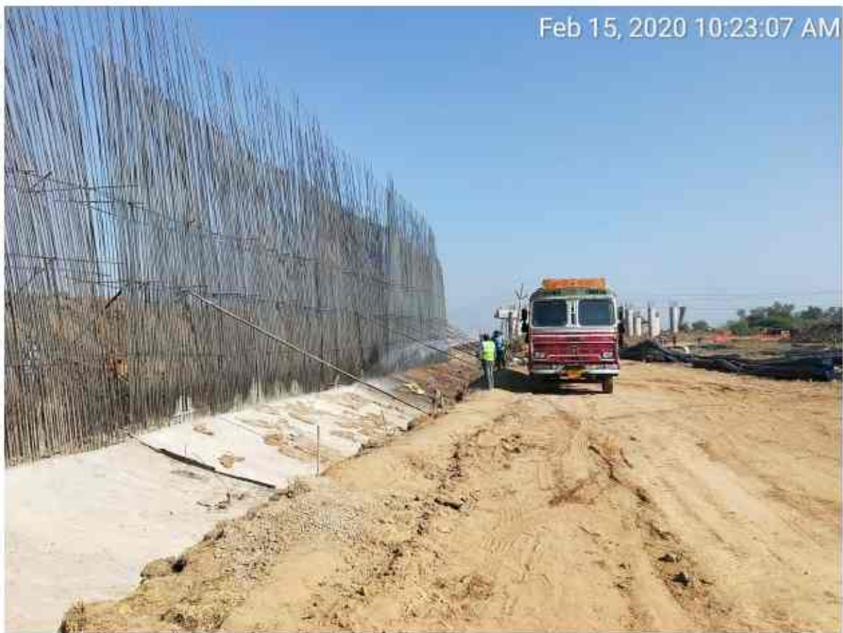
Ch-322 retaining wall curing
