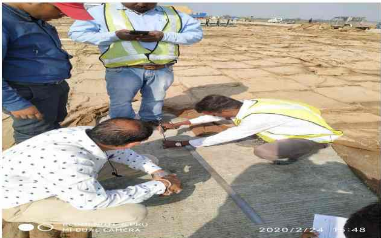
Texture test of PCC pavement
