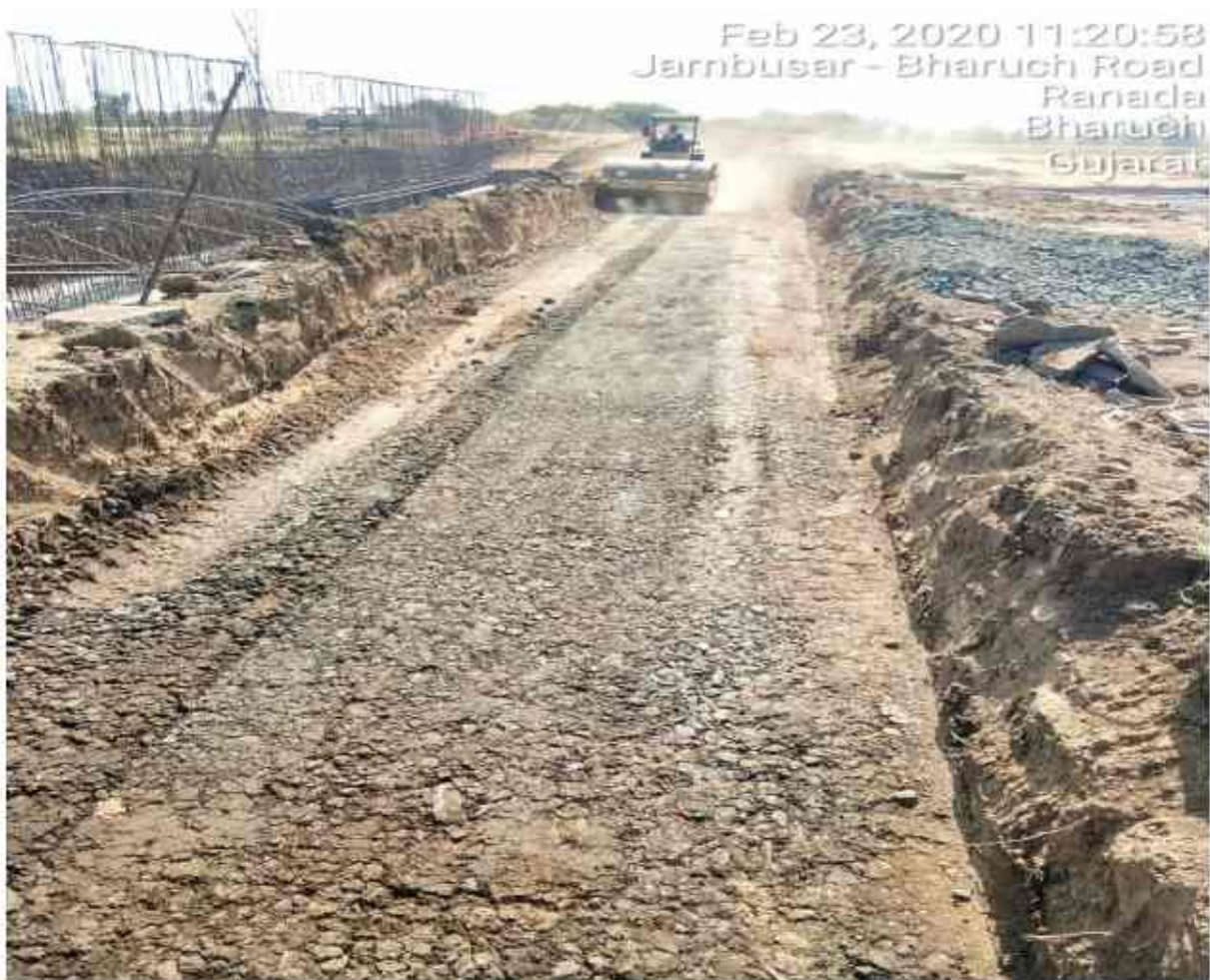
Rolling in progress for ground improvement at Chainage no 309+817 box culvert.
