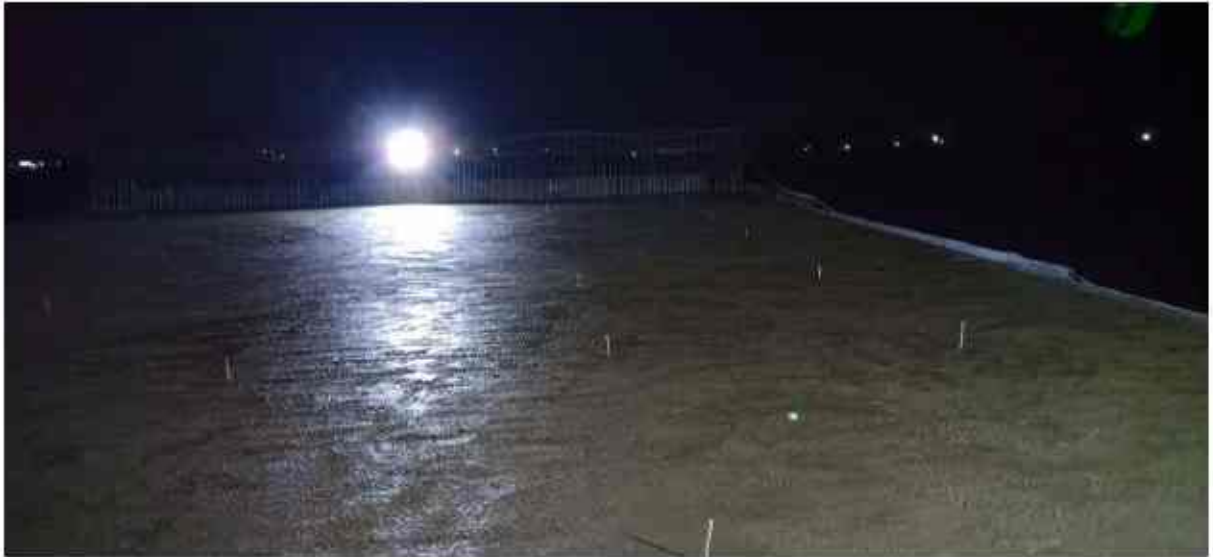
Ch 299+079 Rnstop slab concrete complete
