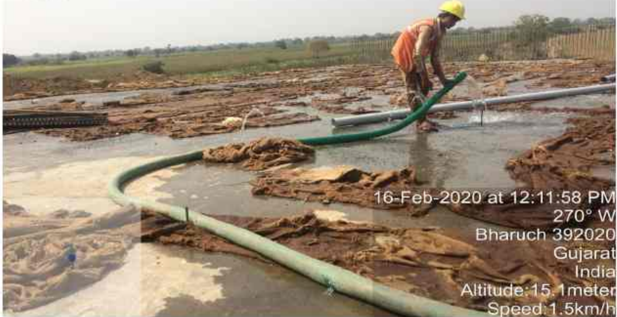
Ch-303+220 pup LHStop slab ANDRHWall curing work in progress
