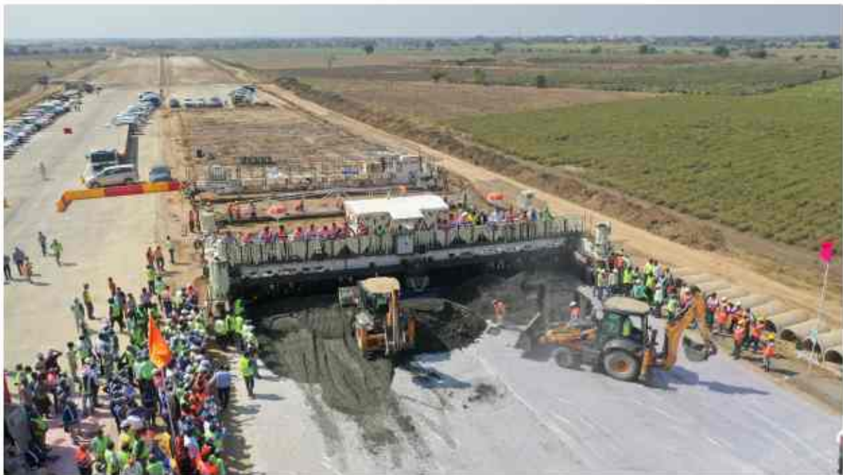
PQC Inauguration by 18.75m Paver
