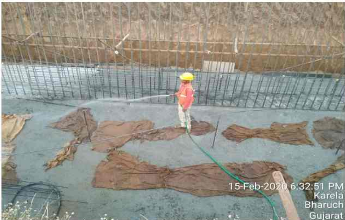
At ch- 309+840 MNB raft A1 bhs curing in progress
