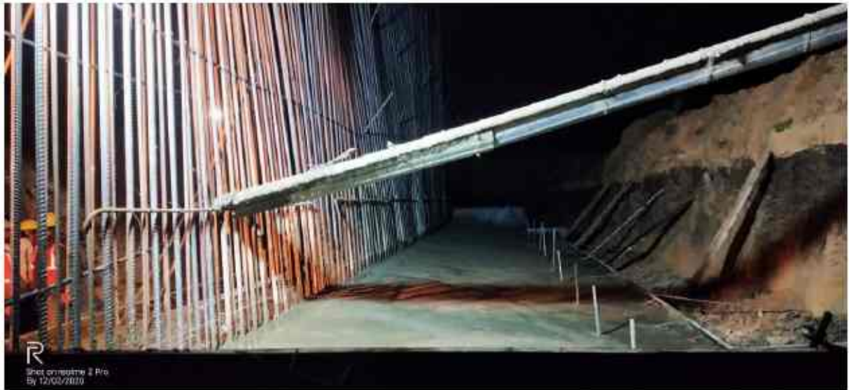
Ch-322+470 to 322+490 rhs retaining wall Footing casting complete
