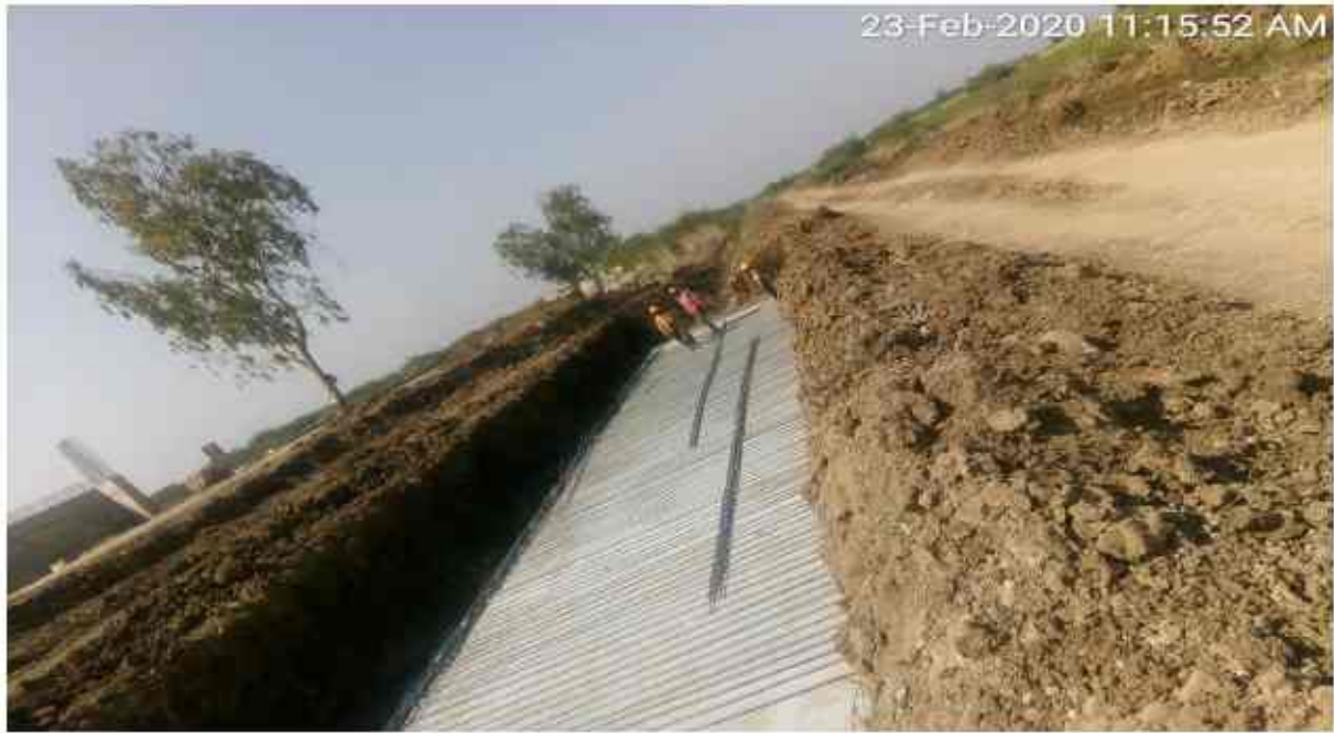
Ch-307+778,Box culverts,Reinforcement laying ,LHS, Progress.
