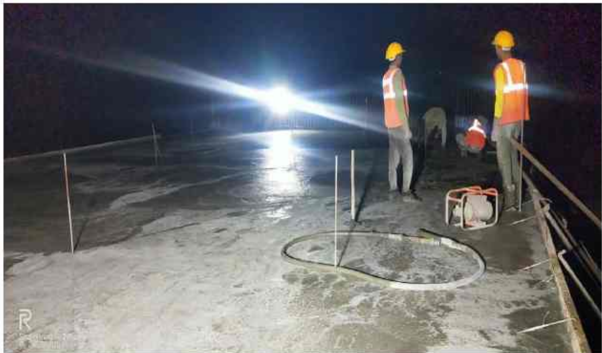
Ch-320-825 lhs pup top slab casting completed
