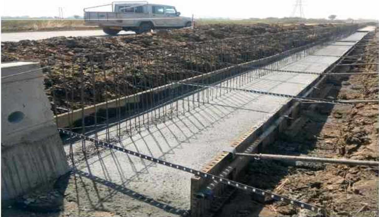
At Chainage no 308+380 to 308+420 toe wall R/Sraft has successfully completed.
