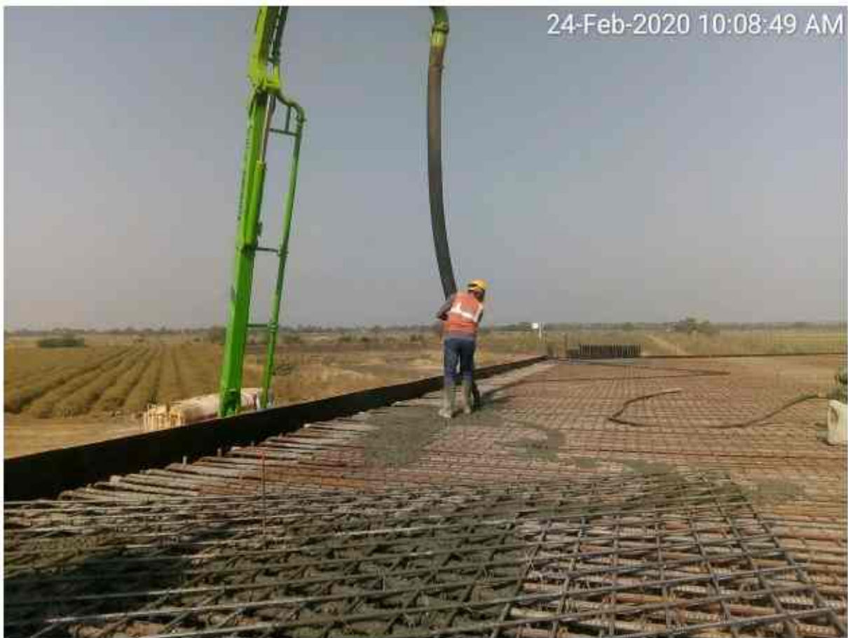
Start Ch-301+214, LVUP, LHS, Top slab Concrete Pouring.
