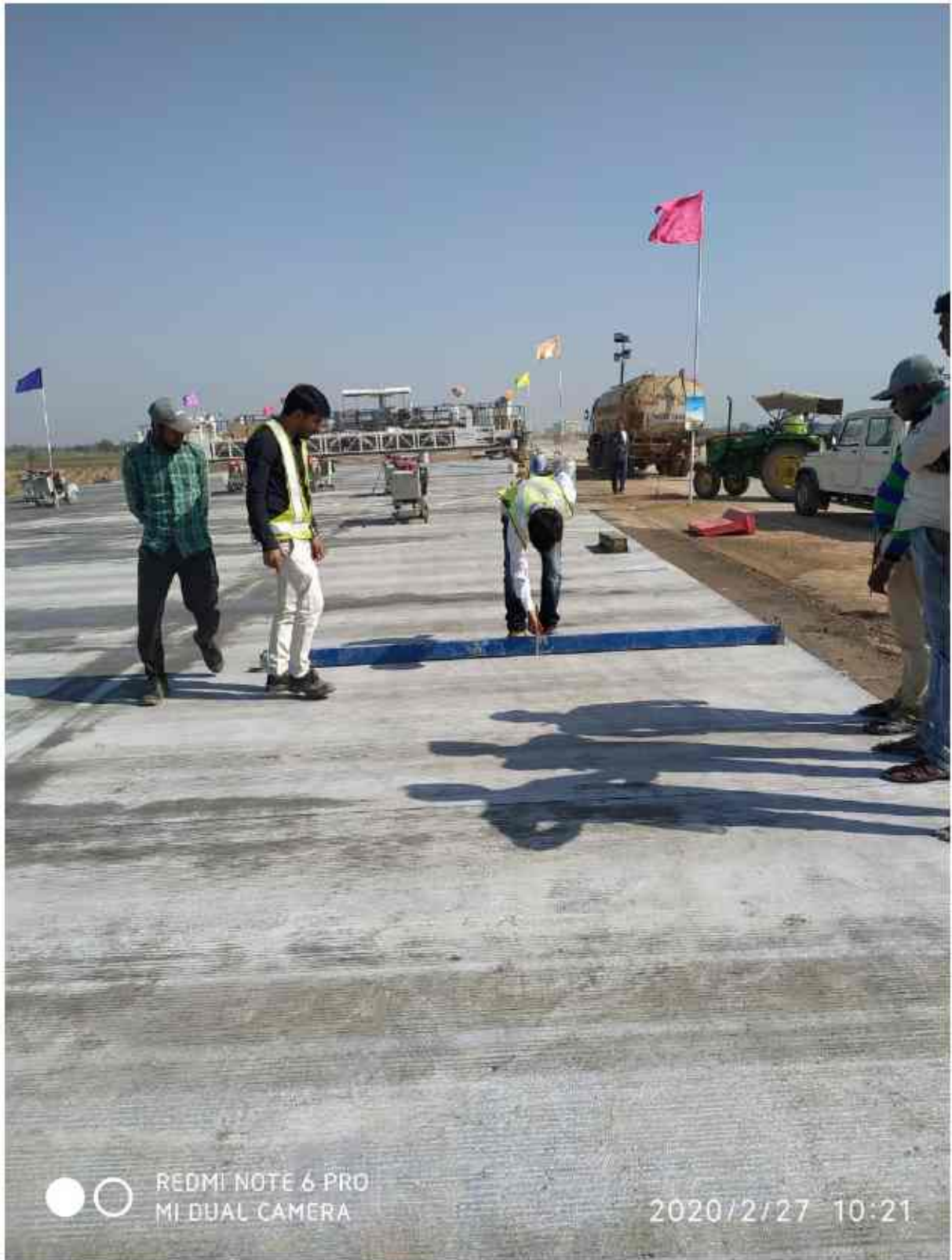
Surface regularity test is in progress at 304+725
