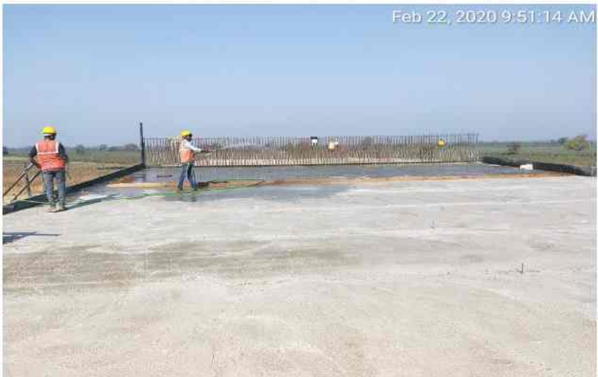
Ch-319+580 rhstop slab curing work in progress
