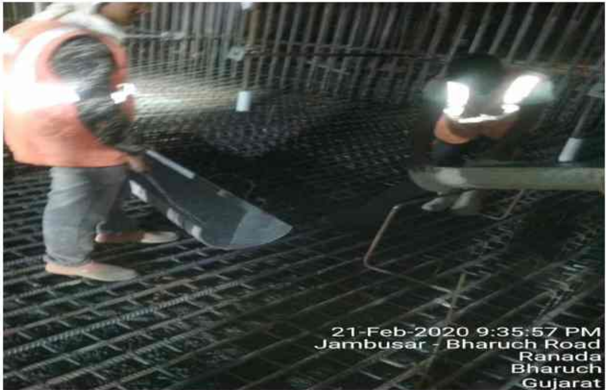
Concrete pouring in progress at ch-306+820 pup service road raft lhs
