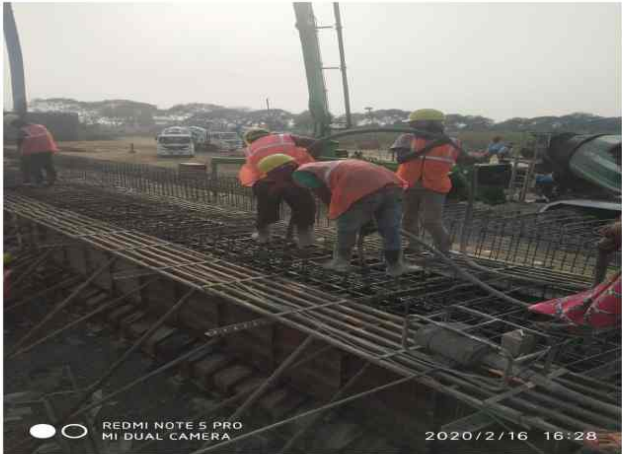
Concrete pouring PSC Girder A1P1 G4 Rhsmb 321+253
