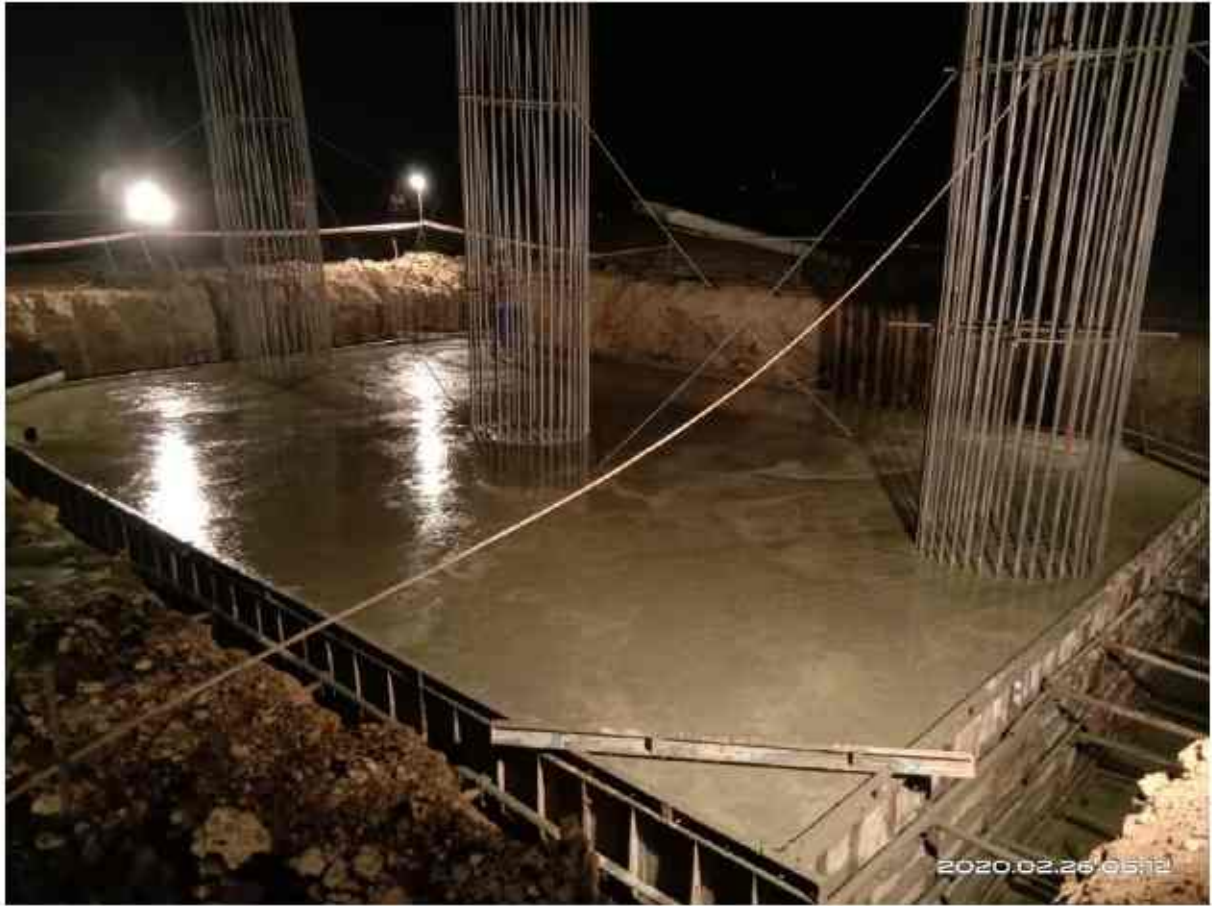
293+014 ROB pile cap RP15 complete
