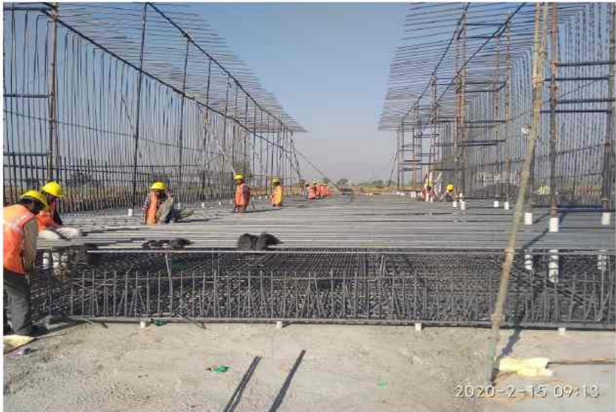
CH 292+400 PUP LHSraft reinforcement work in progress
