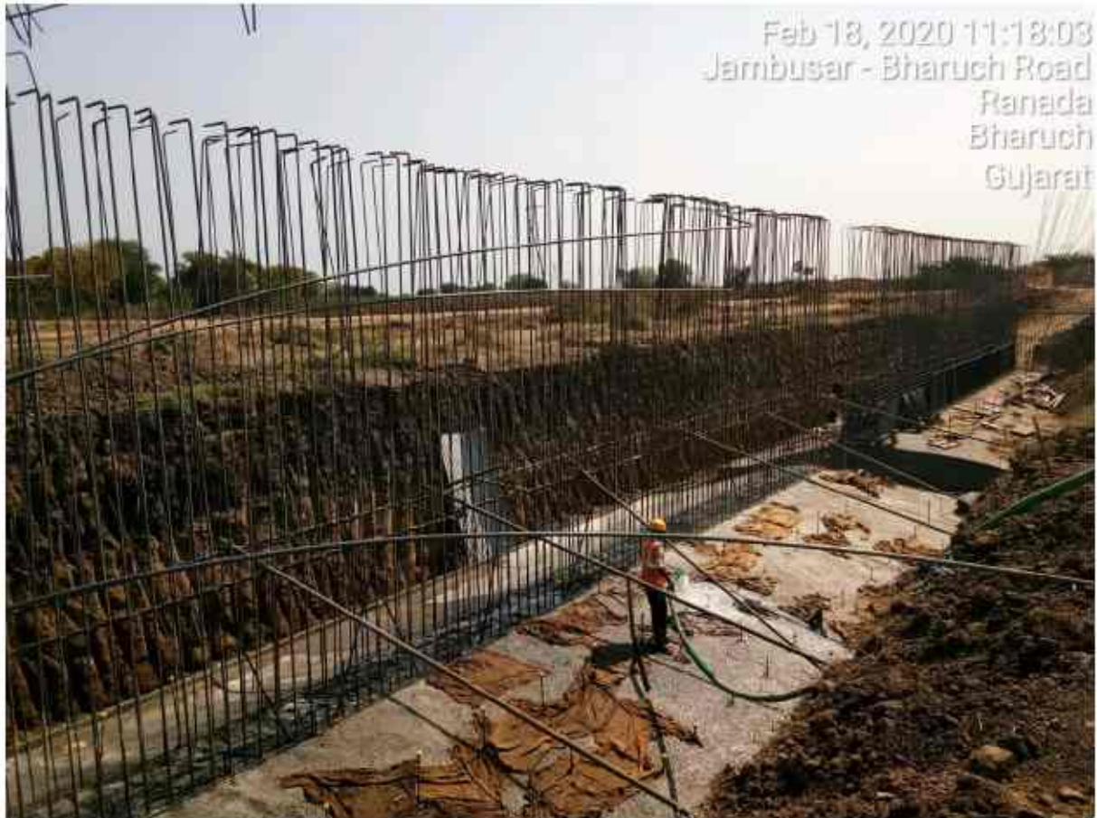
Curing in progress at Chainage no 309+840 MNBA1 BHS.
