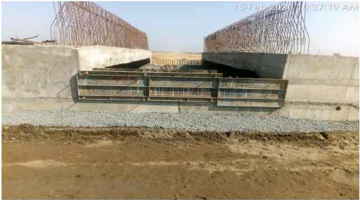
Shuttering for Median-intermediate arrangements,PUP,305+058.
