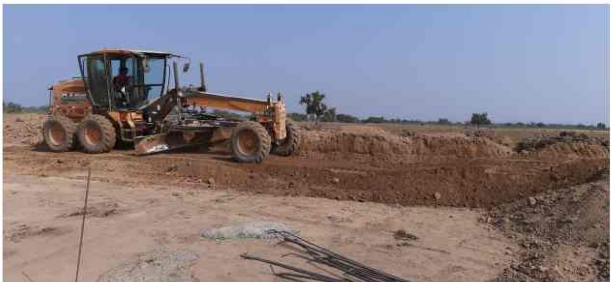
Making of girders bed work in progress at ch 313+808
