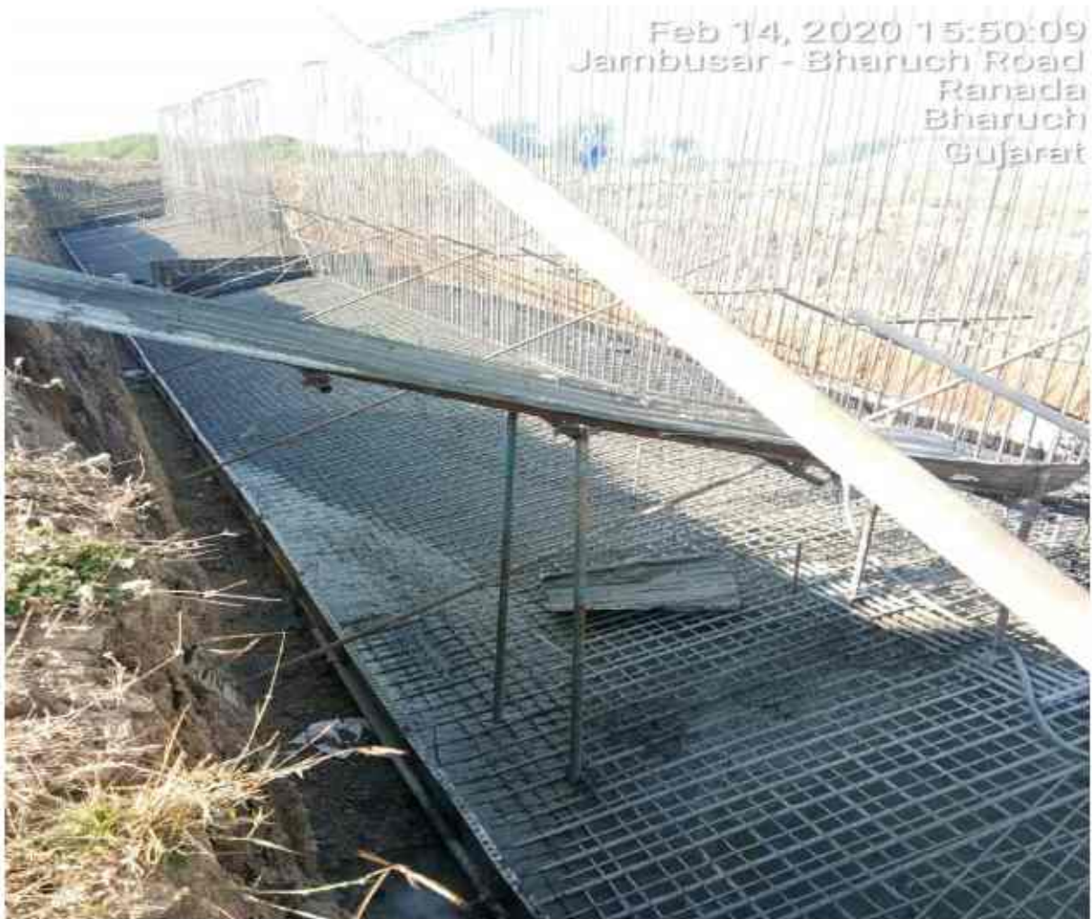
Concreting at Chainage no 309+840 MNB A1 RHSside.
