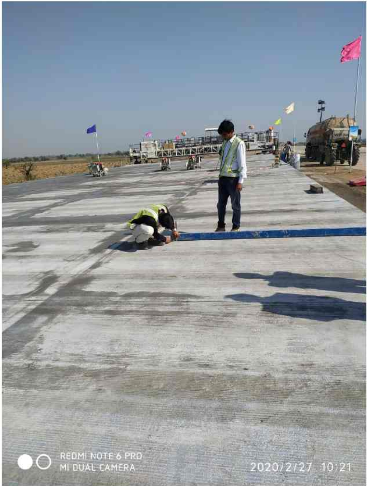
Surface regularity test is in progress at 304+725 (1)
