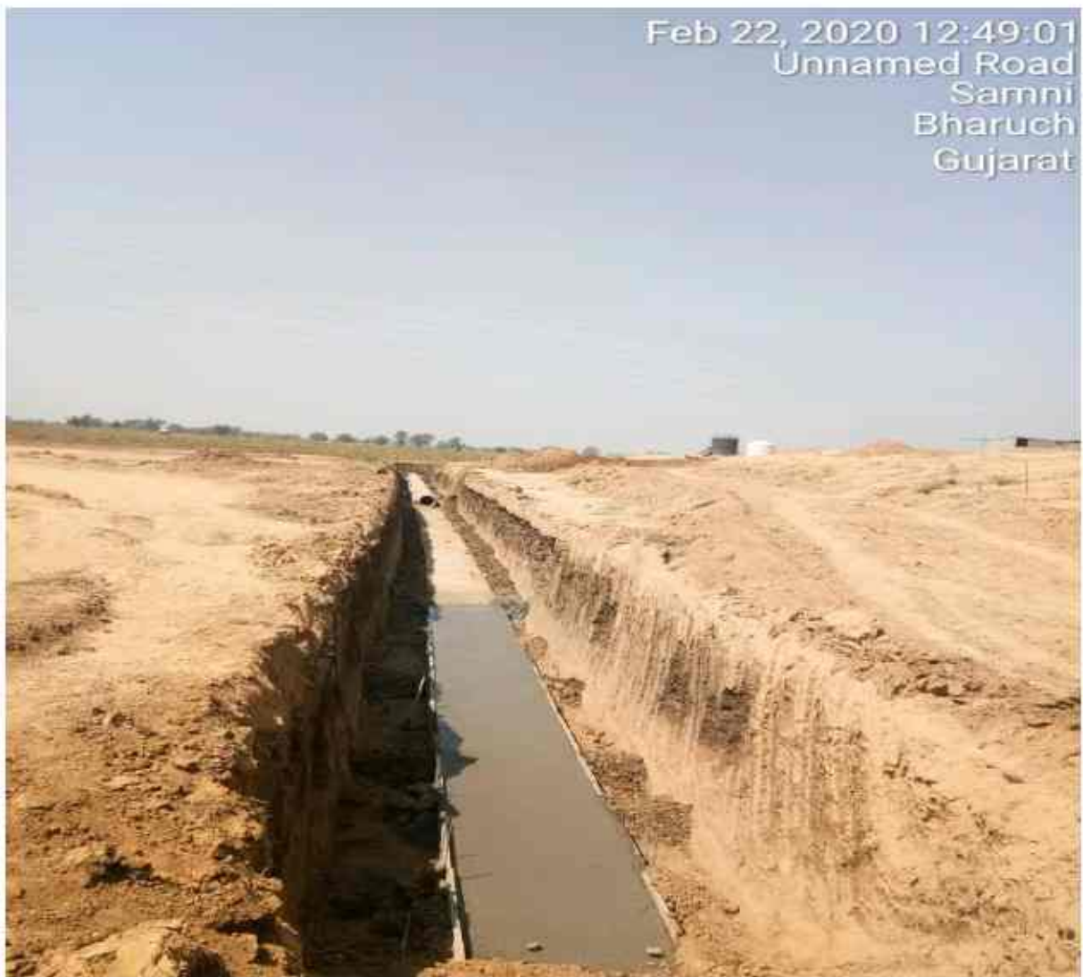
At Chainage no 308+400 utility RHPcc work has successfully completed.
