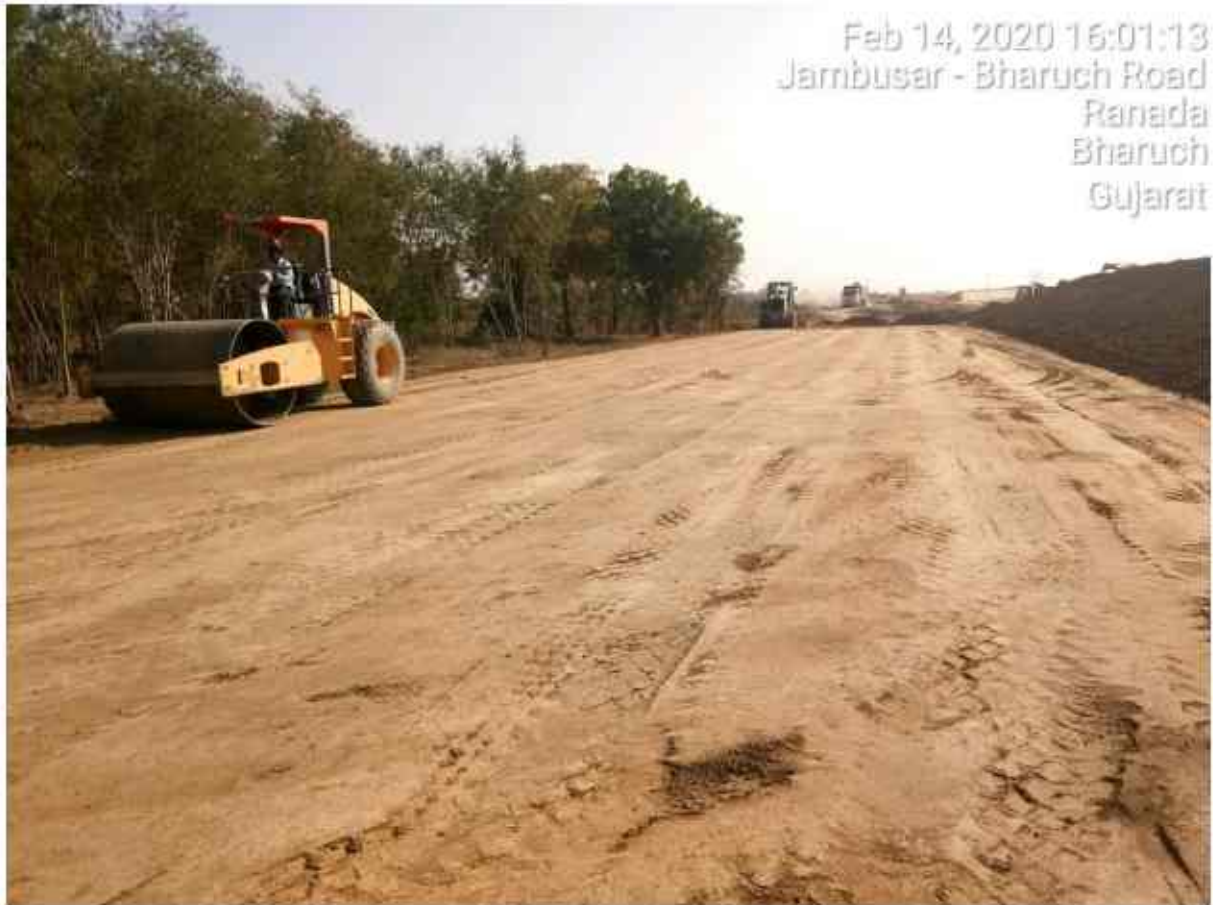
At Chainage no 309+880 MNB RHSbed preparation for girder work in progress.
