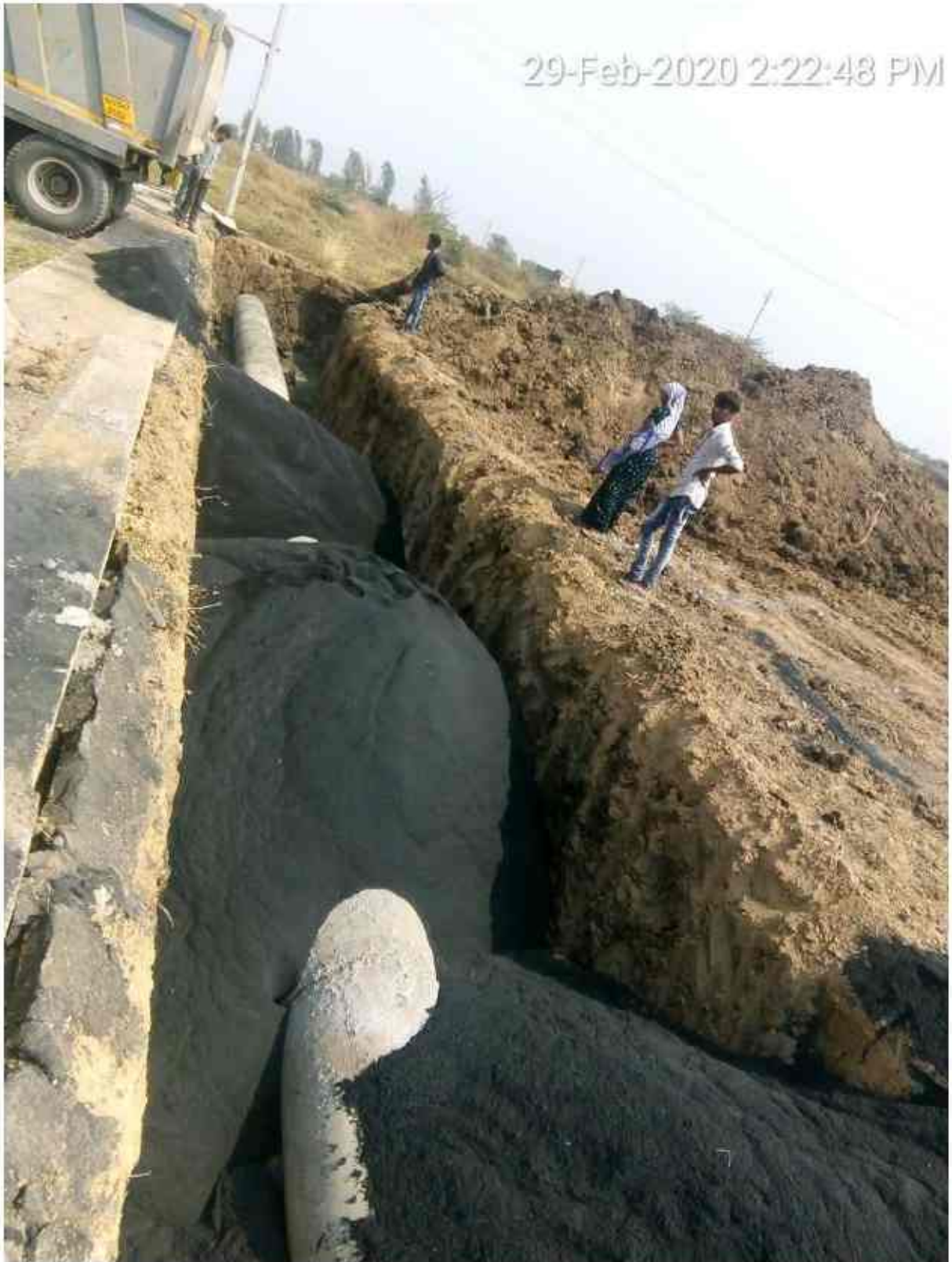
Ch-299+400, Utility, RHS, back filling in progress.
