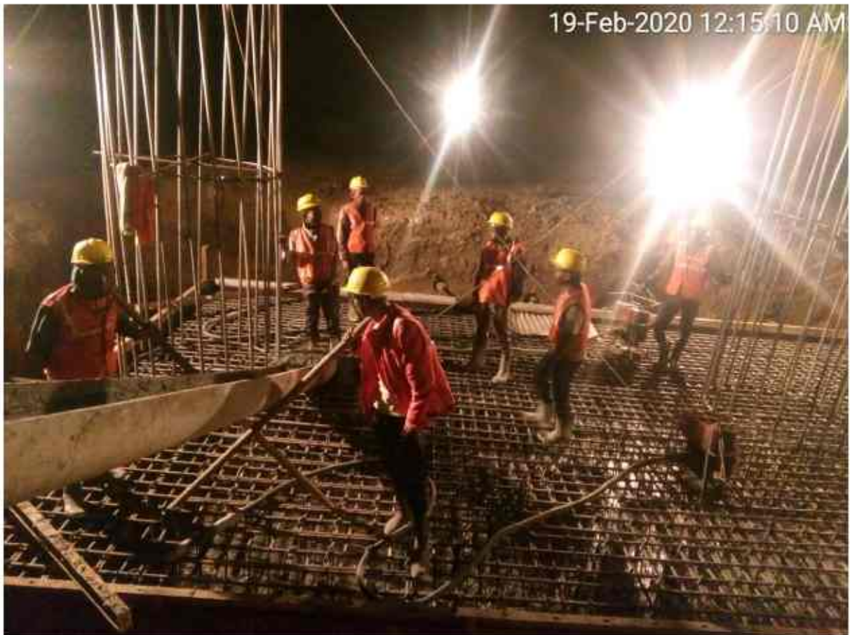
Ch-293+014,ROB-RA2 File Cape Concrete Pouring Progress
