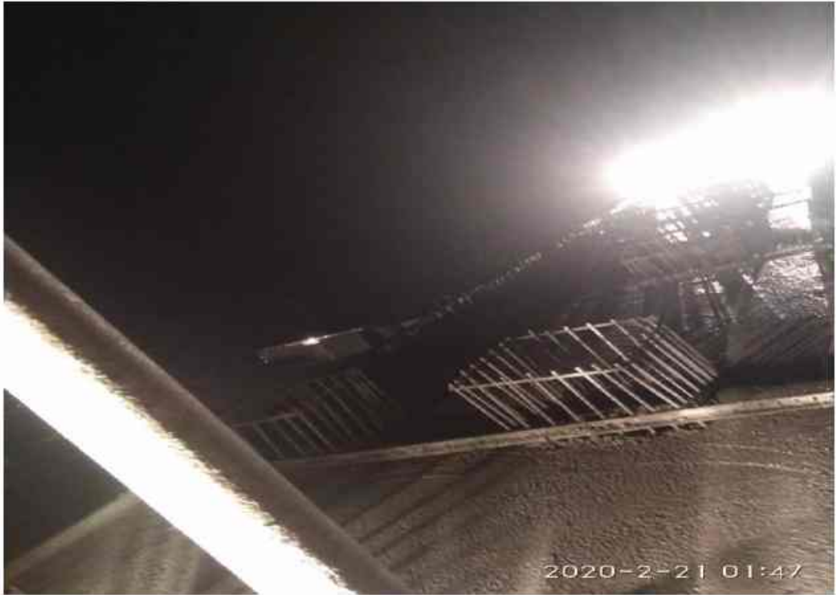
293+014 ROB pier cap LP5 concrete done
