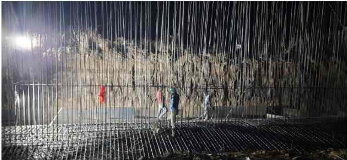
Mnb 313+808 A2 rhsraft concrete work in progress
