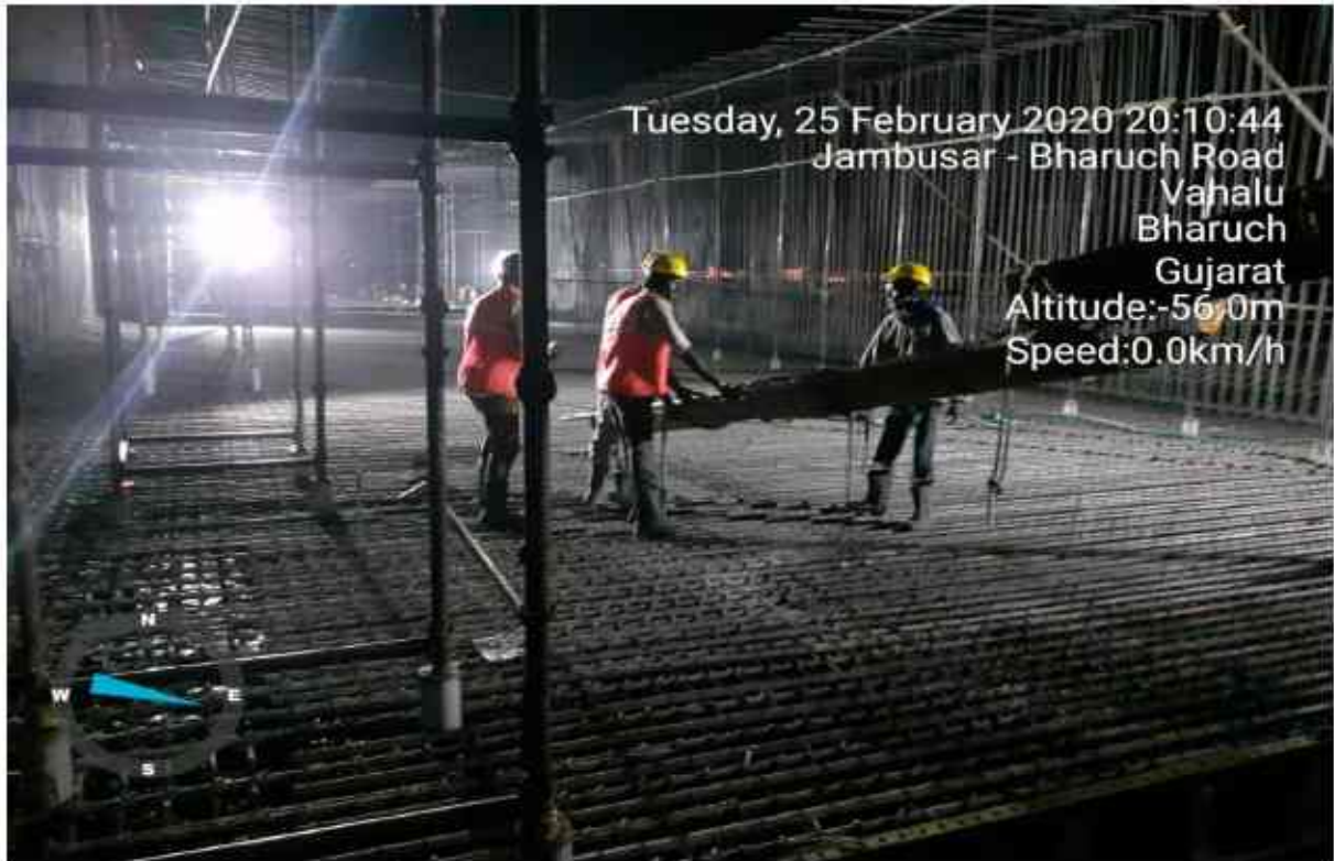
Raft concrete work in progress at ch 292+400
