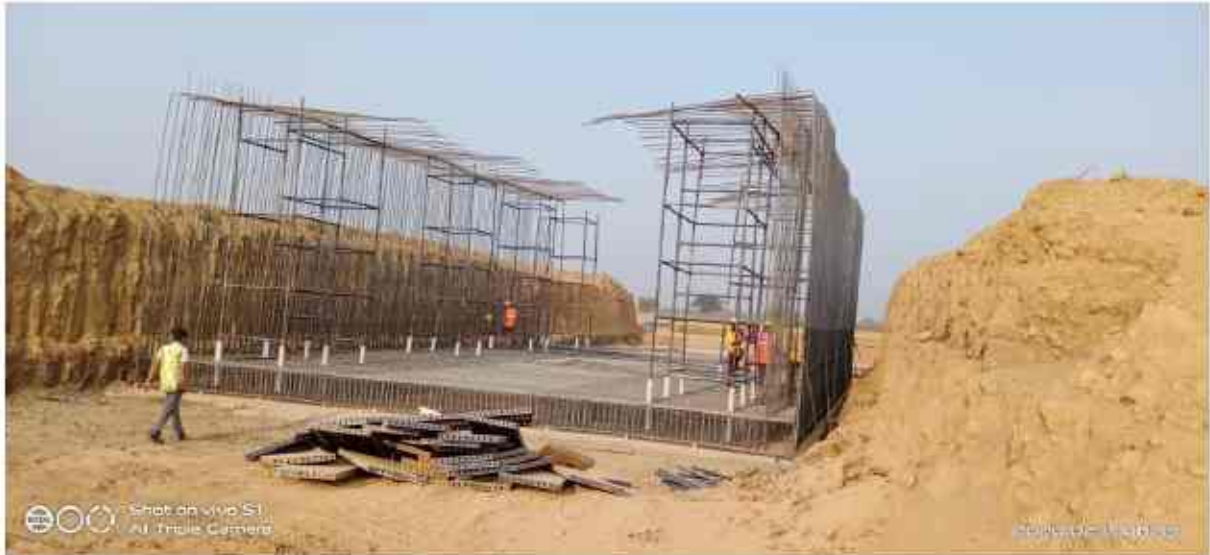
FUP raft Reinforcement in progress at ch-306+820(RHS)
