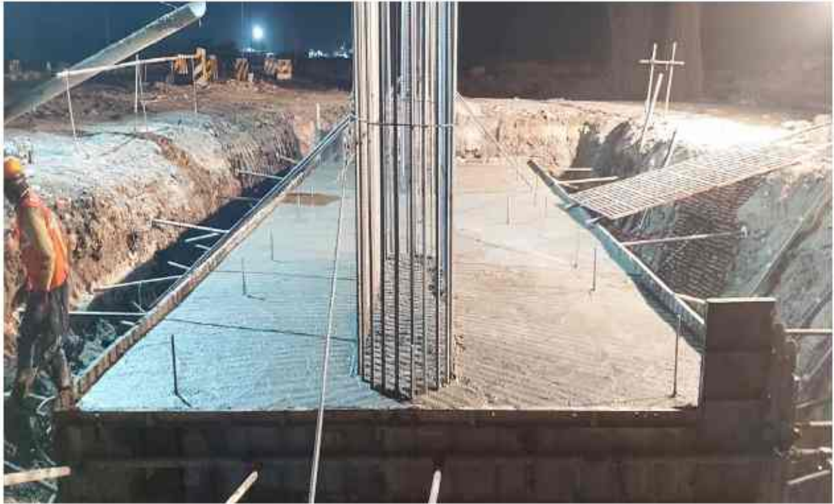
299+354 fly over pile cap P1 LHS concrete done
