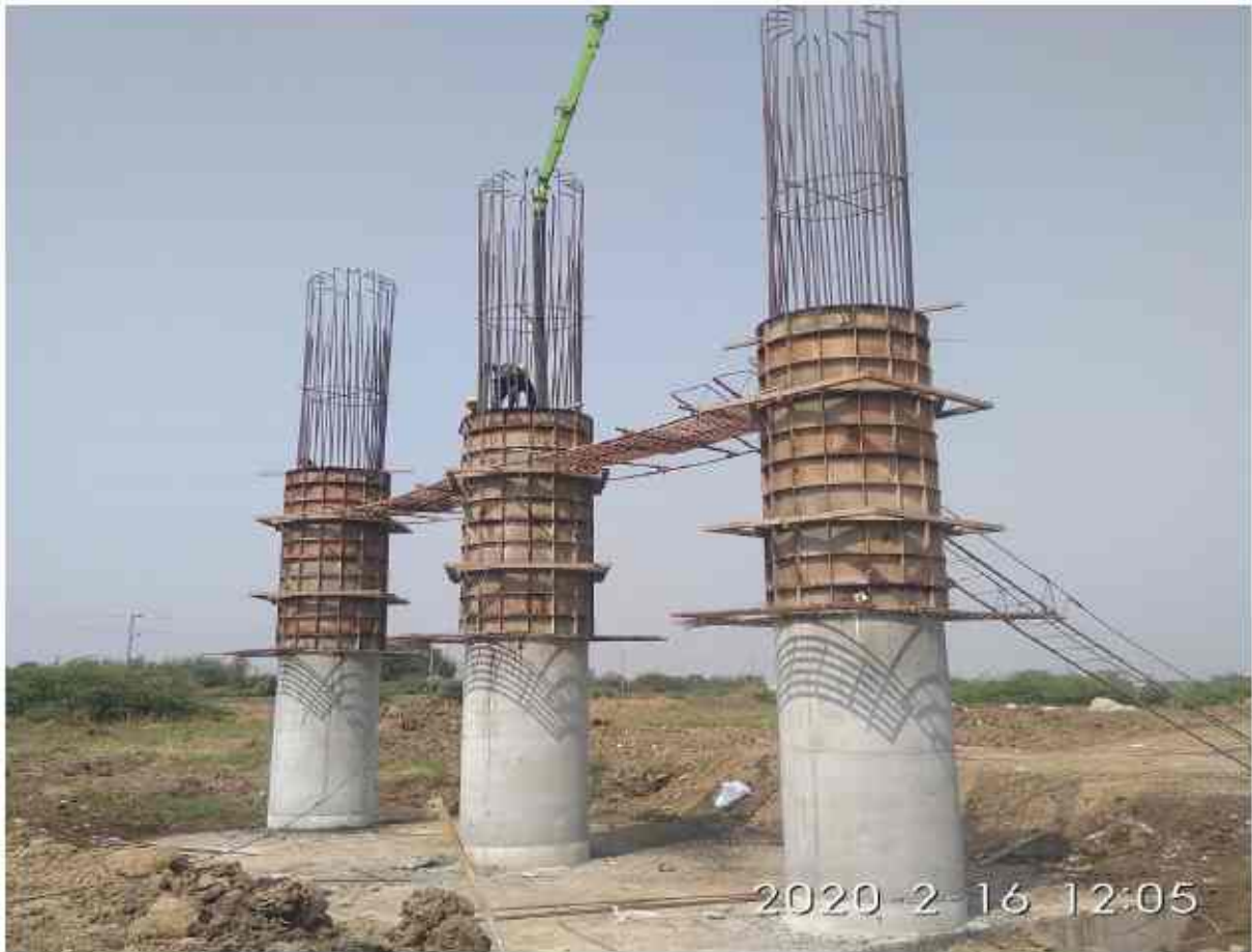
CH 293+014 ROBLP11 Pier shaft 3rd lift concrete pouring work in progress.
