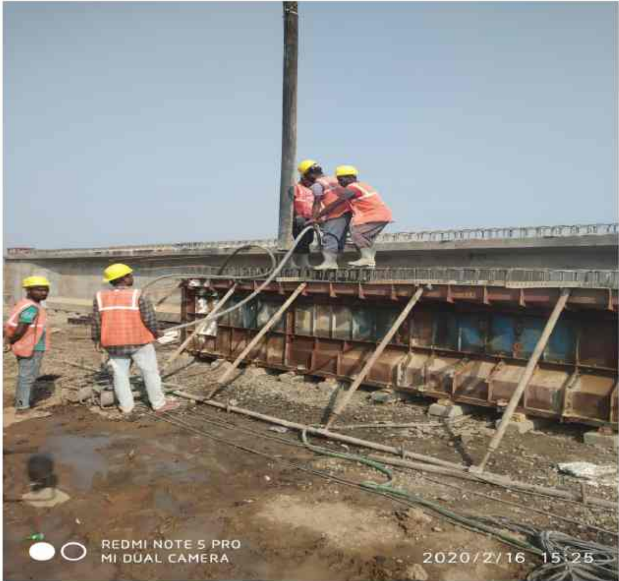
Concrete pouring PSC Girder p2a2 G7 LHSmjb 318+870
