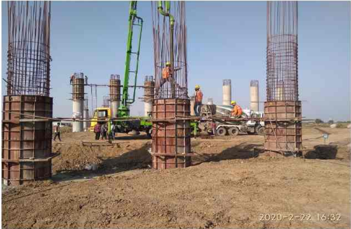
Ch 293+014 ROBLP10 Pier shaft 2nd lift concrete pouring work in progress
