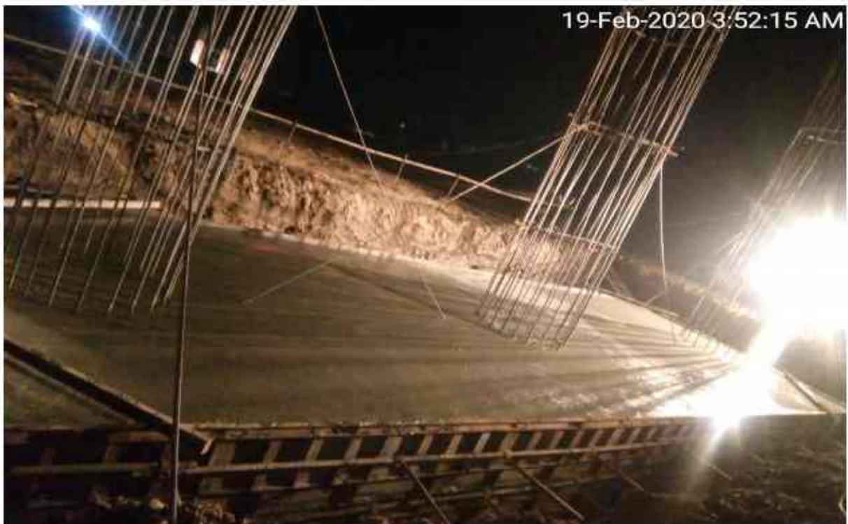
Complete concrete Ch-293+014, ROB-RA2, File cape.
