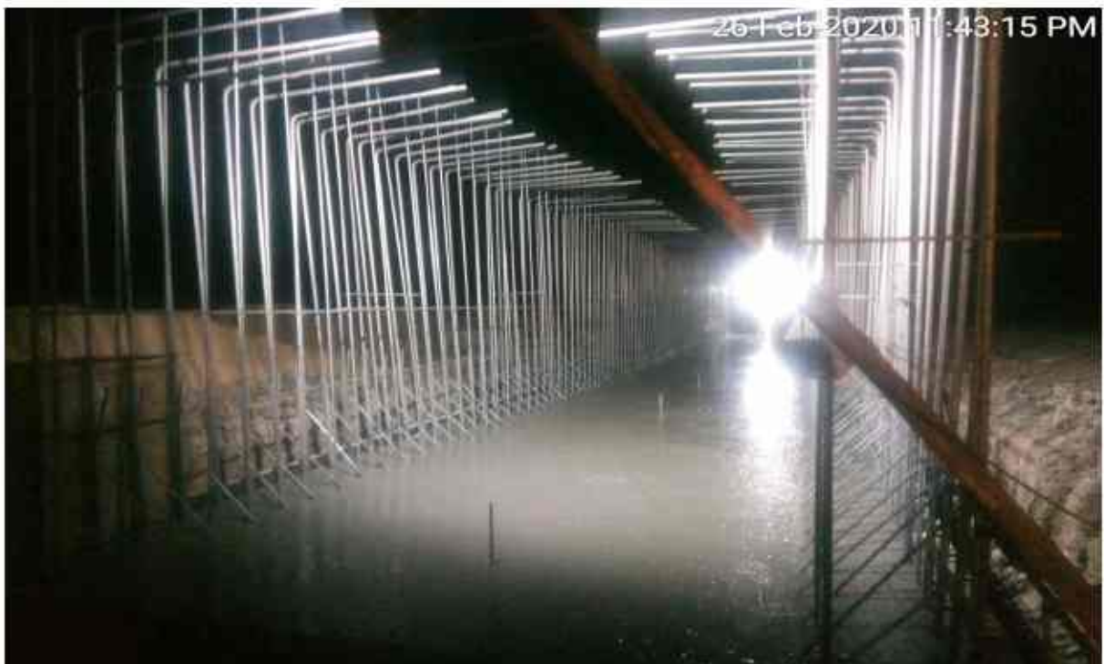
Completed Raft Concrete ch- 292+450,B.C,RHS.
