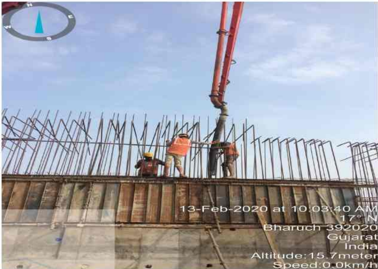
Ch-301+790 pup LHS A1&A2 2nd lift pouring work start
