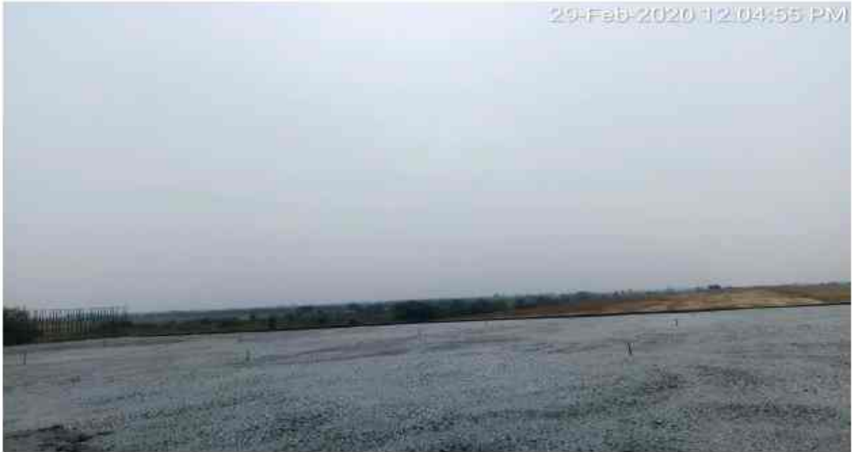
Ch-303+220 R H SFUP Top slab concrete pouring completed.
