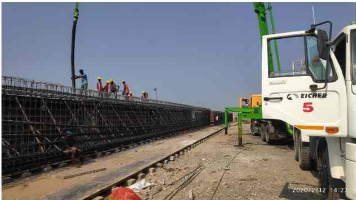
321+253.Mjb.lhs.p1-a2 span.G-3 girder casting is in progress.
