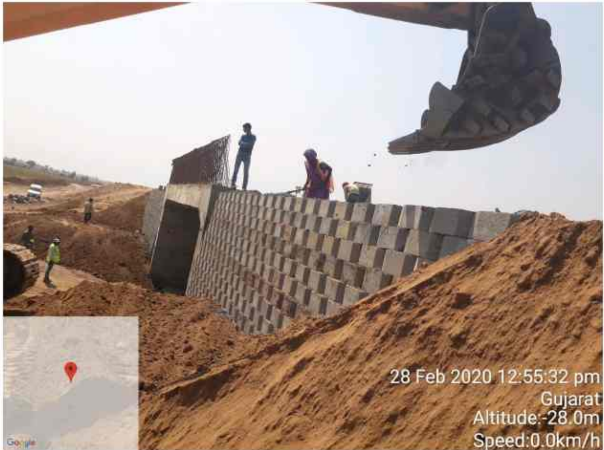
306.060 Retwall block Complete, A1&A2 SDE
