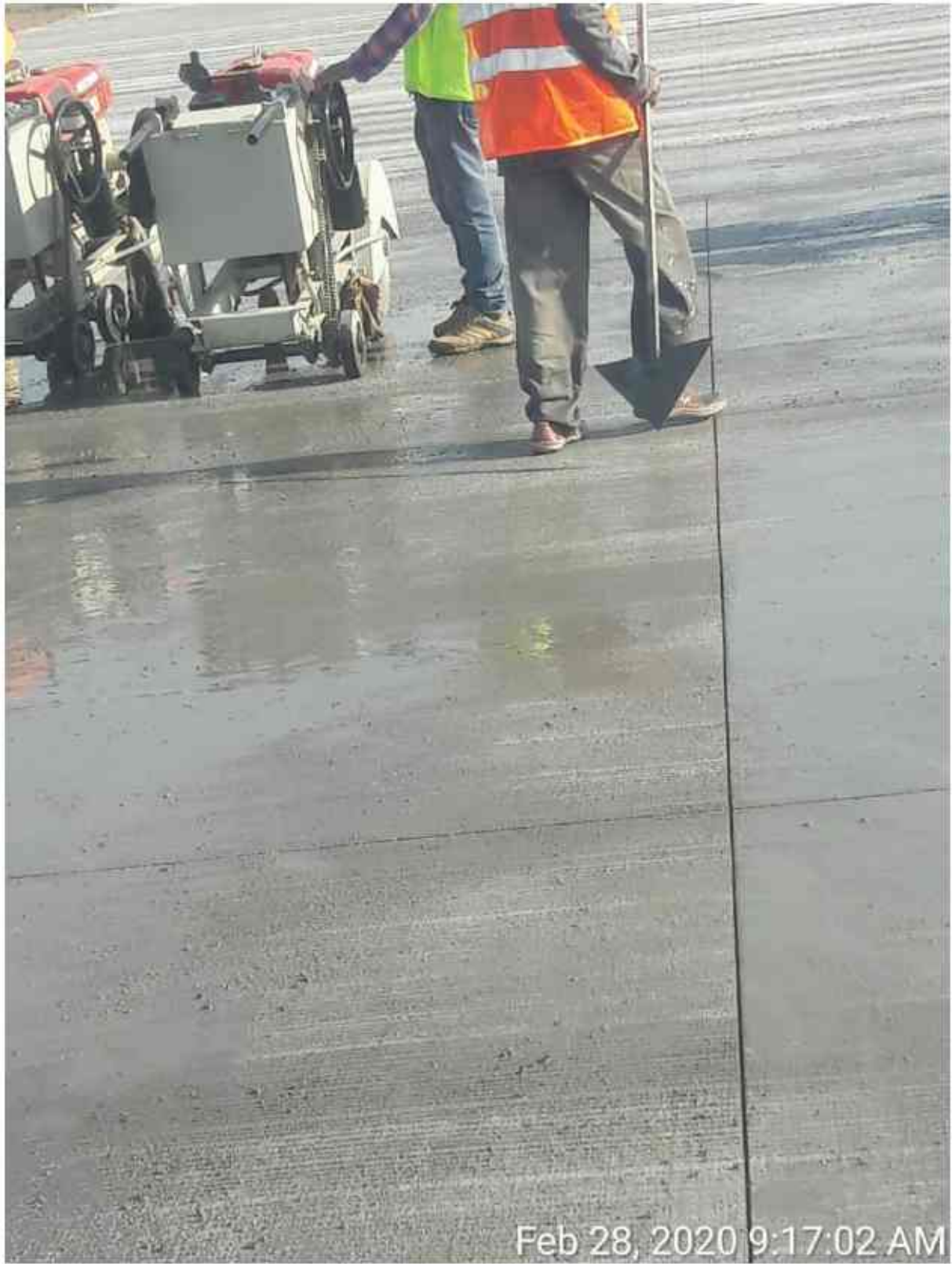
First cutting in progress(1)
