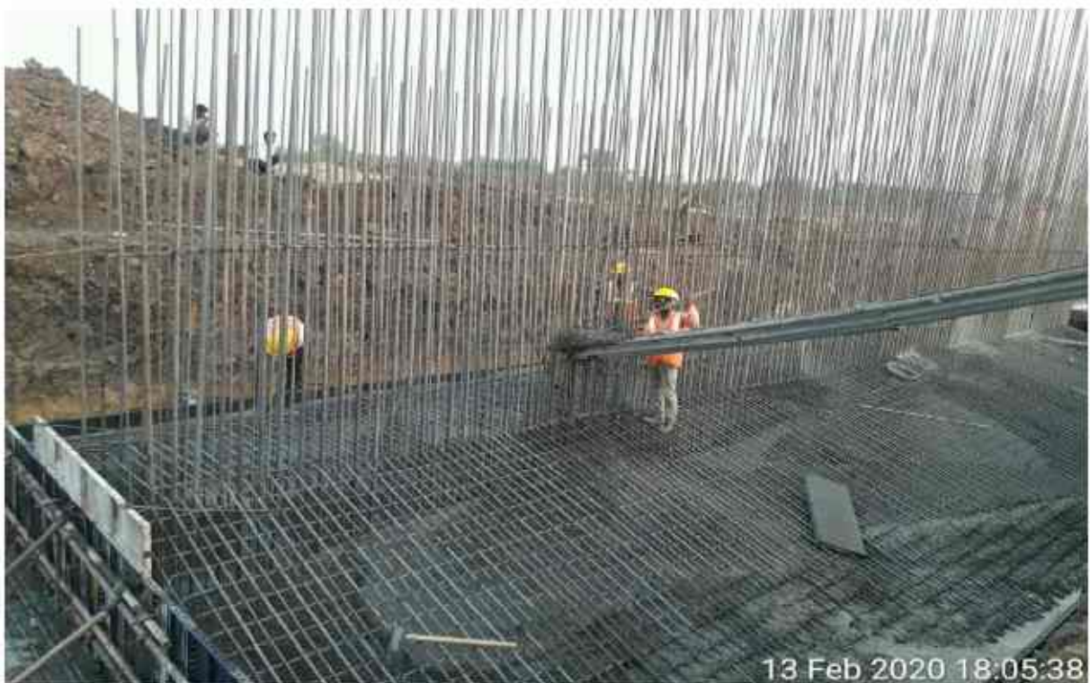
Retaining wall raft concrete is in progress from ch 322+750 to 322+770 r.h.s
