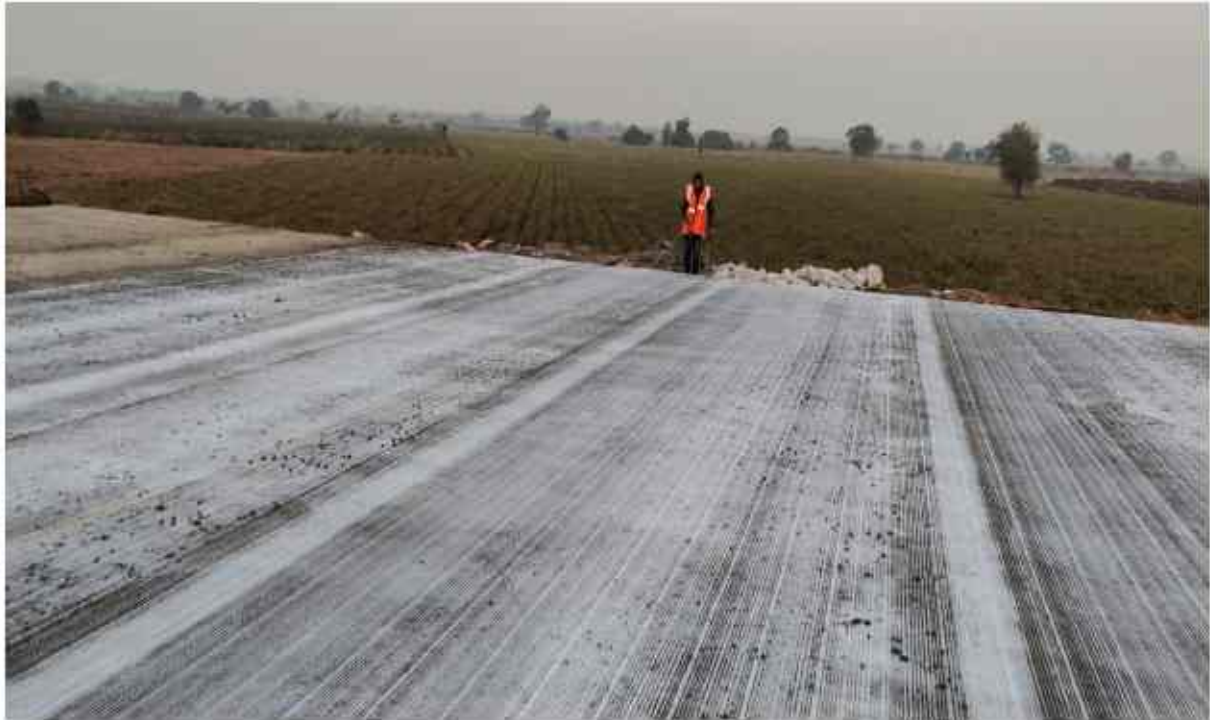
First cutting in progress Ch - 304+650 to 304+700 lhs(1)
