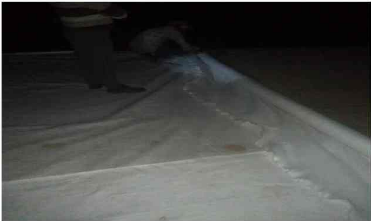
Geo textiles laying all completed.
