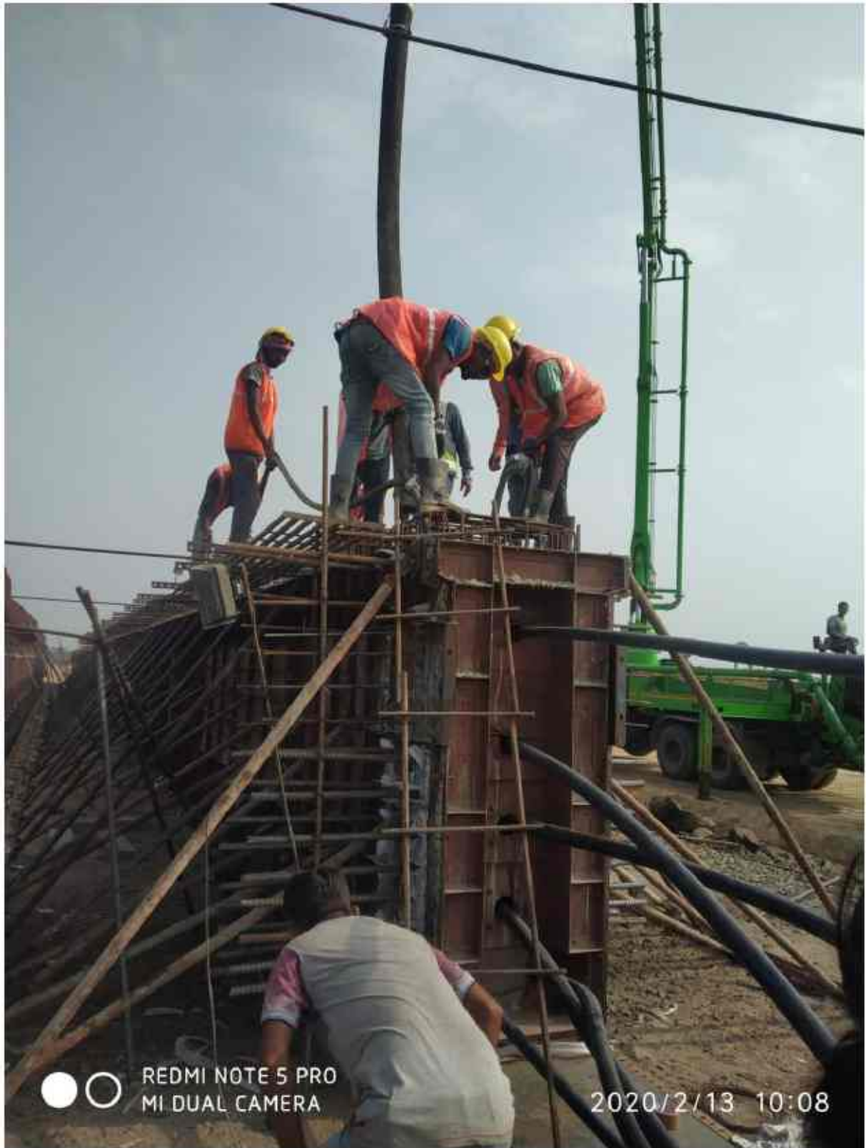
Concrete pouring PSC Girder G4 RHS307+733
