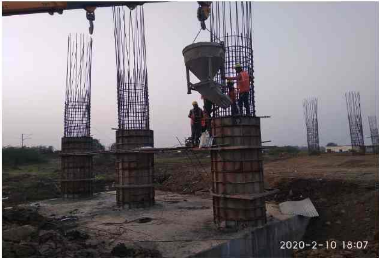
CH 293+014 ROBLP11 Pier shaft 2nd lift concrete Pouring work in progress
