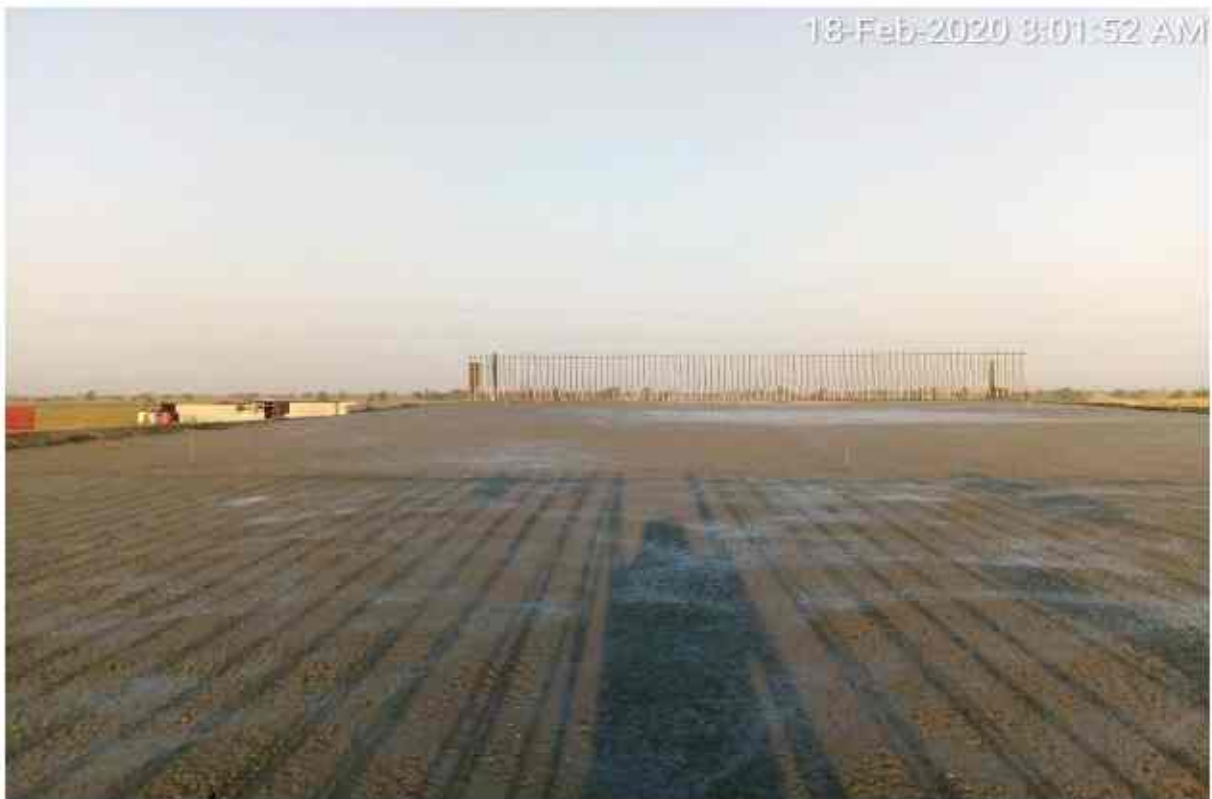
Completed, Concrete Top slab, RHS, LVUP, 308+550.
