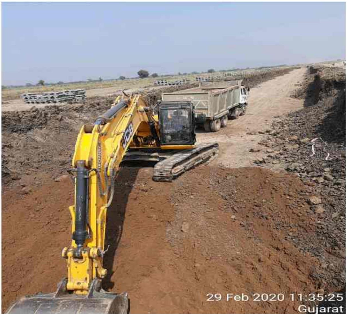
Excavation started in wall 5 at 299+375 flyover
