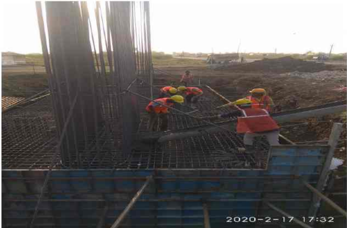
299+354 fly over pile cap P1 LHS concrete start
