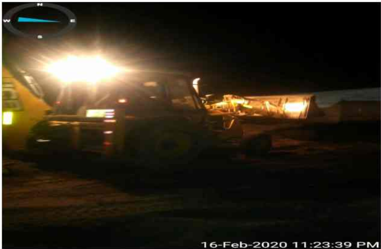
305+ 850 mow filing Re wall A2 side
