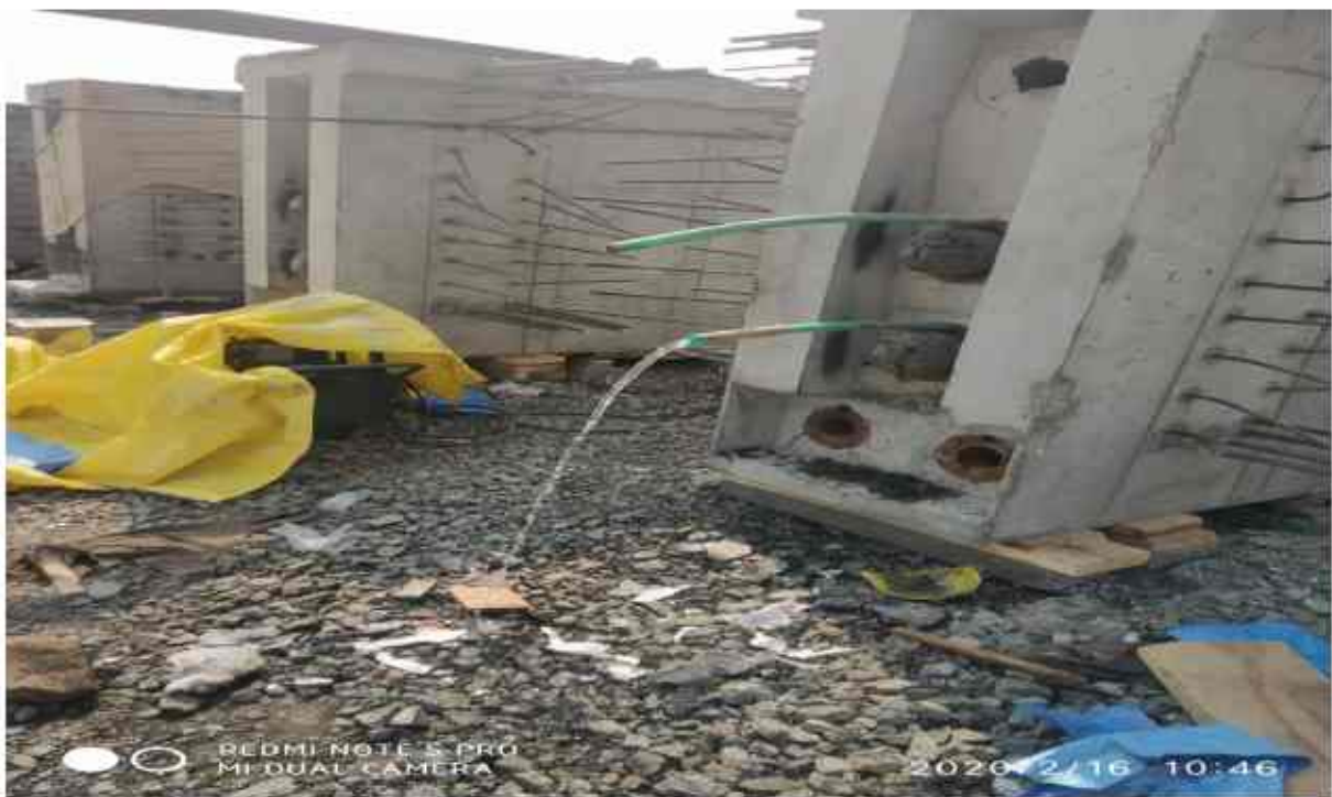
Lime water washing for 318+870 G5 girder p1p2 RHS
