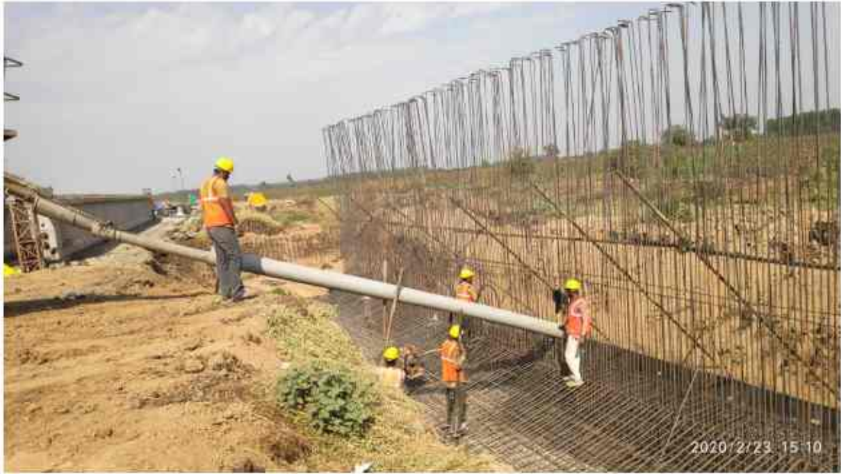
318+930.rhs.retaining wall raft concrete is in progress.
