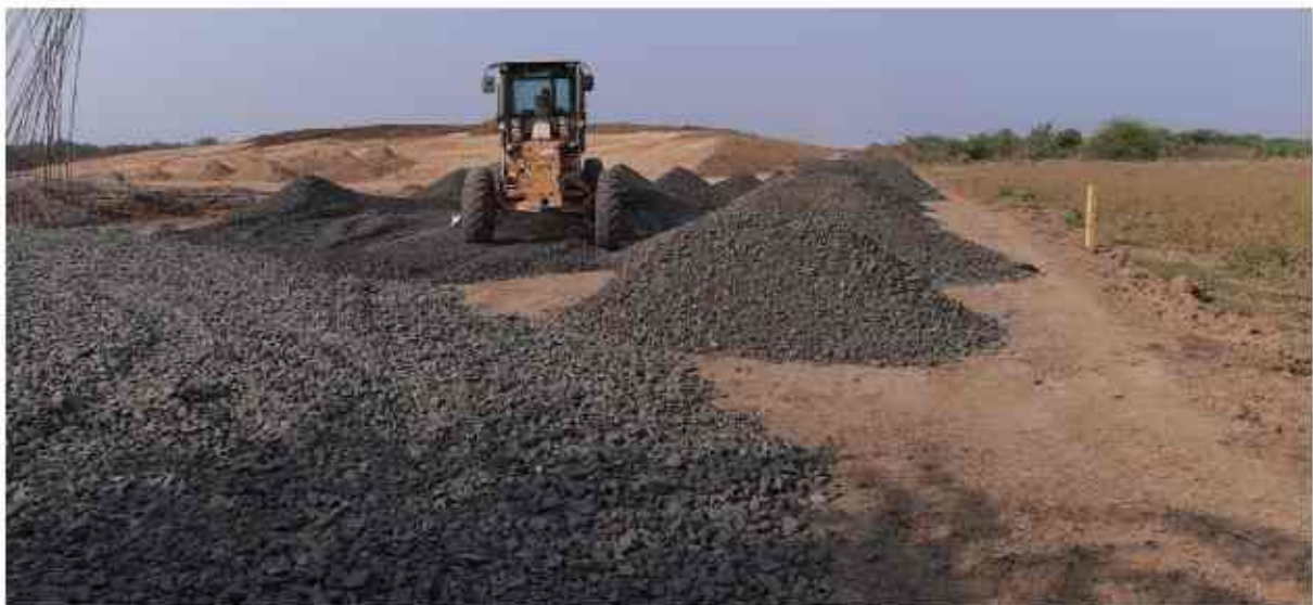
GSB spreading for girders bed at ch 313+808, work in progress.
