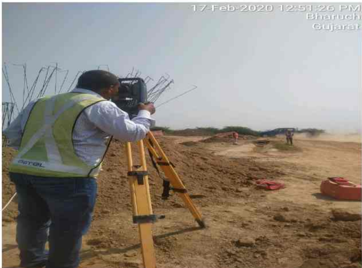
BOX CULVERT LAYOUT CH- 309+818.757 BHS(1)
