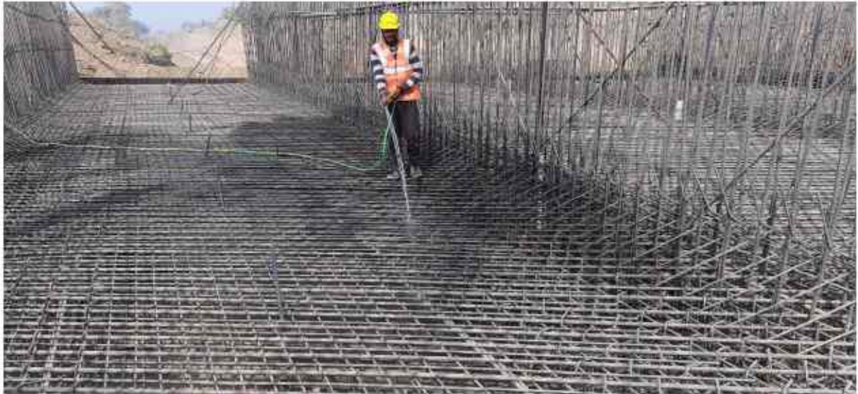
Dust is cleaning before the concrete program, at ch 314+314 MNBraft lhs
