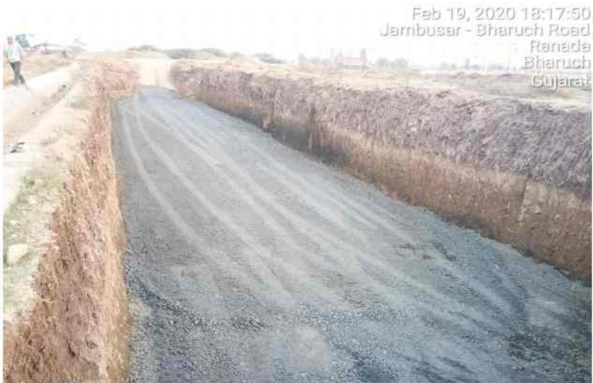
At Chainage no 309+840 MNBA2 BHS bed is prepare for rolling.
