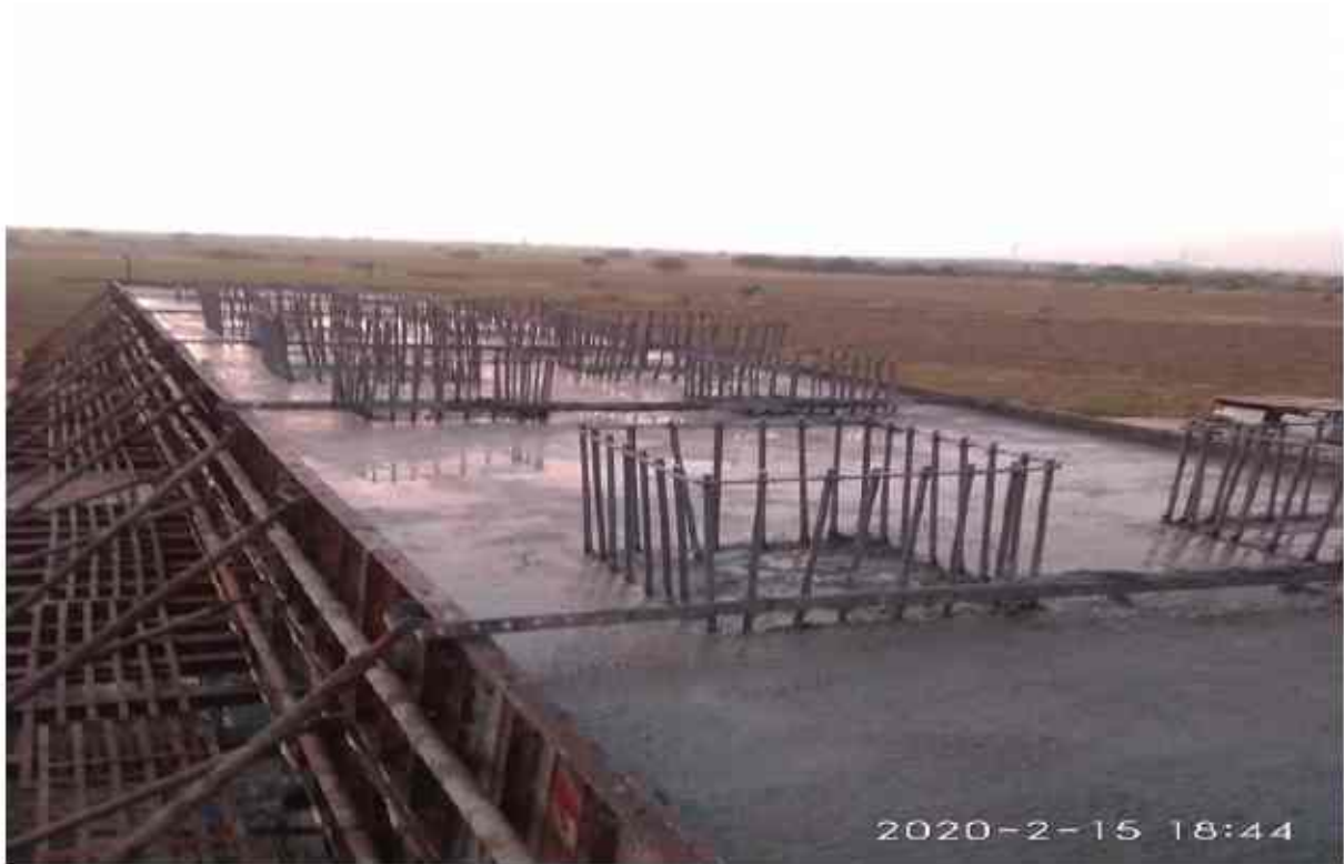
CH 293+014 ROBLP4 Pier cap complete.
