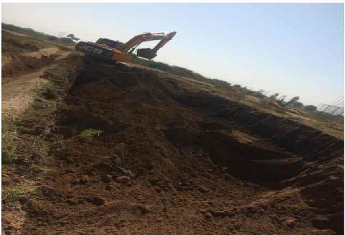
Ch-309+840 MNBBHSA2 side excavation work in progress
