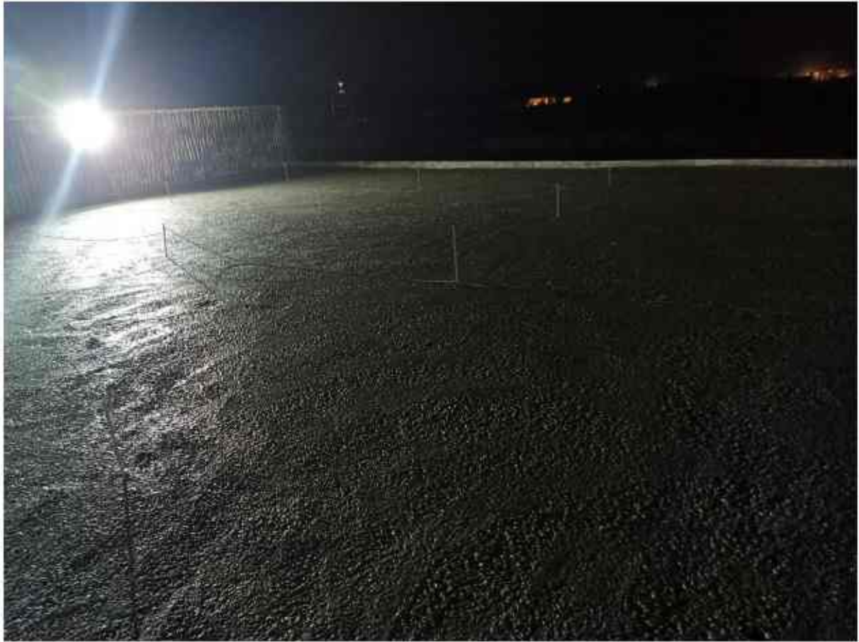
294+085 mnbLhs slab concrete complete
