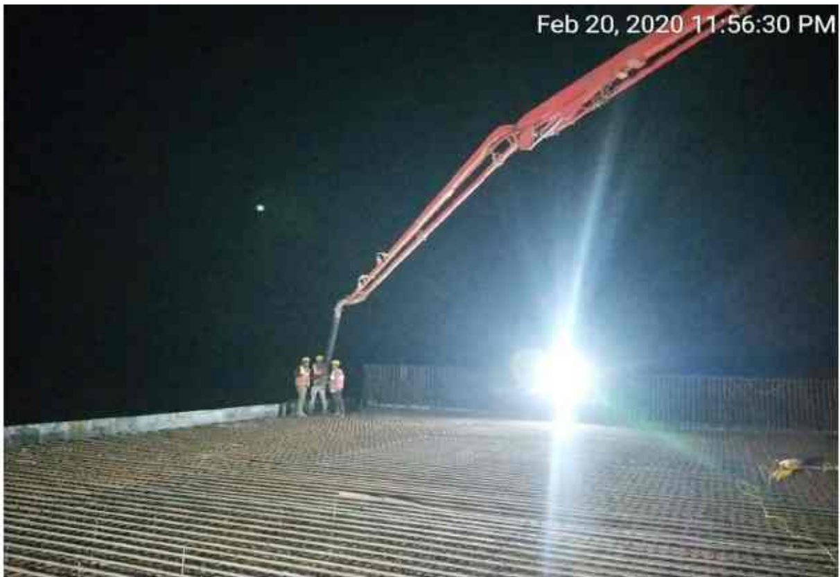
Ch-319+580 pup rhstop slab casting work in progress
