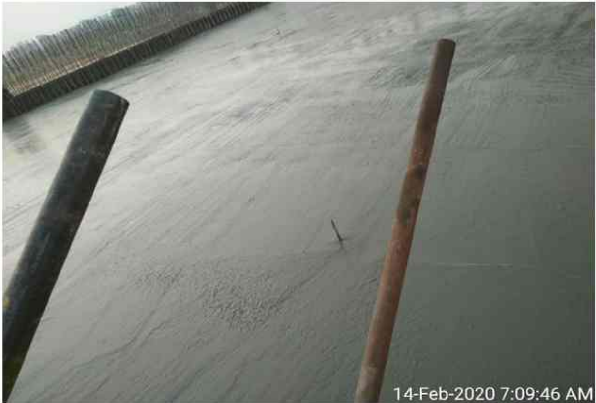
At ch-310+480 pup LHS slab concrete completed
