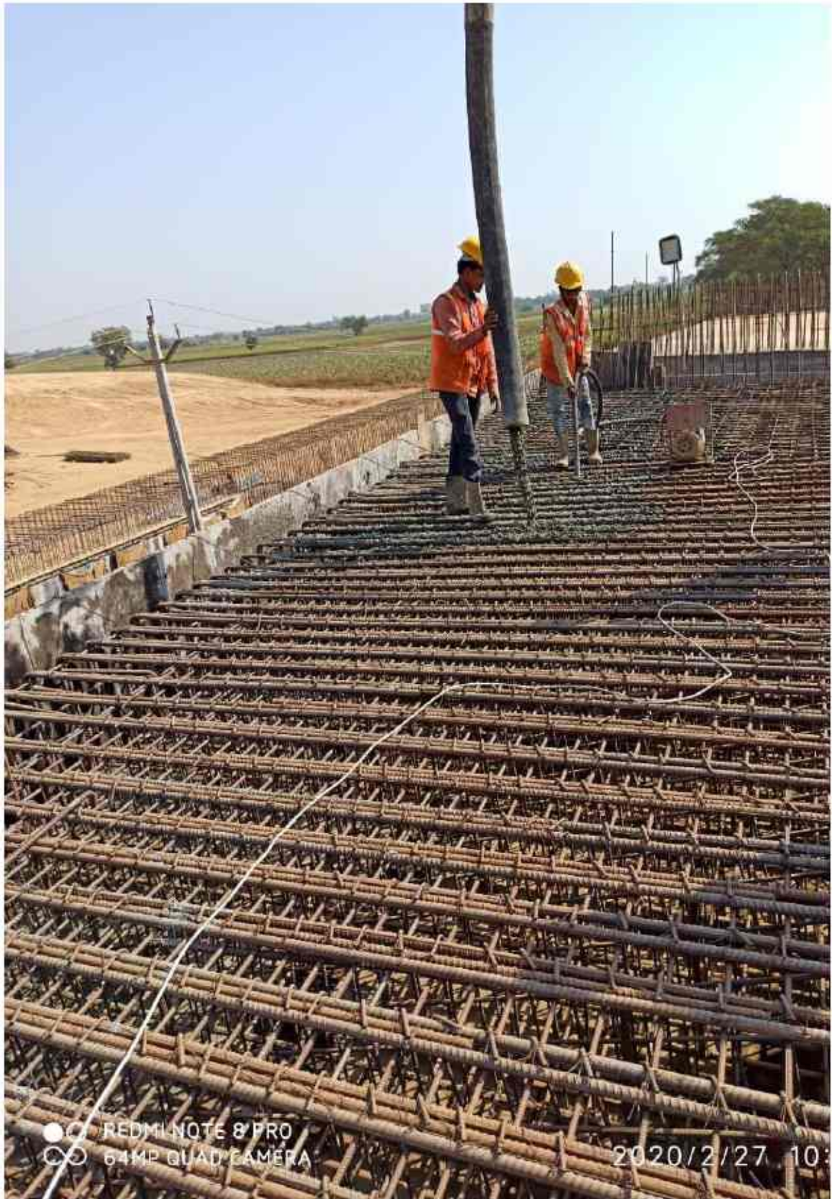
316+536 Lvup LHS slab casting work in progress
