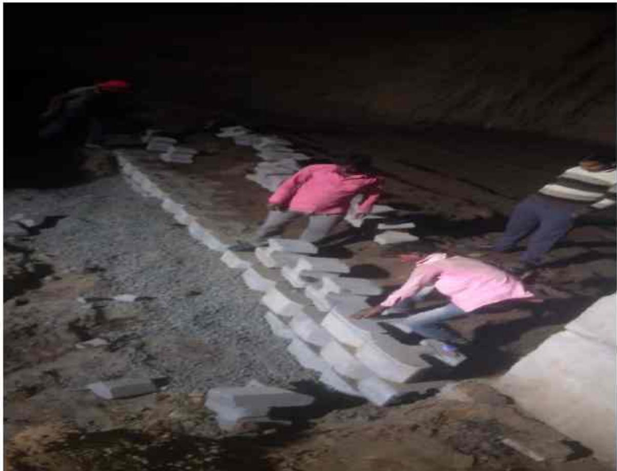
Block Erection CH- 306+060Wall 4
