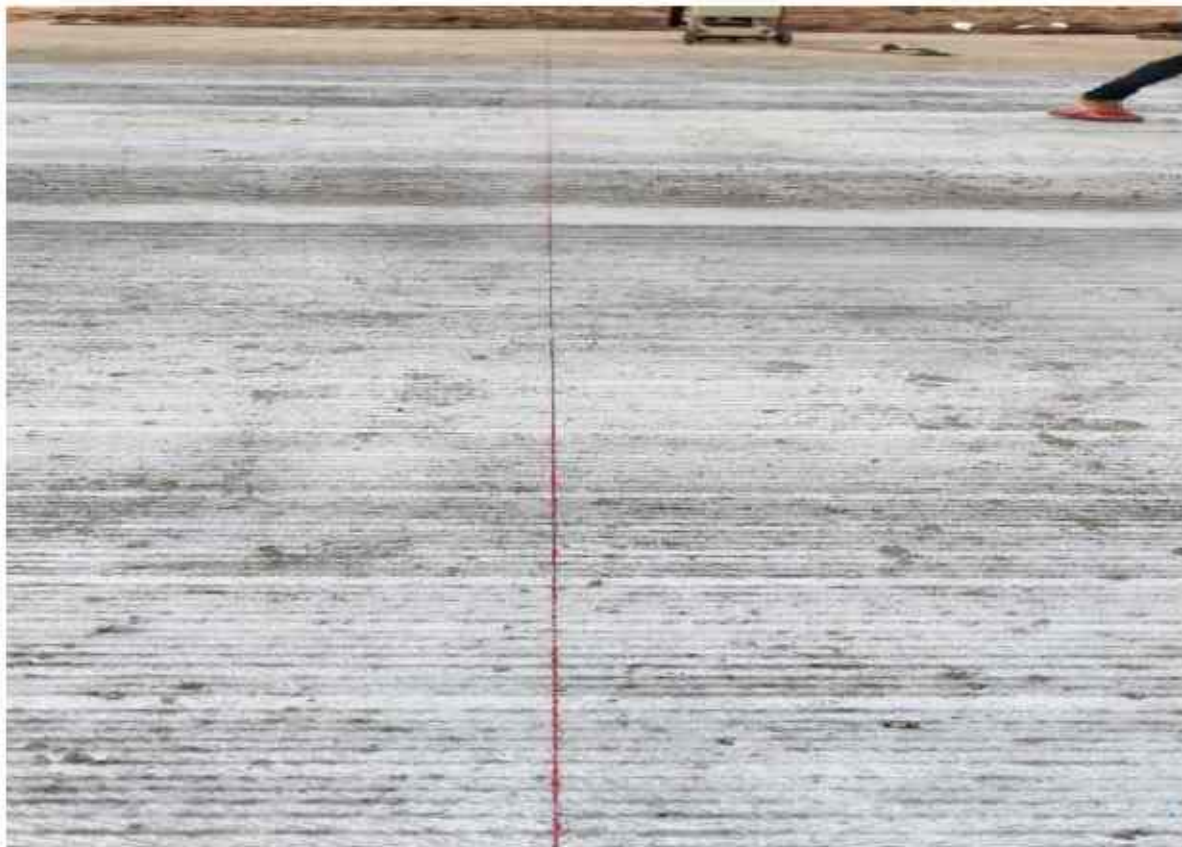
First cutting in progressCh - 304+650 to 304+700 lhs
