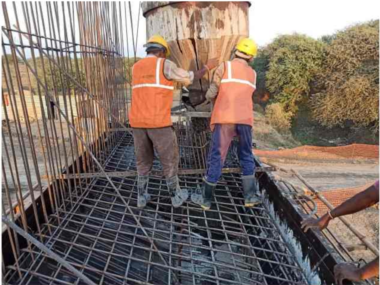
Mnb 297+562 A2 rhs abutment cap concrete start
