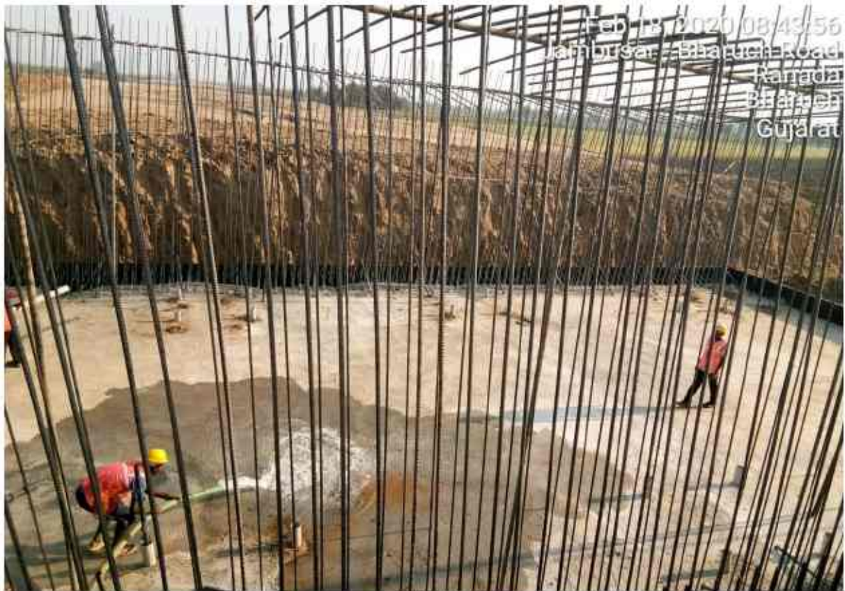
Raft curing in progress at Chainage no 306+820 pup RHS
