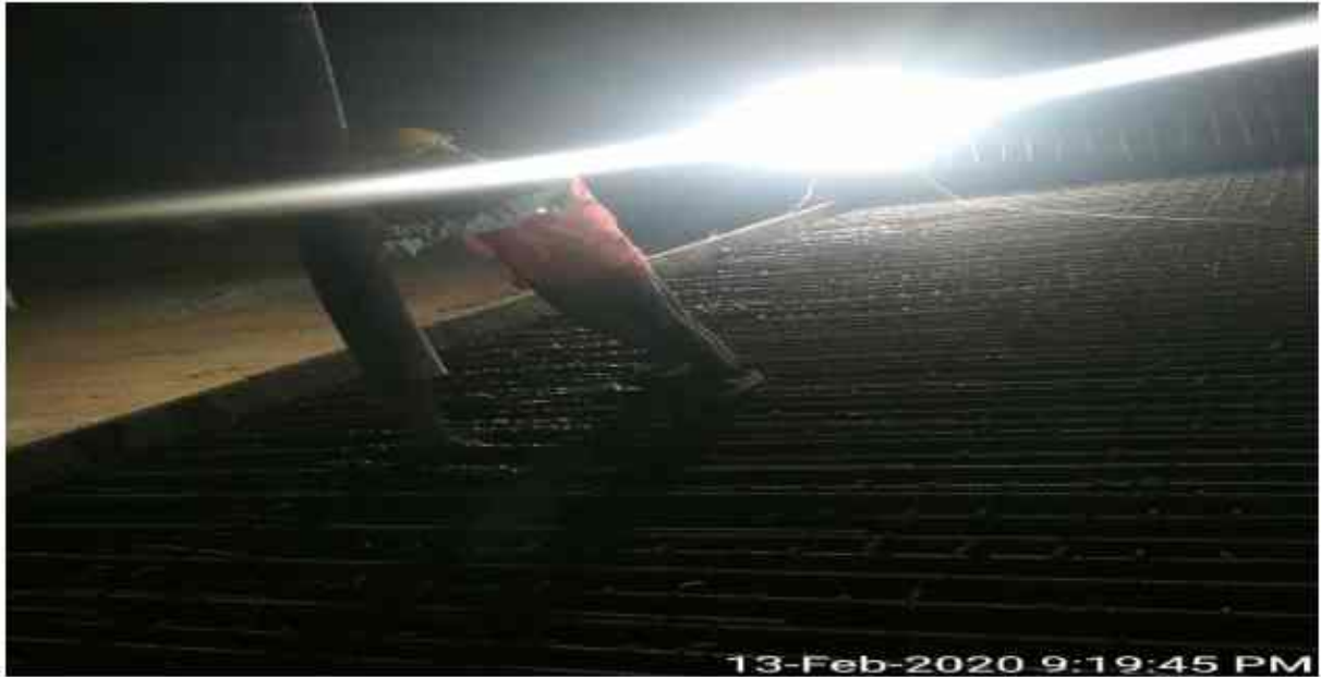
Concrete in progress at ch-310+480 pup lhs slab
