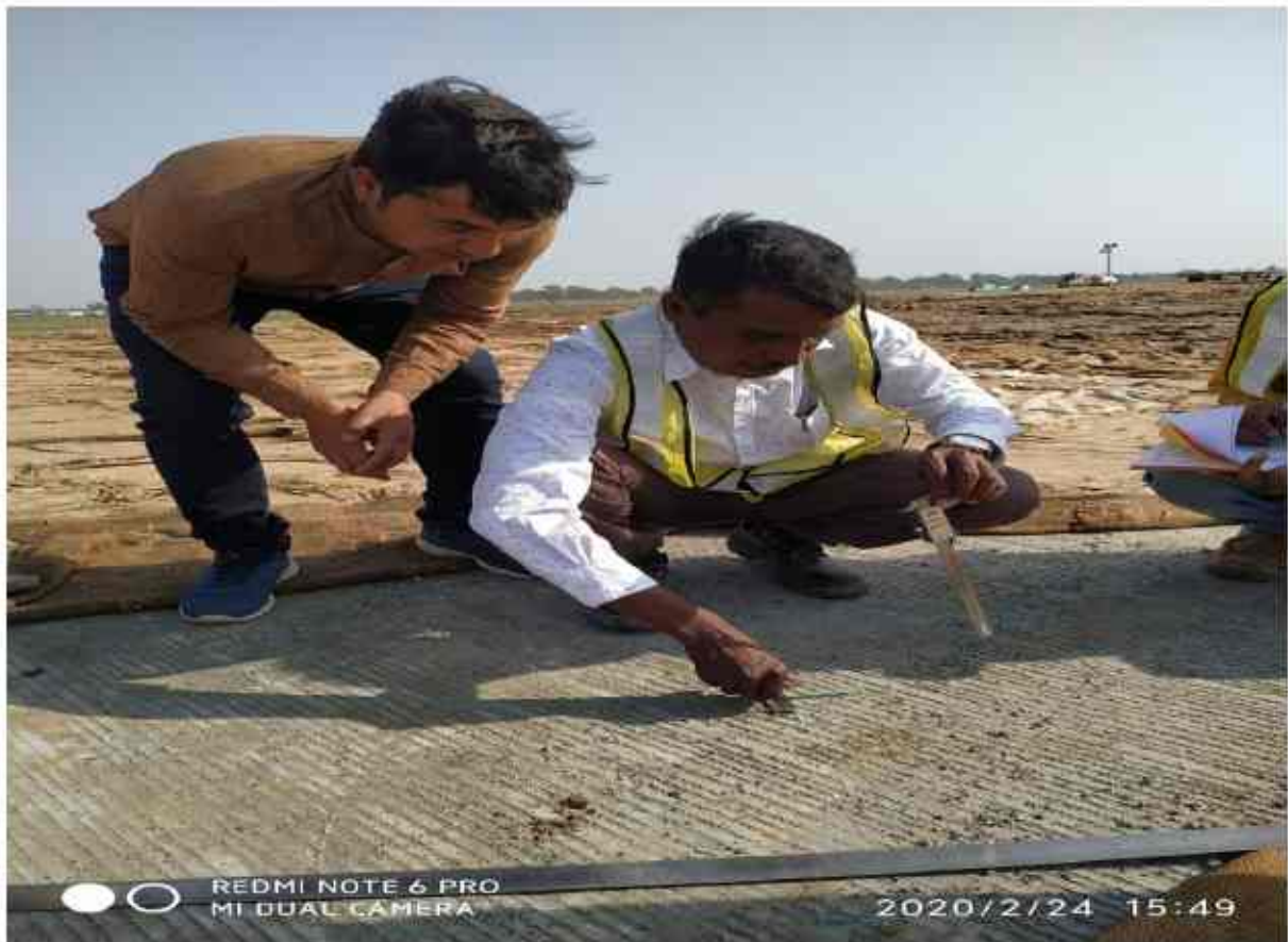
Texture test of PQC pavement(2)
