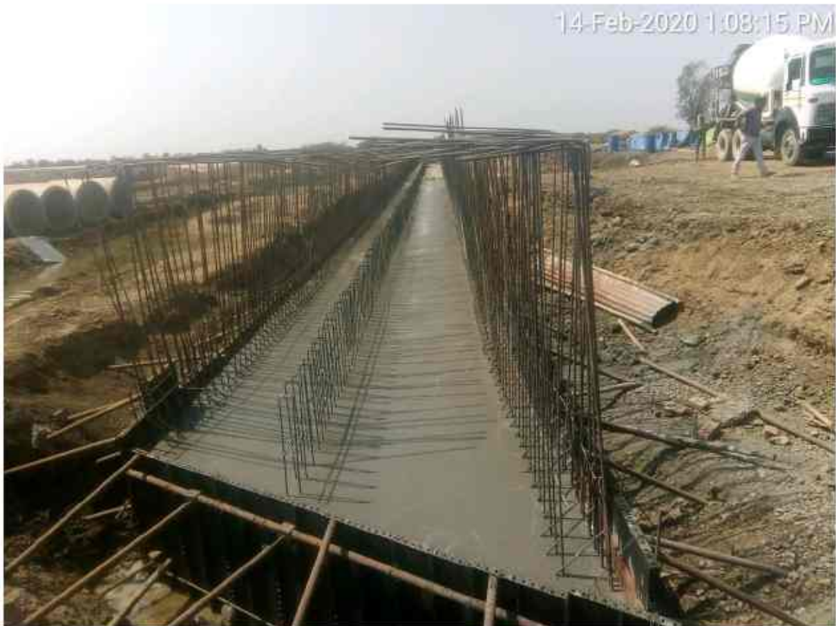
Completed Raft Concrete,307+687, RHS,box culvert.
