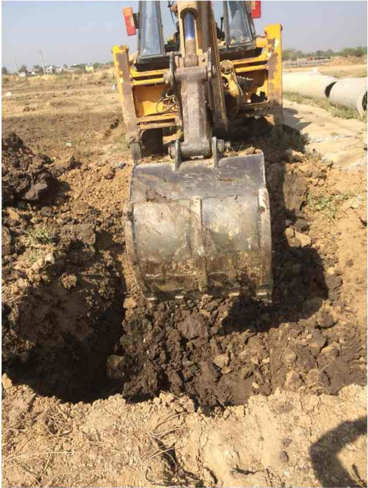
Utility excavation work start at ch-299+400
