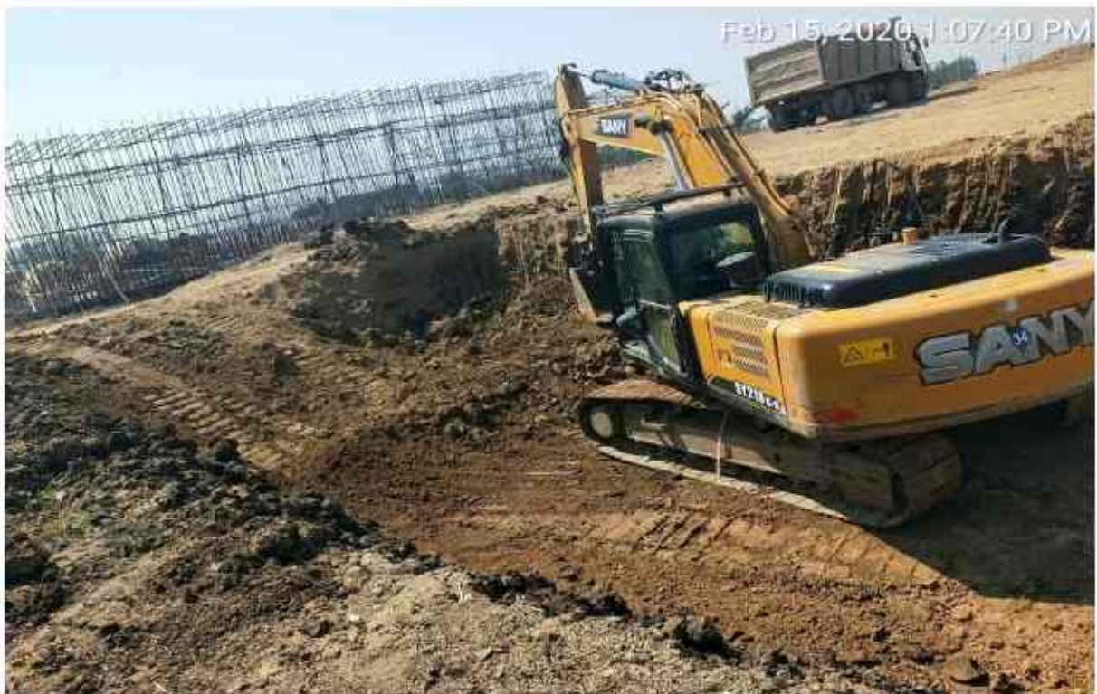
Ch-322+570 to 322+590 rhs retaining wall excavation (w.p)
