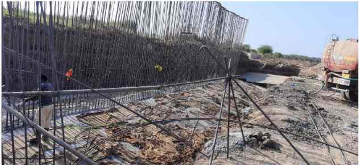
Curing at 313+808 MNBraft
