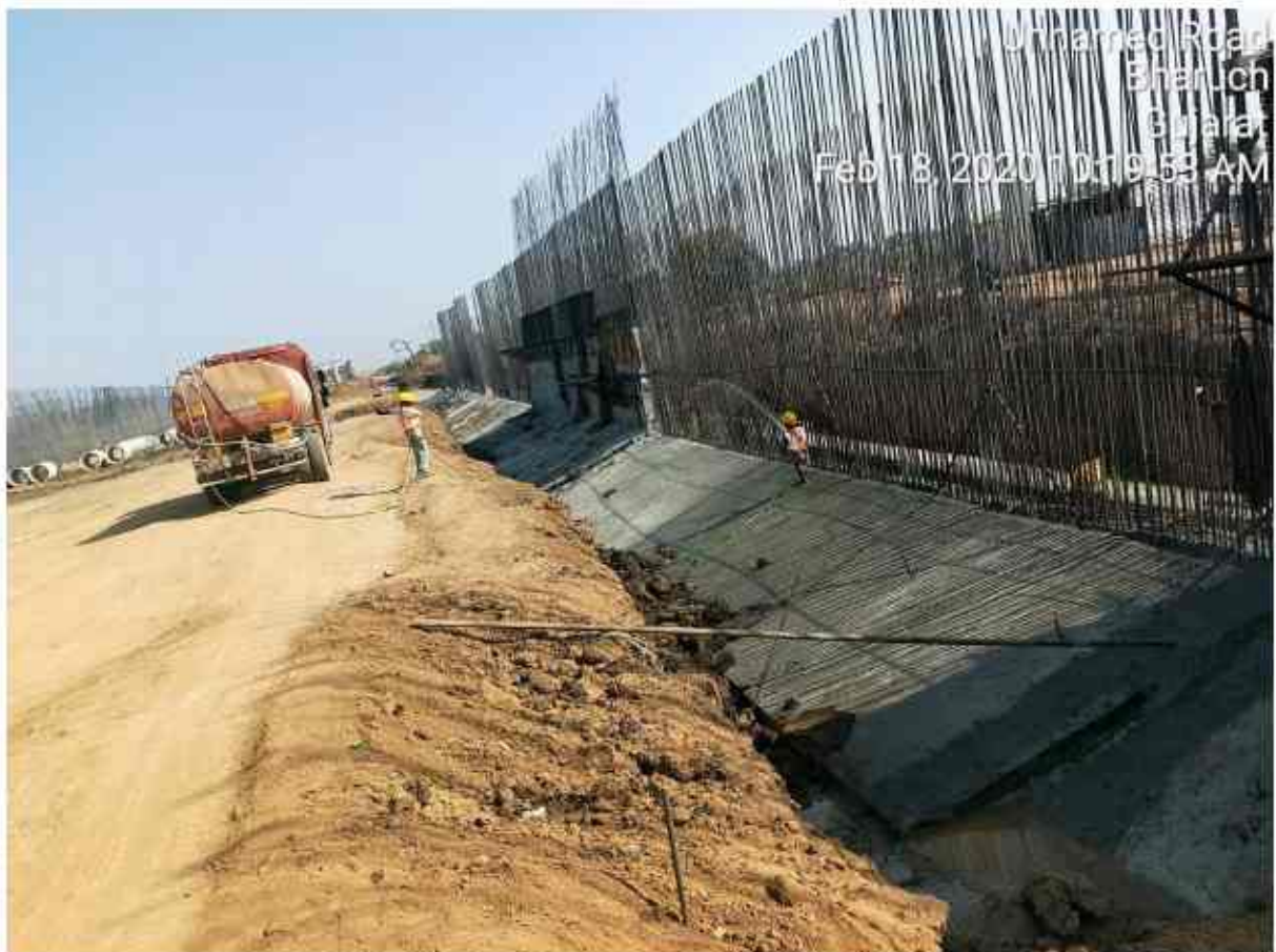
Raft curing in progress at Chainage no 306+820 pup RHS
