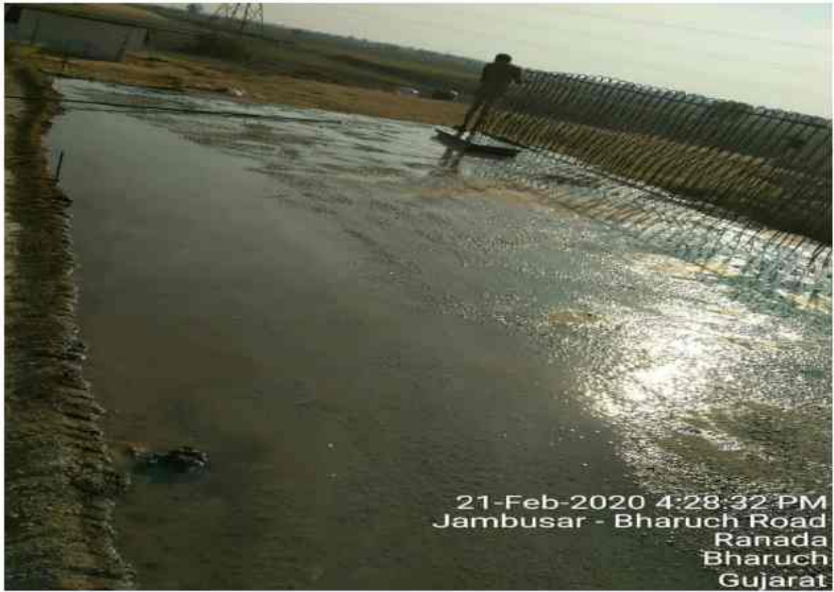
Curing in progress at ch-308+550 pup slab rhs
