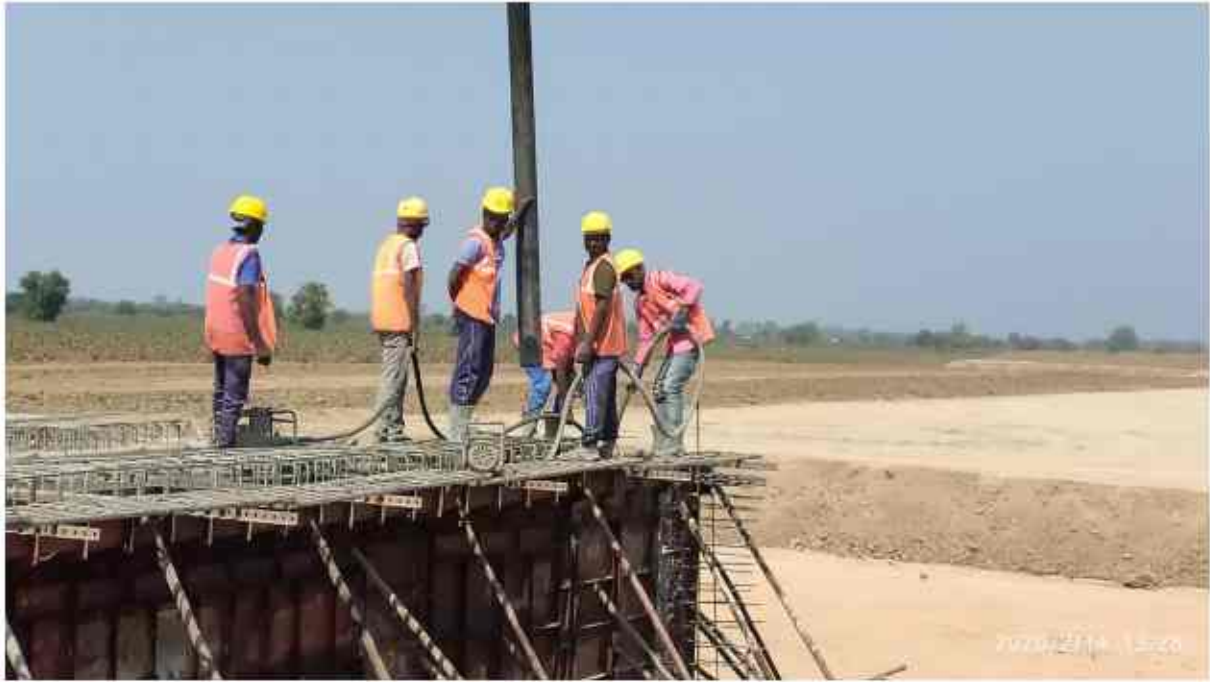
Concrete pouring PSC Girder G3 span PIP2 LHSmjb 318+870
