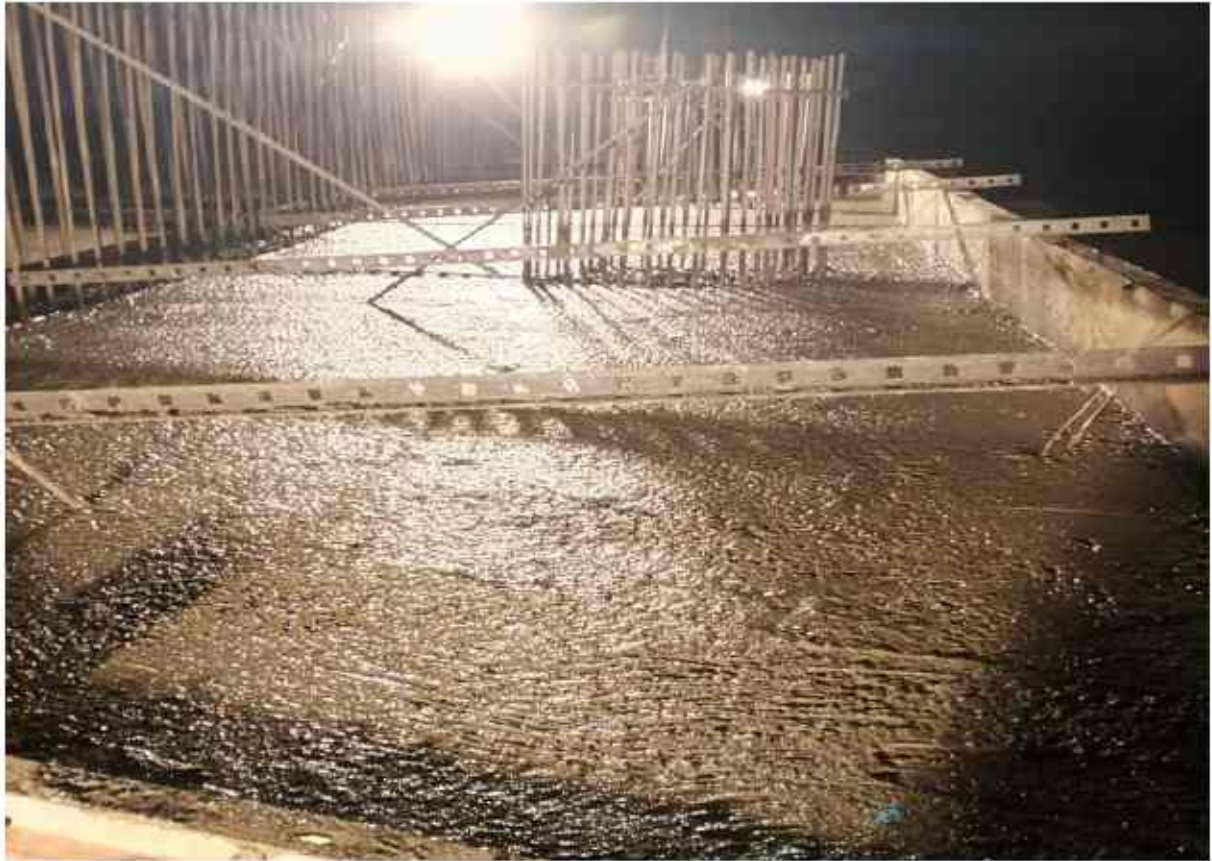
297+562 mnb A2 rhs abutment cap concrete complete
