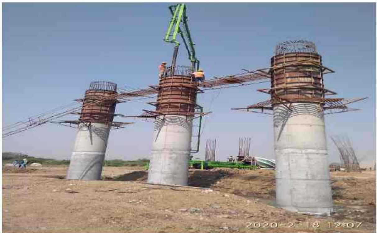
CH 293+014 ROBRP12 Pier shaft final lift concrete Pouring work in progress.
