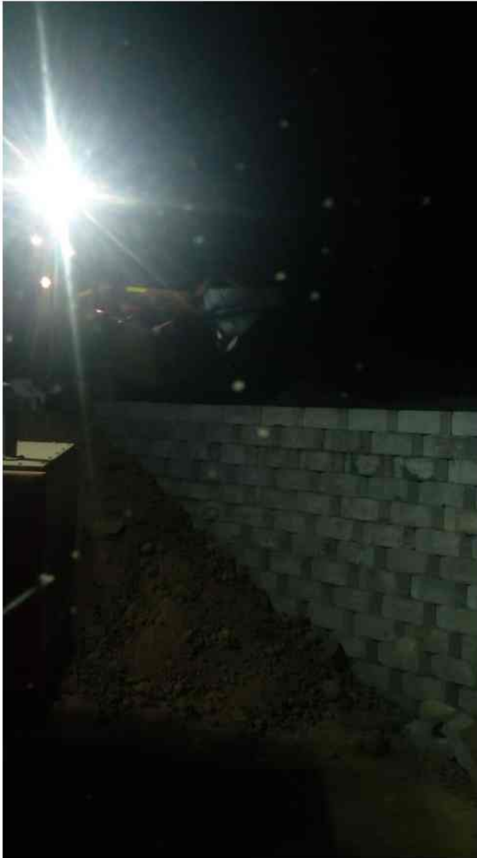
305+ 058 Re wall Block Erection wall 4
