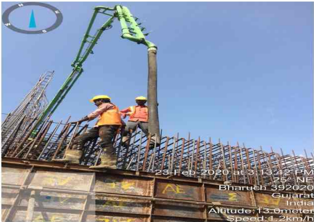
Ch-303+220 pup RHSs A1&A2 final lift wall pouring work start.
