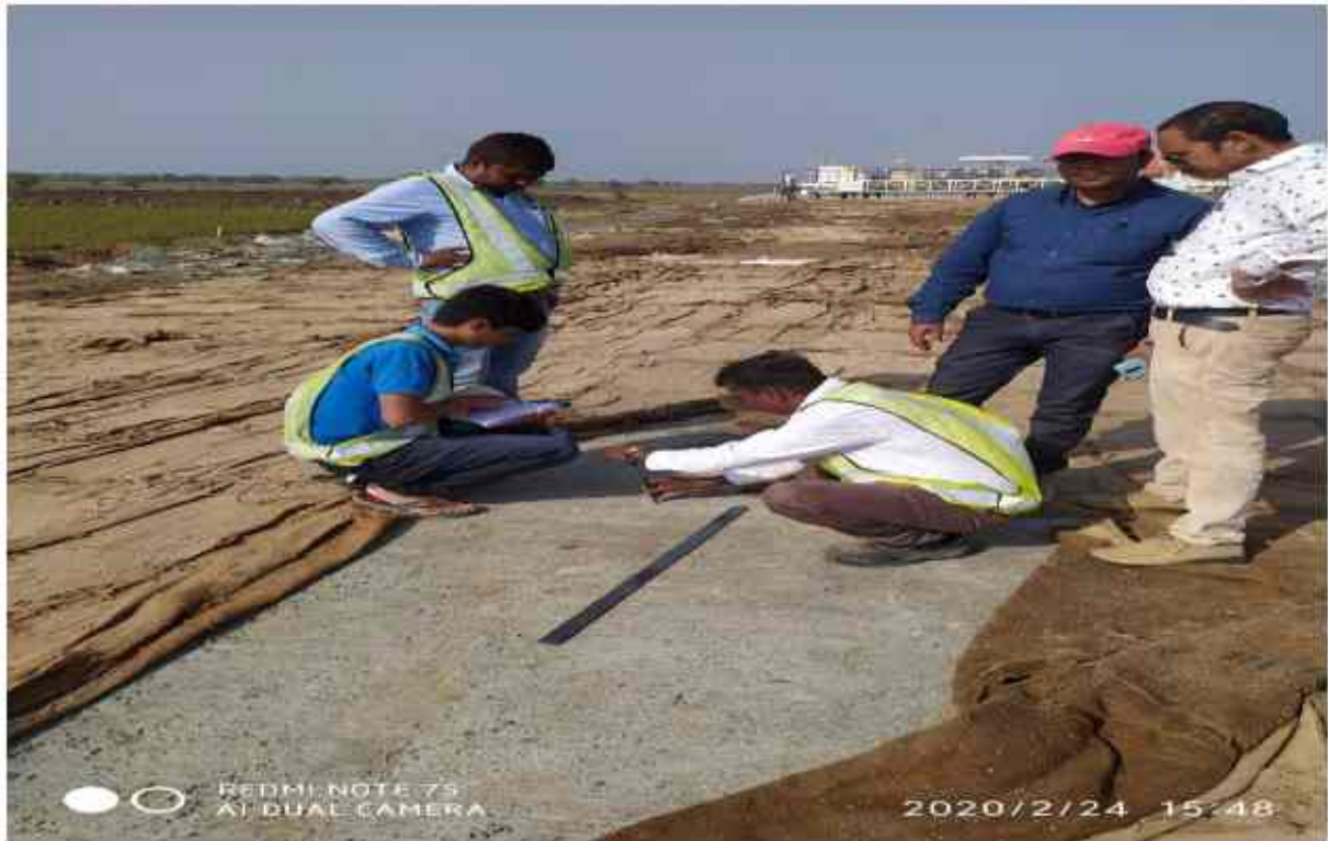
Texture test of PQC pavement (3)
