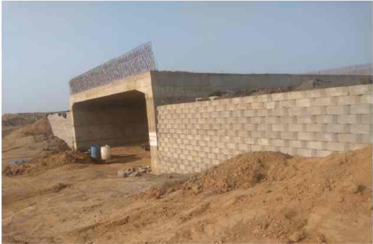
505+058 Re wall Block Erection 22 layer A1 &A2 side
