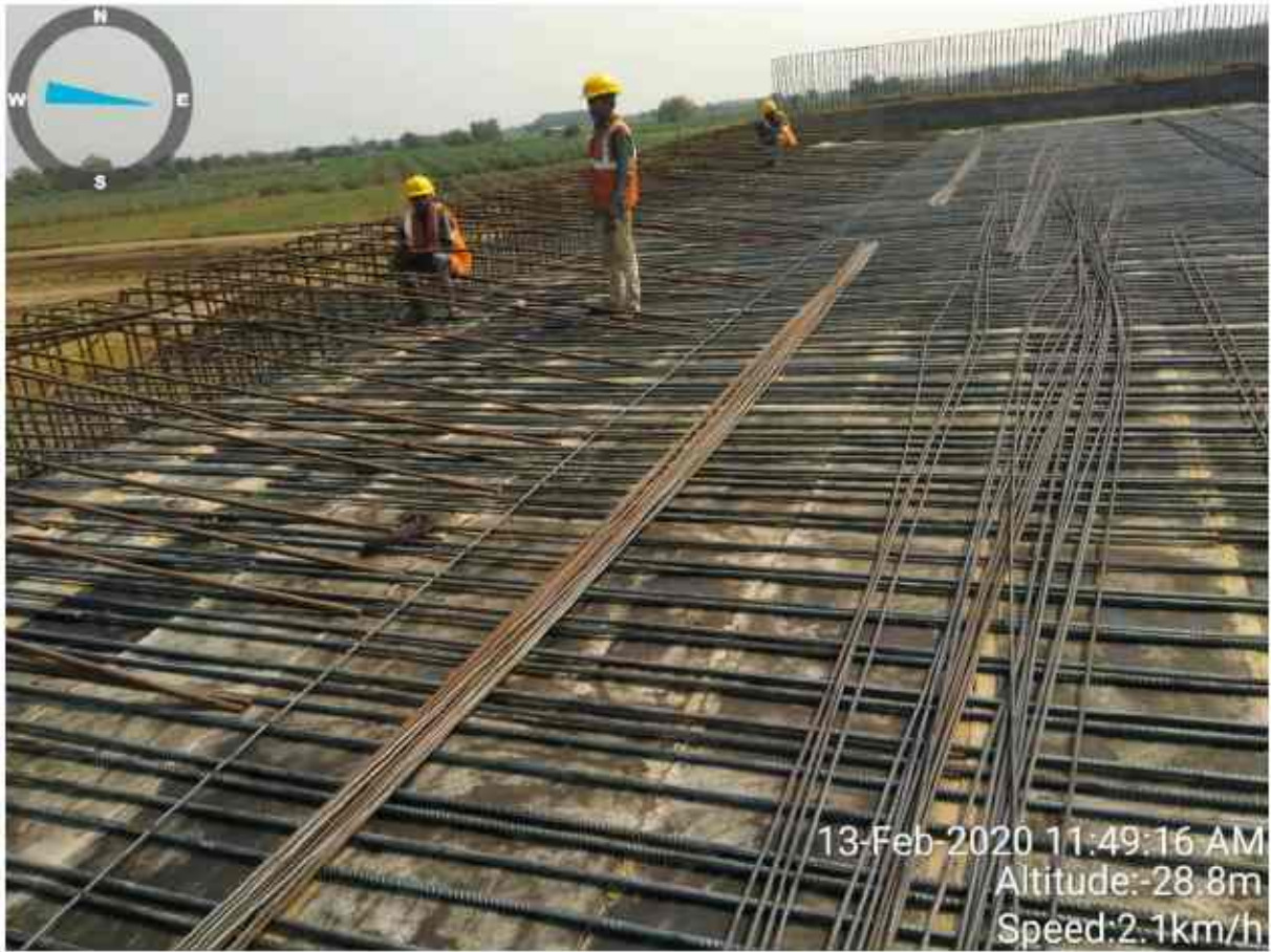
FUP at ch 320+825 Lhs top slab reinforcement work in progress.
