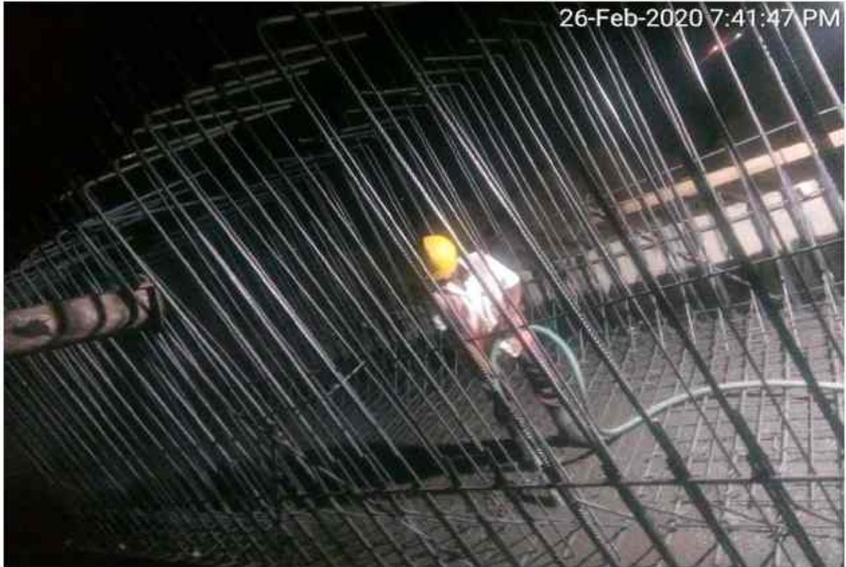
Ch-292+450,Box culvert,RHS,Raft Concrete Pouring Progress.
