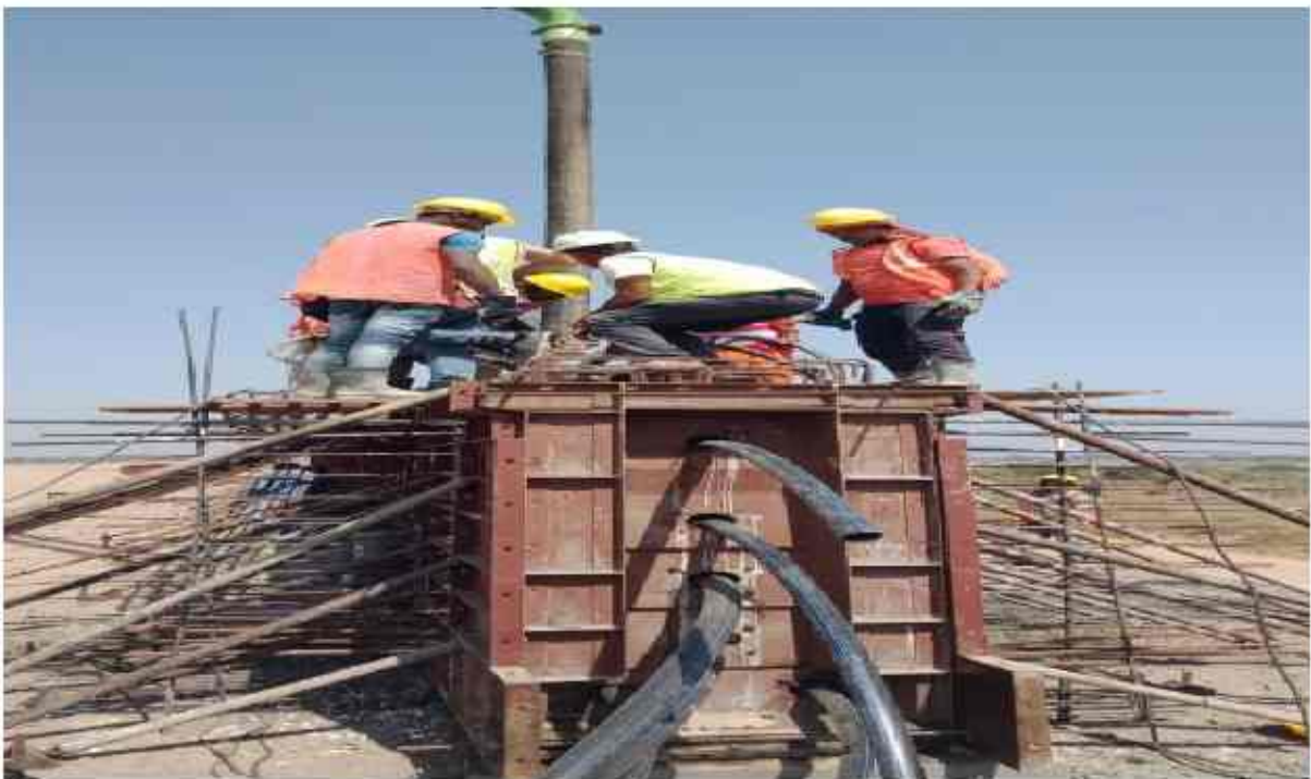
At ch 302+713 mjbpsc girder A1 P1 G-1 l.h.s concrete in progress
