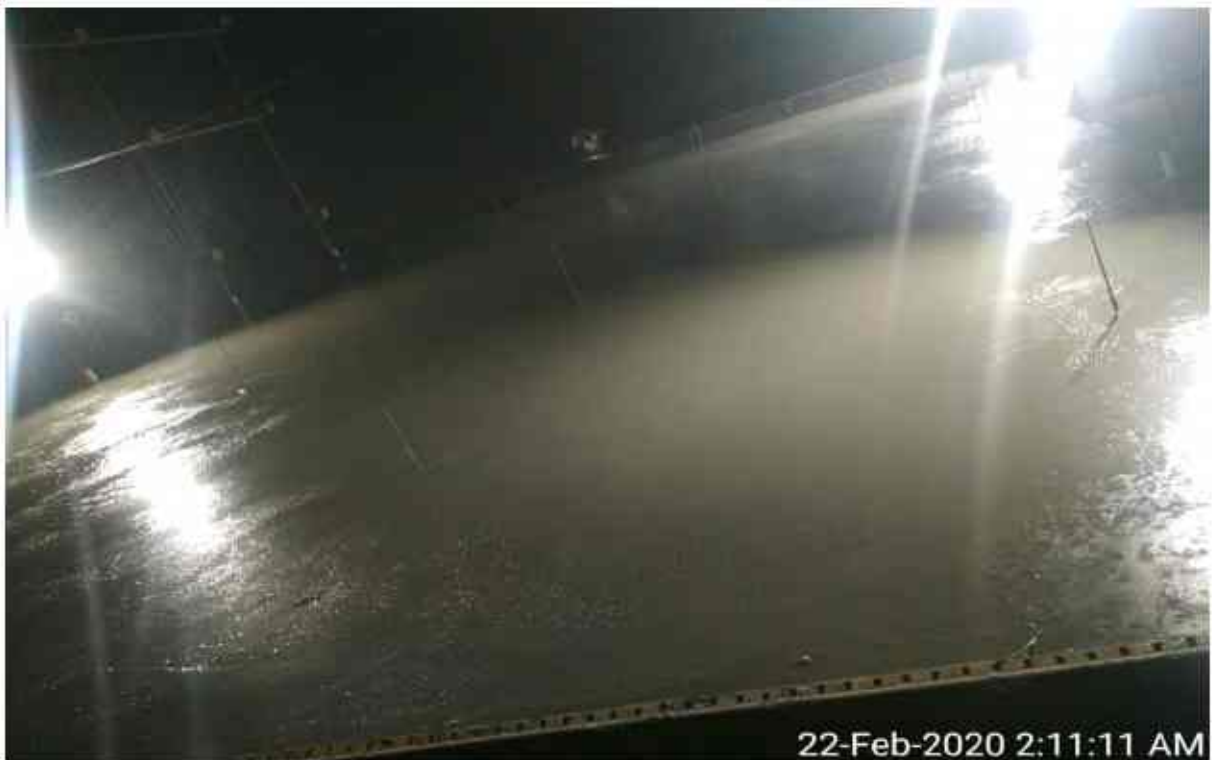
At ch-306+820 FUP service road raft lhs concrete completed
