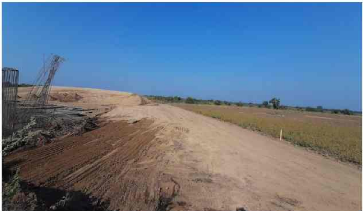
Bed for girder has been prepared up to embankment level.
