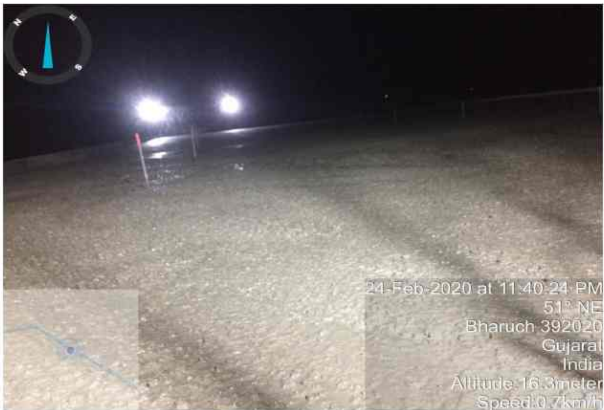
Ch-301+214 lvup LHS slab casting work completed :-
