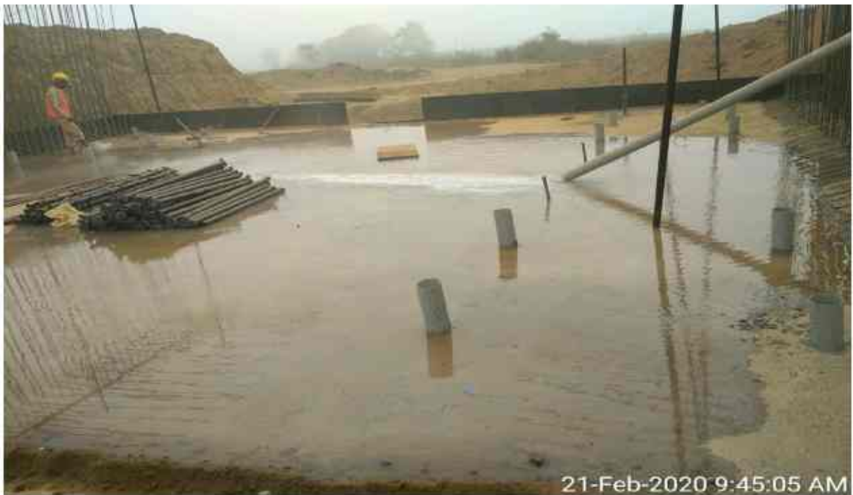
Pup raft curing in progress at ch-306+820
