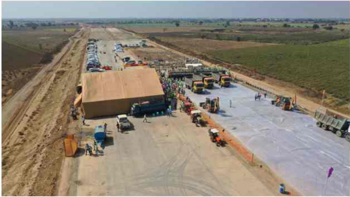
Geotextile Laying for PQC work
