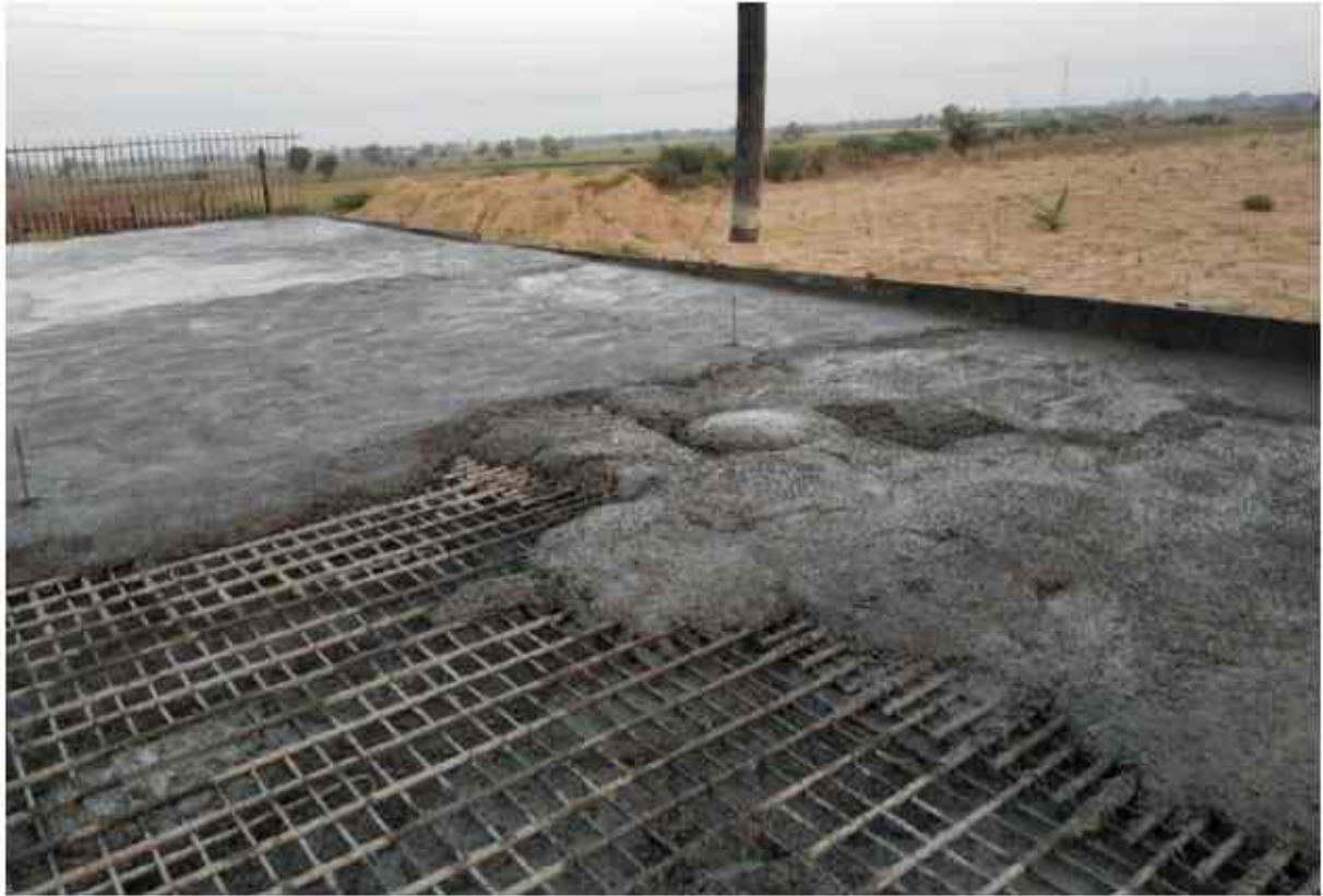
Ch 308+550 LVUP RH Stop slab progress
