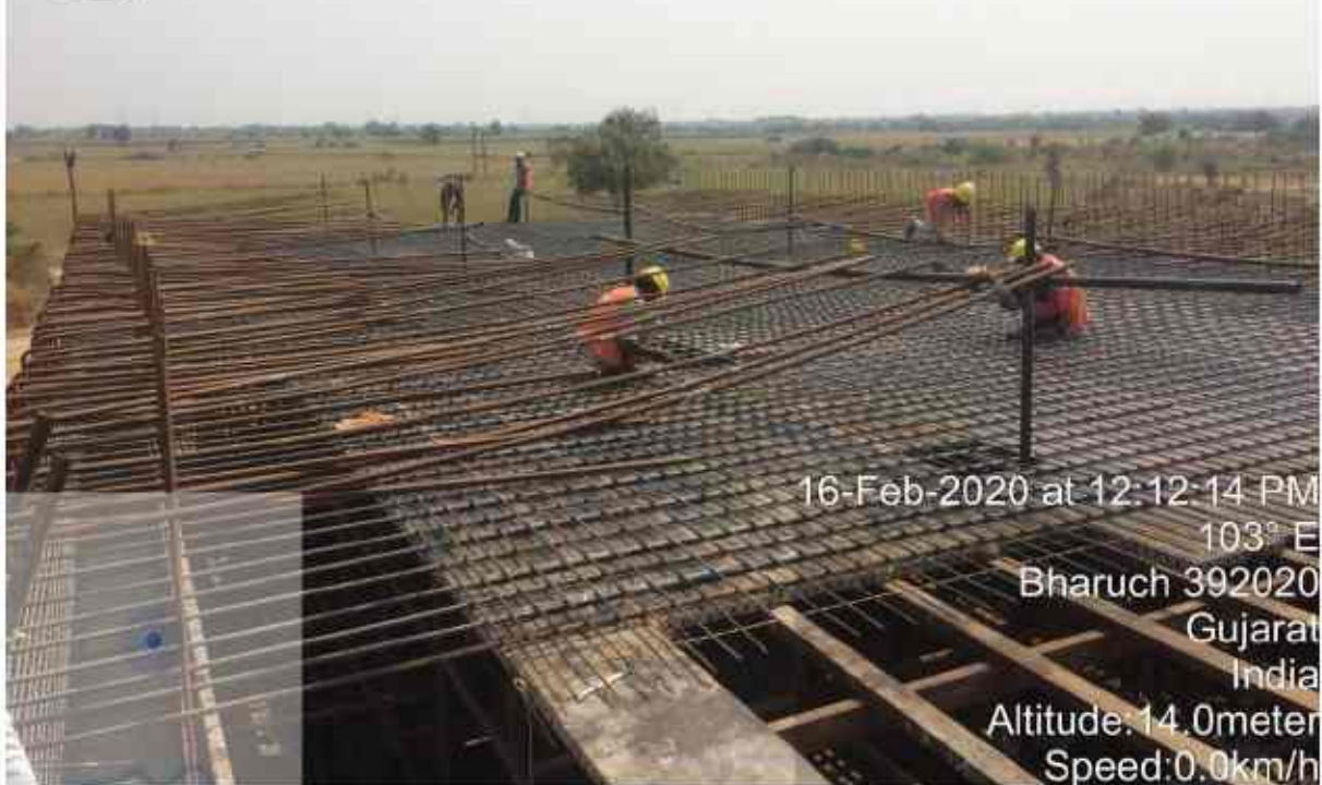
Ch-303+220 pup RHStop slab bottom Main & binder reinforcement work in progress
