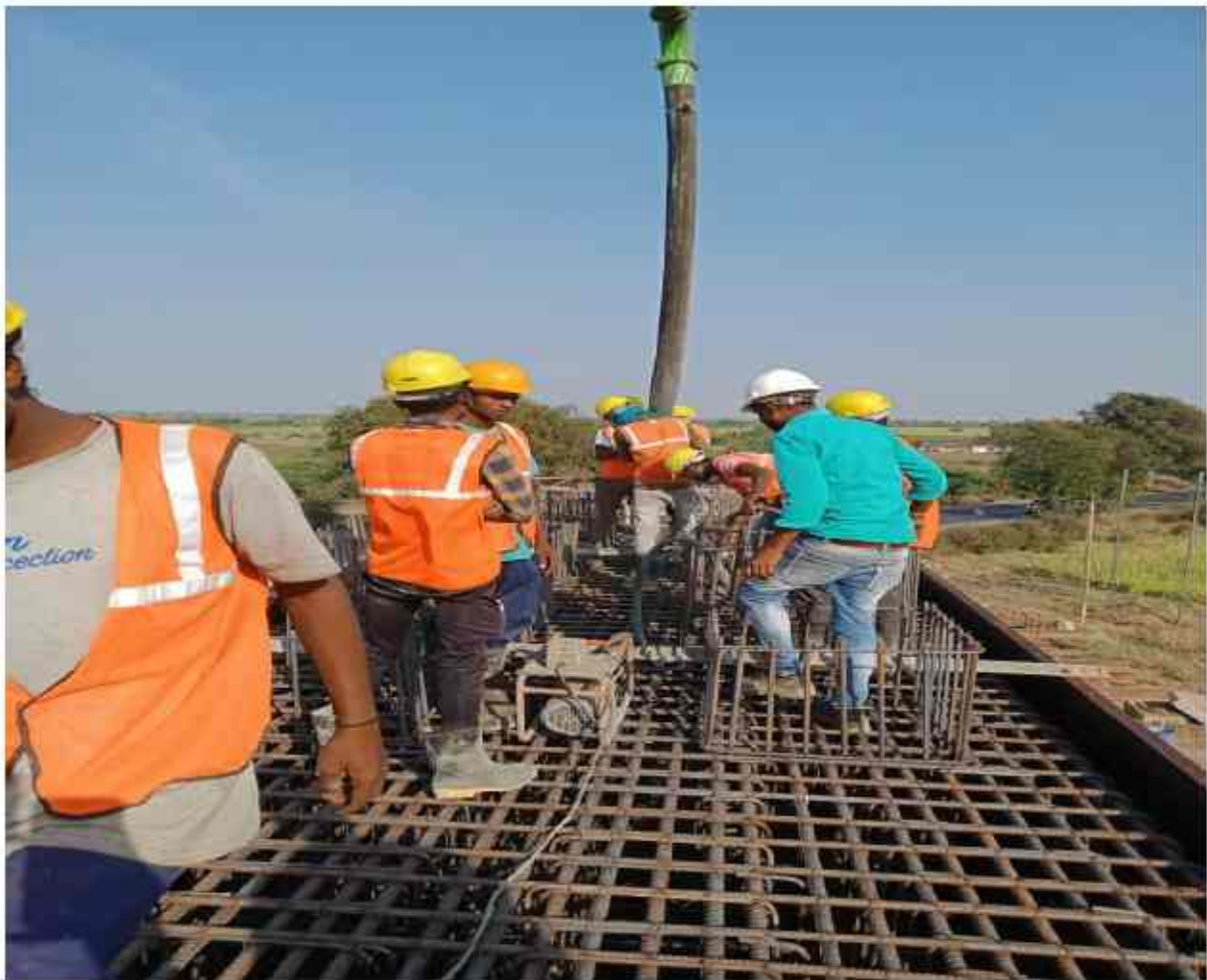
Pier cap concrete work in progress at ch 293+014
