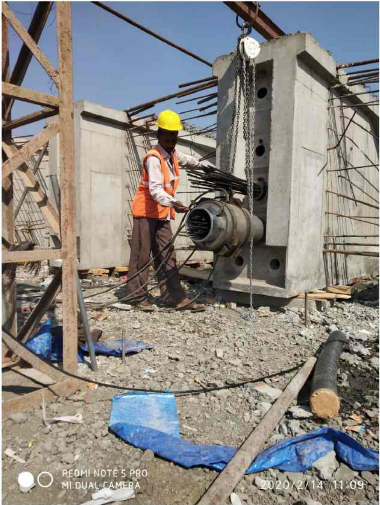
Stressing work of girder G7MJB 321+253 P1-A2 RHS progress
