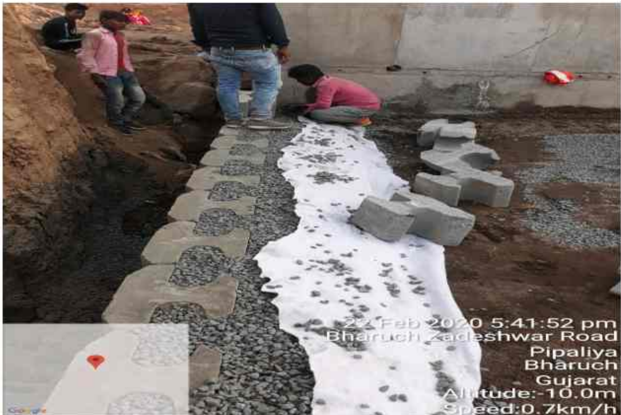
REwall Geo textile laying. 306.060
