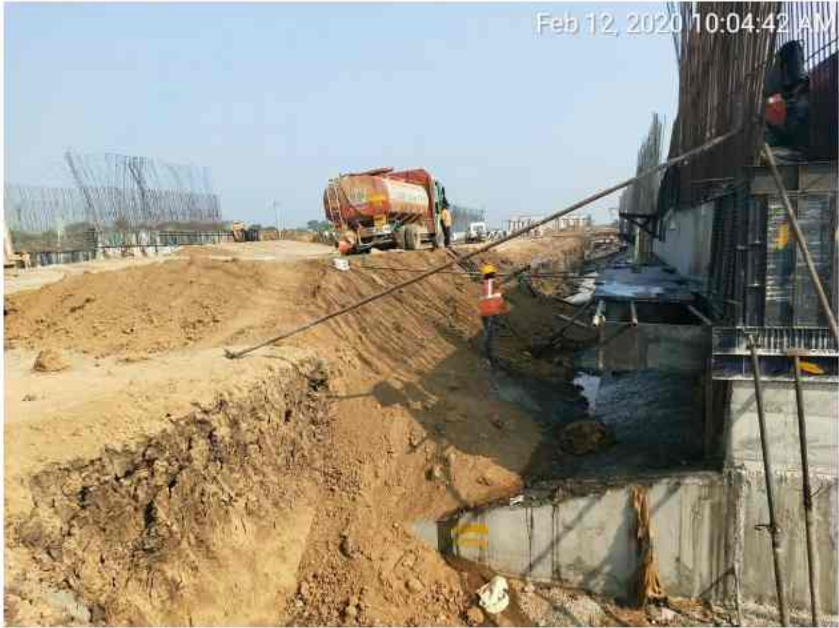
Ch-322 retaining wall curing work in progress
