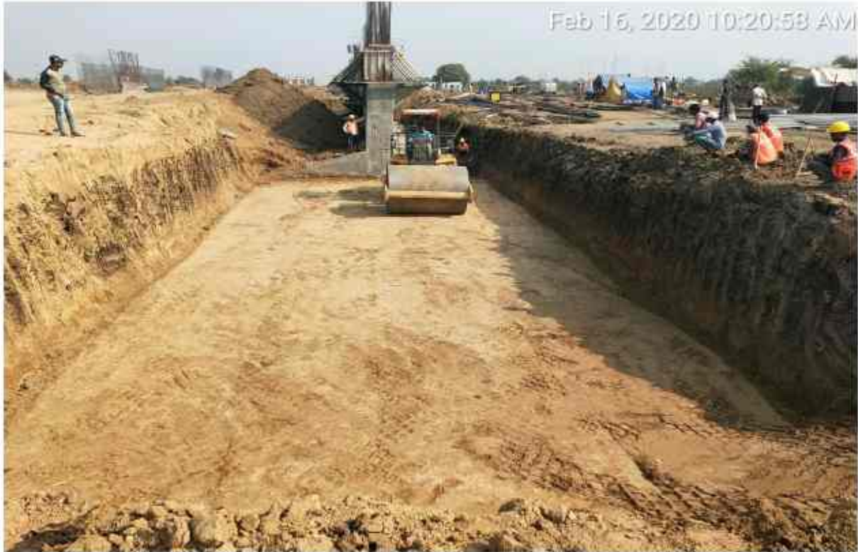
Ch-322+570 to -322+590 rhs retaining wall bed rolling work progress
