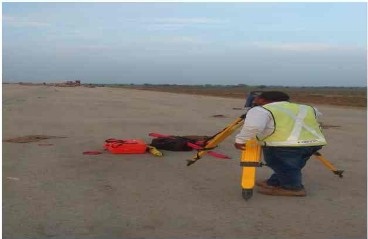
Centre line marking ch 304+750 to 304+990 rhs.
