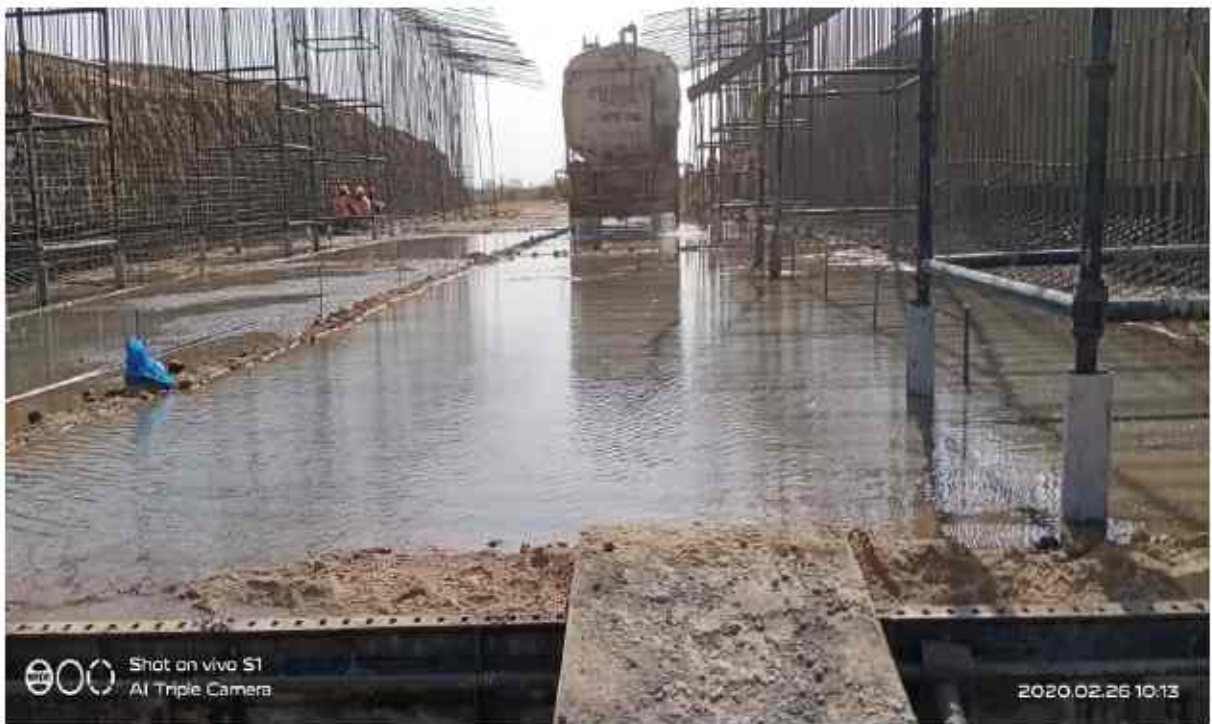
Curing on PUP raft LHSat ch-306+820
