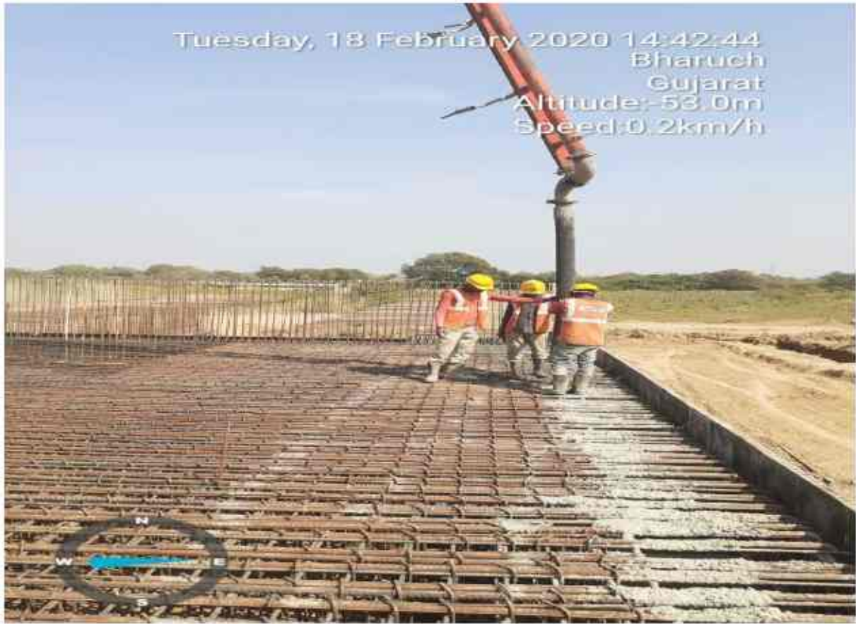
Slab concrete work in progress at ch 294+085 MNB
