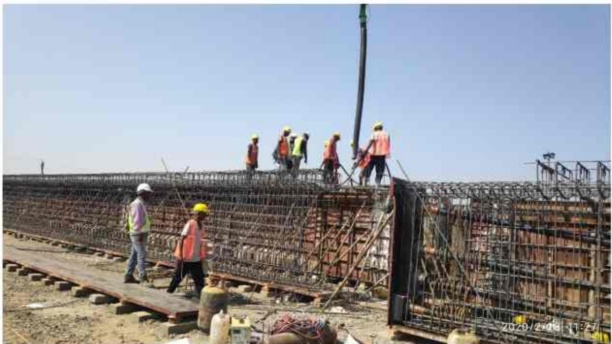
Girder casting is in progress at 321+253.mjb.lhsp1-a2.G-6
