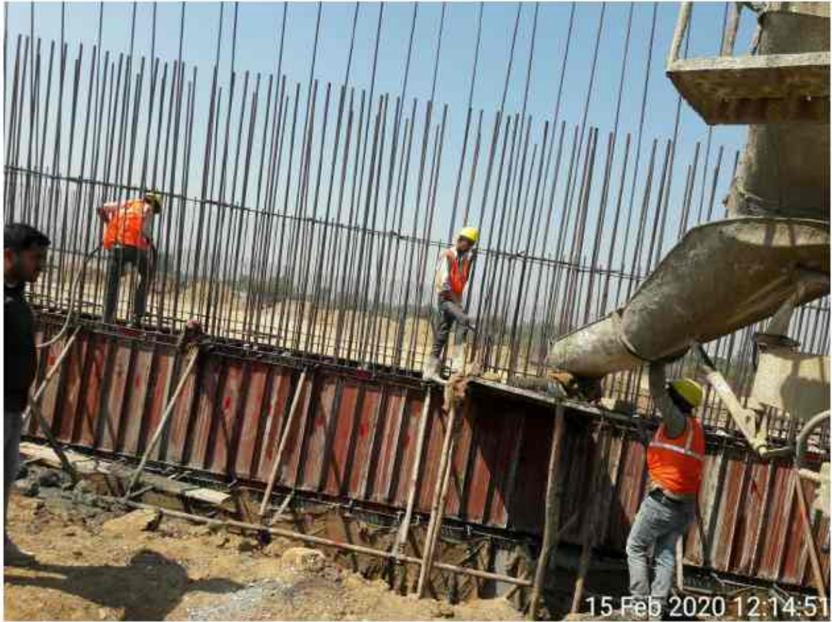
Retaining wall 2nd lift from ch 322+630 to 322+650 Concrete is in progress.
