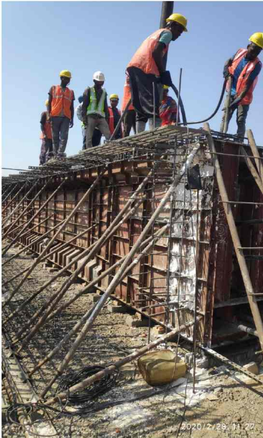
Girder casting is in progress at 321+253.mjb.lhs.p1-a2.G-6 (1)
