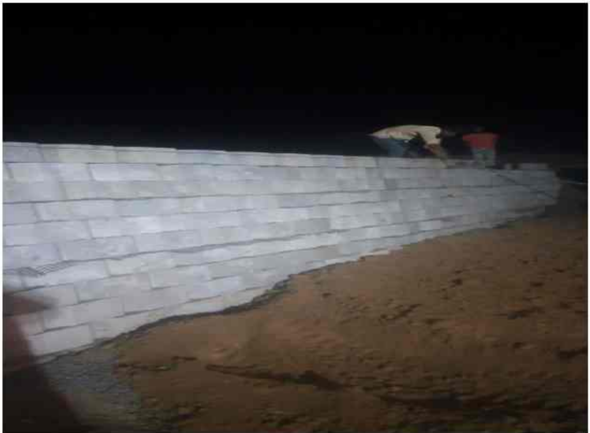
Block Erection wall-2 20th layer
