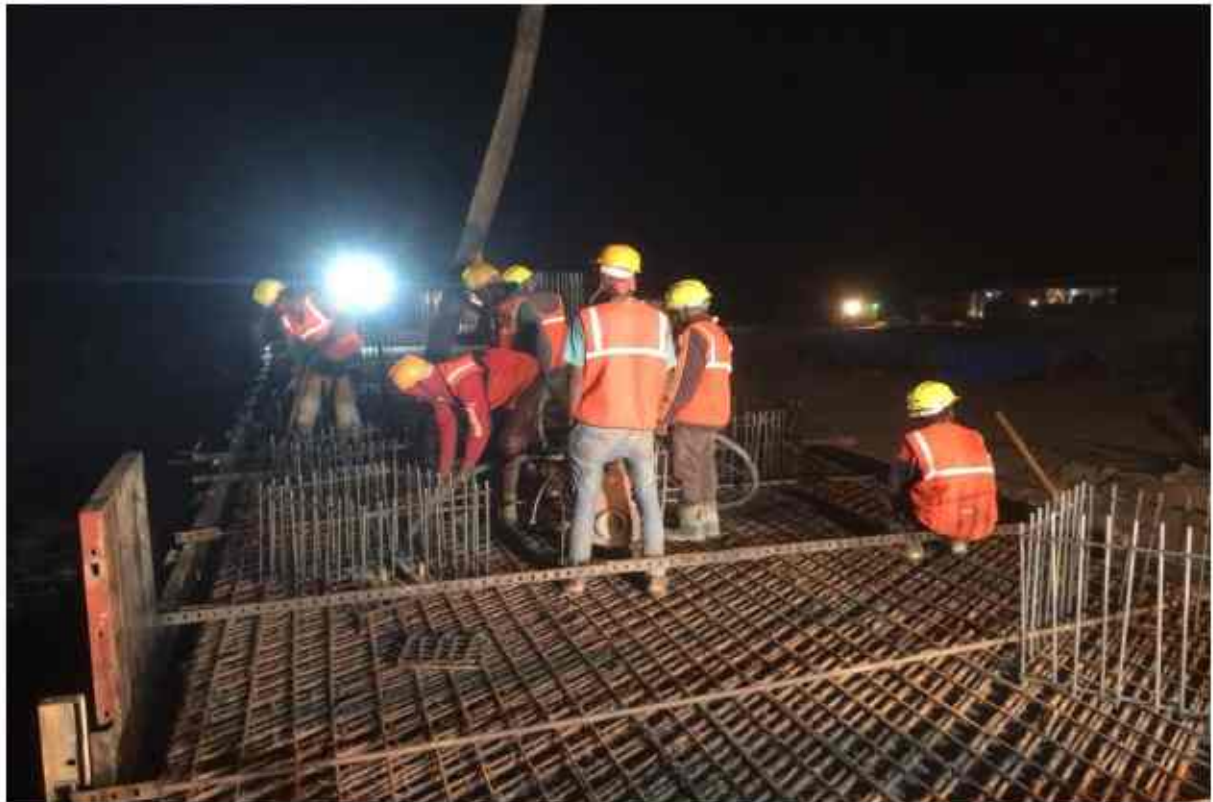
Ch-302+713 mj b LHSp1 Fler cap pouring work in progress
