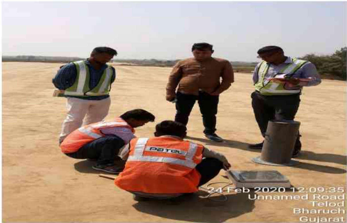
Fdd checking of emb top on ch 321+500 to 321+610 LHS
