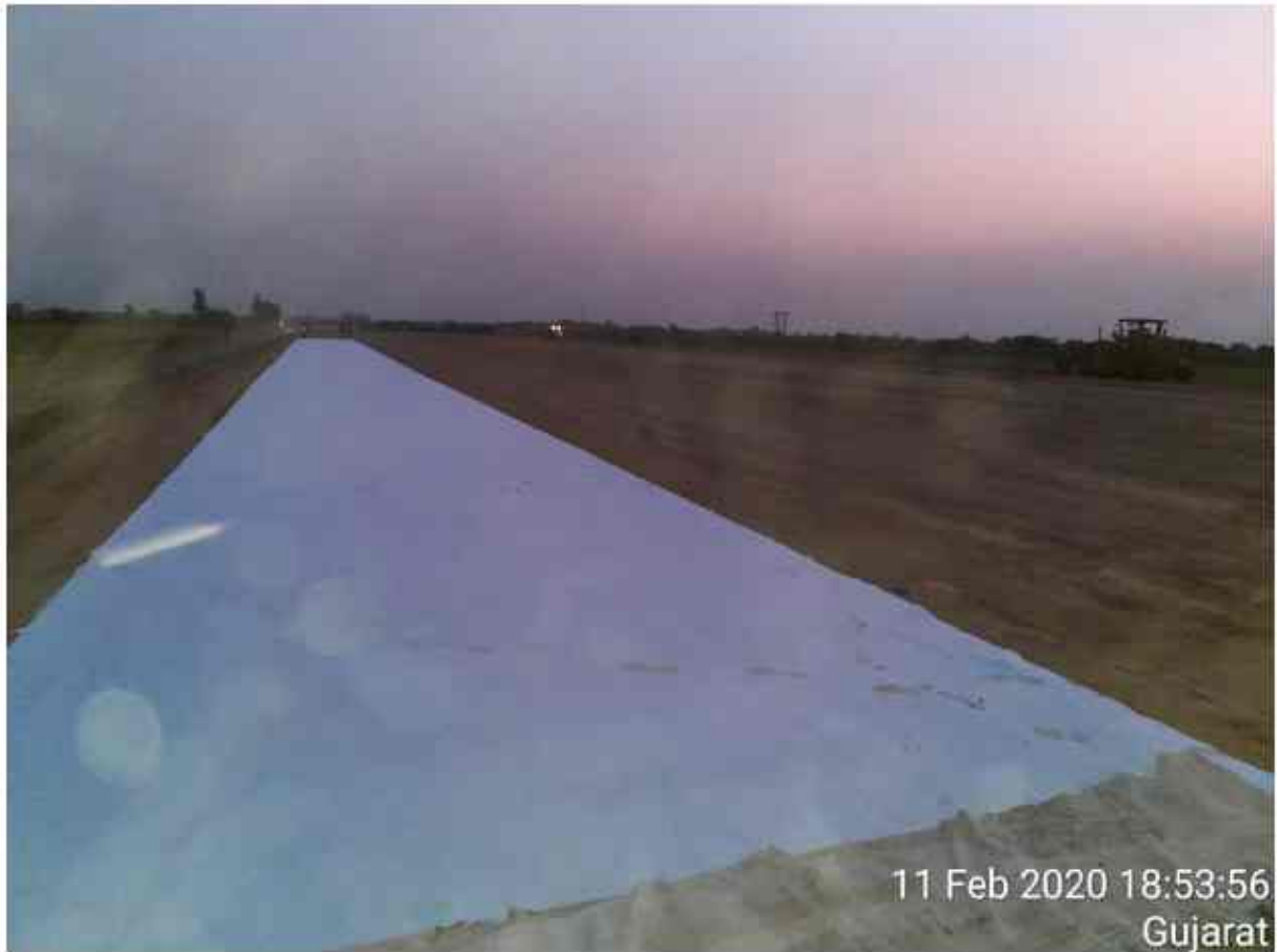
Geotextile spreading at 296+610 to 296+710 rhs.
