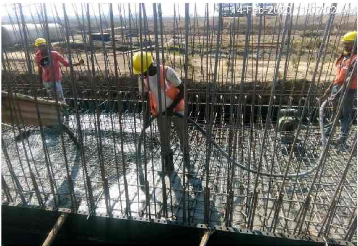
Concrete pouring progress, 307+687, RHS, boxclvrt, Raft.
