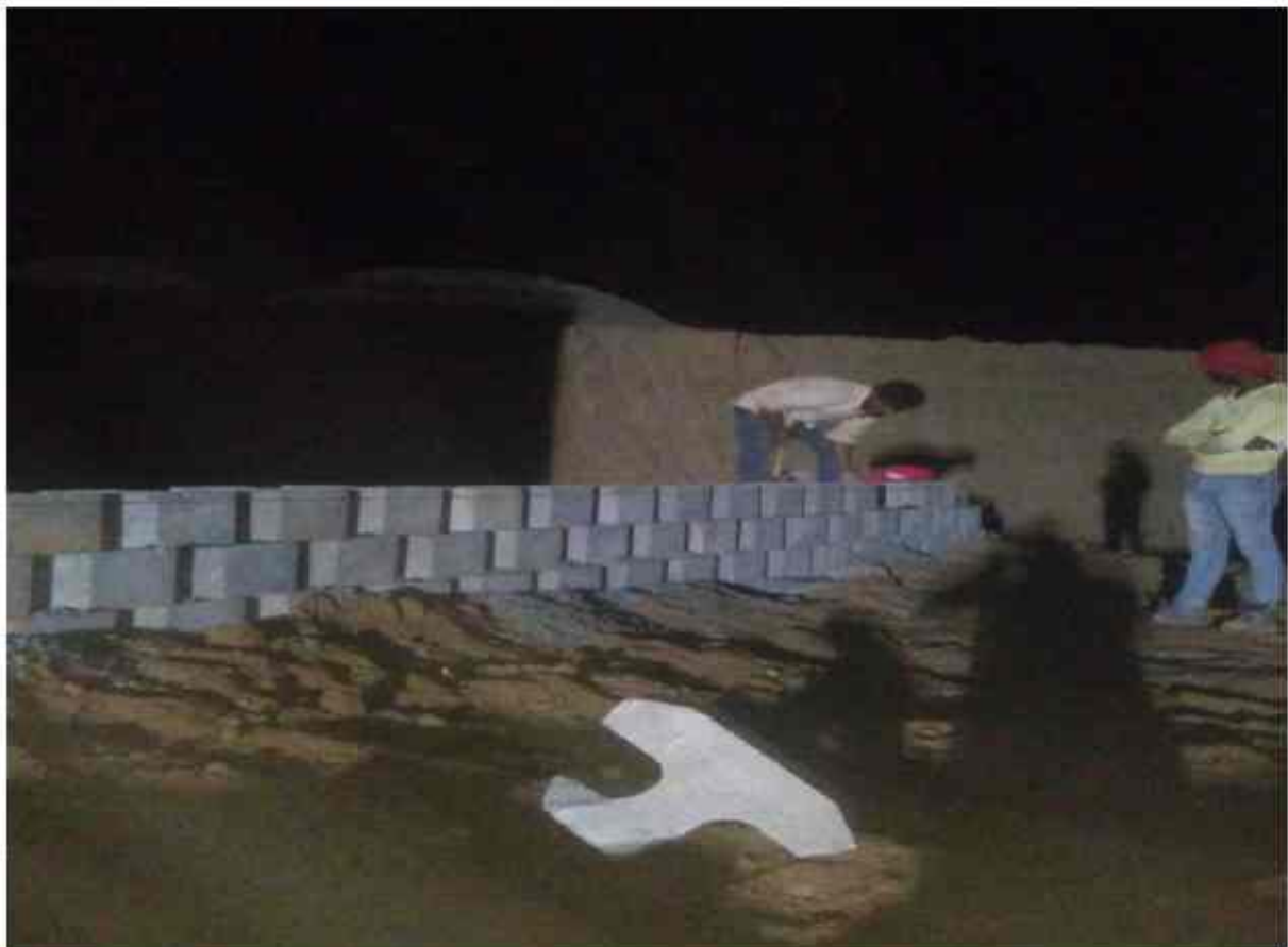
Block Erection wall 3
