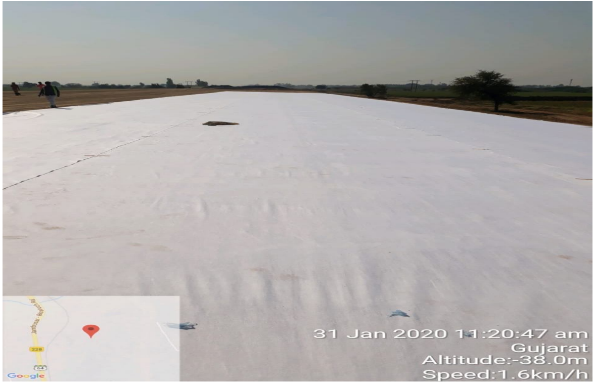
DT.31.01.2020 Geo textiles laying. ch.296.700 to 296.800 Lhs.
