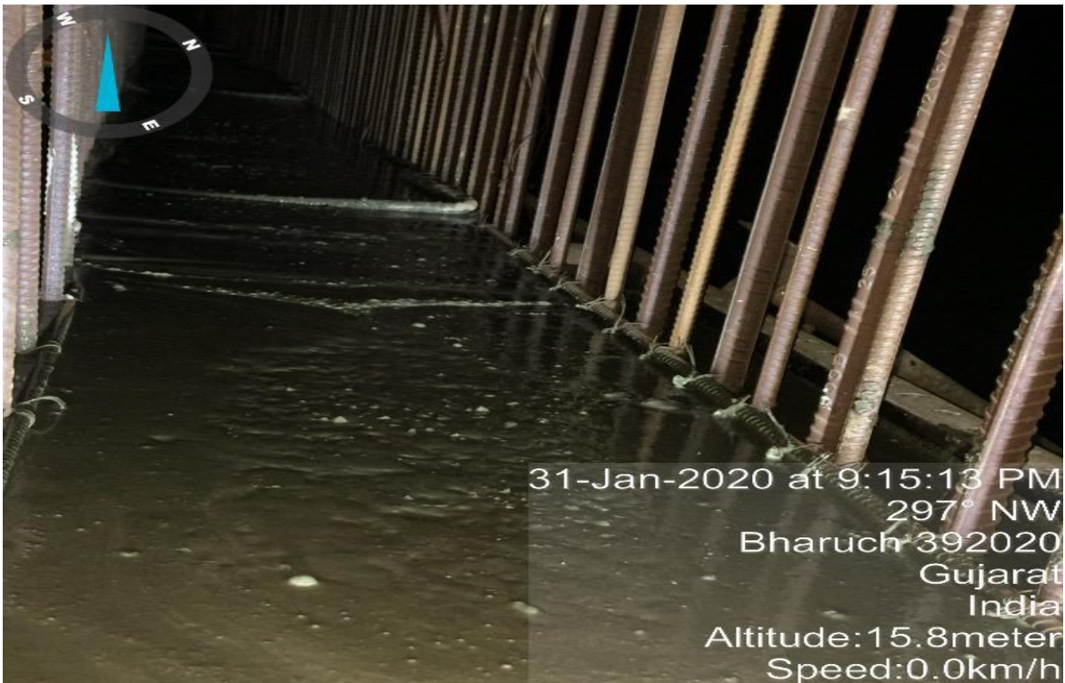
Dt. 31.01.2020 CH-301+790 PUP LHS A1 & A2 1 st lift concreting completed
