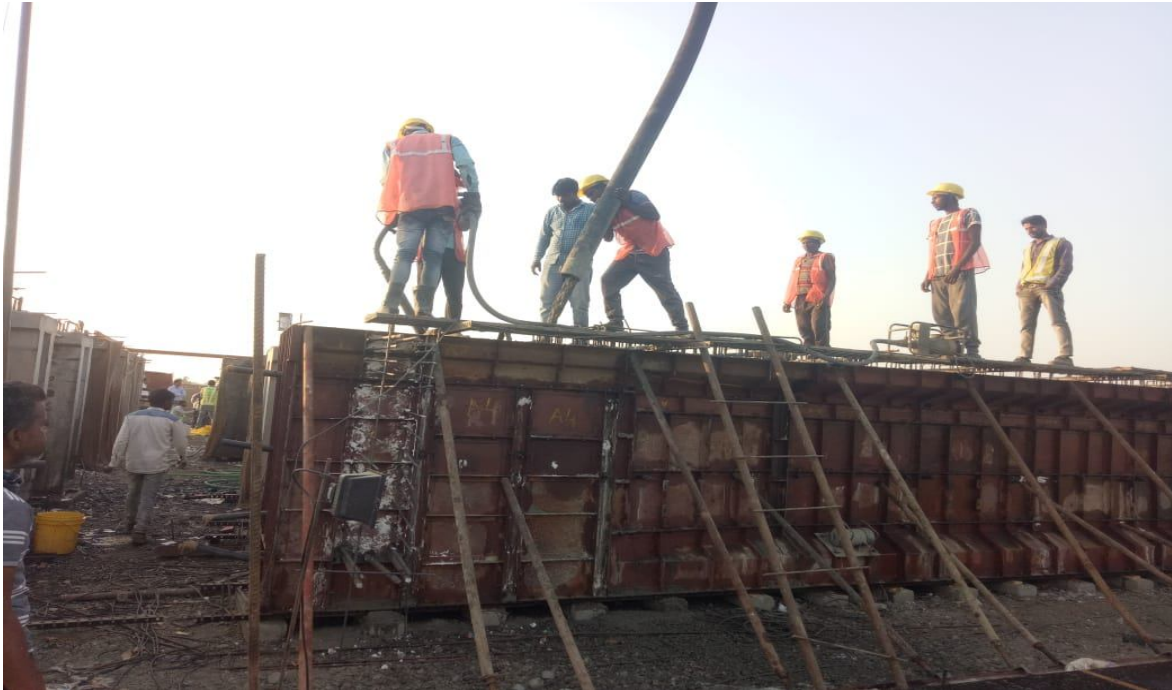
Dt. 31.01.2020 Ch 318+870 MJB PSC girder P1-P2 G7 RHS Concreting in progress
