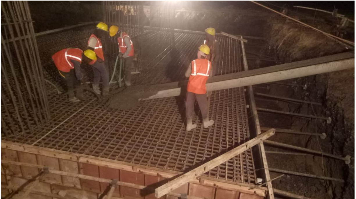
DT.31.01.2020 293+014 ROB Pile cap concrete tart RP13
