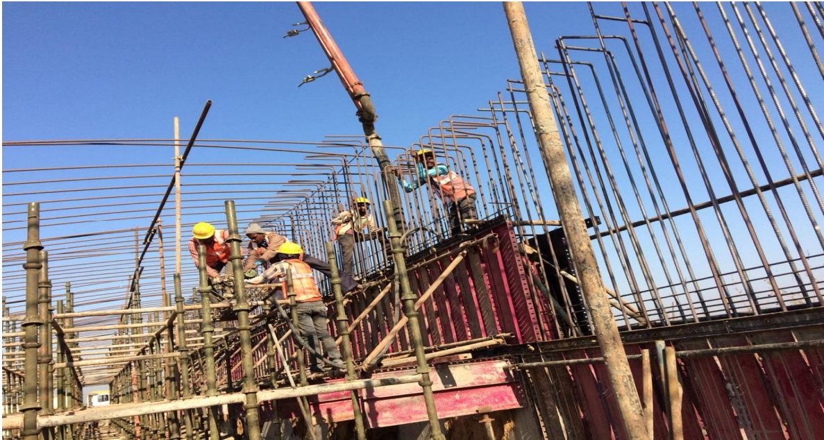
Dt. 30.01.2020 CH 301+214 LVUP A1 & A2 LHS 2 nd Lift Concreting in progress
