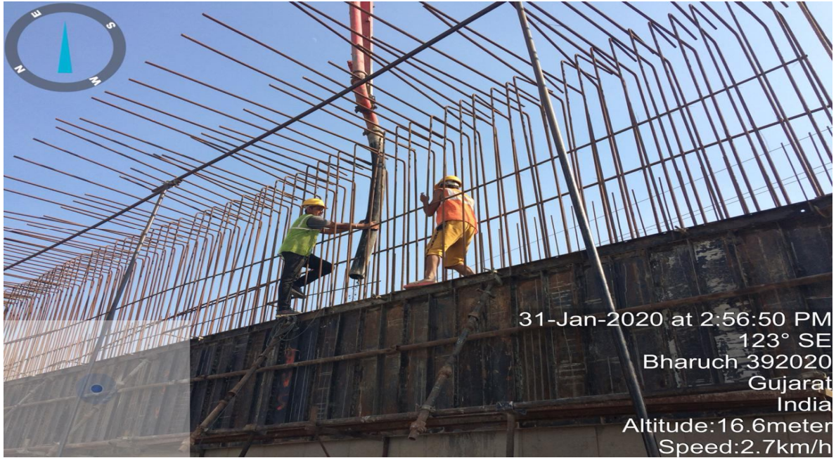
DT.31.01.2020 Ch-303+808 VUP LHS A1 3rd lift wall pouring work start
