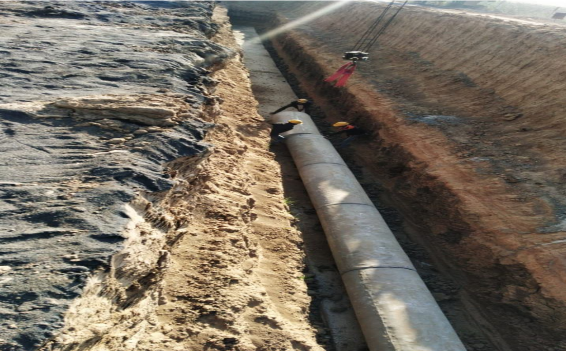
DT.29.01.2020 Ch 303+850 utility pipe laying
