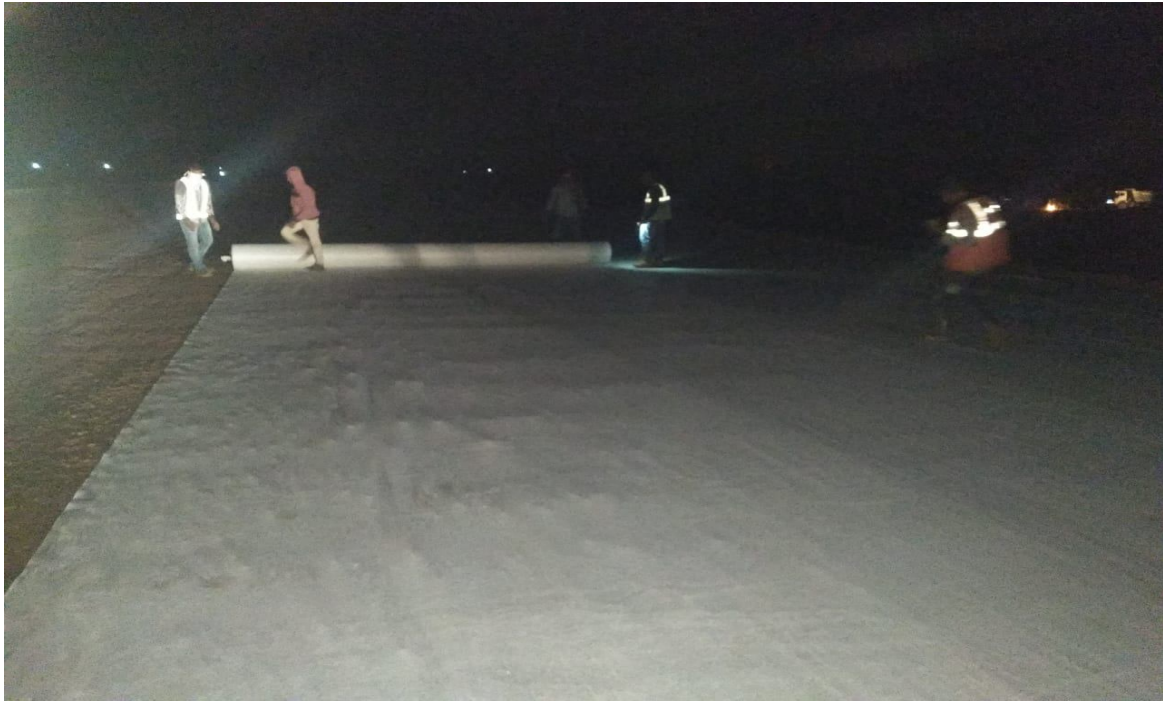
DT.29.01.2020 Geo textile laying on ch 321+780 to 321+960 RHS (2)
