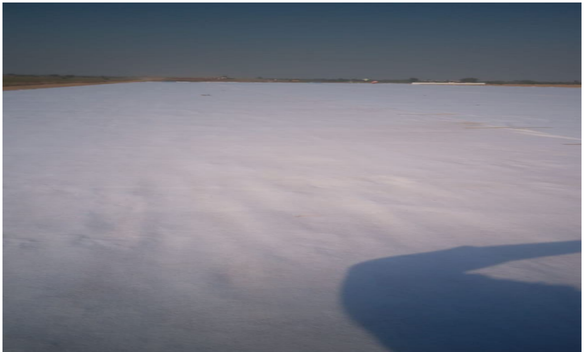
DT.31.01.2020 Geo textile laying 305+100 to 305+200 Lhs
