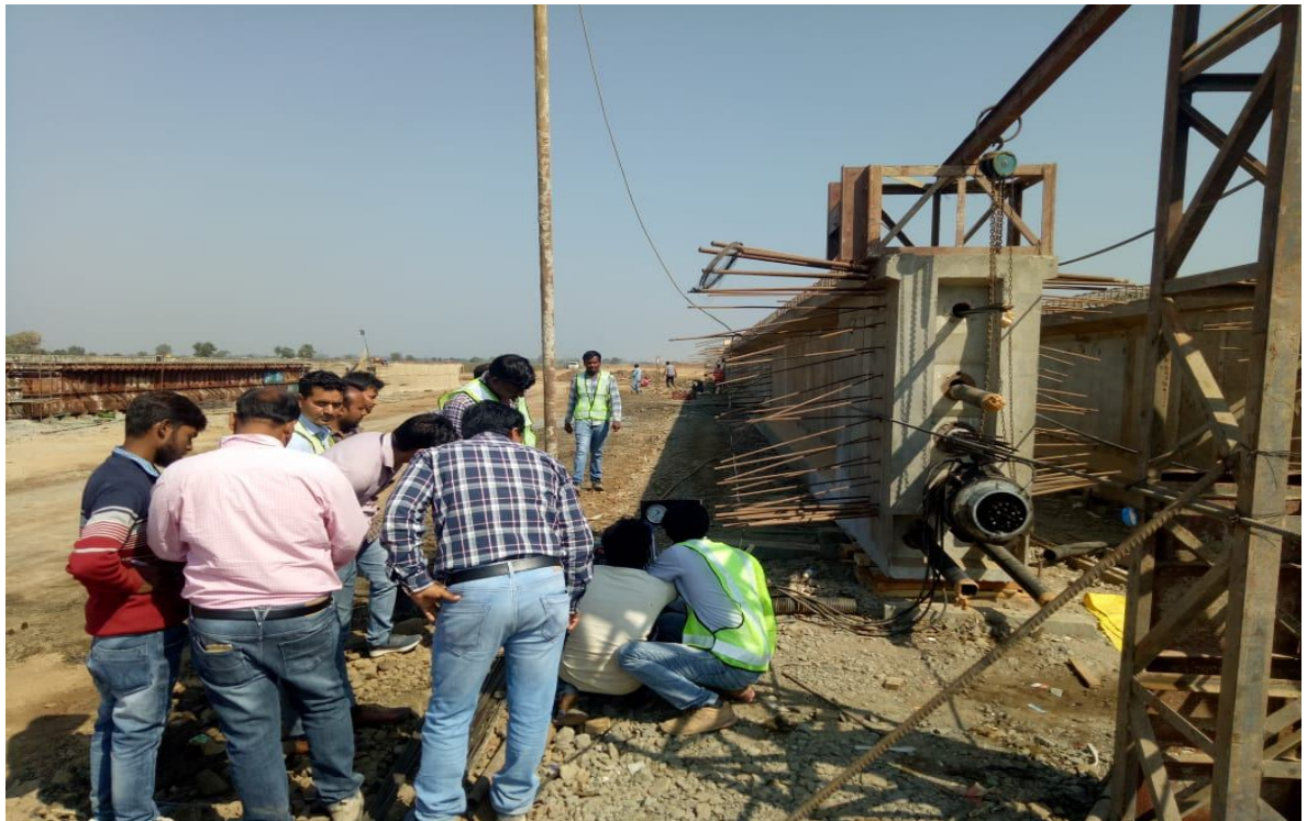
DT.31.01.2020 Ch. 321+253 psc girder a2-p1 G-1 rhs prestressing work in progress
