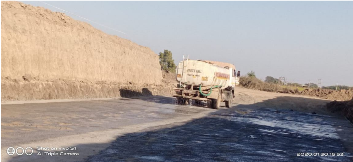
DT.30.01.2020 Curing on pcc of LVUP at ch.306+820
