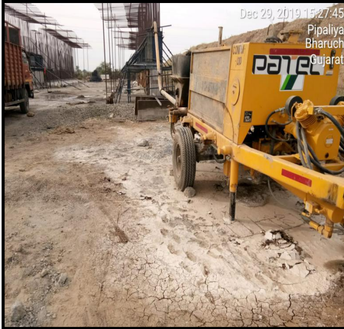
AT CHAINAGE NO 308+550 LVUP RHS A2 WALL 2ND LIFT IS READY FOR CONCRETING
