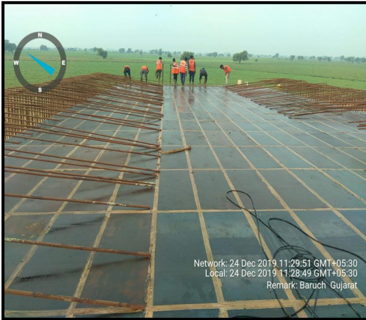
PUP RHS SLAB CURRING WORK IN PROGRESS CH 305+850
