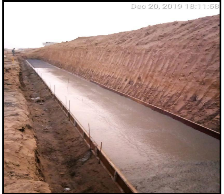
AT CH NO 306+122 TO 306+144 TOE WALL PCC COMPLETED.
