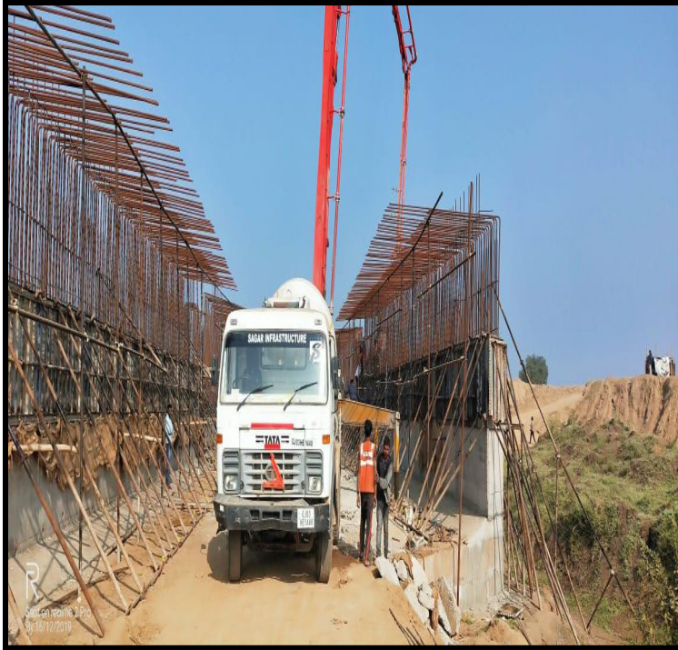
CH-321+673 RHS LVUP WALL 2ND LIFT CASTING WORK
