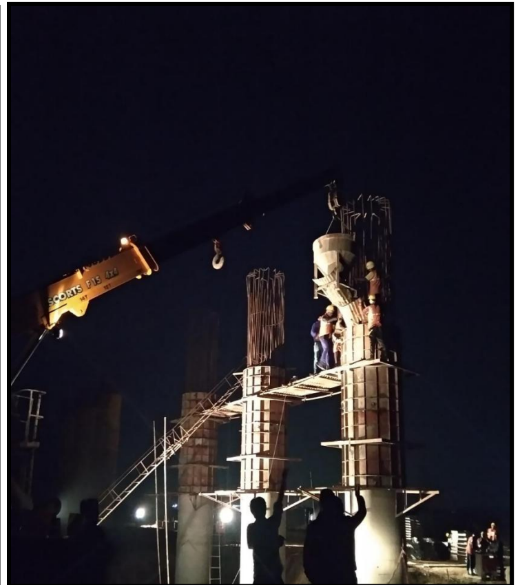
CH 293+014 ROB RP3 PIER SHAFT 3RD LIFT CONCRETE POURING
