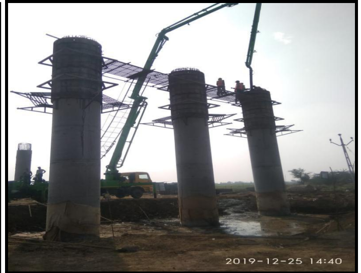
CH 293+014 ROB LP4 PIER SHAFT FINAL CONCRETE COMPLETE.
