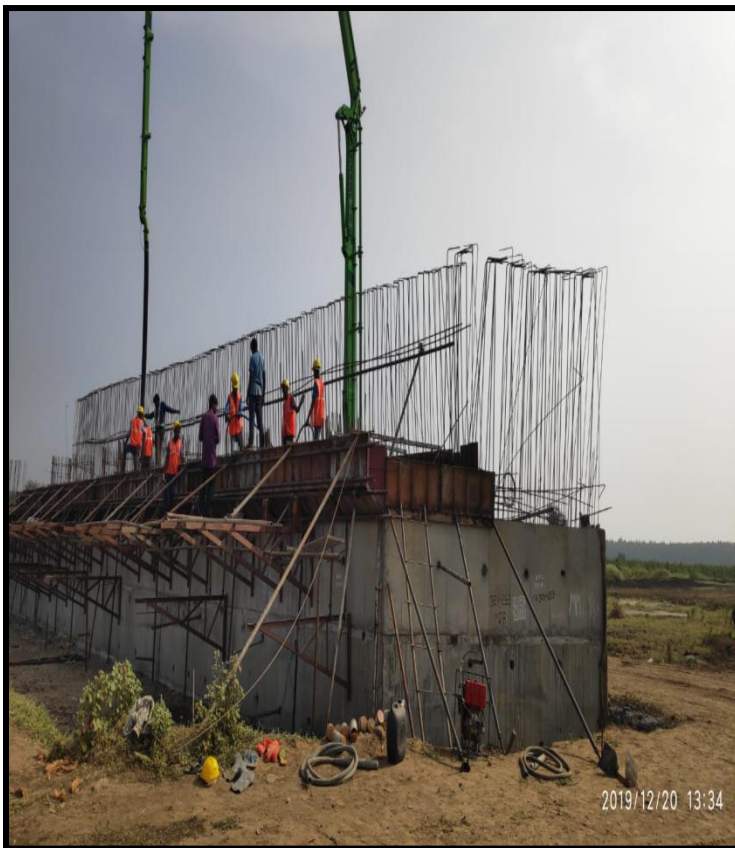
CH NO 321+253.MJB.LHS.A1. ABUTMENT CAP CONCRETING
