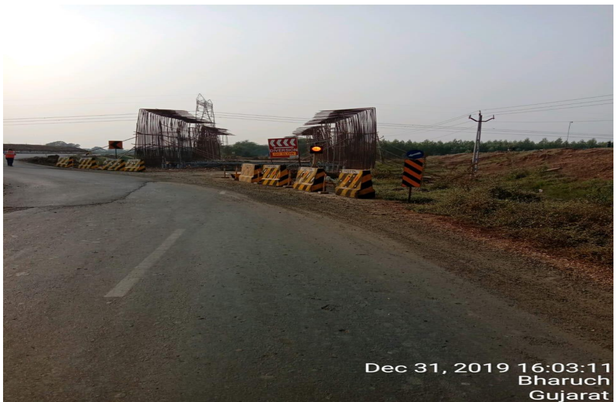
Solar blinker install at Diversion for VUP at ch-312
