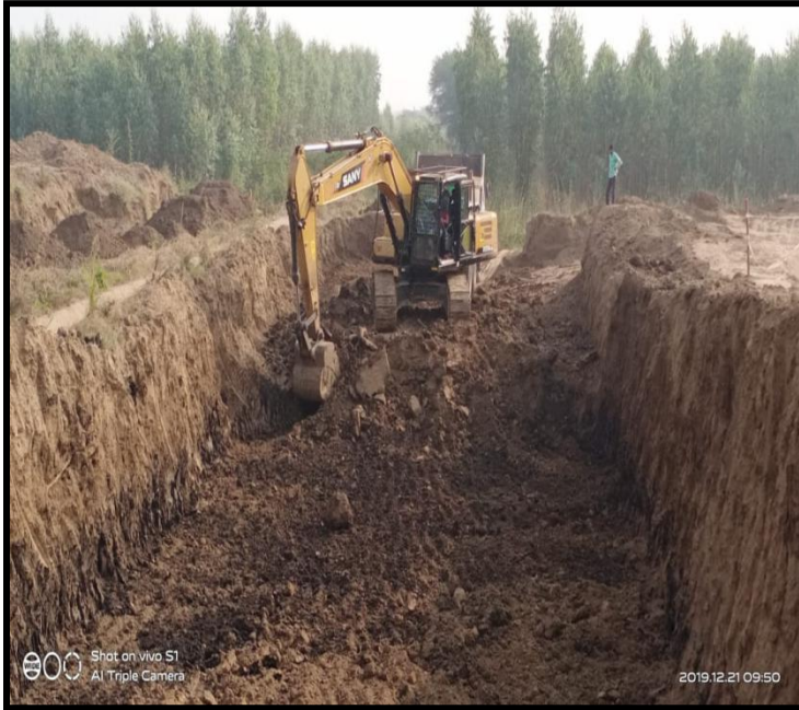
CH 313+055 PUP EXAVATION IN PROGRESS
