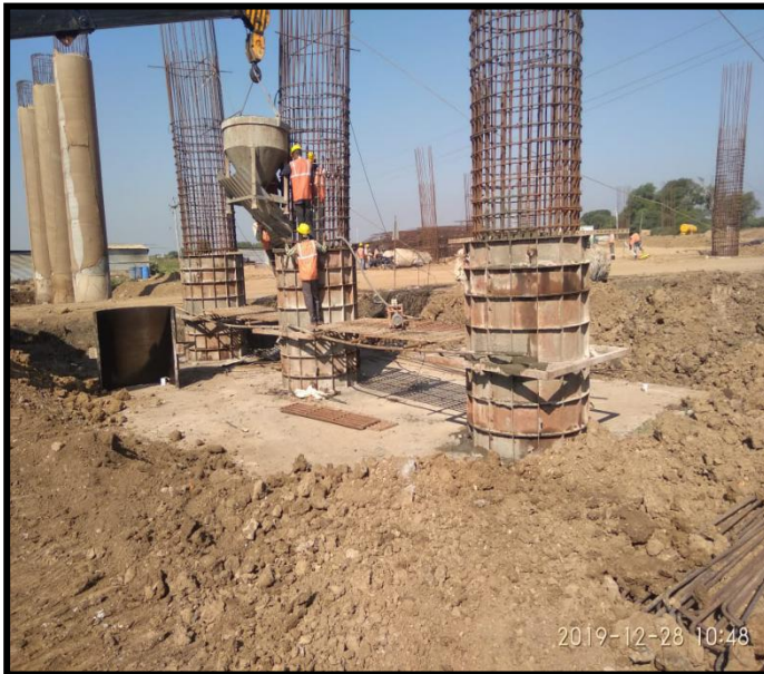
CH 293+014 ROB RP4 PIER SHAFT 2ND LIFT CONCRETE POURING WORK
