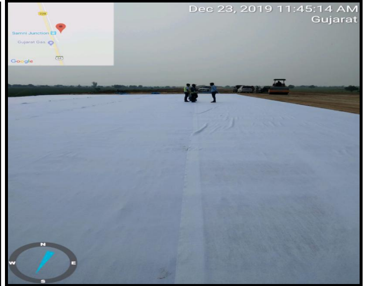
CH - 304+700 TO 304+900 RHS GEO TEXTILE LAYING AFTER SUBGRADE TOP
