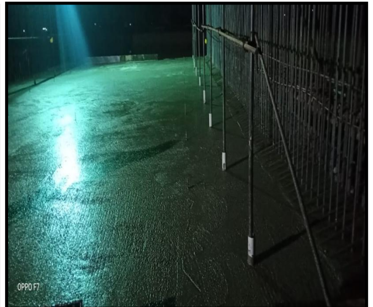
RAFT CONCRETE DONE AT CH 299+079 RHS
