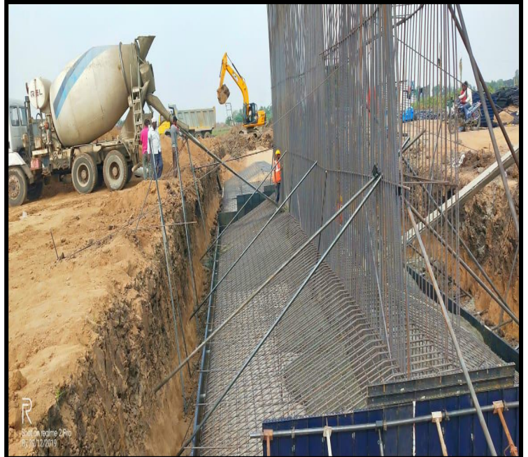
CH-322+570 TO322+590 RHS RETAINING WALL FOOTING CASTING
