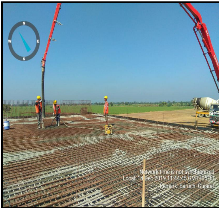
PUP SLAB CONCRETE WORK IN PROGRESS CH 305+850 RHS
