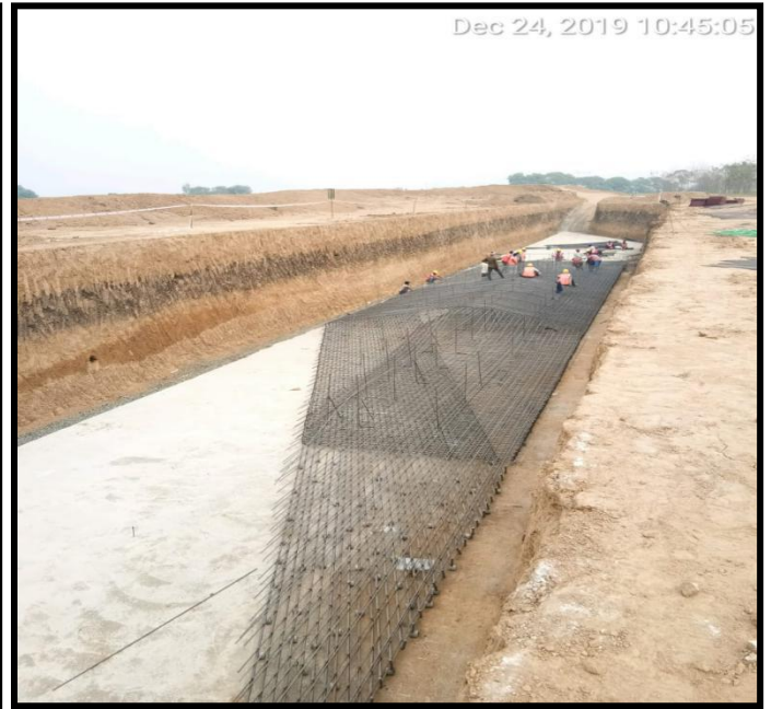
AT CH 310+725 MNB A2 RHS REINFORCEMENT BINDING FOR RAFT
