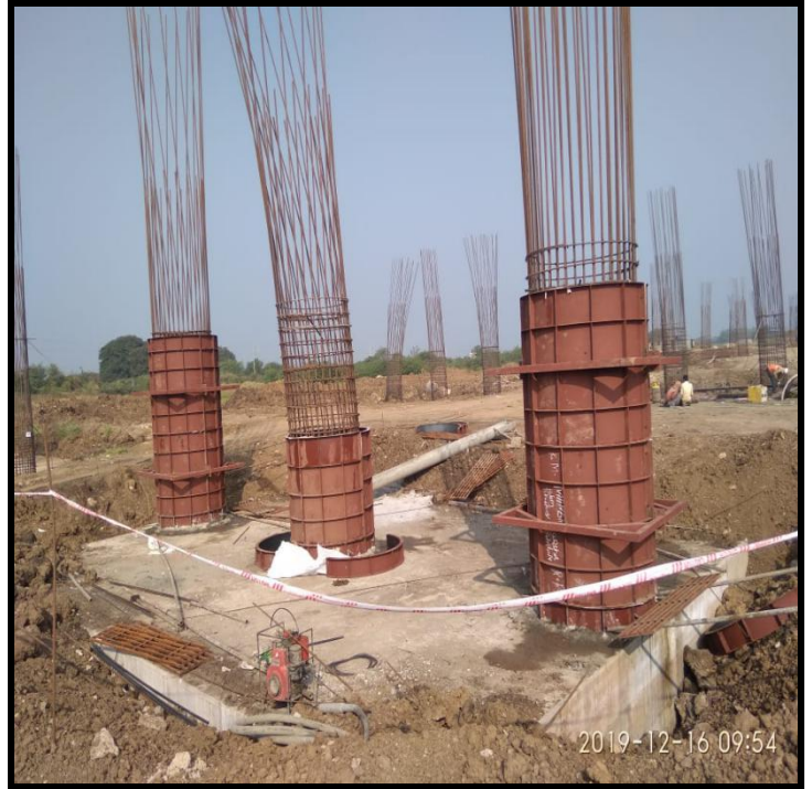
CH 293+014 ROB RP11 PIER SHAFT 2ND LIFT SHUTTERING WORK
