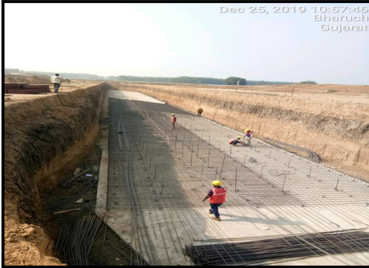
AT CHAINAGE NO 310+725 MNB A2 RHS REINFORCEMENT BINDING FOR RAFT
