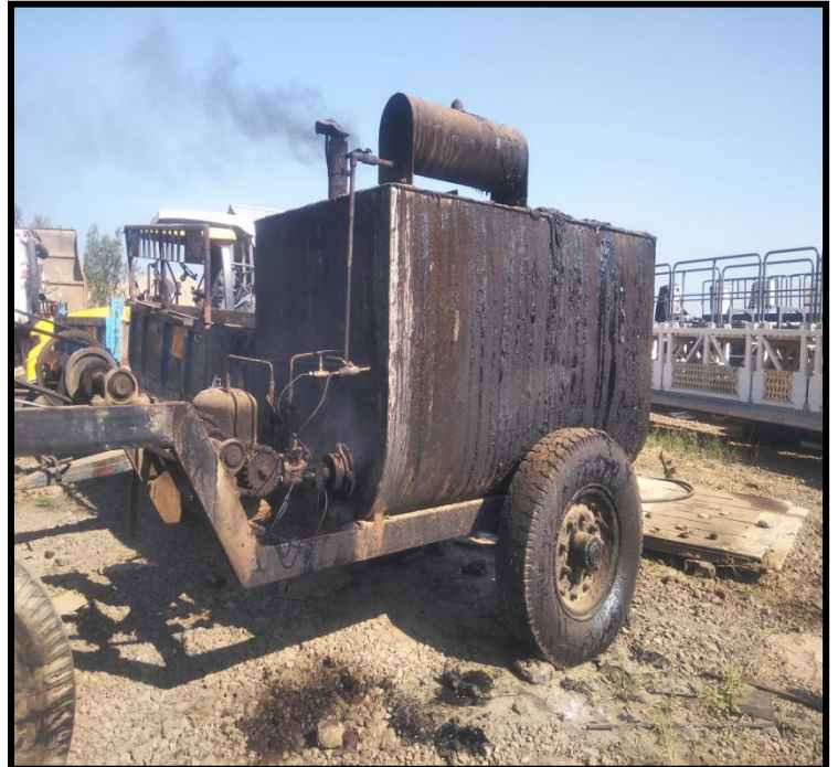
BITUMEN BAUSER EMULSION HEATING AND TESTING GOING ON
