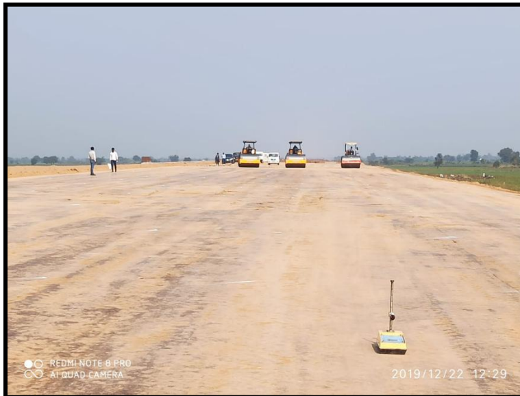
SUBGRADE TOP LEVEL & FDD CHECKING CH - 304+700 TO 304+900 RHS WALL HUNCH CONCRETE WORK IS START PUP CH 306+060 RHS
