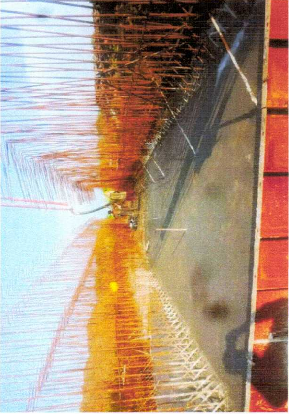
324+236 RAFT CONCRETE POURING WORK IN PROGRESS
