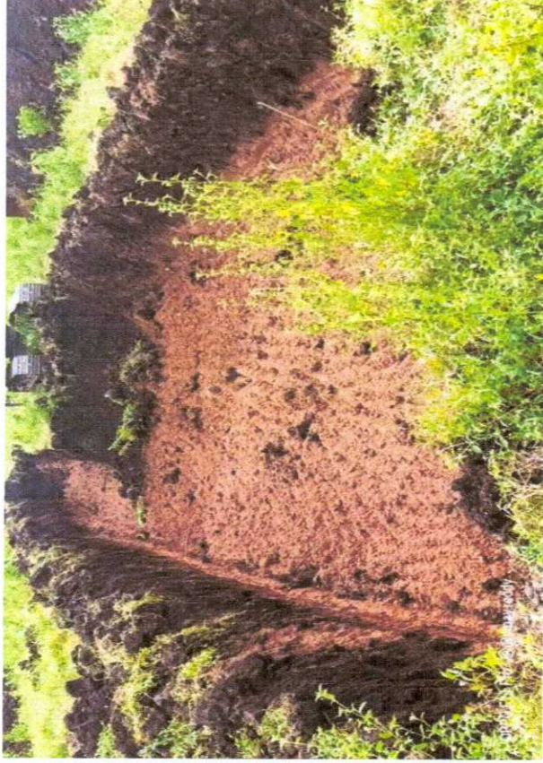
331+950 LHS TOE WALL EXCAVATION WORK IN PROGRESS
