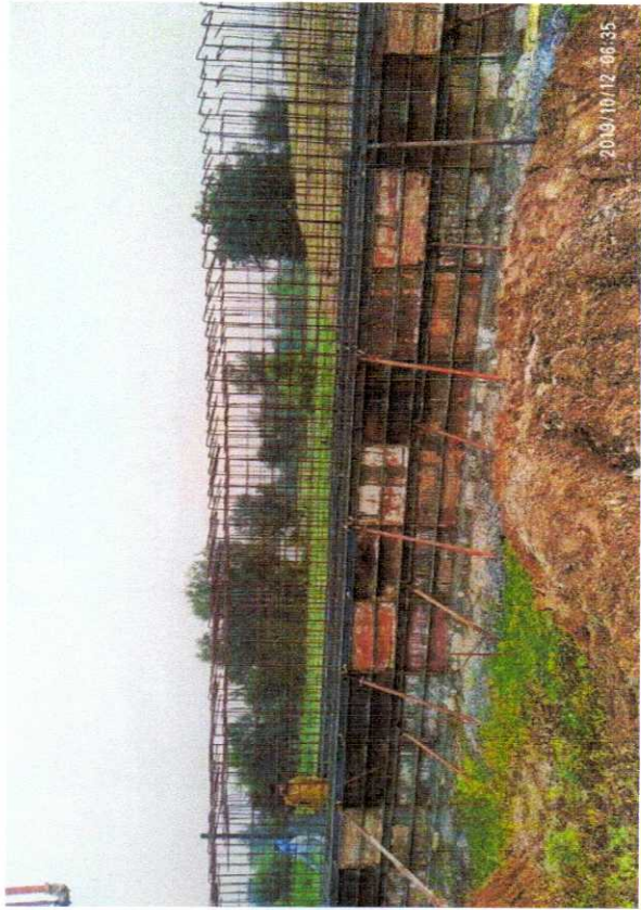
335+074 BC BOTTOM HAUNCH CONCRETING STARTED (RHS)
