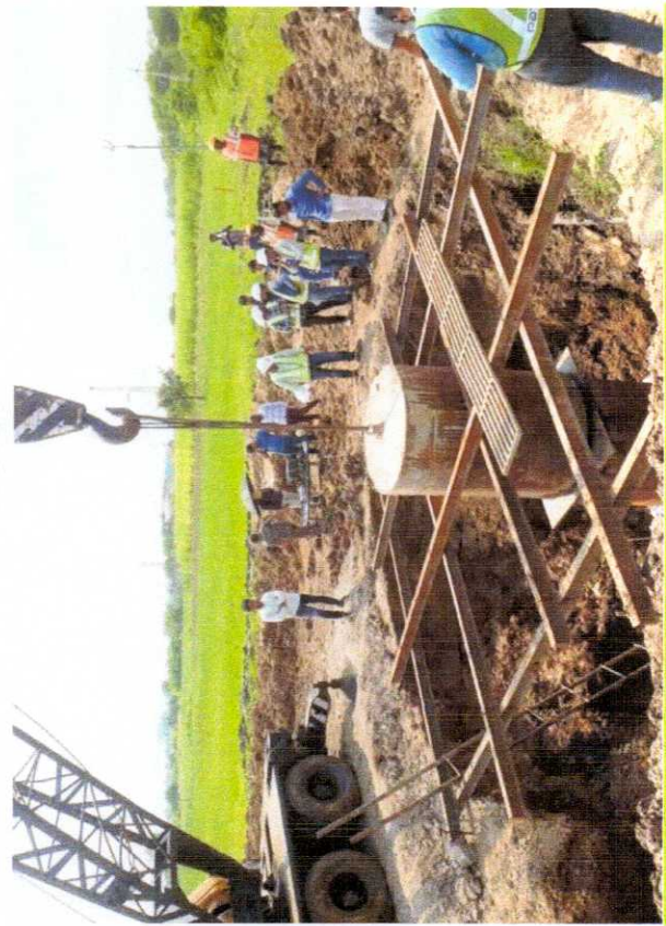
323+074 PILE CAP AND PIER LHS CONCRETING WORK
