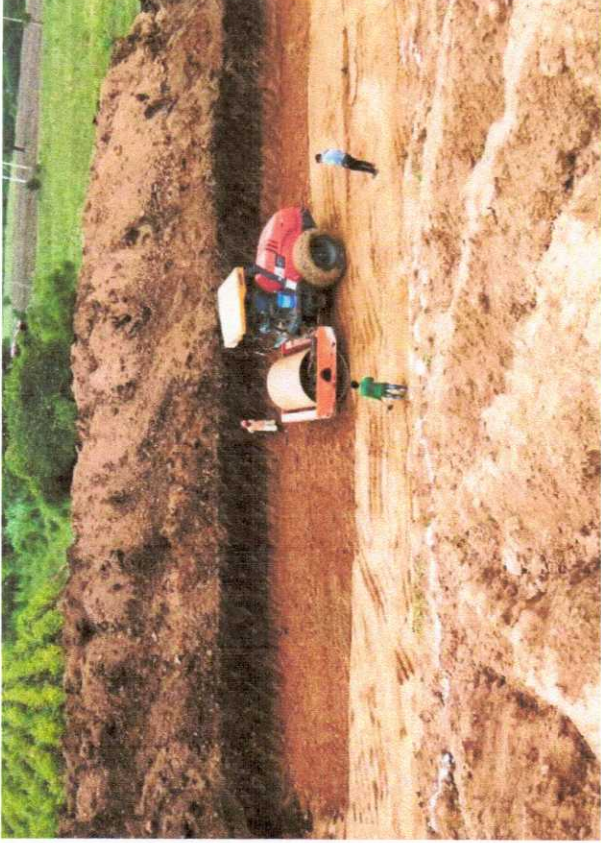
323+270 RHS RAW BED COMPACTION WORK IN PROGRESS
