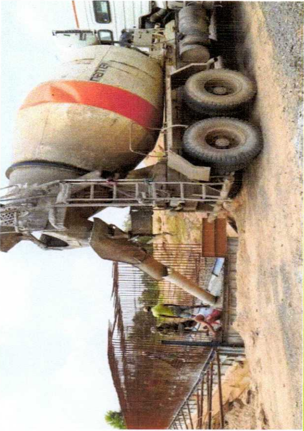
335+074 BC BOTTOM HAUNCH CONCRETING STARTED (RHS)
