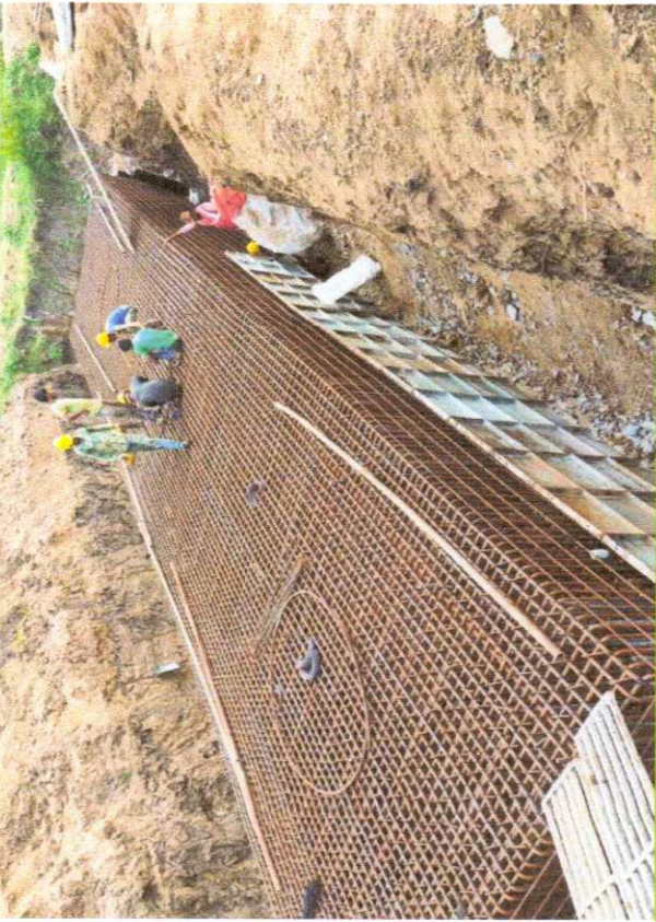
323+074 RAFT LINK BAR & SHUTTERING WORK IN PROGRESS
