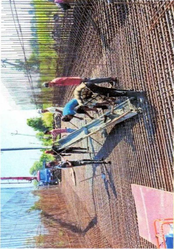
330+402 VUP RHS RAFT CONCRETE POURING IN PROGRESS
