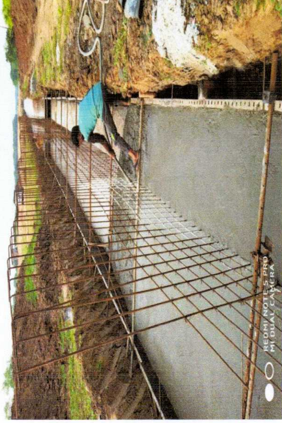
354+860 TOE WALL RAFT POURING IN PROGRESS
