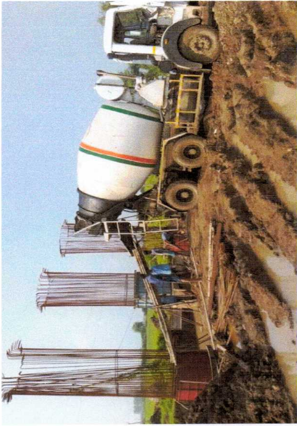
323+074 PIER LEFT & RIGHT SIDE CONCRETE POURING STARTED
