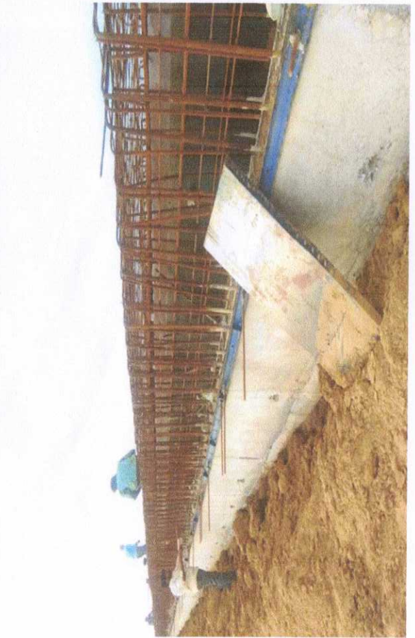
336+930 Cage Binding going on
