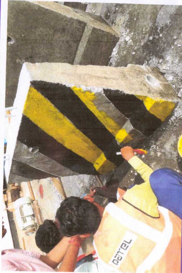
Jersey Crash Barrier Painting Work In Progress
