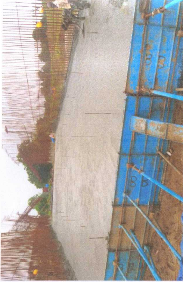
335+402 VUP Raft (RHS) Concrete Pouring Completed
