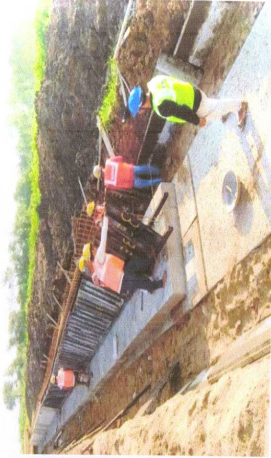
341+700 Toe Wall Shuttering in Progress
