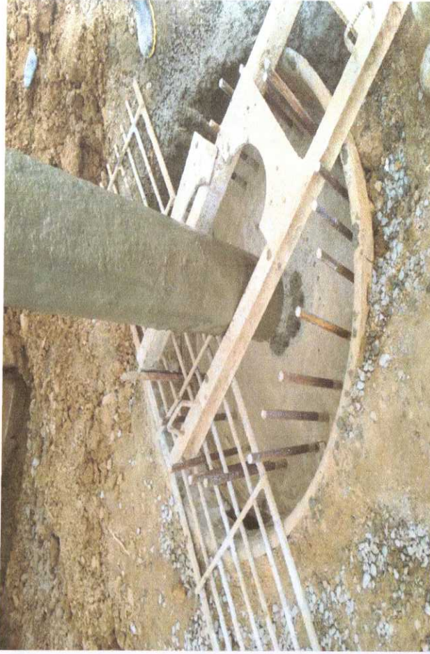
344+383 Flyover Pile No 8 RP1 Work In Progress
