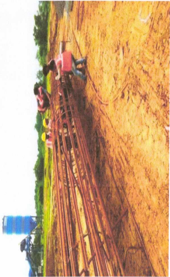
336+930 Cage Binding going on
