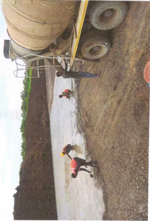
341+600 LVUP PCC Work In Progress
