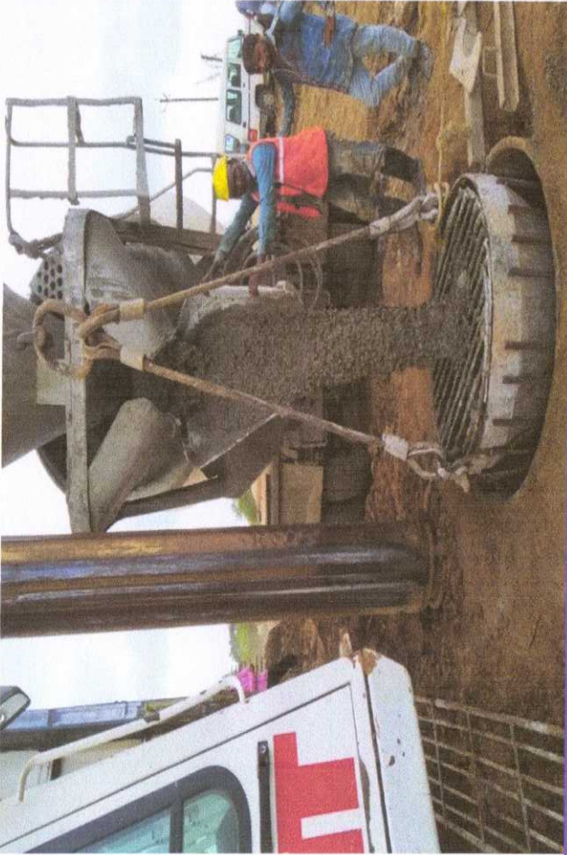
344+383 Flyover Pile No 8 RP1 Concreting Started
