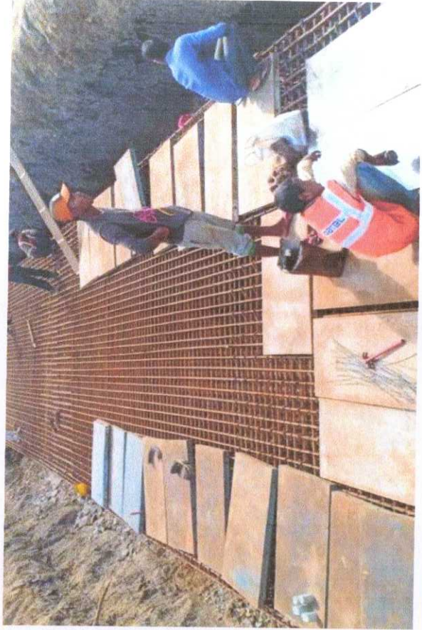
323+074 LP2 Pile cap Reinforcement Binding and shuttering in Progress
