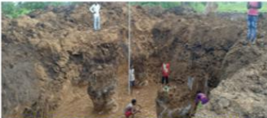
323+074 PILE CAP EXCAVATION WORK ON PROGRESS RA1
