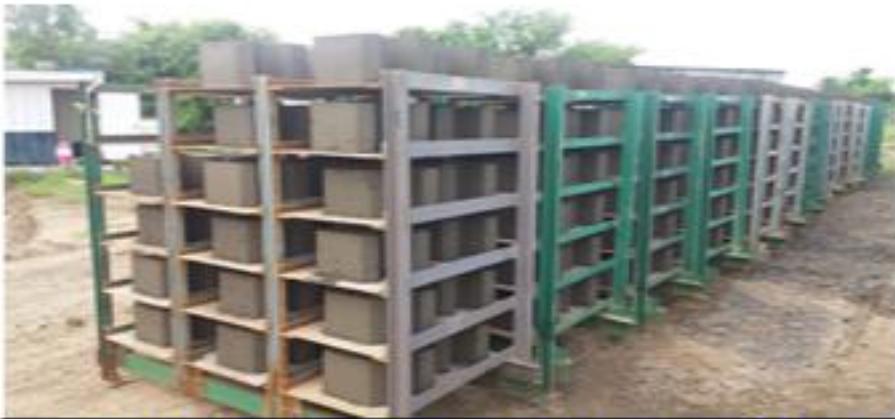
RE WALL BLOCK CASTING IN PROGRESS. 19.08.2019
