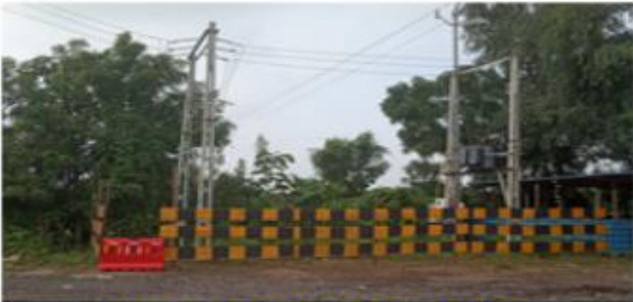
SAFETY AT VIRPUR BASE CAMP
