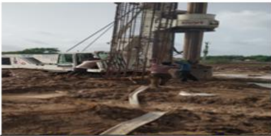
353+666 INTERCHANGE CAGE LOWERING 13.08.2019
