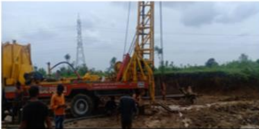
324+193 BORE COMPLETED PILE NO -05 LA2
