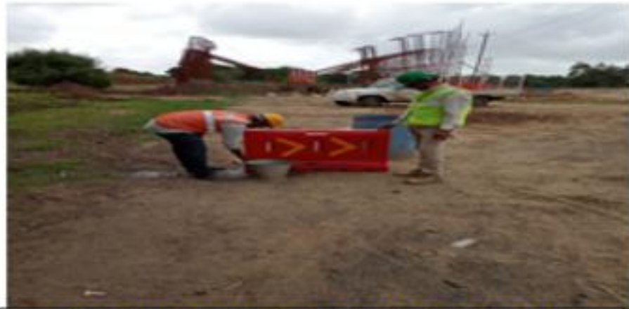
PLACING OF SAFETY BARRIER 20.08.2019
