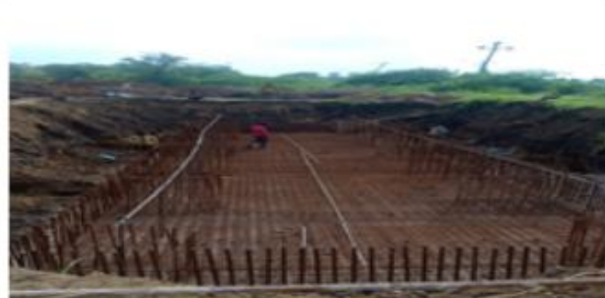
323+074 PILE CAP REINFORCEMENT STEEL BINDING IN PROGRESS FOR LP1
