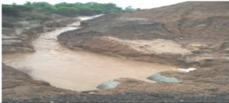
APPROACH FOR MJBR 336+835 DAMAGED / WASHED OUT DURING RAIN AND FLASH FLOODS FROM 31.07.19 TO 08.08.2019
