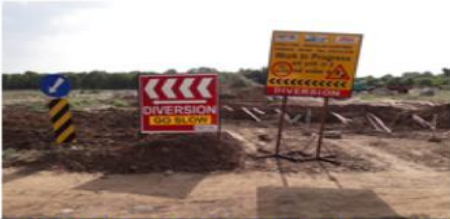
349+441 VOP DIVERSION WORK IN PROGRESS
