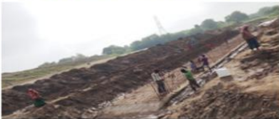
335+664 RAFT REINFORCEMENT WORK ONGOING FOR BOX CULVERT (LHS)
