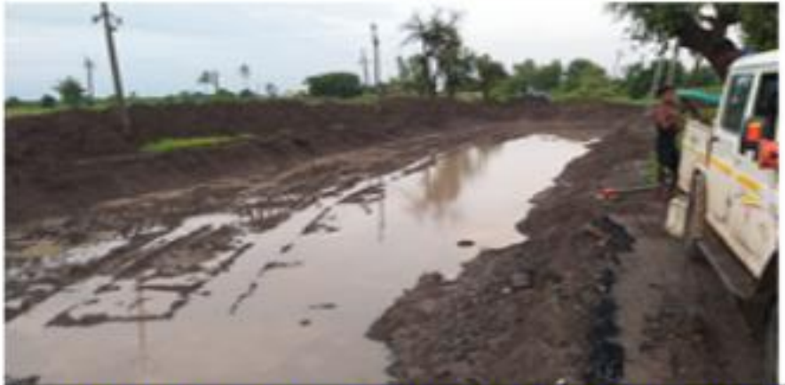
330+402 VUP DEWATERING WORK COMPLETED
