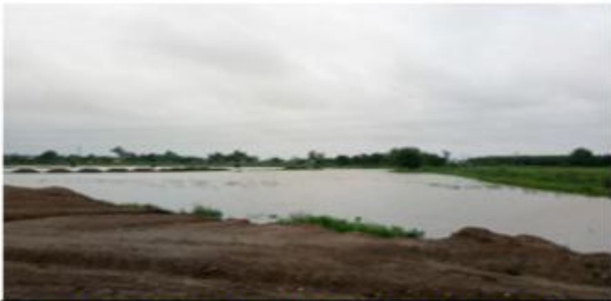
332+050 TO 332+150 FLOODED WATER 10082019
