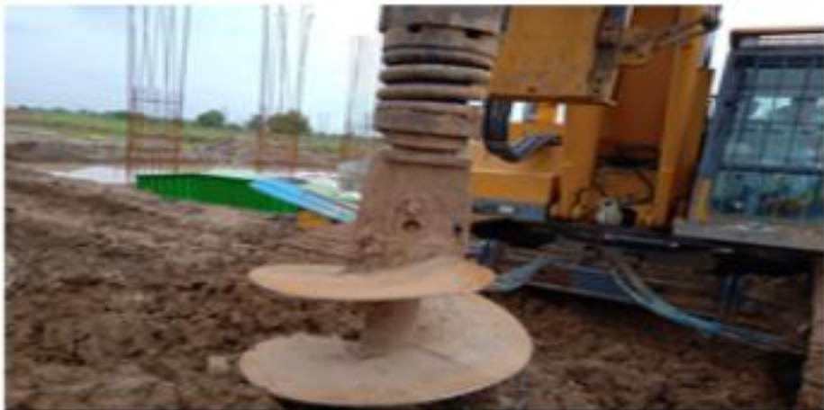
323+074 interchange RP2 Pile no 1 boring start 14.08.2019
