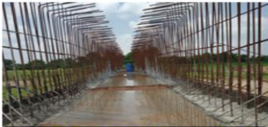
335+074 CURING OF BOX CULVERT LHS RAFT
