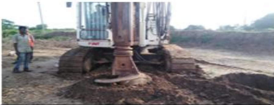
344 +383 BORING STARTED AT RP1 PILE NO 4
