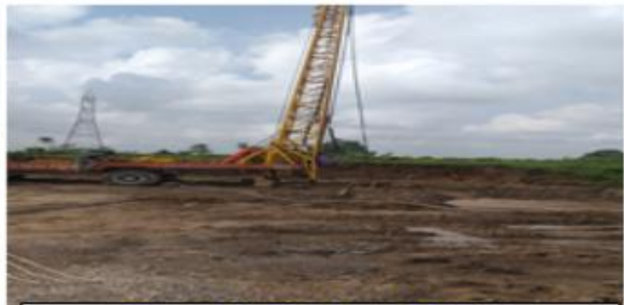
324+193 PILE NO 5 LA 2 BOARING
