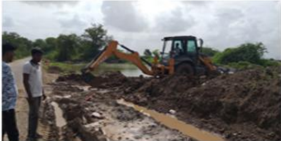
323+074 working front improvement in progress for piling A1
