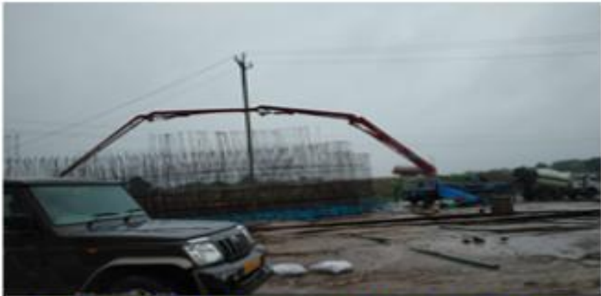
335+402 VUP LHS RAFT CONCRETING IN PROGRESS 16.08.2019
