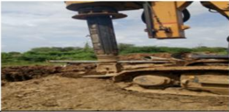
323+074 PILE NO 6 RA 1 BORING START
