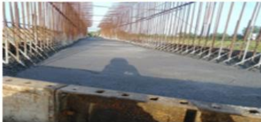
335+075 BOX CULVERT LHS RAFT COMPLETED
