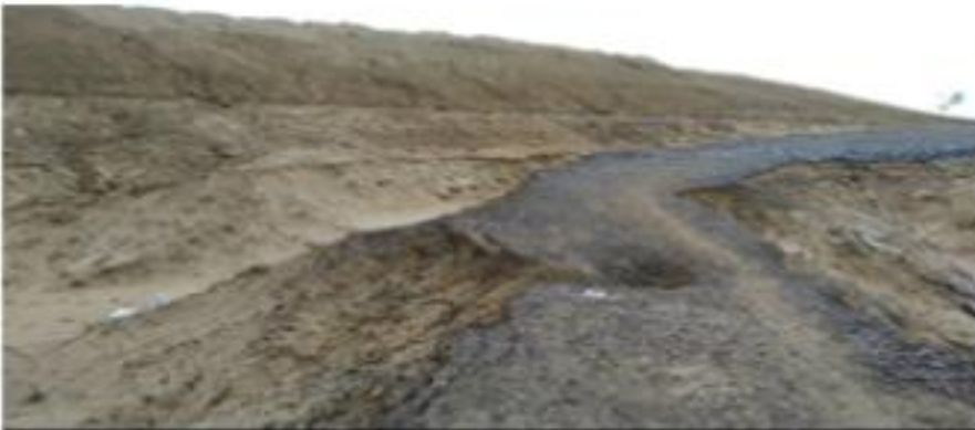
APPROACH FOR MJBR 336+835 DAMAGED / WASHED OUT DURING RAIN AND FLASH FLOODS FROM 31.07.19 TO 08.08.2019
