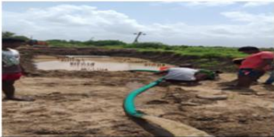
Ch 323+074 pile cap p1 LHS dewatering work start 19.08.2019
