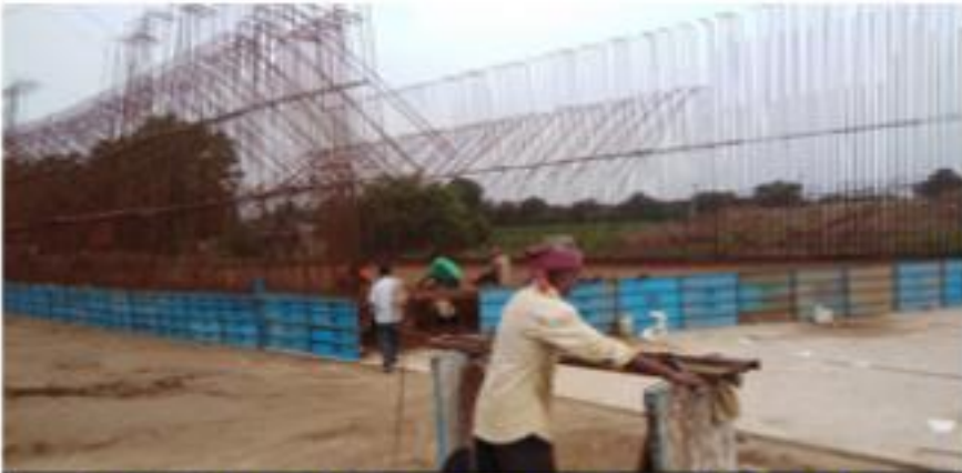
335+402 steel fixing work in progress 14.08.2019
