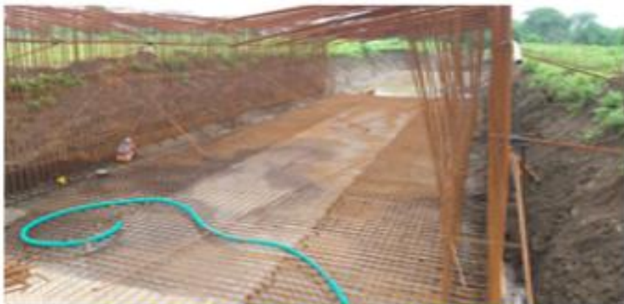
329+062 MUD CLEANING FROM RAFT
