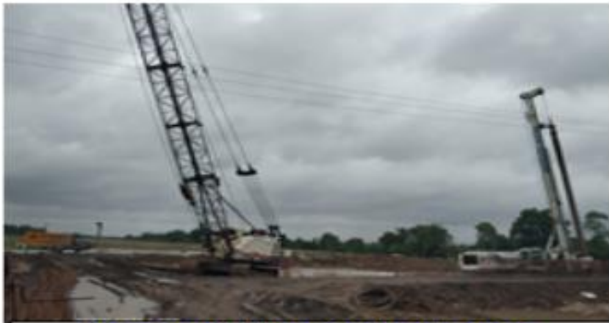
353+666 PILING WORK IN PROGRESS
