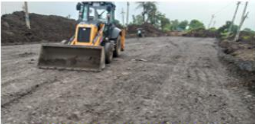
330+402 VUP RHS GSB IMPROVEMENT
