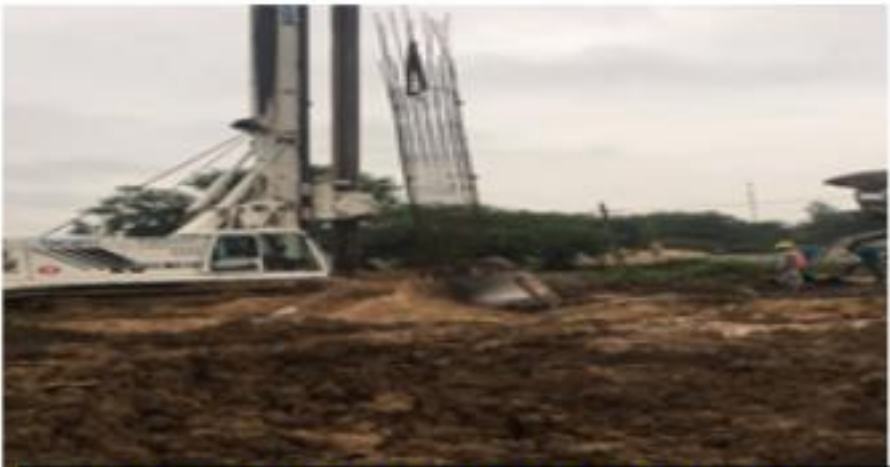
353+666 LP4 PILE NO 4 CAGE LOWERING
