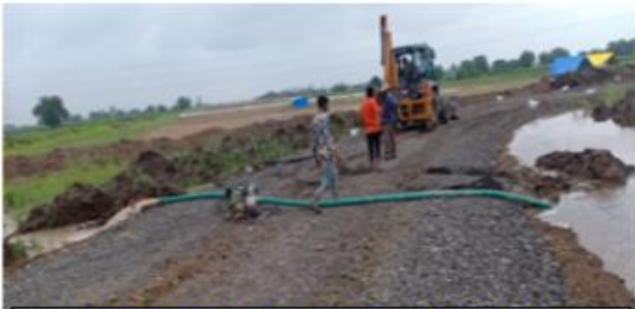
326+957 VOP DEWATERING IN PROGRESS
