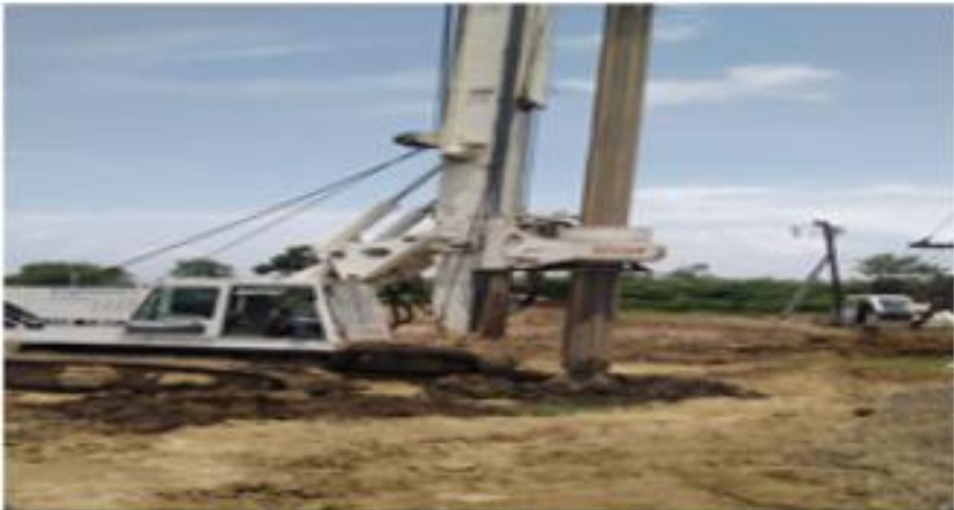
353+666 PILE NO. 6 BORING START OF LPS. INTERCHANGE 21.08.2019
