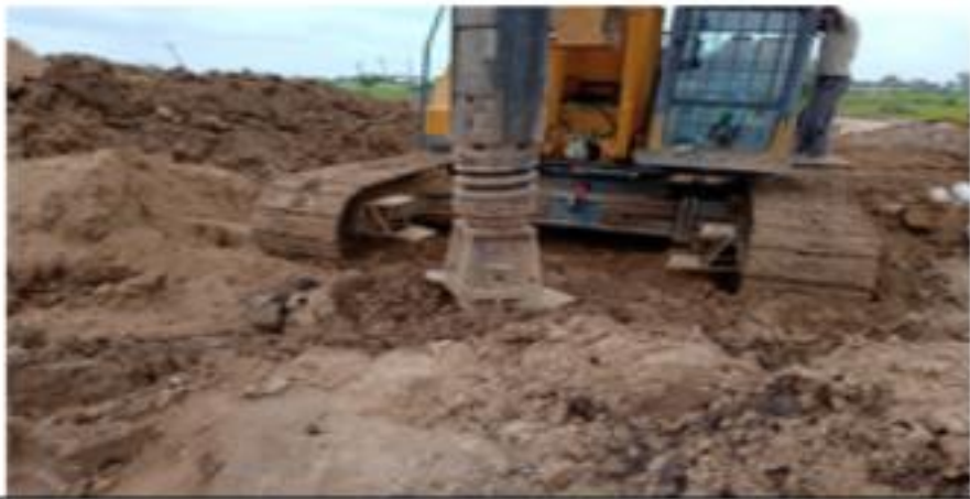
323+074 interchange RP2 Pile No 7 Boring start 15.08.2019
