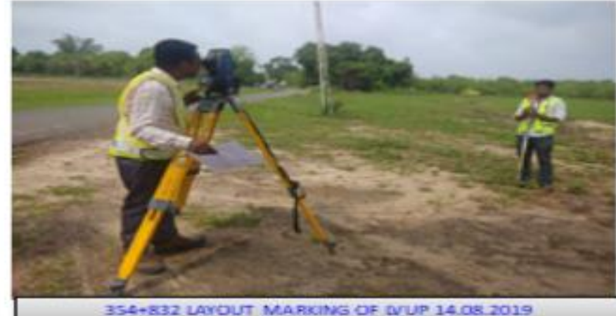
354+832 LAYOUT MARKING OF (VUP) 14.08.2019
