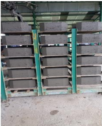
RE Wall Block casting in Progress
