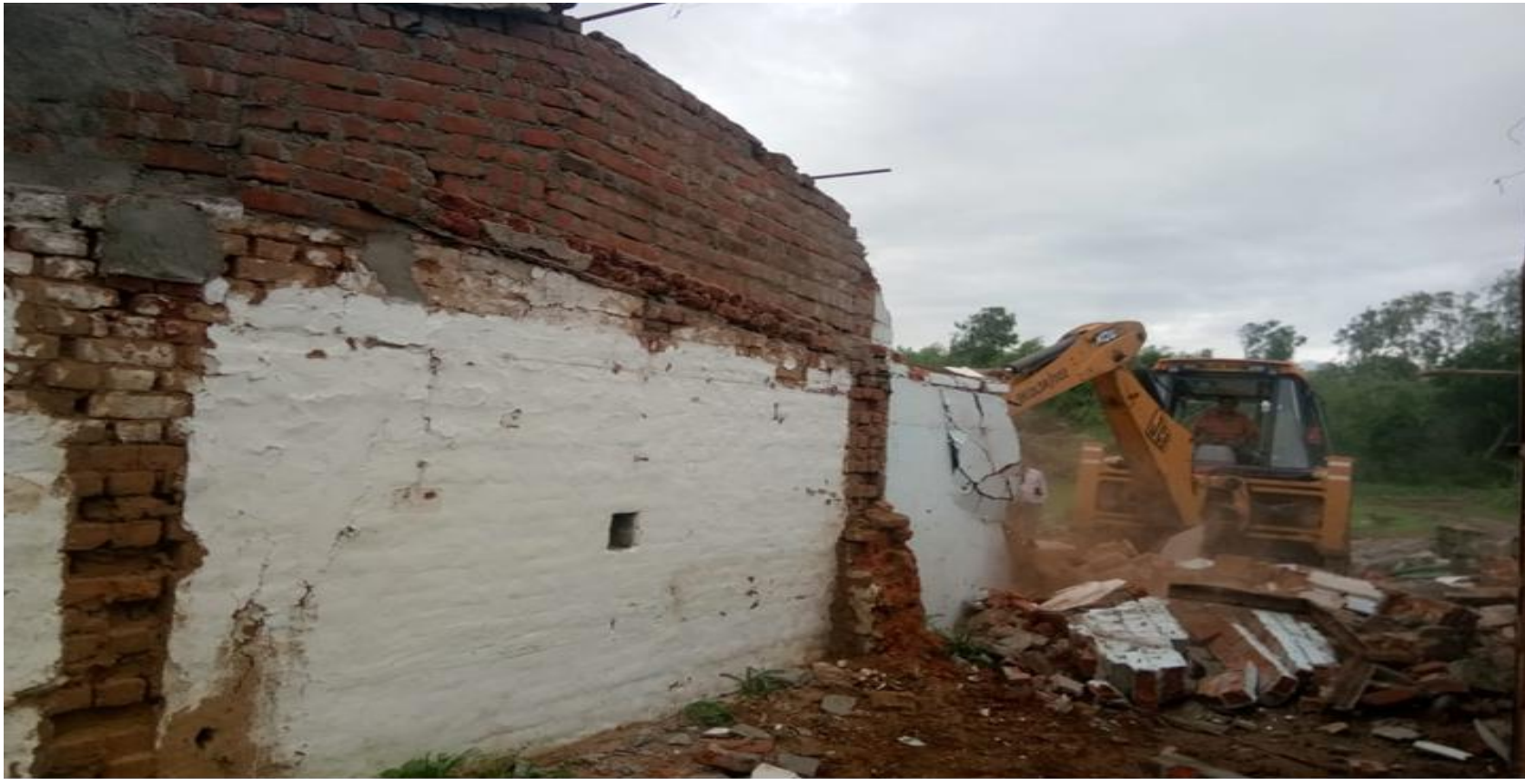
Ch. 353+700 - House dismantling
