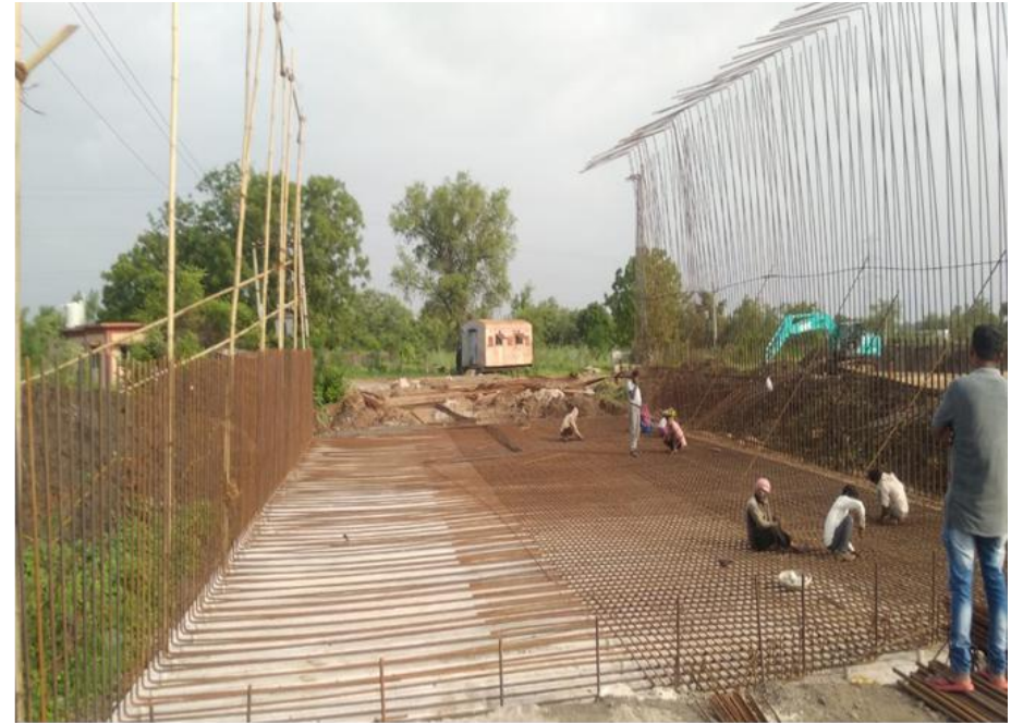
Ch. 341+824 - VUP Steel Binding
