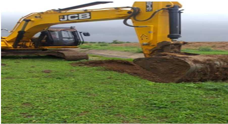
Ch. 324+236 - Box Culvert Excavation
