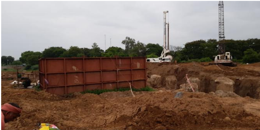
Ch. 349+045 - VOP Piling work
