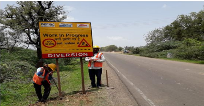
Safety Sign Board Installation
