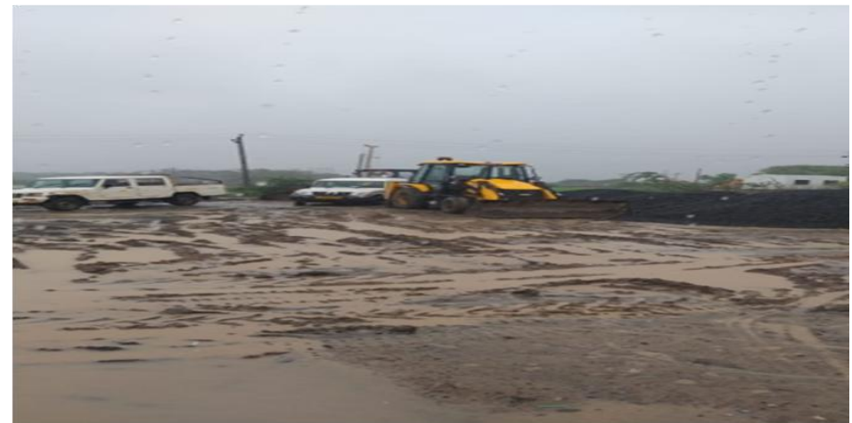
Ch. 323+074 - Heavy Rainfall at Interchange
