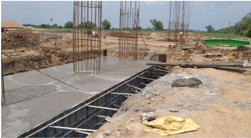
Ch. 323+074 - Interchange Pile Cap Concreting
