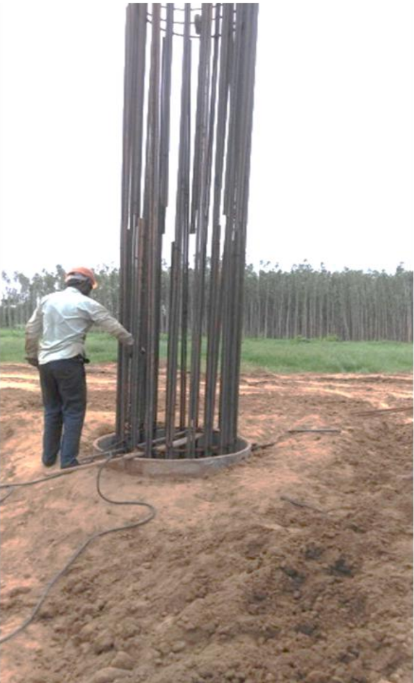
Ch. 343+566 - Minor Bridge Cage Lowering
