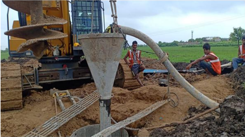
Ch. 323+074- Interchange Pile casting
