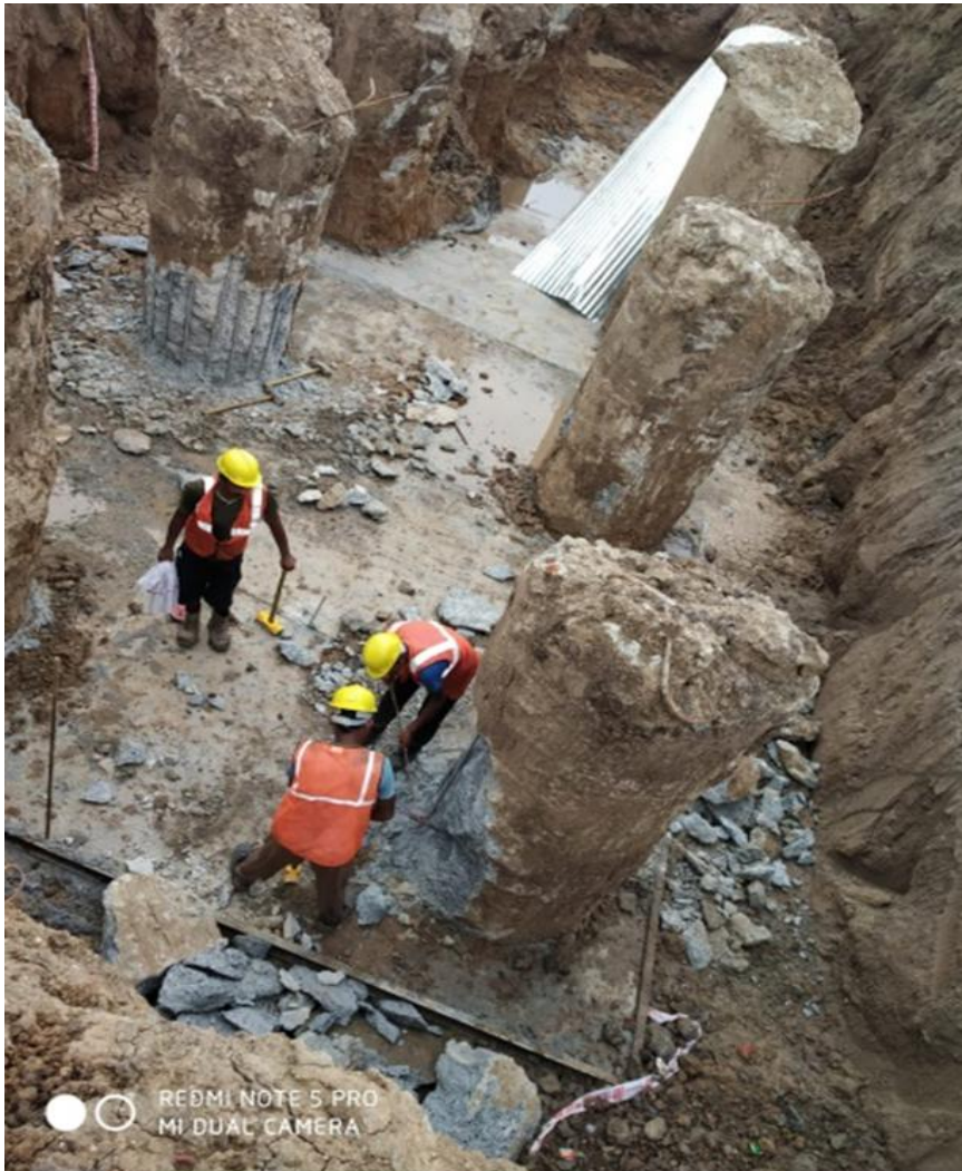
Ch. 353+666 - Interchange Pile Chipping Work
