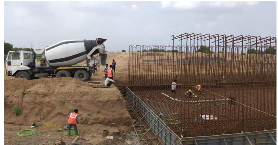
Ch. 324+410 - CUP Raft Concreting
