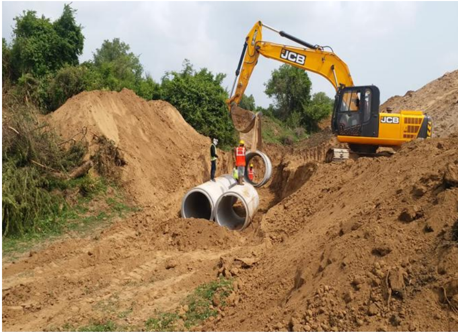
Ch. 337+050 - Pipe laying for approach road
