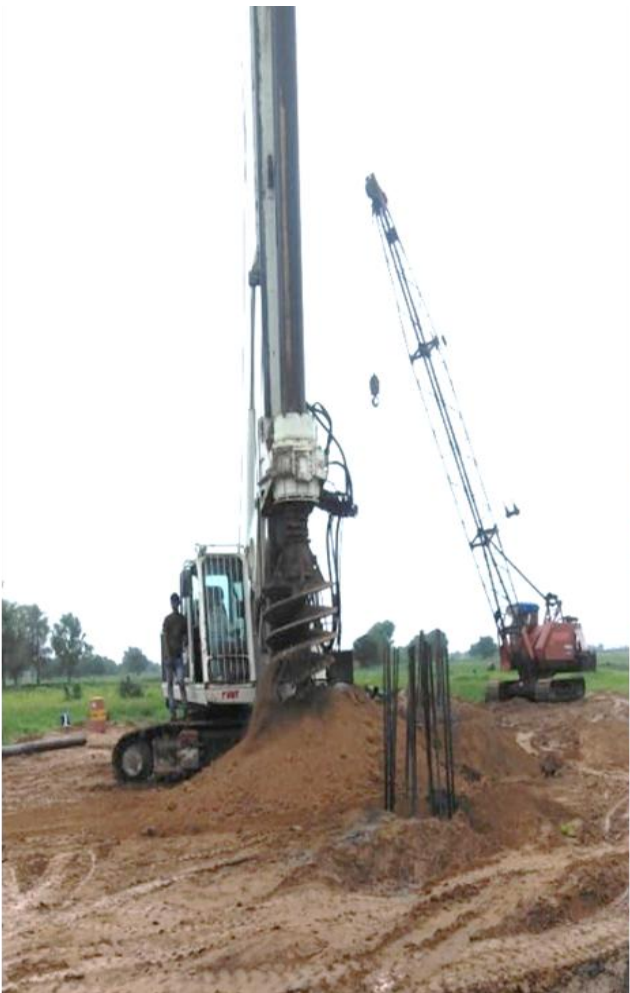
Ch. 343+566 - Minor Bridge Pile Boring
