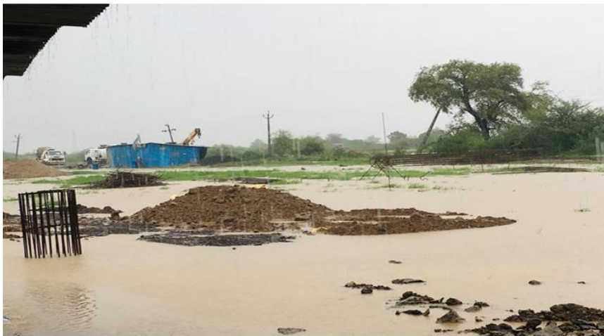
Ch. 323+074 - Heavy rainfall at Interchange
