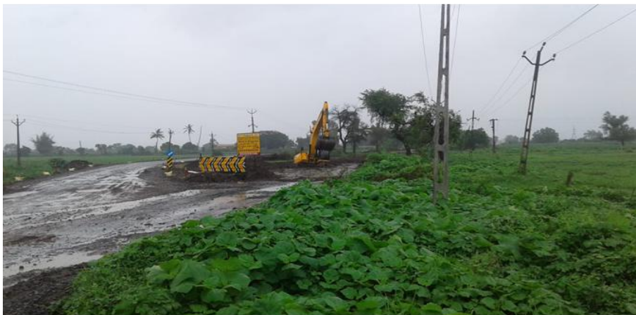
Ch. 330+402 - VUP Excavation work
