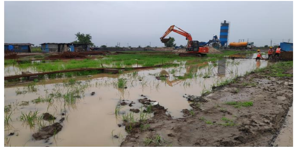
Ch. 323+074 - Work stopped due to Rain
