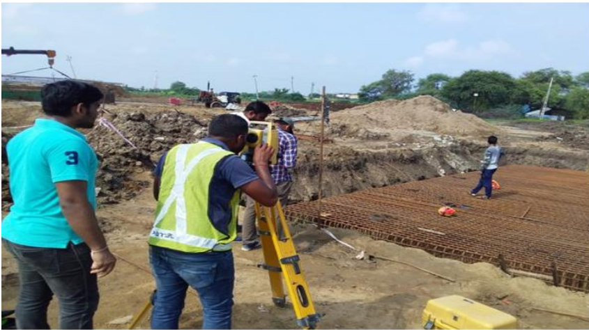
Ch. 323+074 - LHS Pile Cap layout marking
