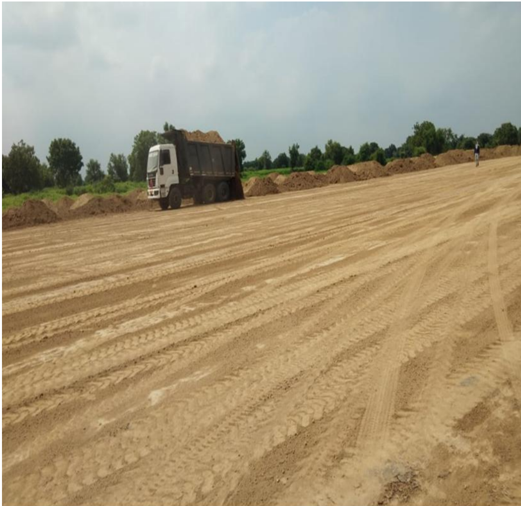
Ch. 344+500 - Soil Dumping
