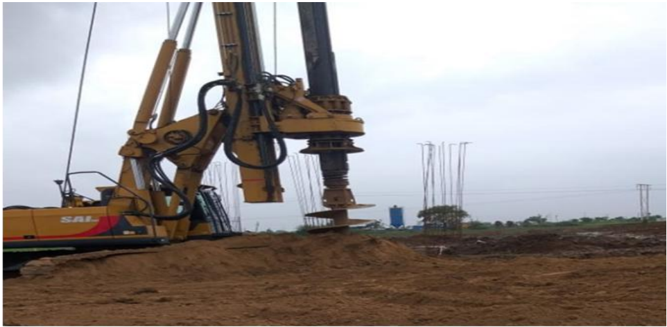
Ch. 323+074 - Interchange Pile Boring
