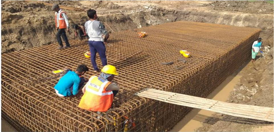
Ch. 323+074 - Pile cap steel binding work
