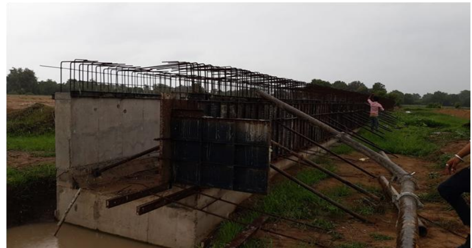
Ch. 349+809 - Box culvert LHS Wall 1st Lift Casting
