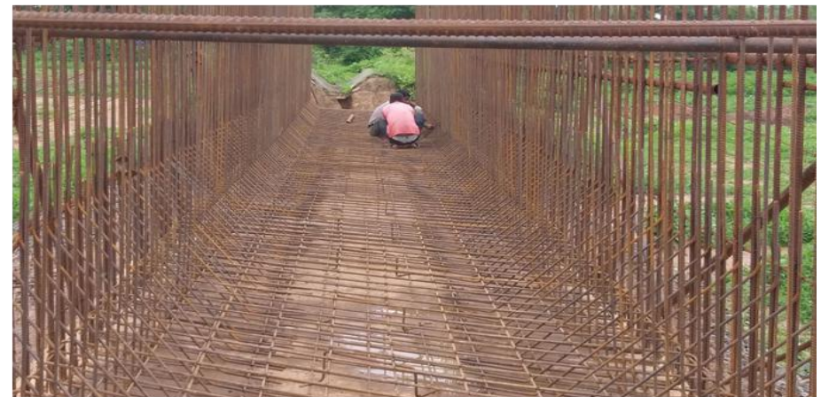
Ch. 335+074 - Box Culvert Reinforcement
