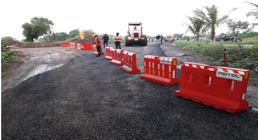
Ch. 349+400 - DBM laying for Diversion
