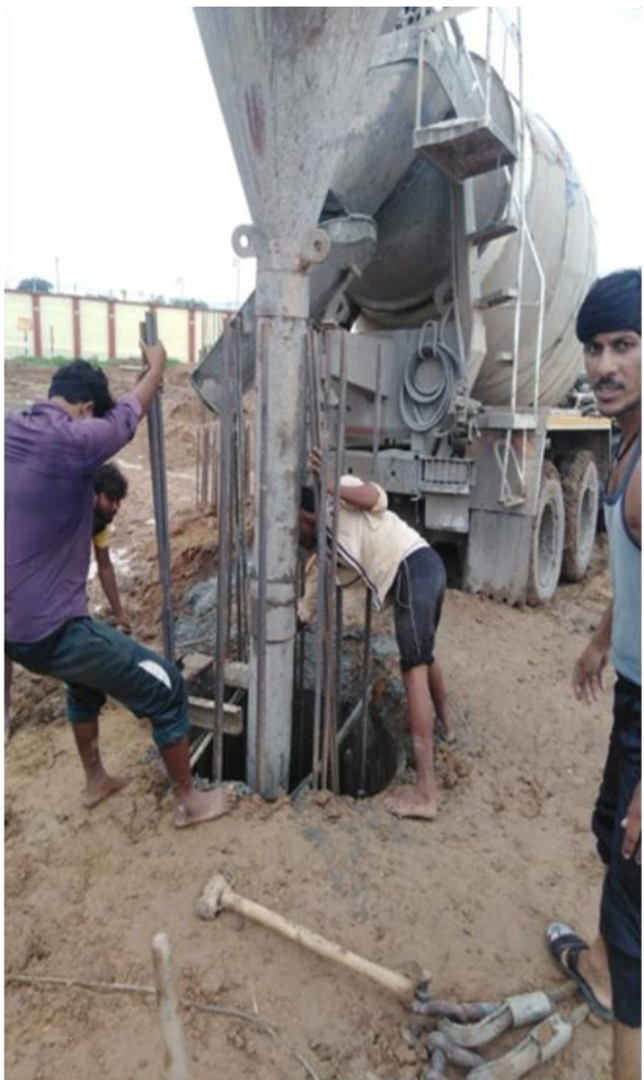
Ch. 343 +566 - MNB Casting of pile 7 segment 3 abutment 2
