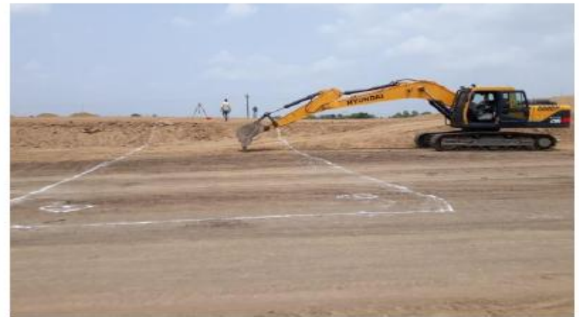
Layout and Excavation of Box Culvert ( CH: 323+425)
