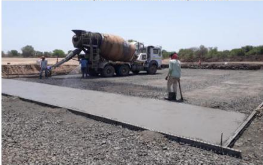
Leveling Coarse at CUP
