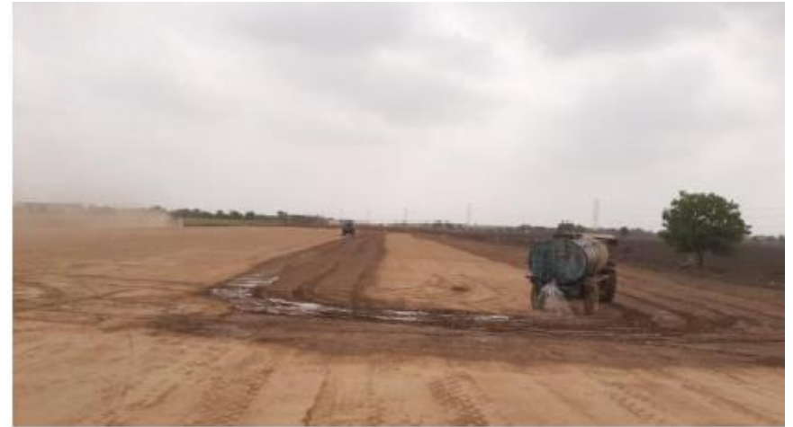
Watering on Embankment (339+200 to 339+400)
