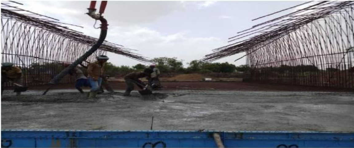
Concreting in progress (CH: 336+020)
