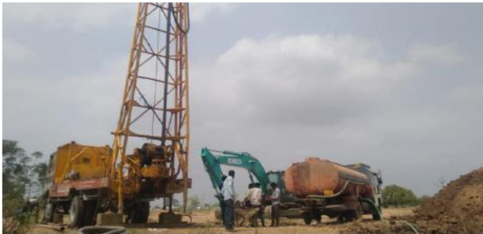
Test pile Boring (CH: 344+383)
