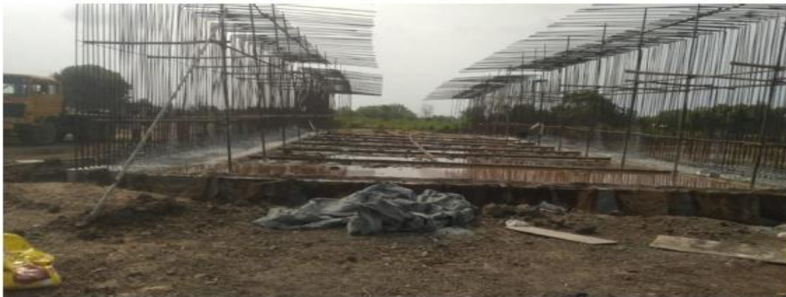
Water pounding for Curing at CUP (CH: 340+855)
