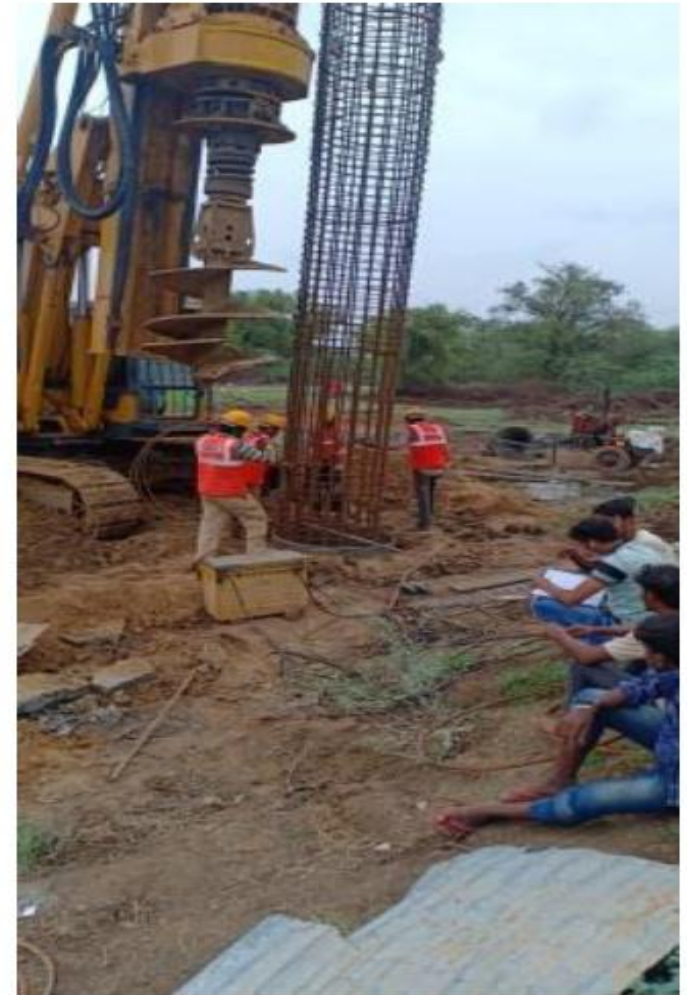
Piling work at Interchange (CH: 323+075)
