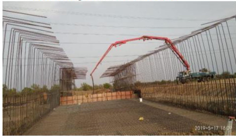
Raft Concreting of CUP
