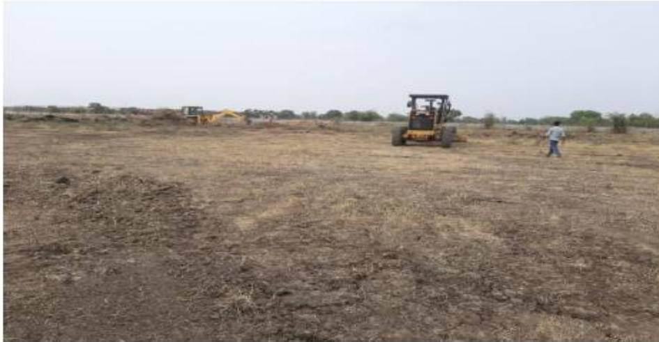
Clearing & Grubbing in progress (CH: 328+000 to 328+420)
