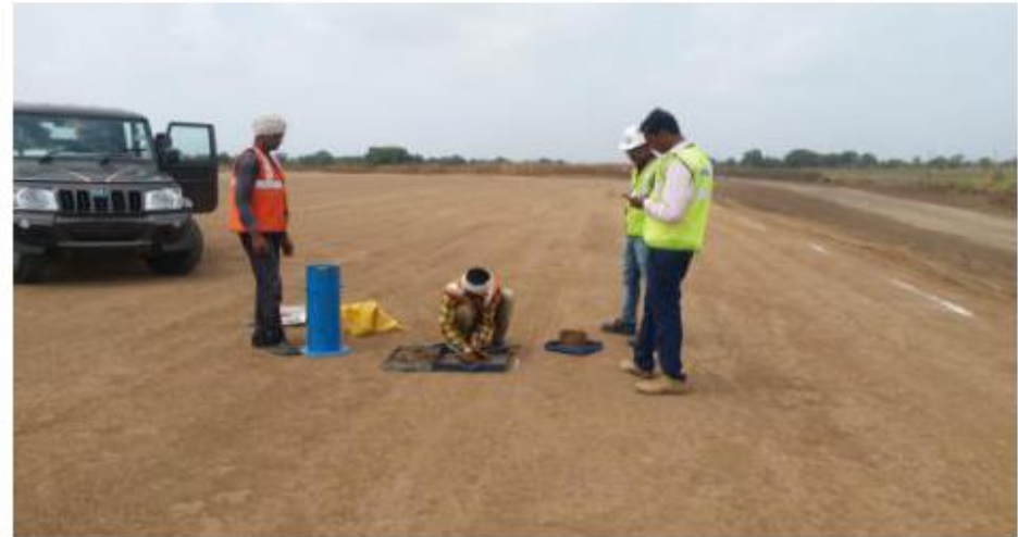
FDD Testing of Embankment at Site
