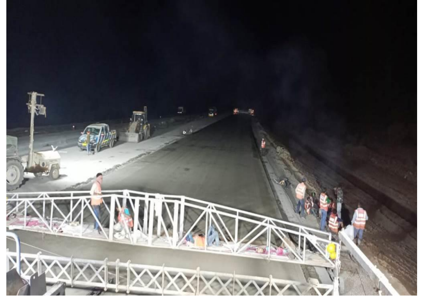
PQC Laying surface 350+295 to 350+740 LHS
