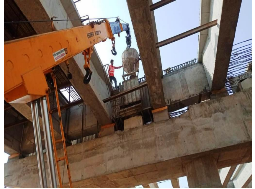
353+666 Interchange RP6 End X Girder concrete Pouring
