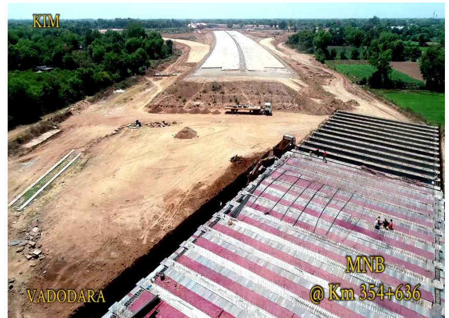
Shuttering work for Slab at MNB 354+636
