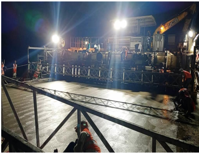
PQC Laying 350+295 to 350+740 LHS shoulder
