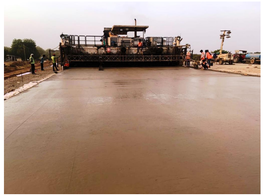
PQC Laying 350+295 to 350+740 LHS shoulder
