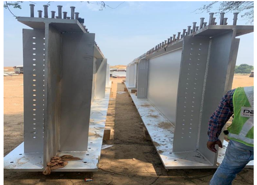
352+946 ROB steel girder assembling work
