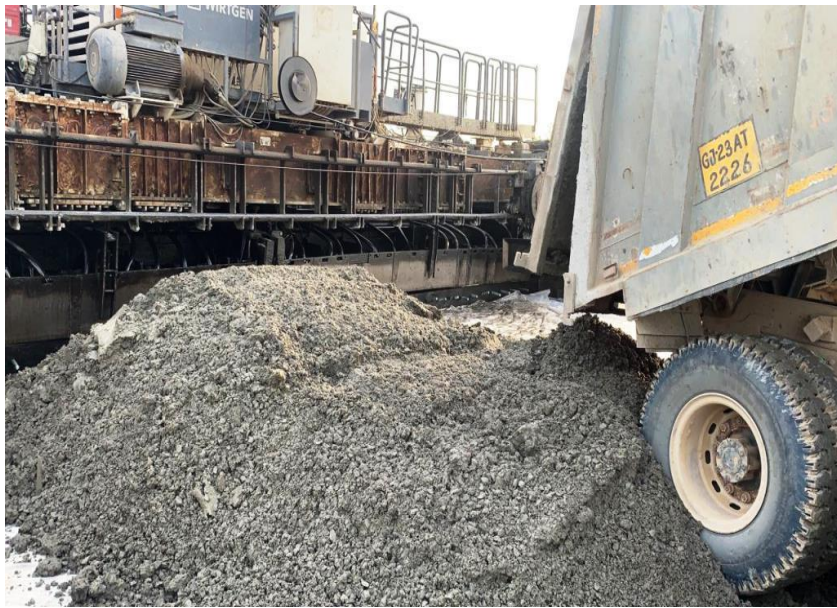
PQC Laying 350+295 to 350+740 LHS shoulder
