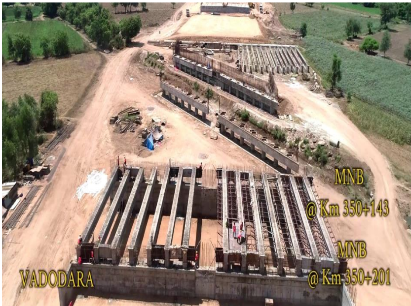
Shuttering Work for Slab at MNB 350+201
