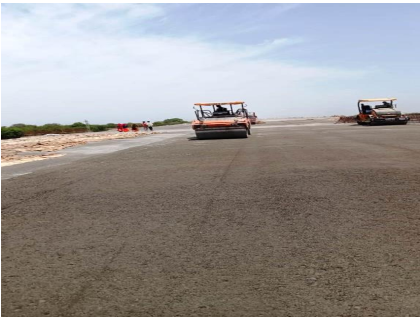
DLC laying at ch 331
