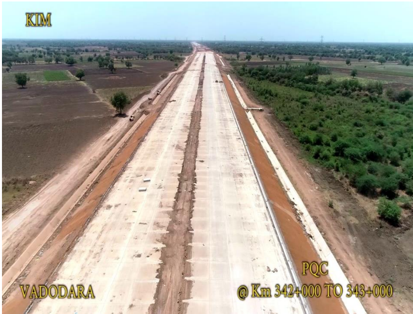
Slope Protection by Coir Mate technology 342 to 343
