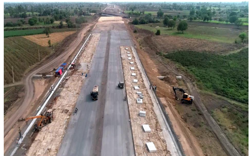
Precast U Drain Placing 331
