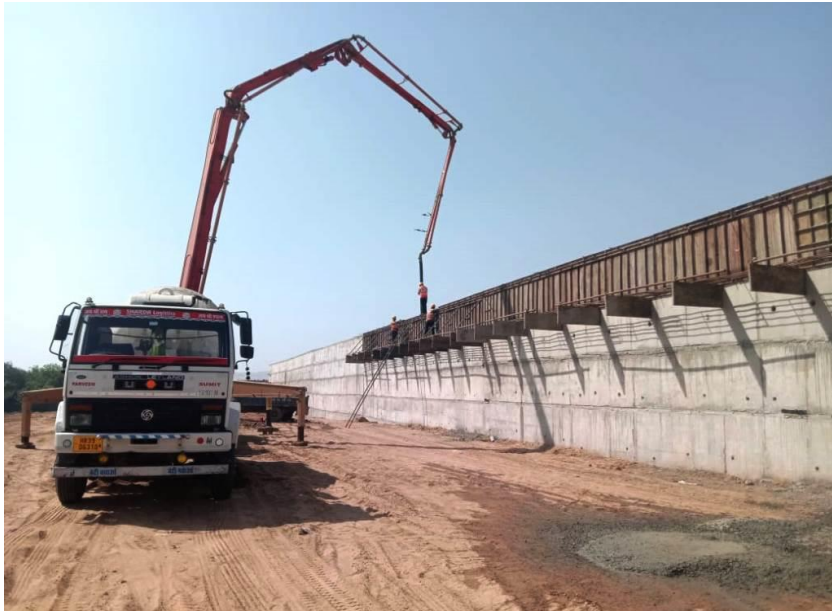
Retaining Wall Final Lift concrete Pouring 353+165 to 353+185
