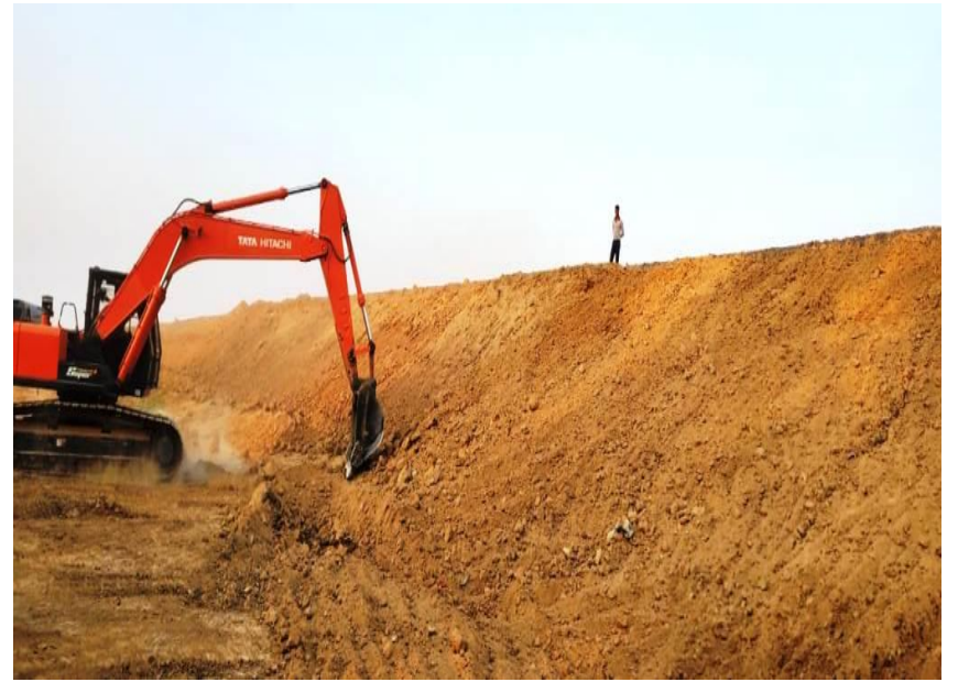
Slope Dressing work at km 350
