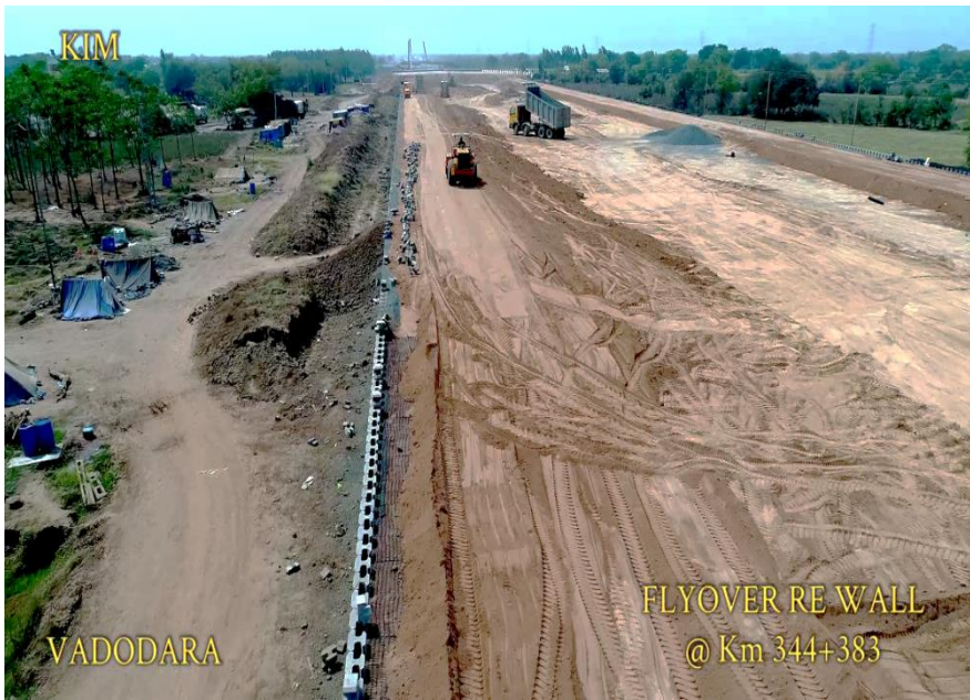
RE wall Flyover 344+383
