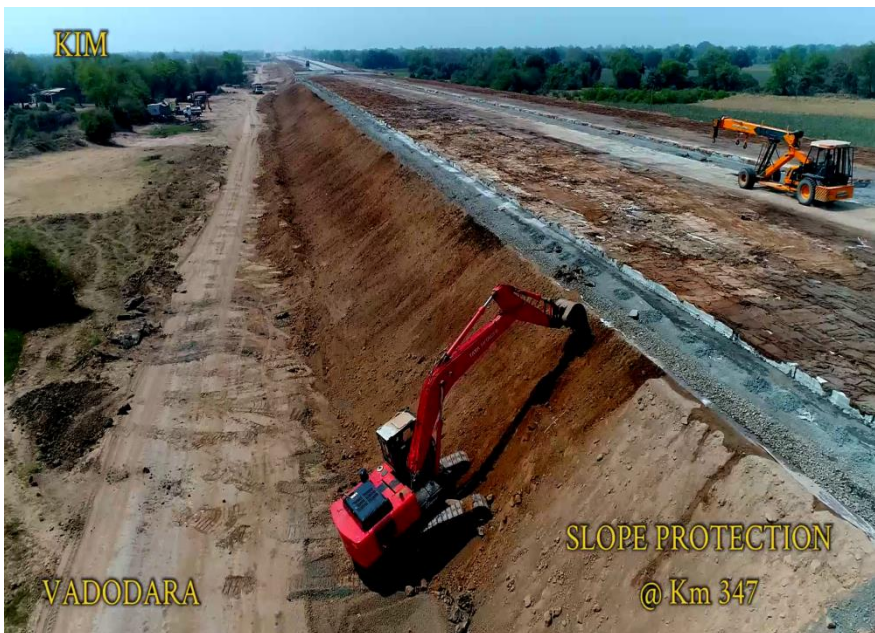
Slope Protection work 347
