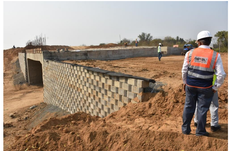
Reinforced Earth wall for structure Approach
