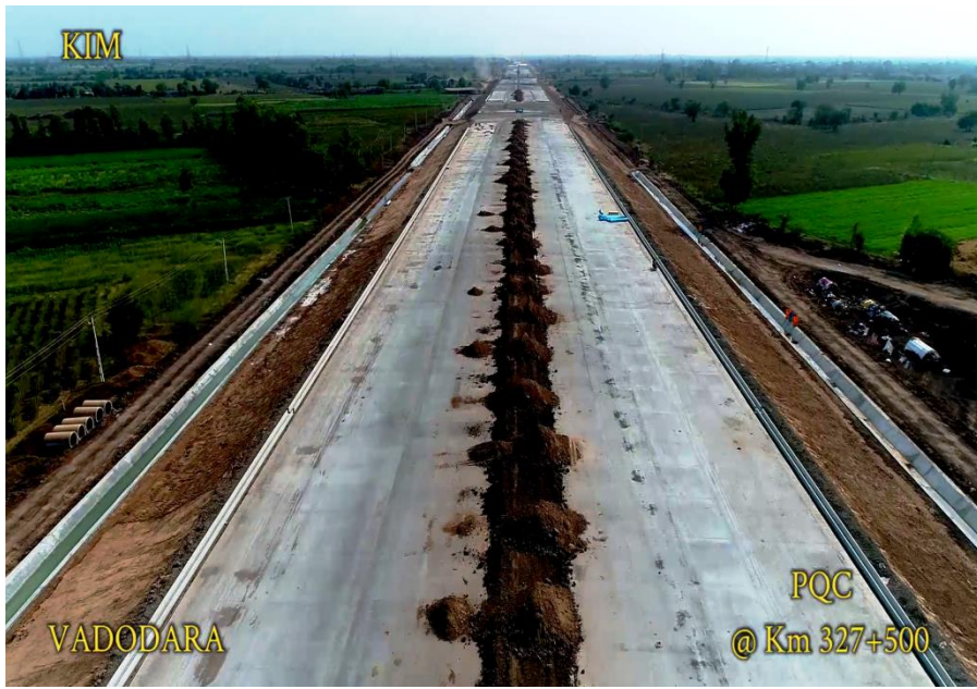
Road status- PQC, Pre cast U Drain, Toe Drain 327+500
