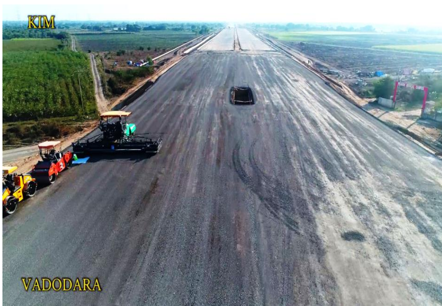
DLC work is in Progress at km 338
