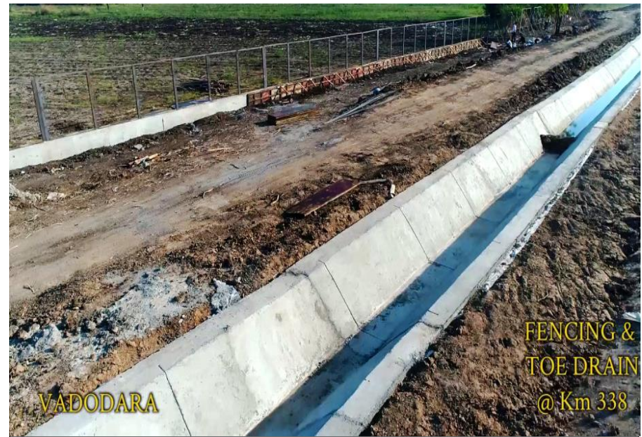
Fencing & Toe Drain at Km 338
