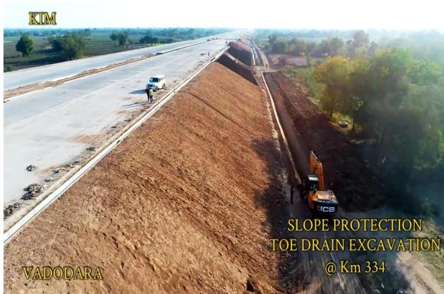
Slope protection work & toe drain excavation at km 334
