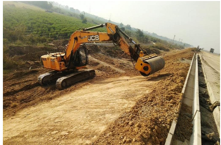
Slope rolling work going on@349+850 RHS
