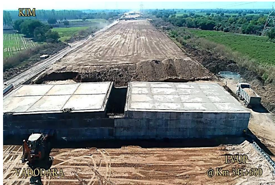
341+600 LVUP Approach RS Wall in Progress
