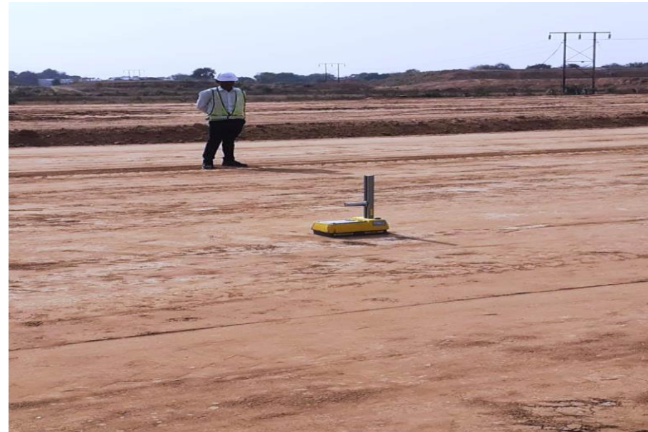
FDD TESTING Ramp 3 at ch 0+560 to 0+760 3rd LHS
