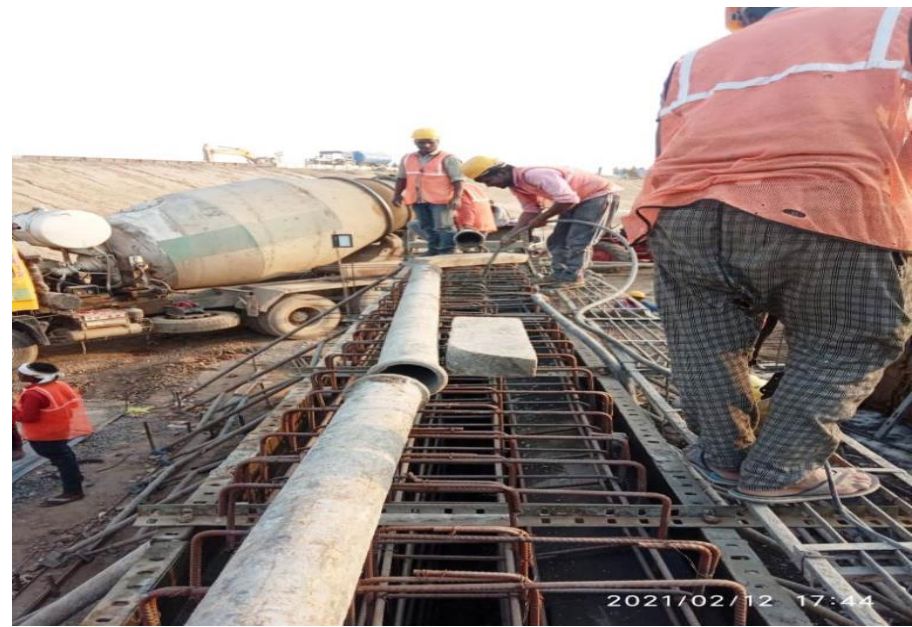
336+810 MJB PSC Girder concrete Pouring work
