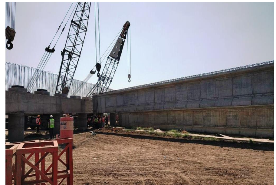
343+566 MNB girder launching Work
