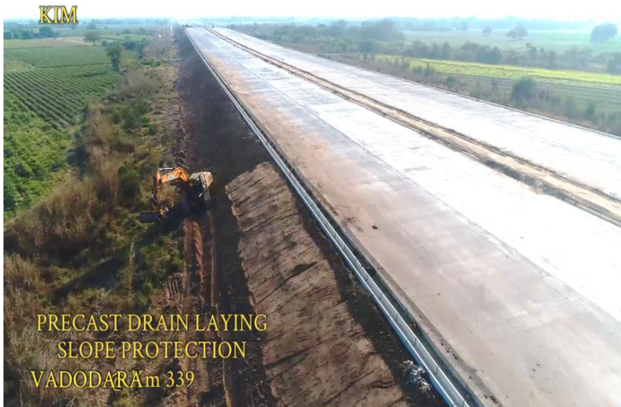
Precast U Drain & Slope Protection at km 339
