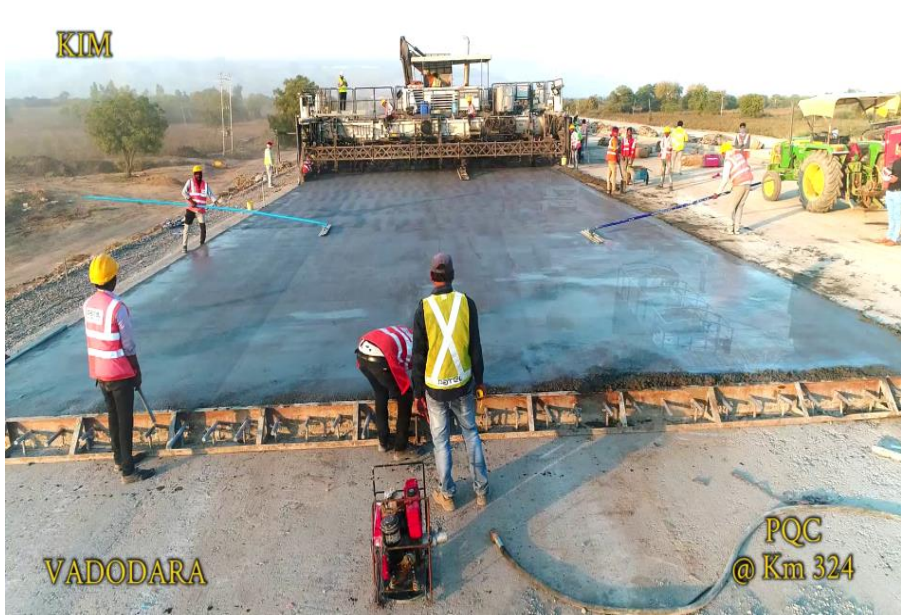
PQC Work at Km 324
