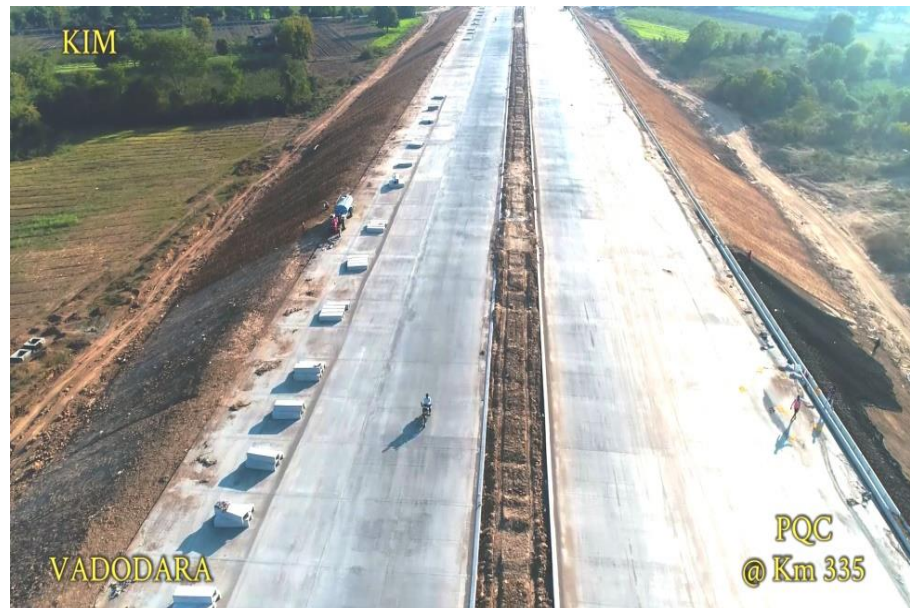
Slope Protection with GEO Cell & Coir Mate at Km 335
