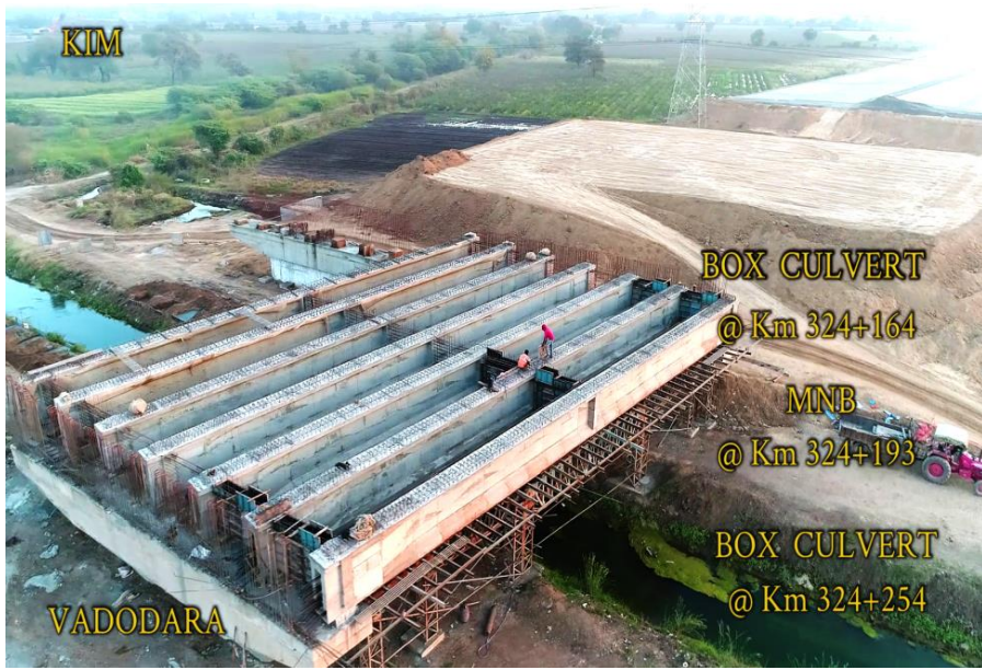
324+193 MNB cast in situ PSC Girder
