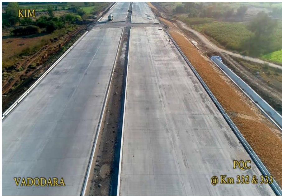
Road Status from KM 332 to 340
