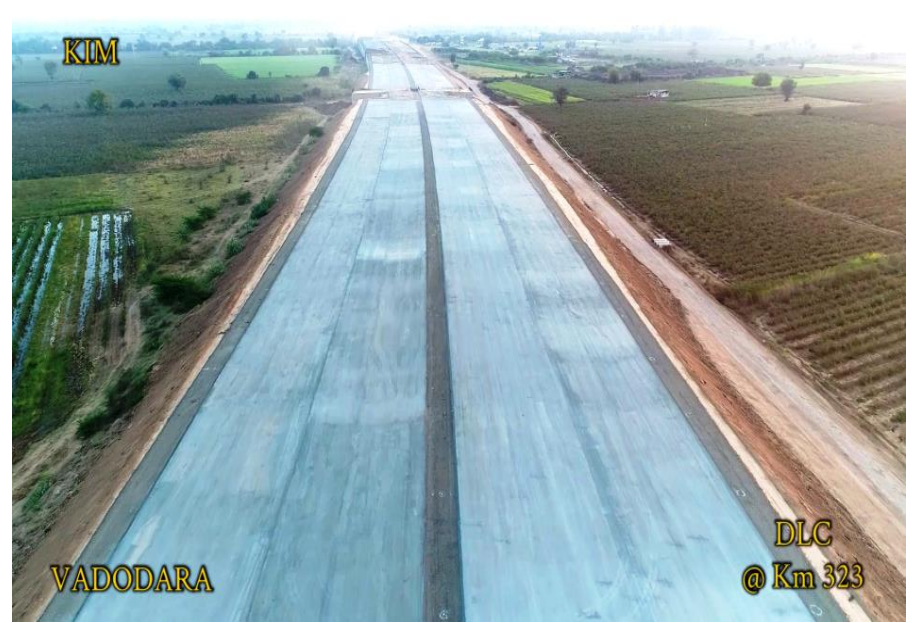
DLC work at Km 323
