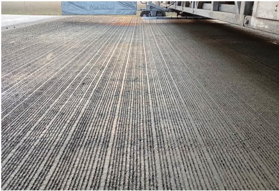
Texturing of PQC 326+464 to 326+791 LHS
