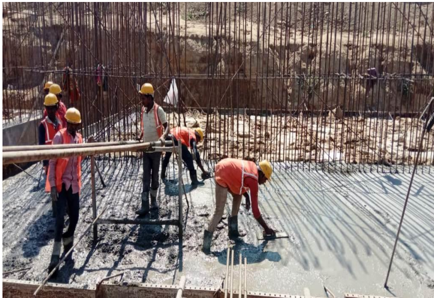
336+810 MJB LA1 Pile cap Casting Completed
