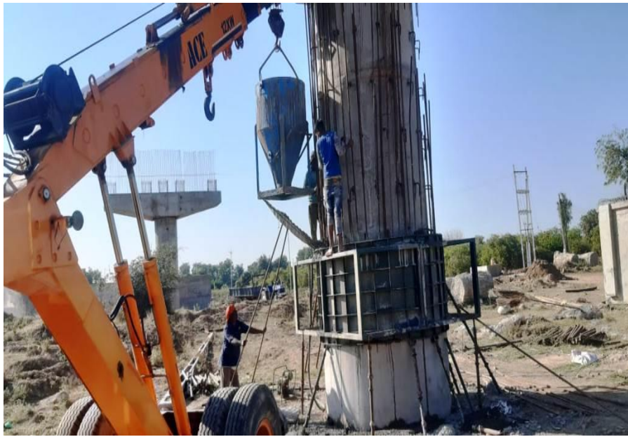
349+441 VOP 2nd lift jacking Pouring in progress
