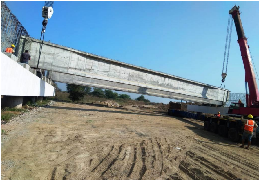
330+640 MNB Girder launching in Progress
