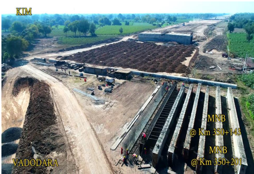
350+143 MNB approaches earthwork in Progress
