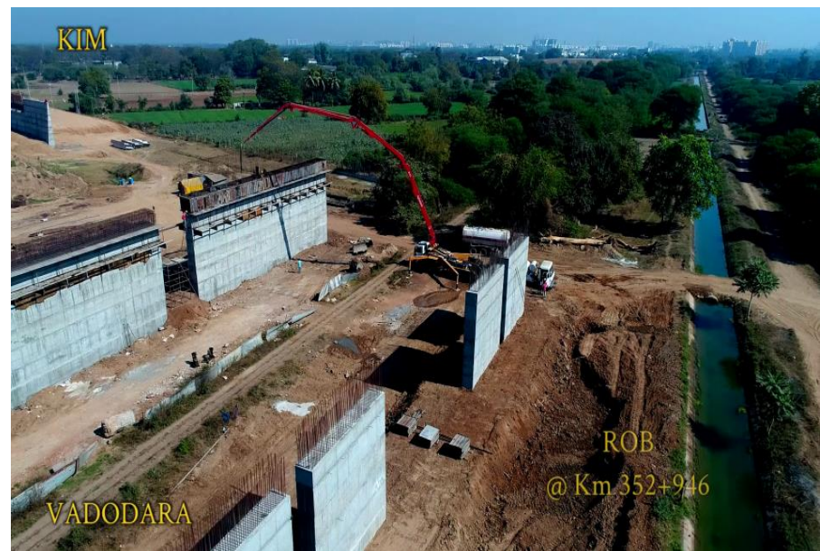
352+946 ROB Abutment wall work in Progress
