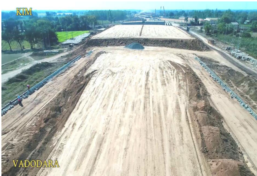
344+360 to 344+100 Approach & RS Wall of flyover in Progress
