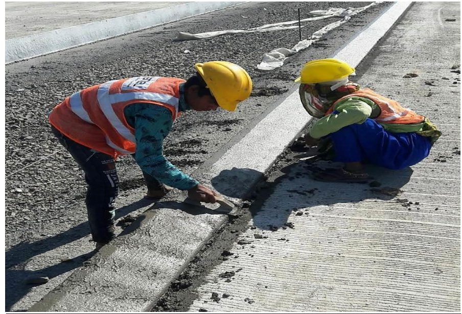
Kerb Finishing at ch 326 + 600
