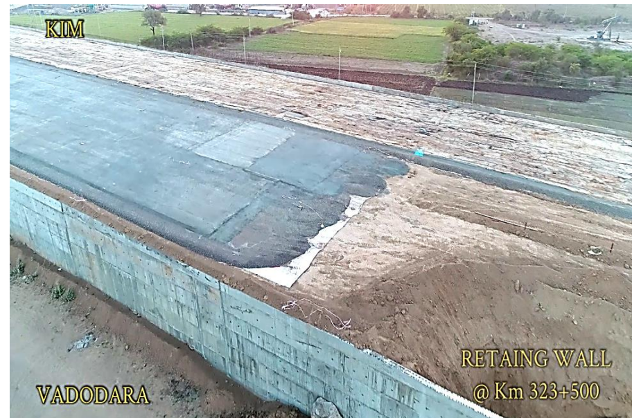
323+500 Retaining Wall completed Page 78 of 89
