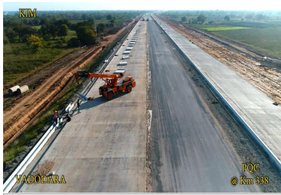
Precast U Drain Placing work is in Progress at Km 338
