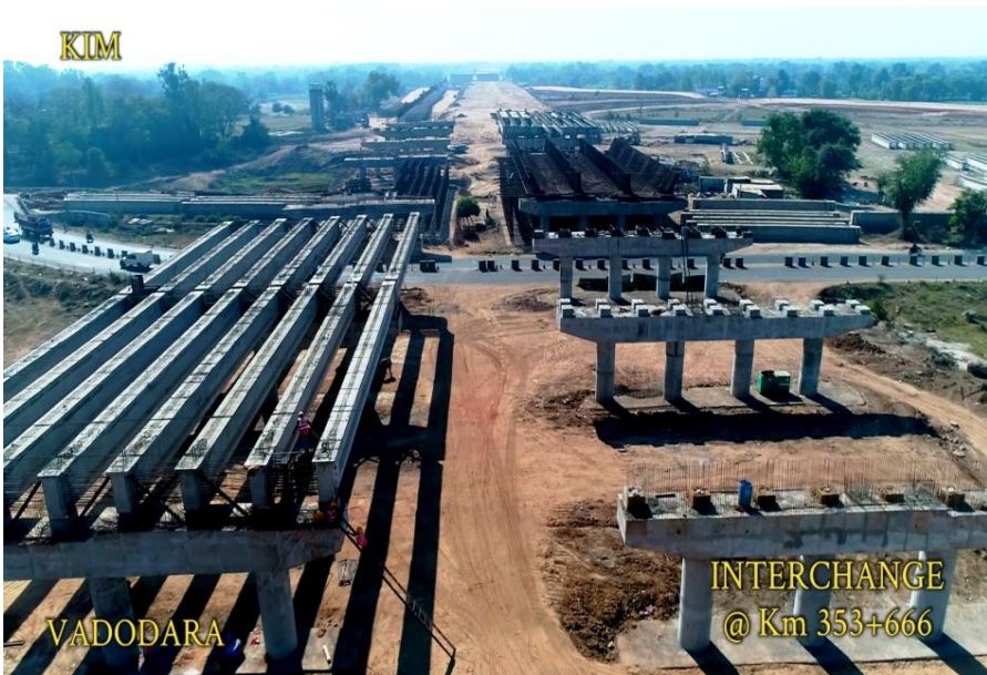
353+666 Interchange Girder launching in progress
