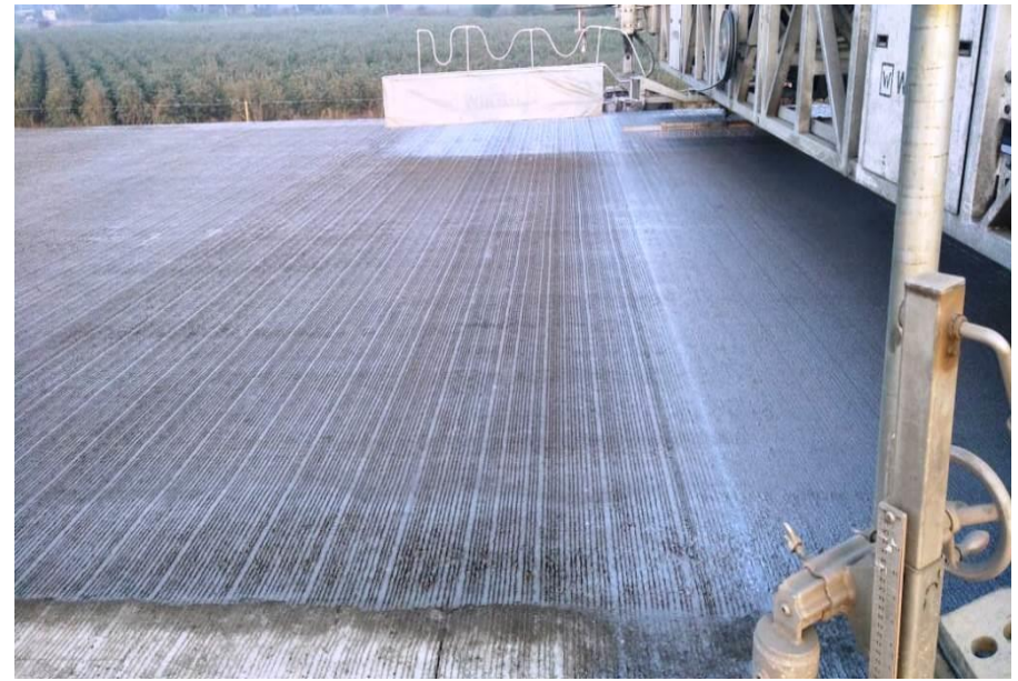
Curing compound spraying 326+459 to 326+786 LHS
