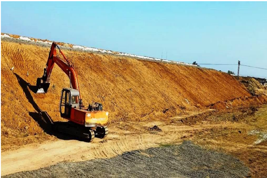
Slope Dressings CH 354+040 TO 354+200 LHS
