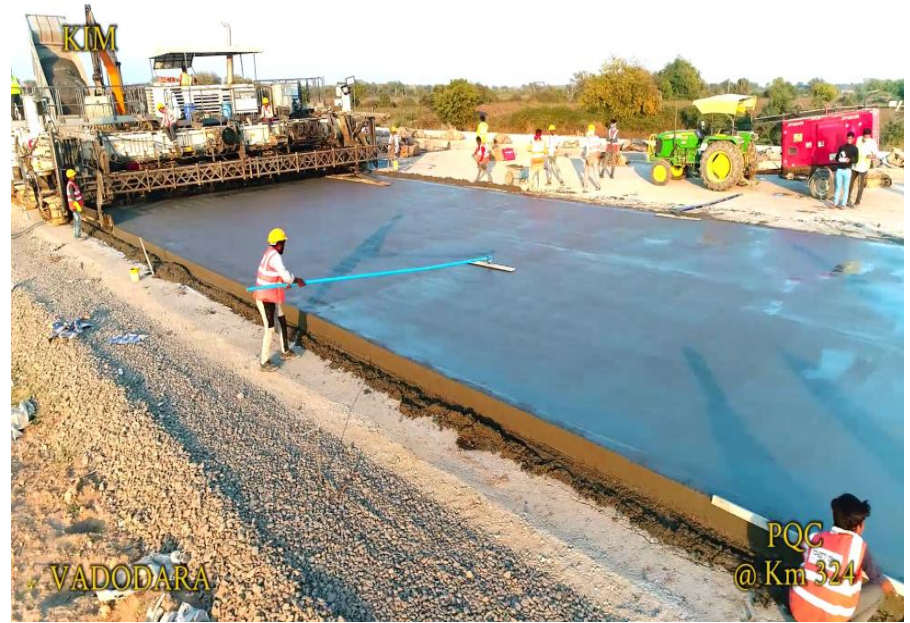
PQC Work at Km 324
