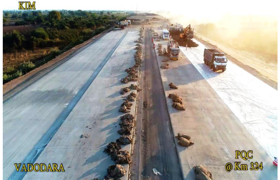
PQC Work at Km 324
