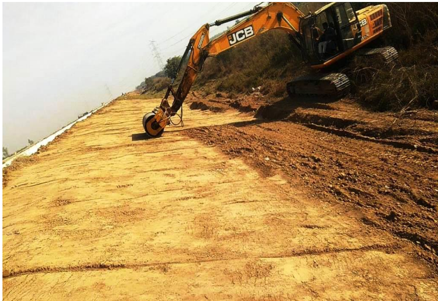
Slope Rolling work going on@340+200 RHS
