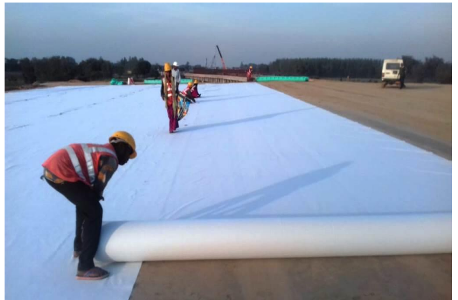
Geo Textile Laying at ch 343+200
