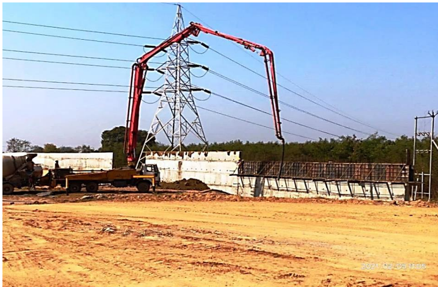
Retaining wall 4th Lift concrete Pouring 331+990 to 332+010
