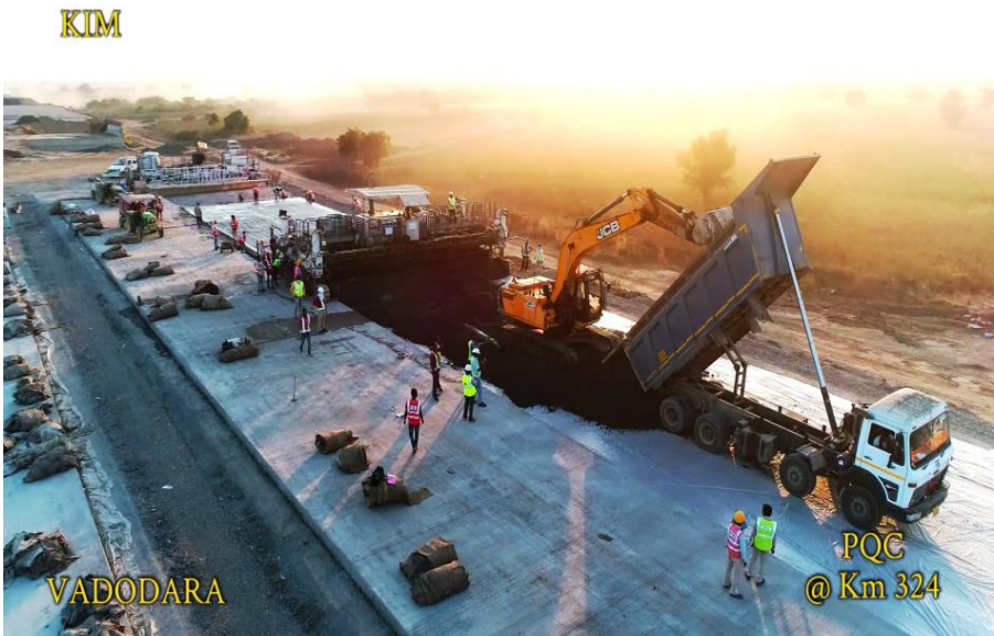
PQC Work at Km 324
