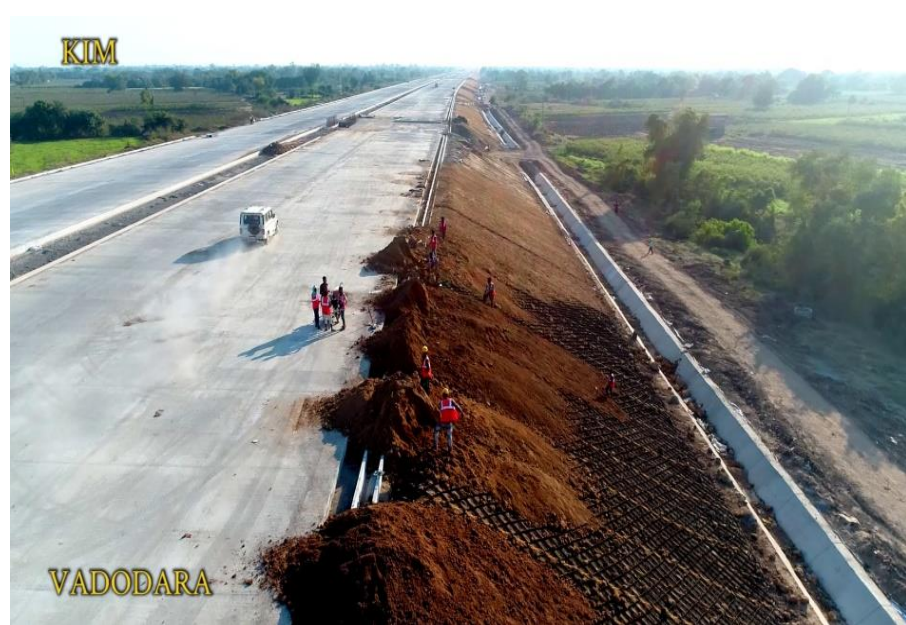
Slope Protection with GEO Cell at KM 334
