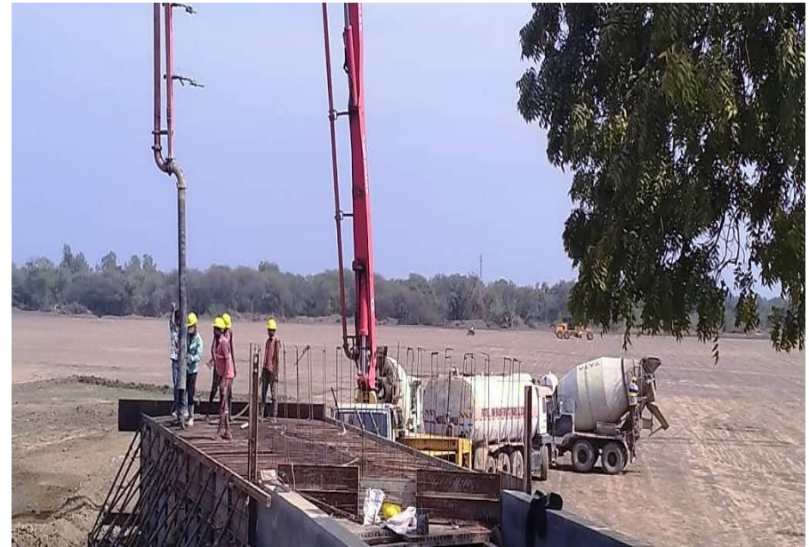
345+978 Box Culvert Service Road RHS slab Haunch Wall Concrete Pouring
