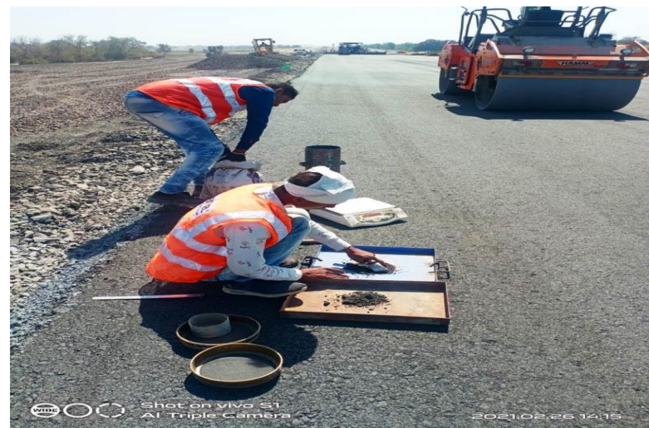
DLC Layer FDD Testing at Ch 346+960 to 347+060
