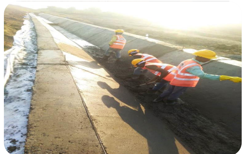
Toe Drain laying is in process @332+350 LHS
