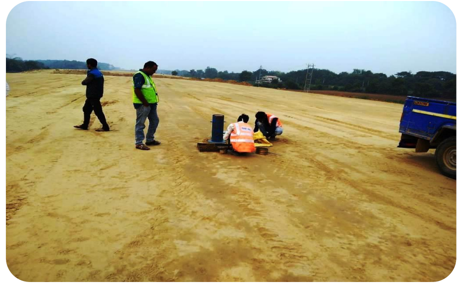
FDD CHECKING OF EMB LAYER AT CH 348+000 TO 348+130
