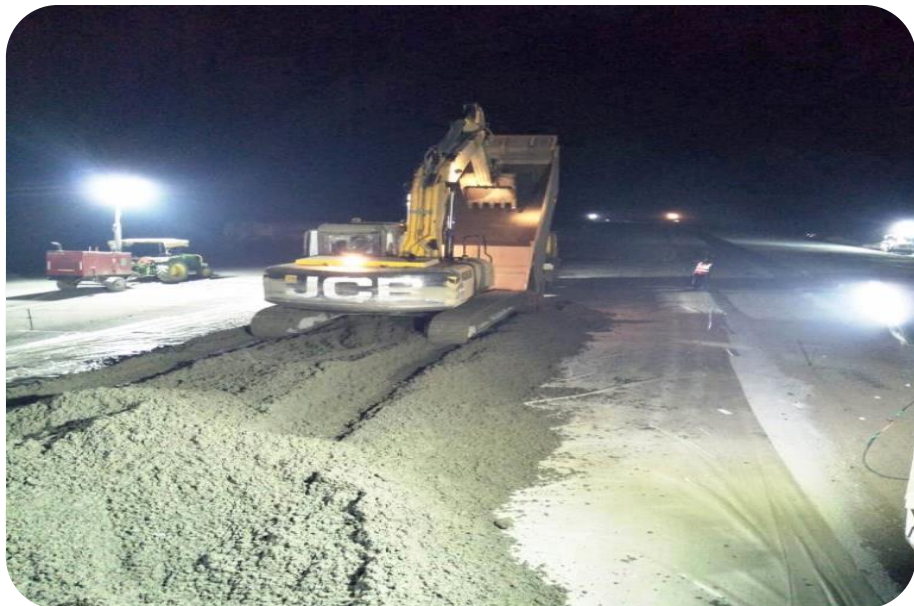
PQC LAYING 326+445 to 326+805 LHS
