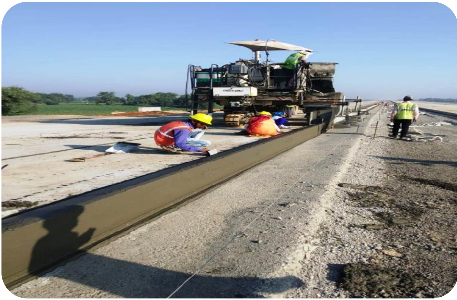
KERB LAYING WORK AT CHAINAGE 345+950 LHS
