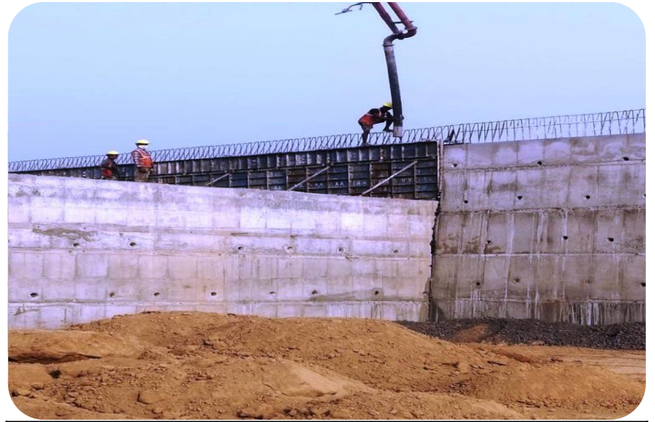
337+022 LVUP PARAPET WALL CONCRETE POURING
