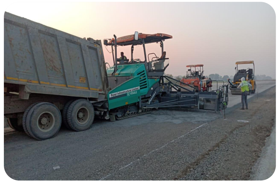
DLC LAYING AT CH 328+420 MEDIAN SIDE
