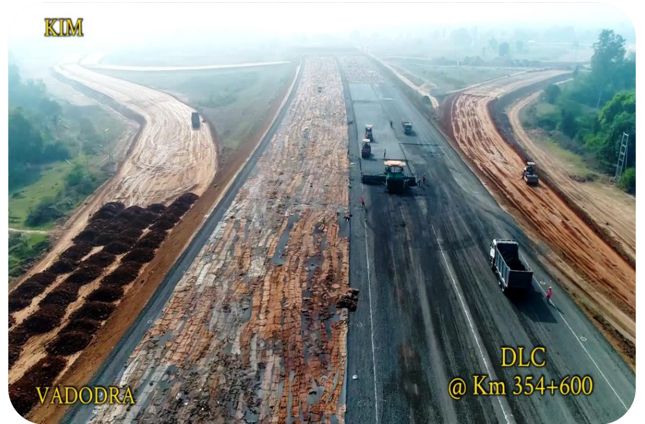
DLC WORK AT KM 354+600
