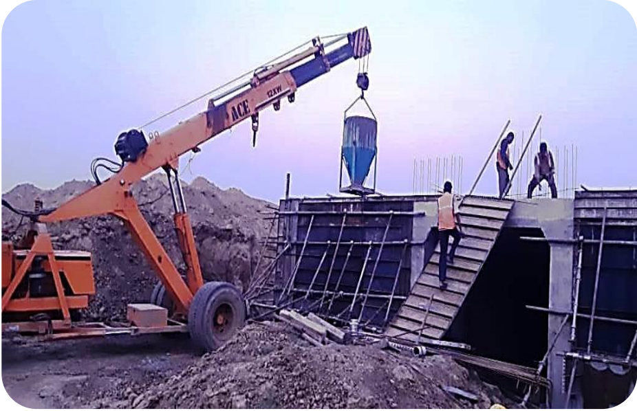
351+009 Retaining wall LHS final lift concrete Pouring.
