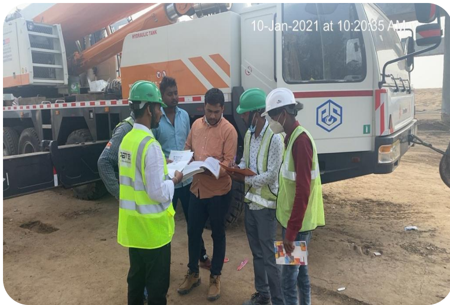
CRANE INSPECTION AT CH-353+666 LOCATION
