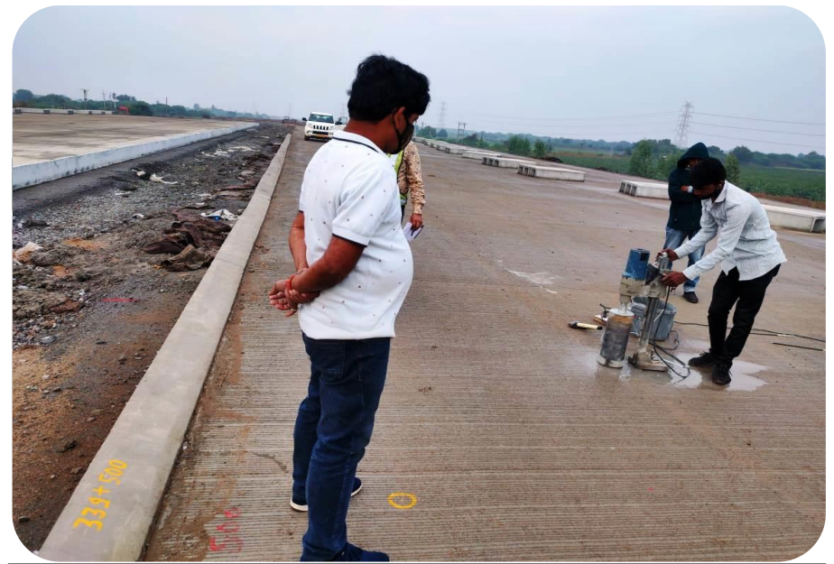
CORE CUTTING SAMPLE OF PQC AT CH 339+500
