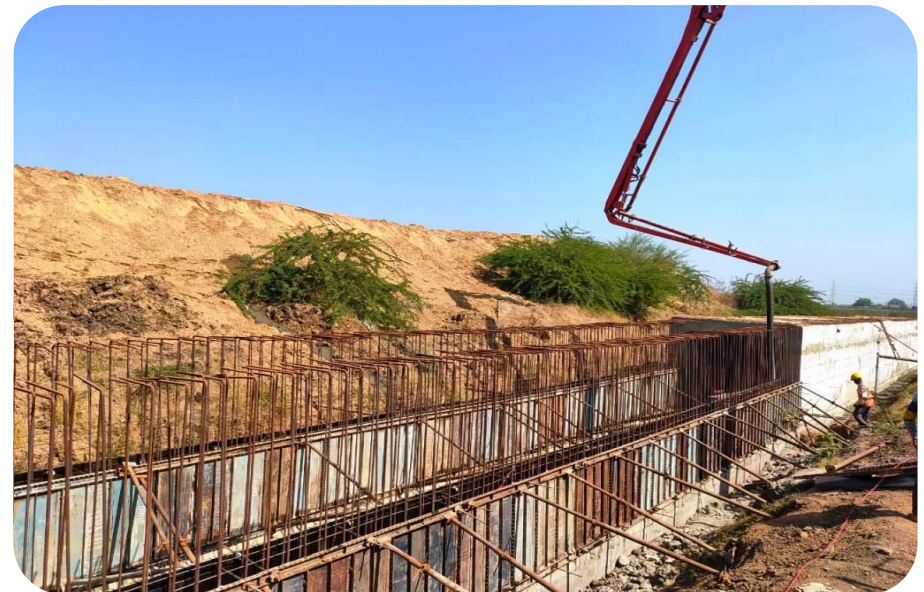
324+254 BC LHS A1 wall first lift concrete Pouring Page 85 of 87
