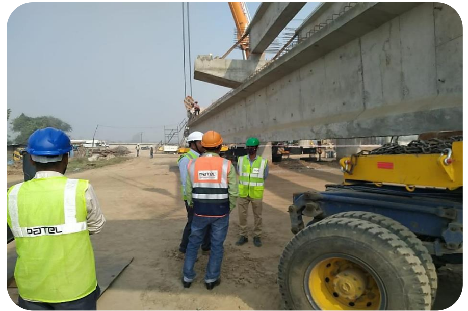
GIRDER LAUNCHING LOCATION CH 353+666
