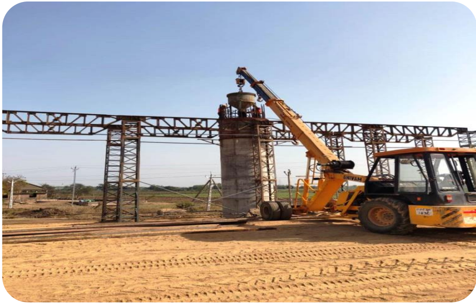
326+957 VOP A1 4th and A2 final lift concrete Pouring
