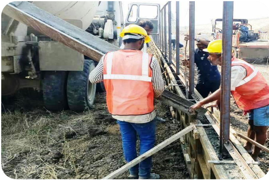
FENCING RCC WALL IS IN PROGRESS AT CH - 339 + 550 RHS
