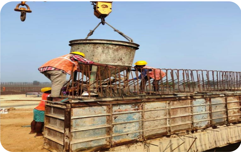
324+410 CUP LHS cushion wall concrete pouring
