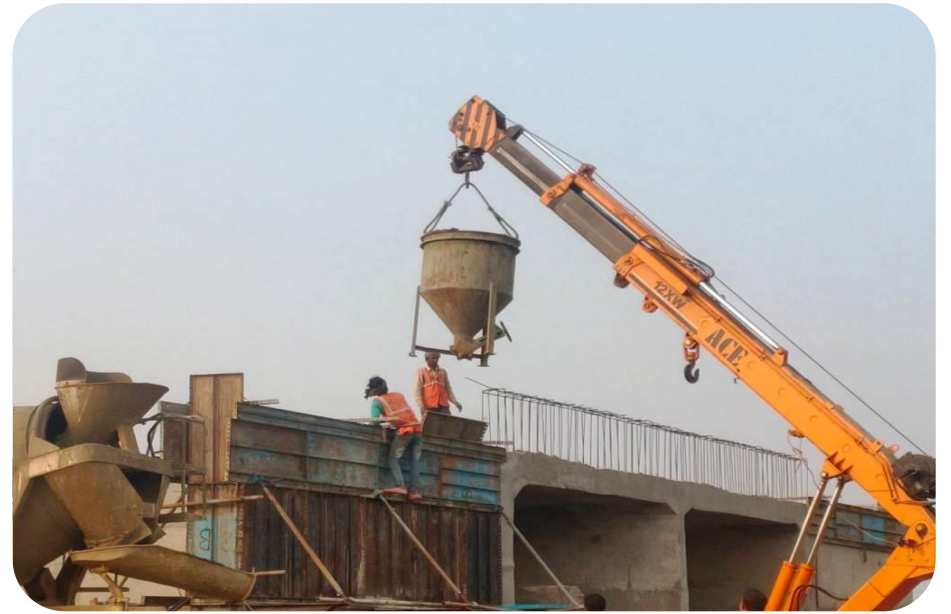
330+853 BOX CULVERT RETAINING WALL CONCRETE POURING
