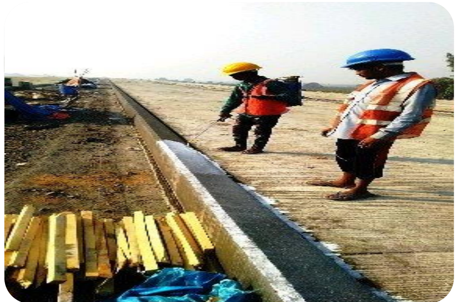
CURING COMPOUND SPRAYING ON KERB @327+890 LHS
