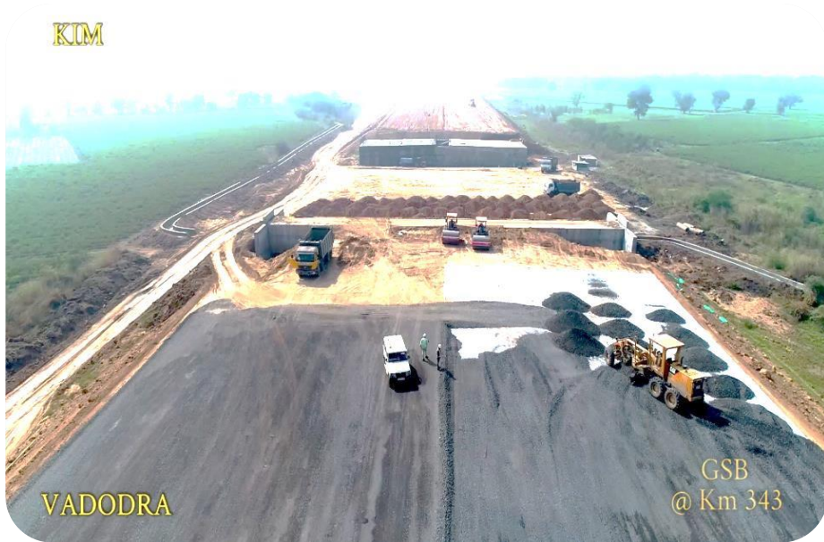
GSB WORK AT KM 343
