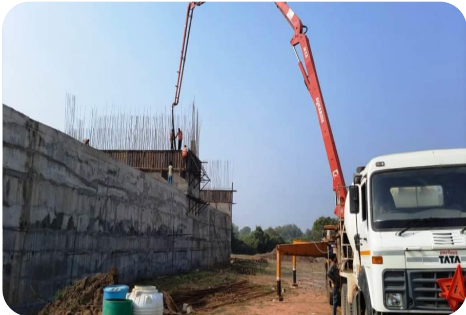
352+700 RHS side Cantilever Earth Retaining wall concrete pouring
