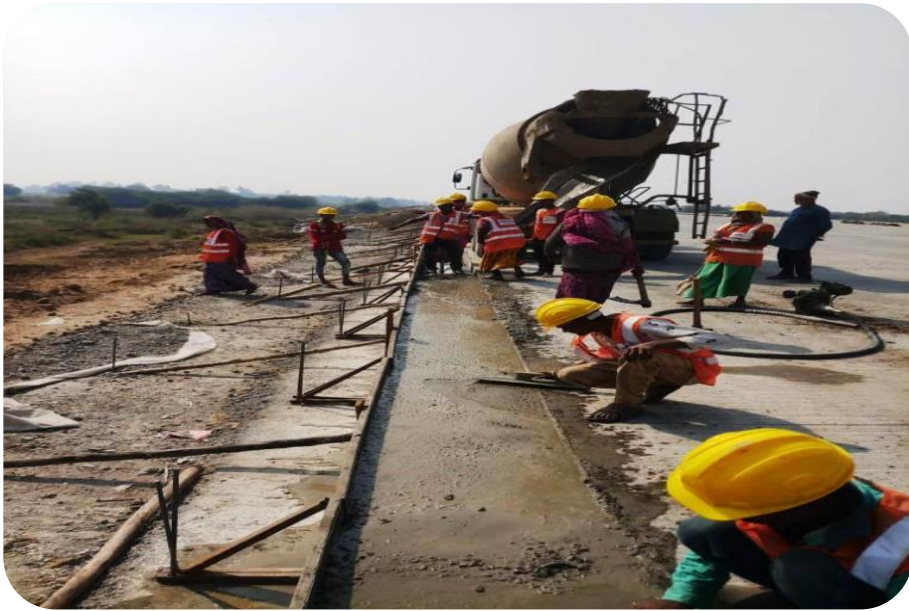
UTILITY DUCT LAYING CONCRETE WORK IS IN PROGRESS@333+580 RHS
