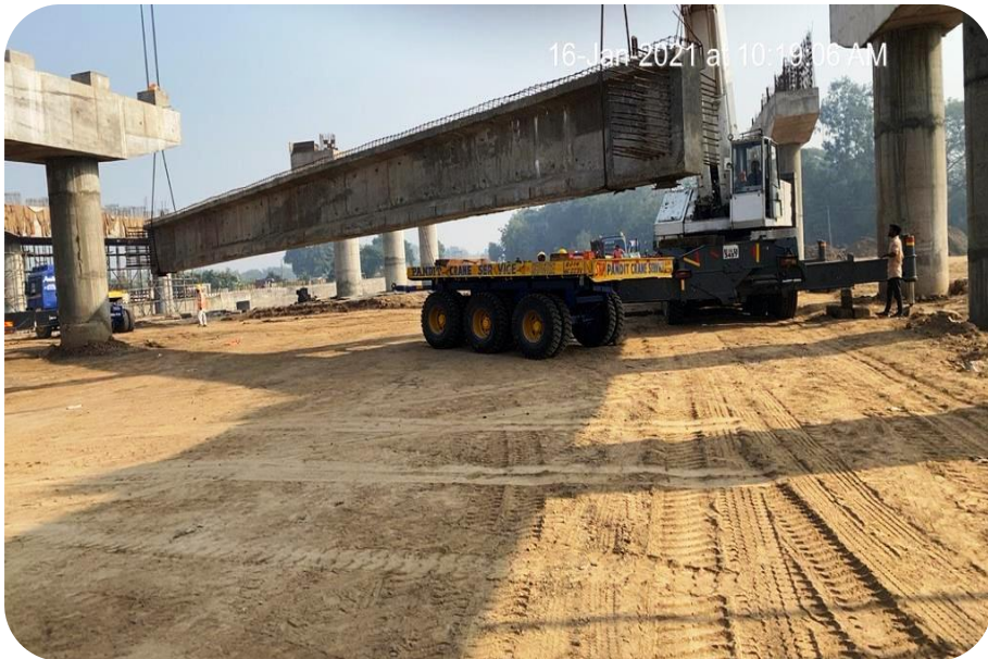
GIRDER LAUNCHING AT KM 353+666 INTERCHANGE
