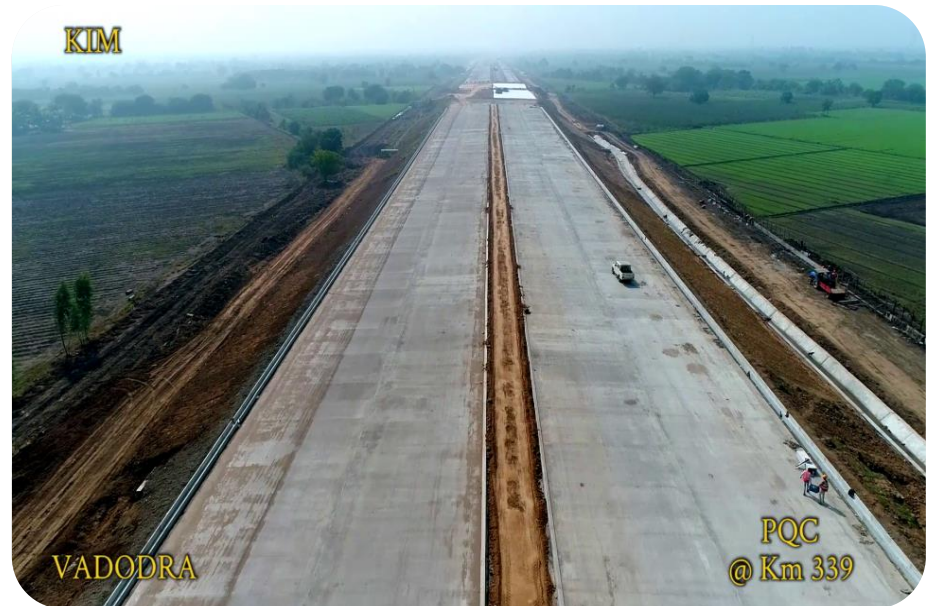
TOE DRAIN AT KM 339
