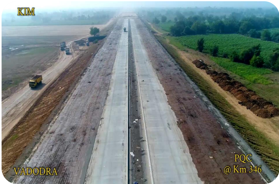
PQC AT KM 346
