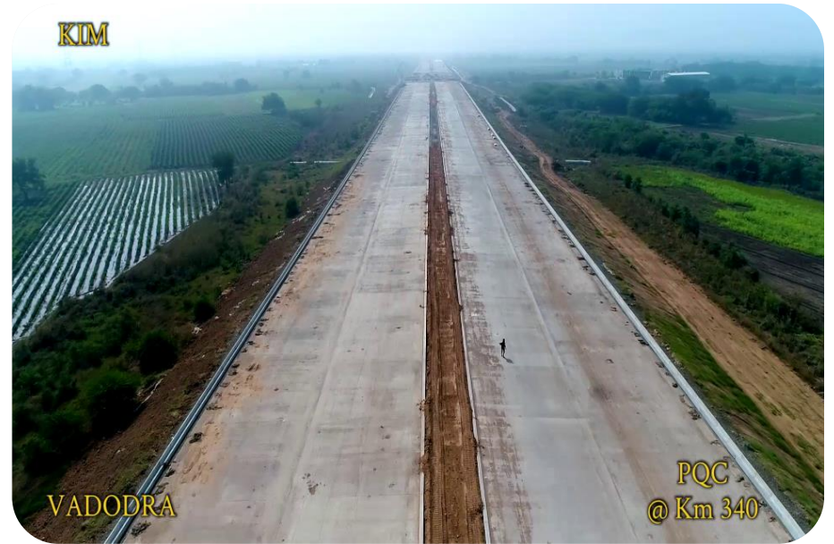
ROAD STATUS OF PQC WORK & PRECAST "U" DRAIN AT KM 340
