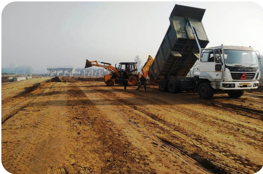
Dumping at ch 344+000 to 344+300
