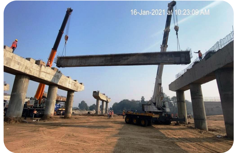
GIRDER LAUNCHING AT KM 353+666 INTERCHANGE Page 84 of 87
