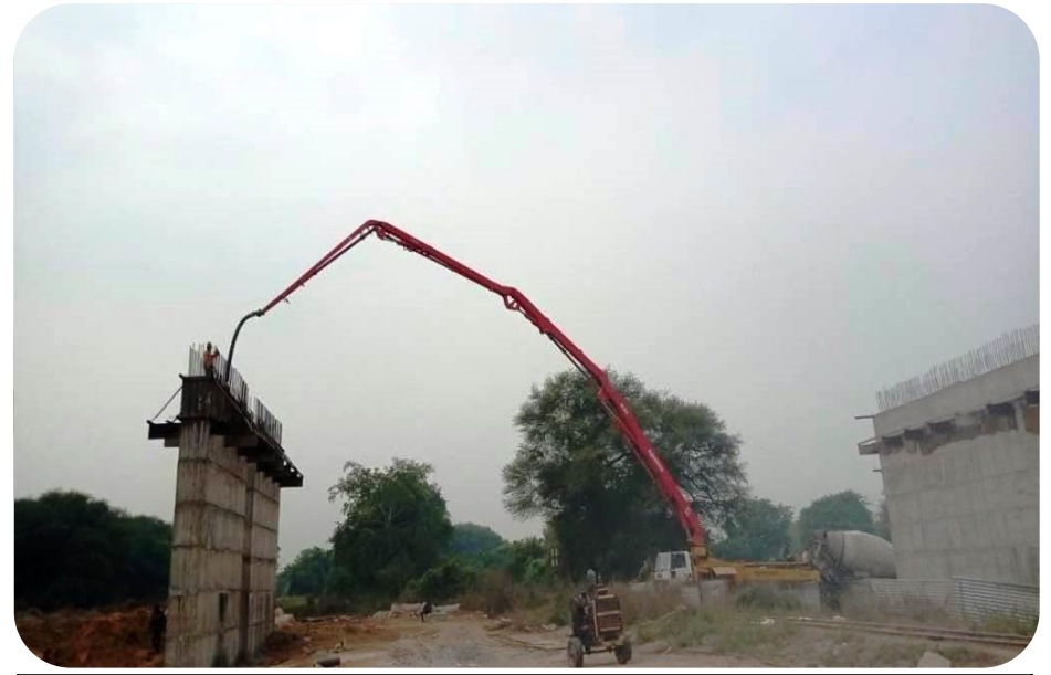
352+946 ROB PIER SHAFT CONCRETE POURING WORK
