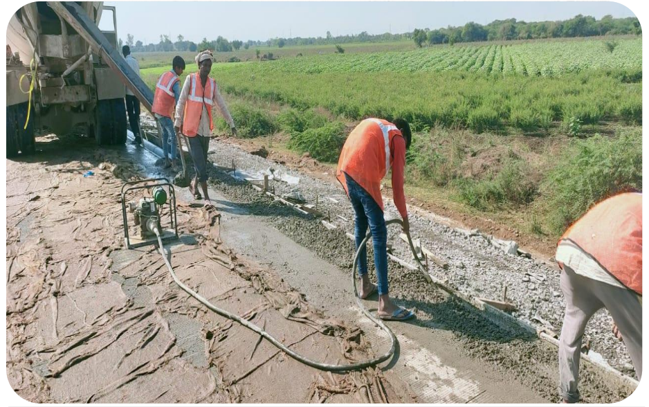
UTILITY DUCT CONCRETE WORK AT CH 334+200
