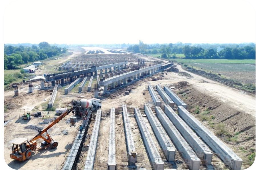
354+636 MNB GIRDER CASTING WORK
