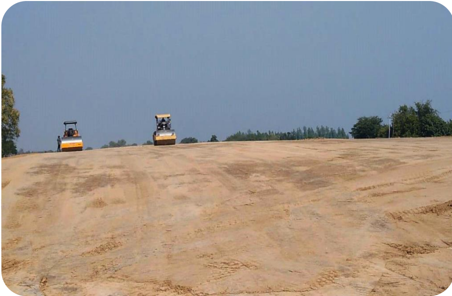
WATERING & ROLLING EMBANKMENT LAYER CH.351.860 TO 351.950
