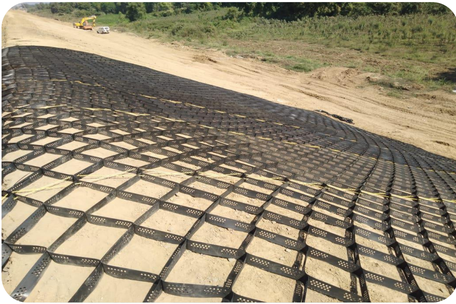
SLOPE PROTECTION WITH GEO CELL AT CH 335+500
