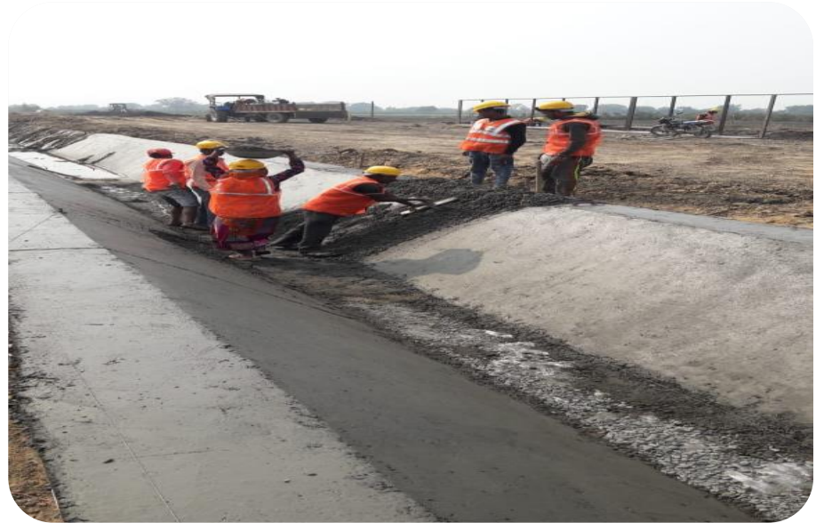
TOE DRAIN FINISHING WORK TOE DRAIN AT CH 339+300
