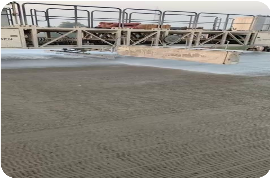
TEXTURING & CURING COMPOUND OF PQC 327+358 TO 327+500 LHS
