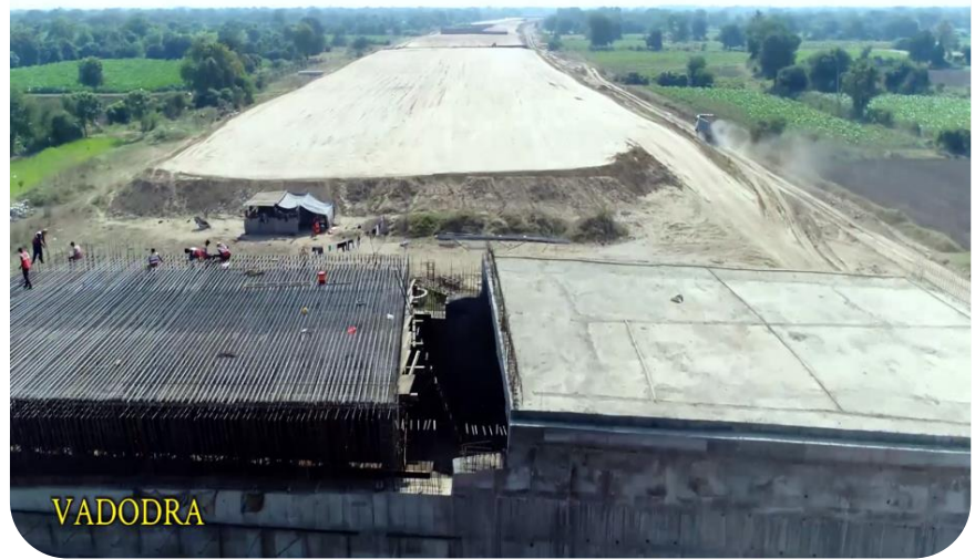
351+284 VUP SLAB REINFORCEMENT WORK
