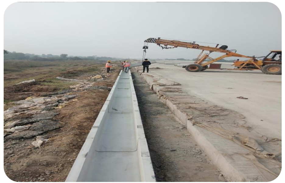
PRECAST "U" DRAIN LAYING AT CH 334+700
