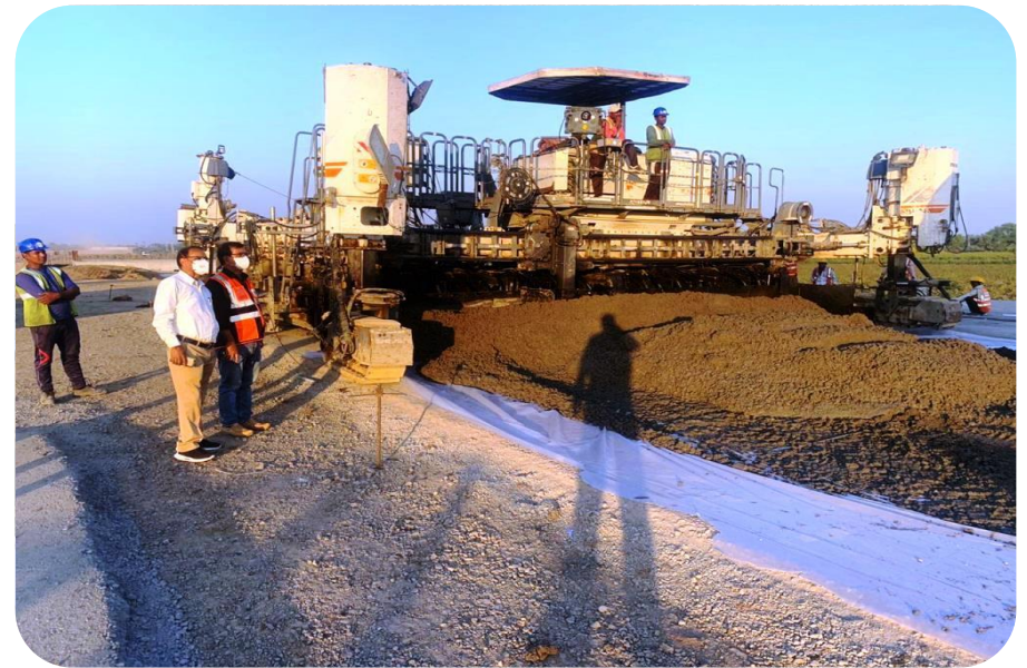
PQC LAYING CH 328+250 TO 328+770 RHS
