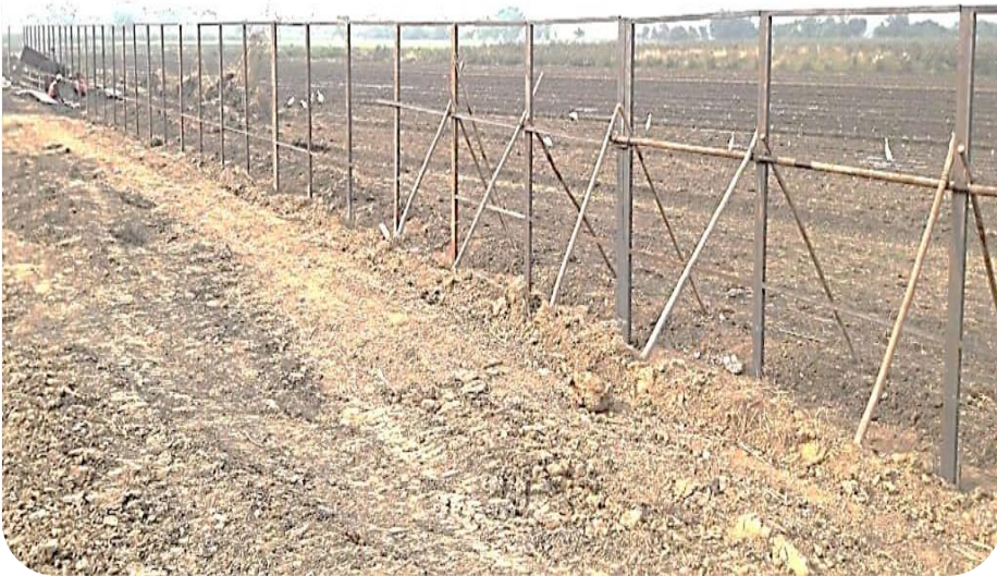
CHAIN LINK FENCING WORK AT CH 339+300
