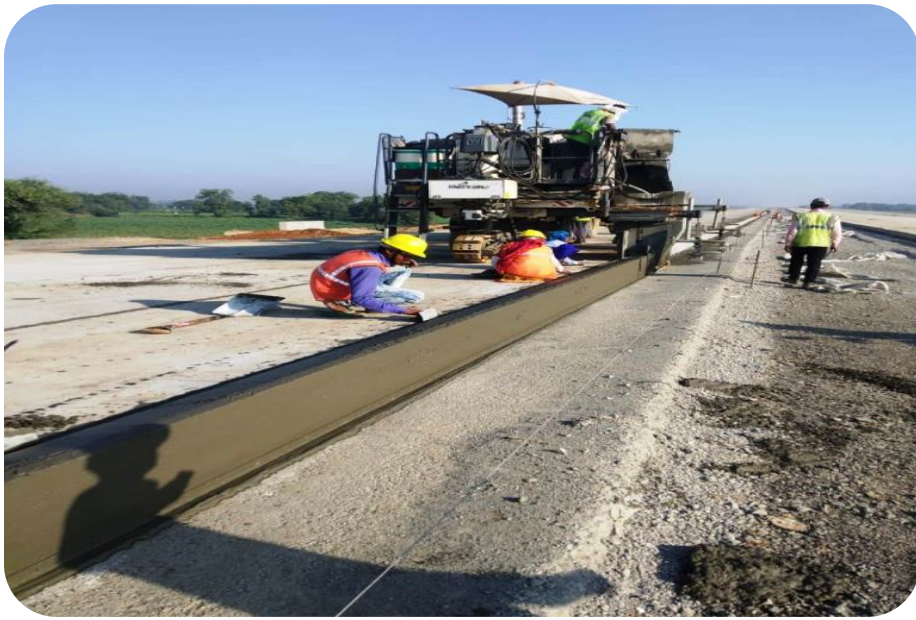
KERB LAYING WORK AT CHAINAGE 345+950 LHS
