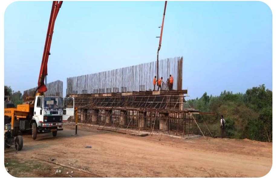
350+143 MNB ABUTMENT CAP CONCRETE POURING WORK
