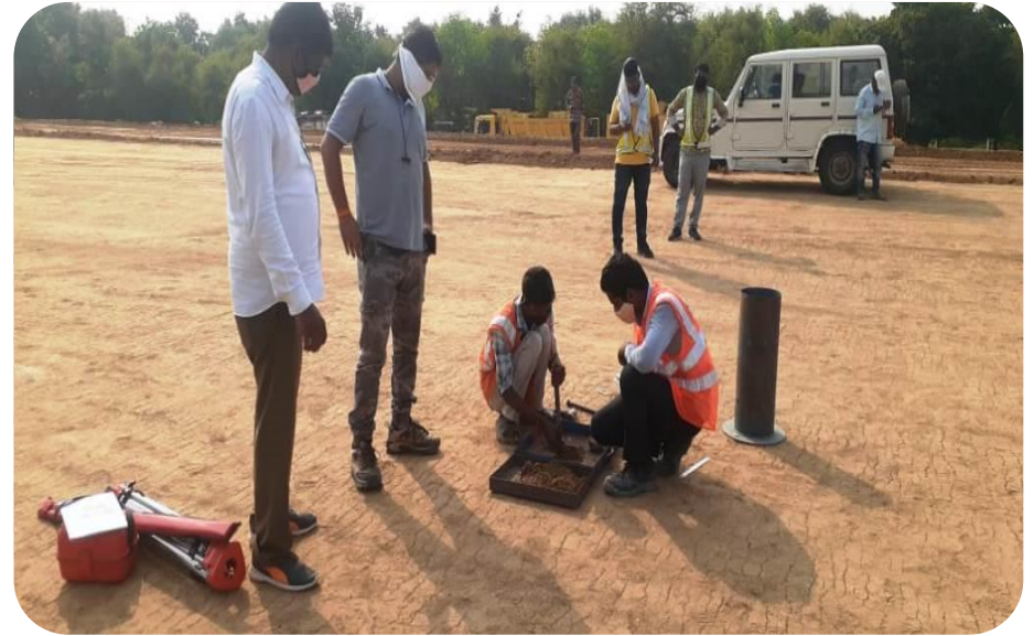
FDD Testing of SG TOP 349+260 to 349+380
