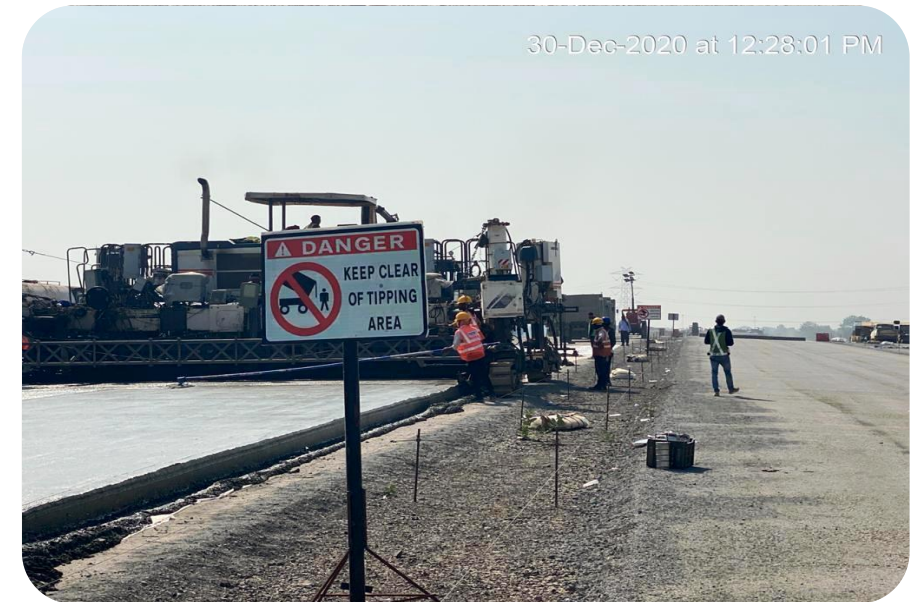
PQC LAYING 337+110 to 337+342 RHS
