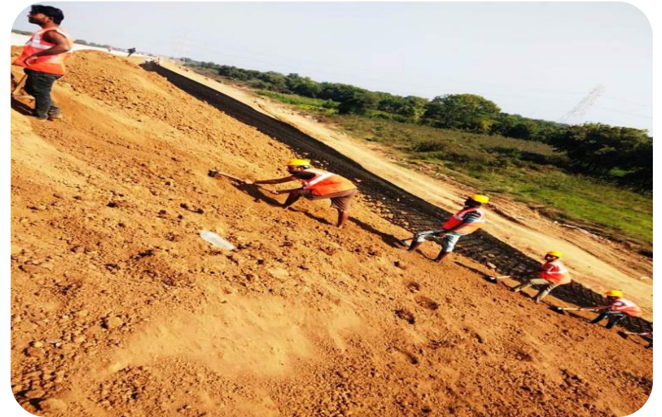
SOIL FILL IN PROGRESS ON GEO CELL AT CH 335+560 RHS
