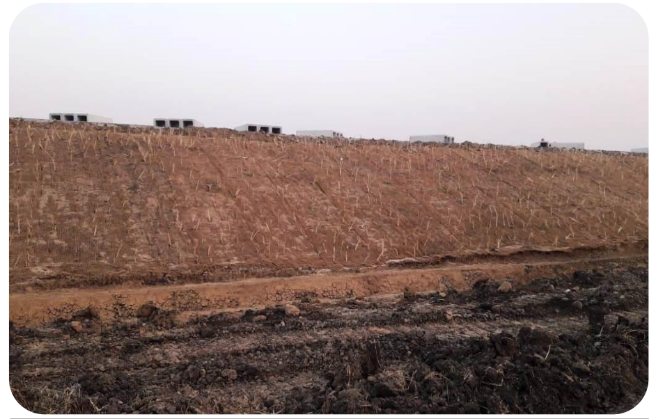
SLOPE PROTECTION WITH COIR MATE WORK AT CH 339+300
