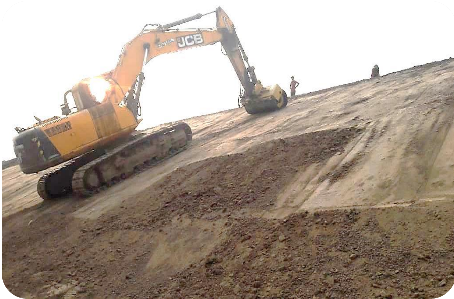
SLOPE ROLLING AT CH 335+600
