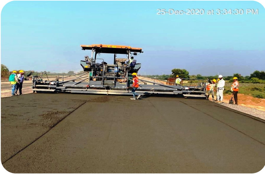
DLC LAYING AT CH 336+300
