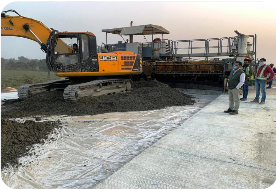
PQC LAYING AT CH 345 RHS
