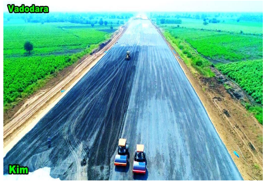
328+500 GSB Rolling in Progress
