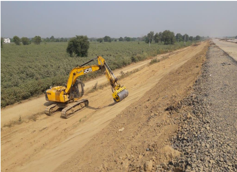
Slope Rolling work 332+400 LHS
