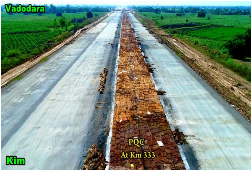
Curing of PQC with sprinkler at 333
