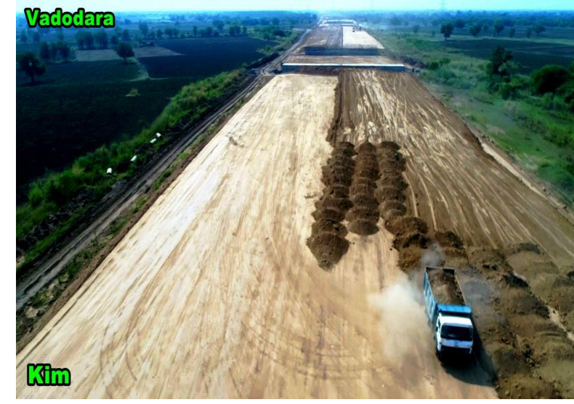
Km 343 subgrade in progress
