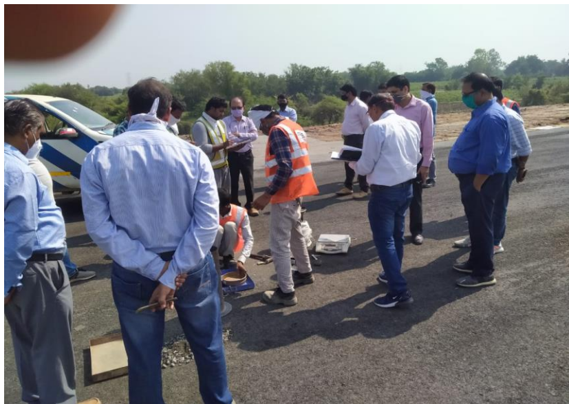
FDD Checking at ch 334+275 to 334+350 RHS
