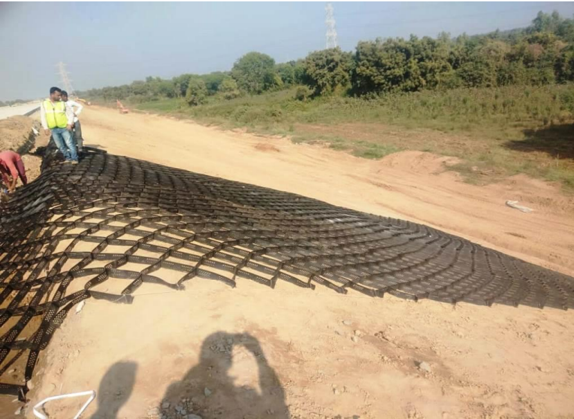
Geo cell laying in progress 335+500 RHS
