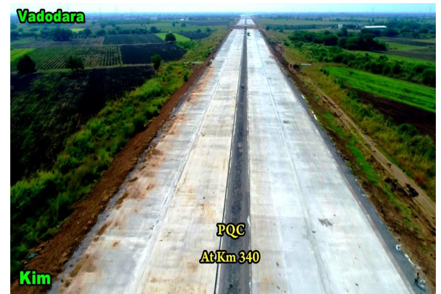
PQC work at Km 340
