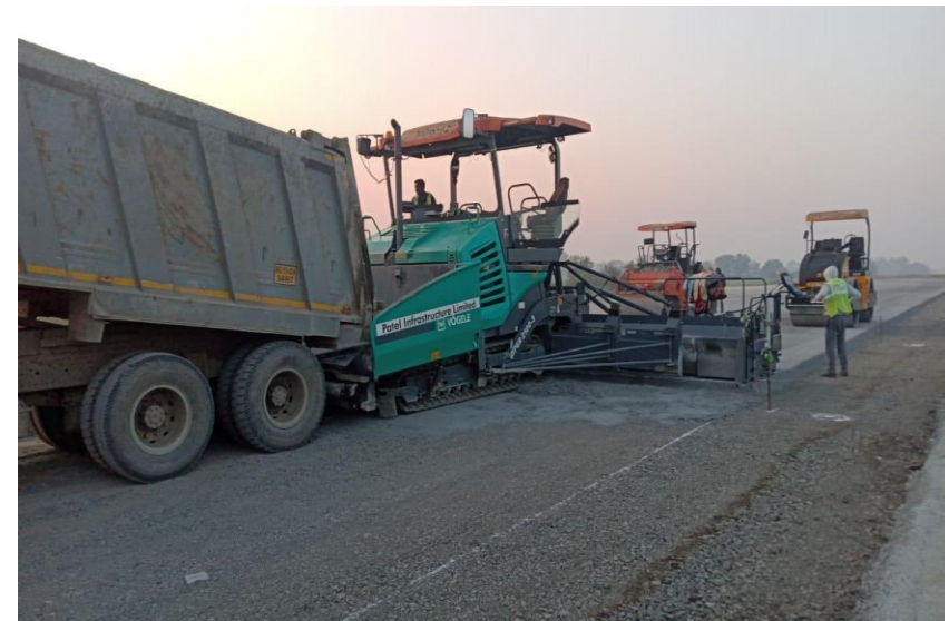
DLC Laying work is in Progress at ch 328+420 Median Side
