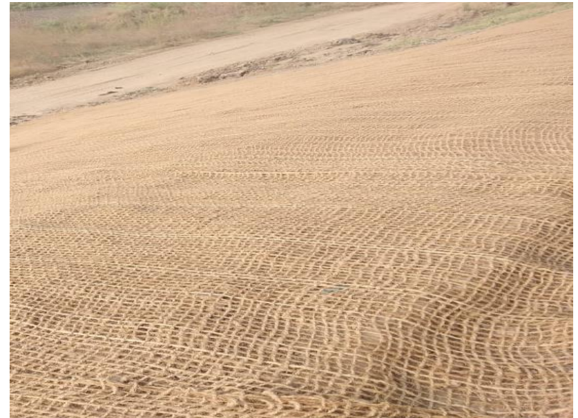
Slope Coir mate work at ch 339+400 LHS
