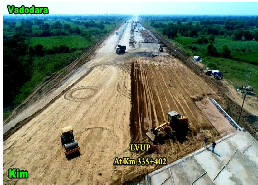
335+402 LVUP Approaches RE Wall in progress
