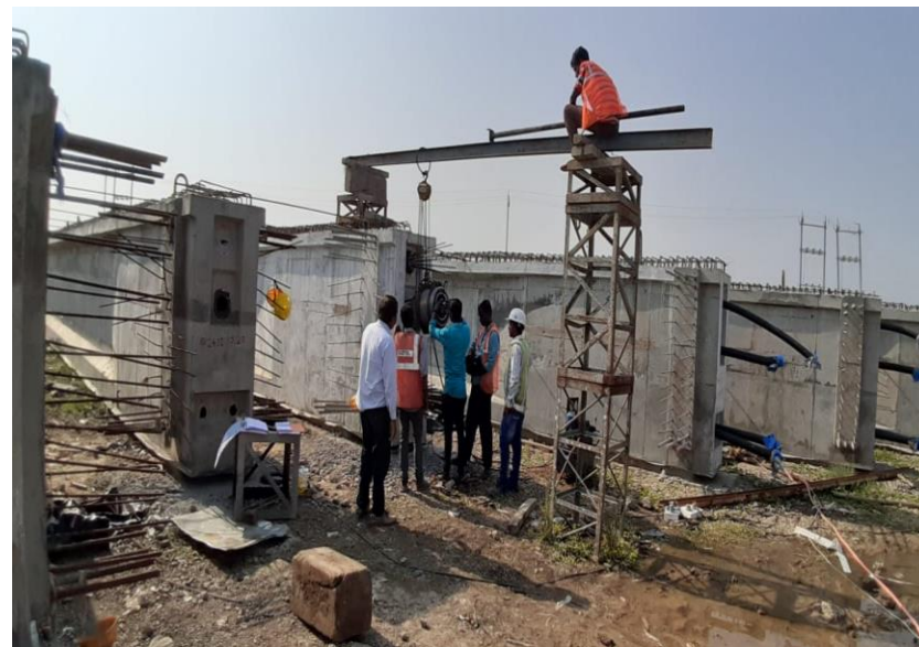
330+640 MNB PSC Girder stressing work in progress
