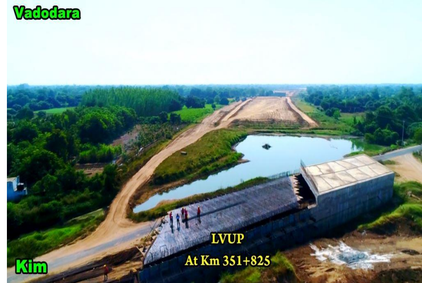
351+825 LVUP RHS slab in progress
