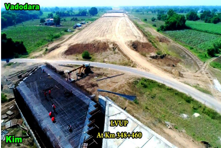
348+460 LVUP RHS Slab in progress
