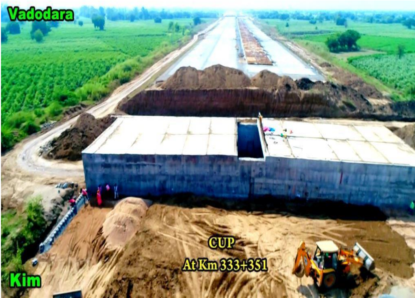
333+351 CUP RE Wall in progress
