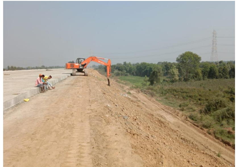
Slope dressing at ch 335+500 to 335+600 RHS
