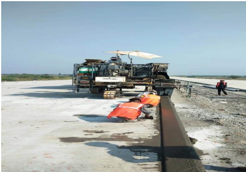
Kerb laying in progress at ch 339+840
