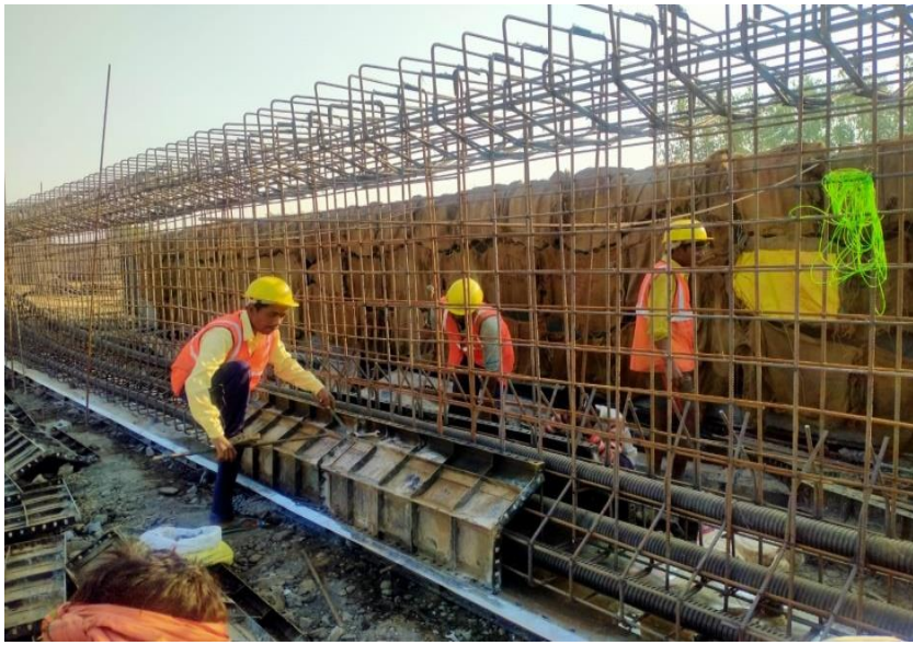
343+566 MNB PSC Girder Profile & Shuttering work
