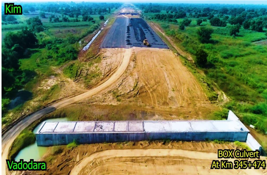
345+474 Box Culvert Slab Completed
