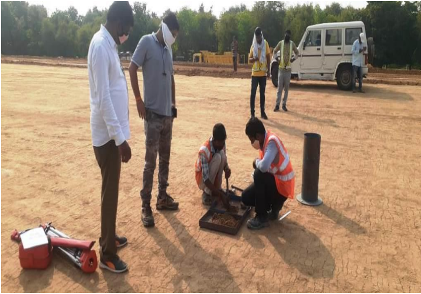
349+260 to 349+380 FDD Testing of SG TOP
