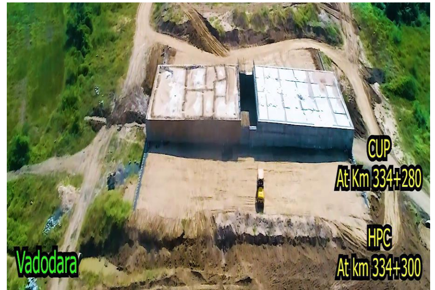
334+280 RS wall in Progress
