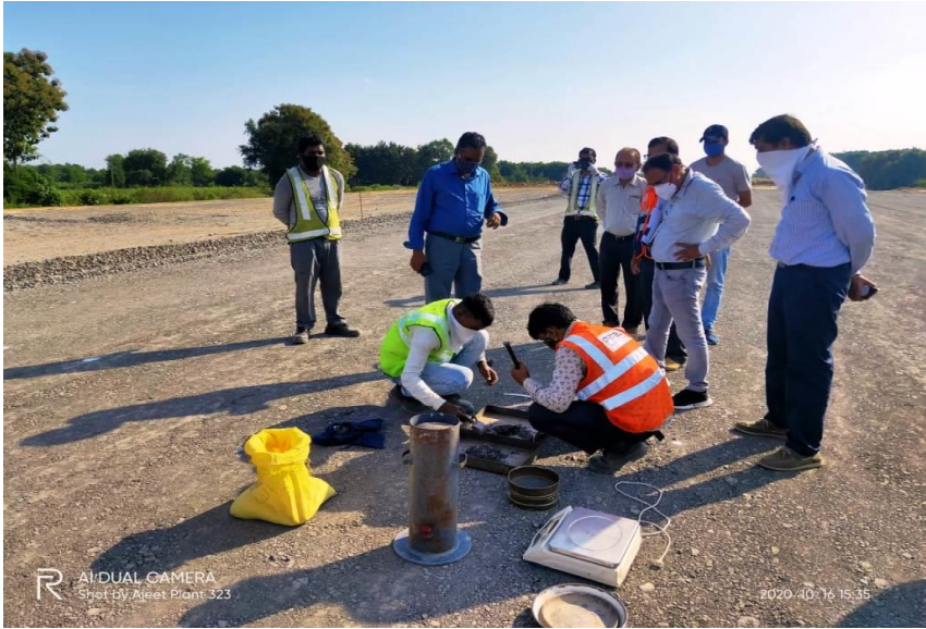
349+300 FDD Testing of GSB Bed
