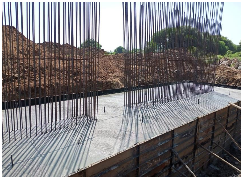
352+946 ROB Pile cap concrete Pouring completed
