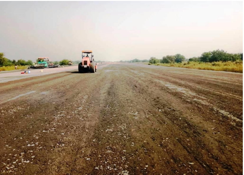
GSB TOP IN PROGRESS 345+160 TO 345+380 RHS
