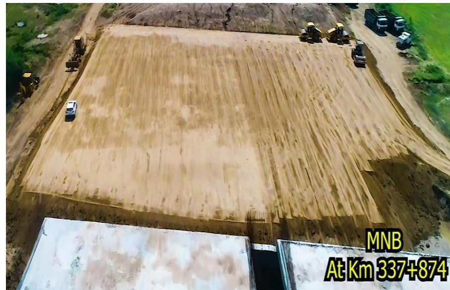
337+874 Embankment work in progress
