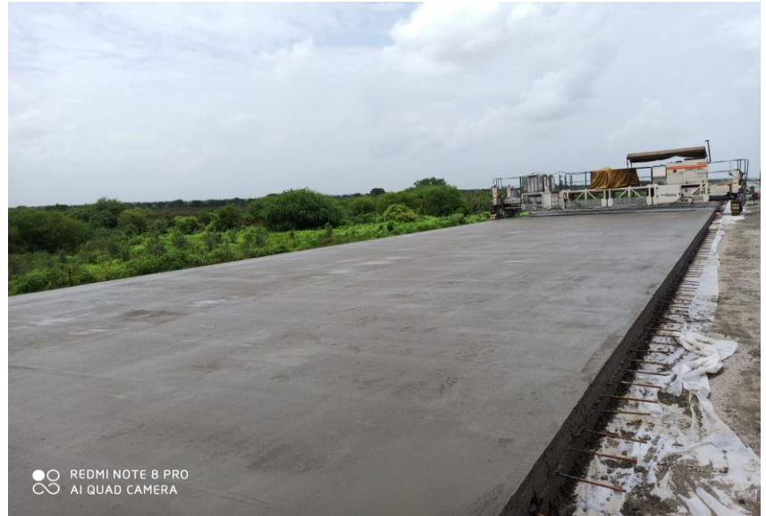
PQC Laying at Ch. 339+770 TO 339+924 LHS Side
