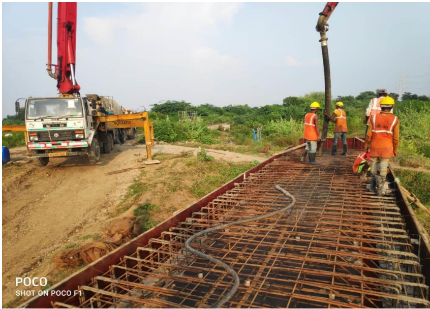
324+164 Box Culvert slab concrete Pouring
