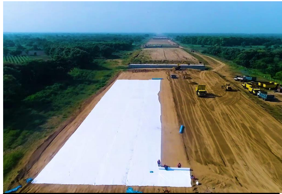
349+200 Geo Textile Laying
