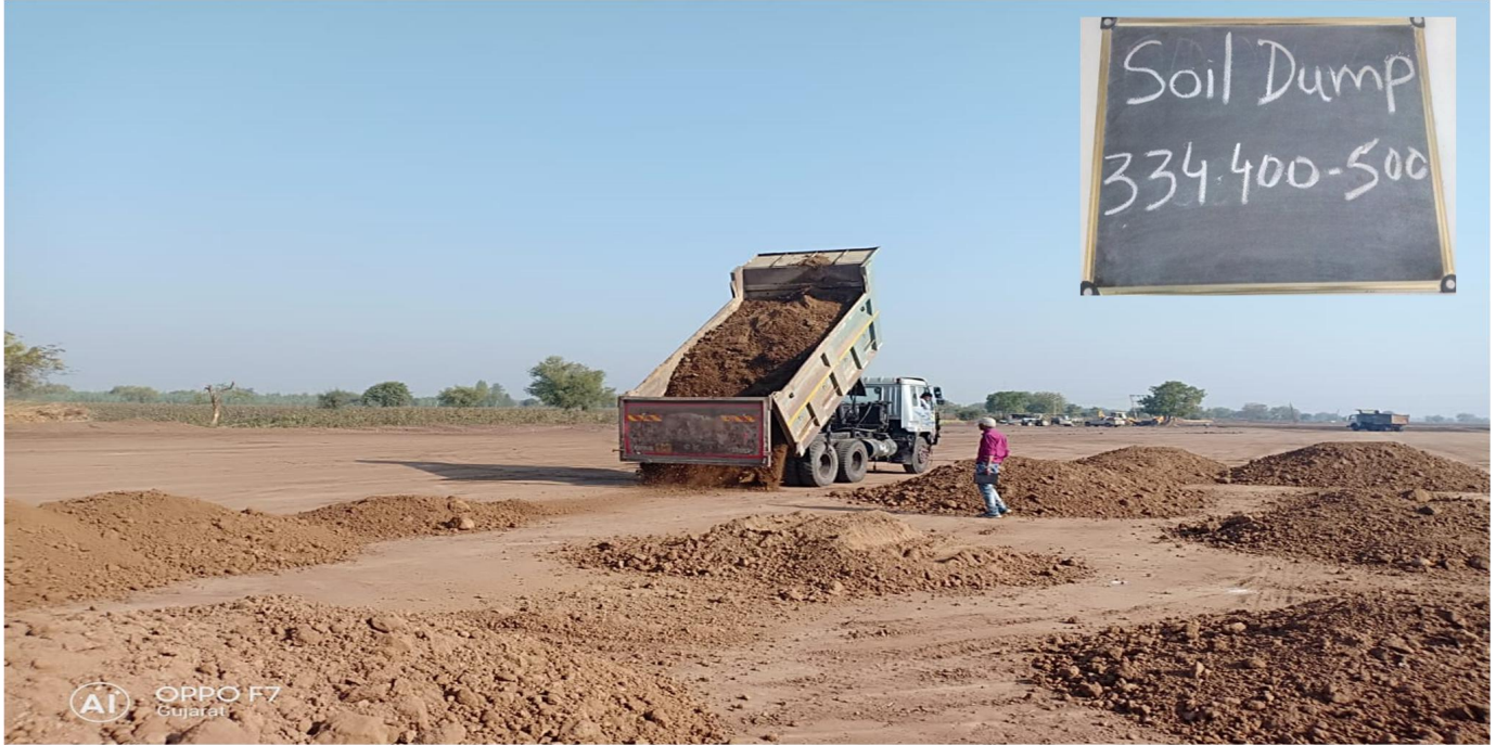
334+400 to 334+500 SOIL DUMPING FOR EMB.
