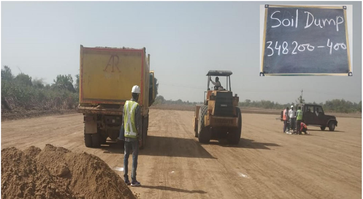
348+200 to 348+400 SOIL DUMPING FOR EMB.
