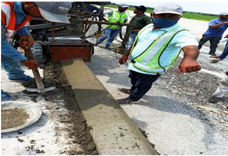
339+420 Kerb laying work RHS
