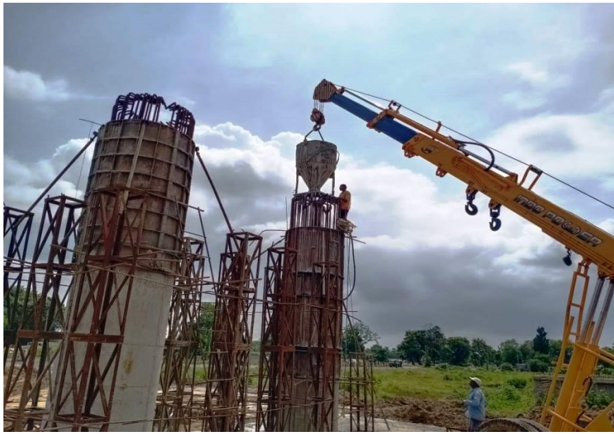
353+666 Pier shaft Concrete Pouring work Interchange
