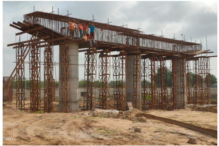
353+666 INTERCHANGE PIER CAP STEEL BINDING WORK
