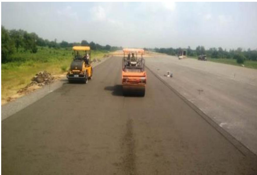
332+190 to 332+390 DLC Rolling work LHS
