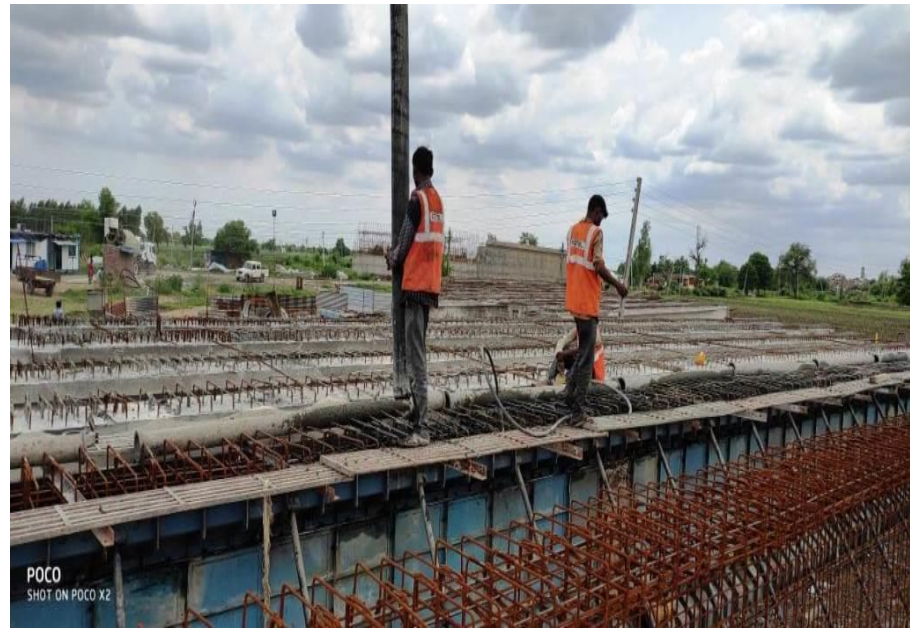
329+344 GIRDER CASTING PROGRESS LVUP
