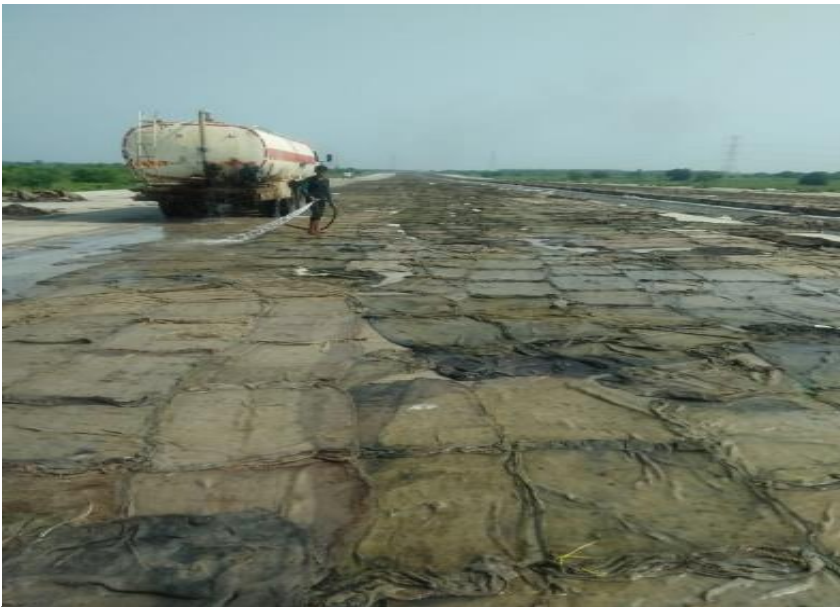
339+800 PQC Curing LHS
