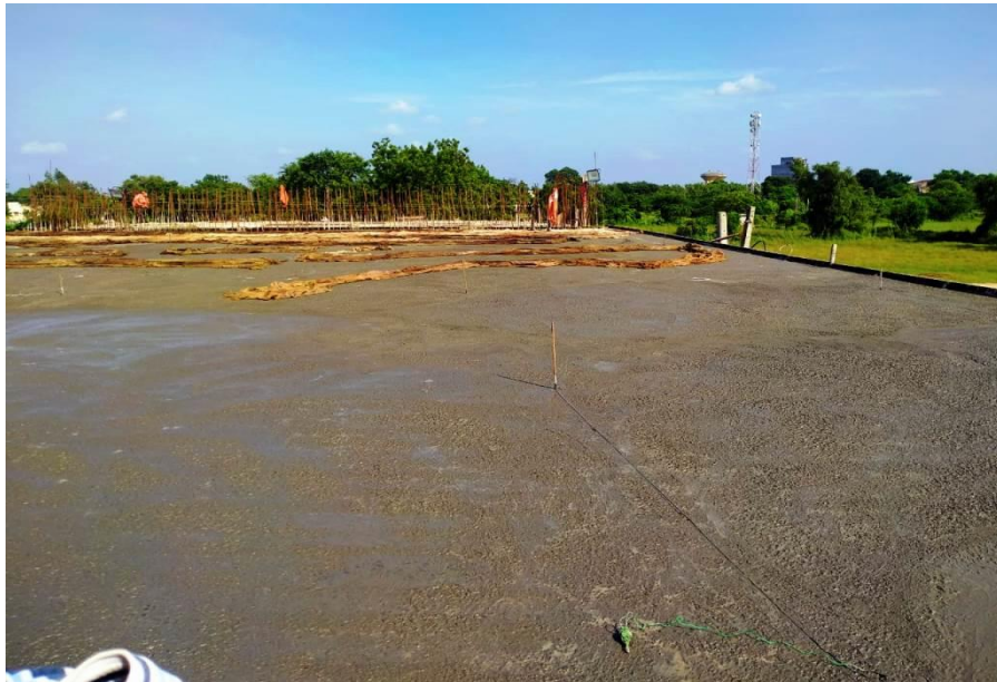
343+856 LHS Slab Casting Completed LVUP
