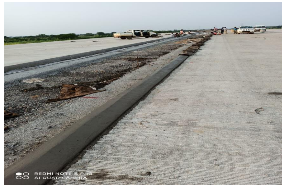
339+420(RHS) Kerb laying work Kerb
