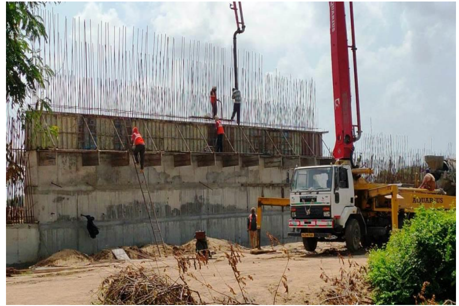
RETAINING WALL 353+440 LIFT CONCRETE POURING IN PROGRESS
