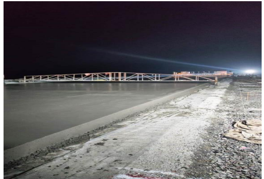
339+775 TO 340+020 PQC Laying work RHS
