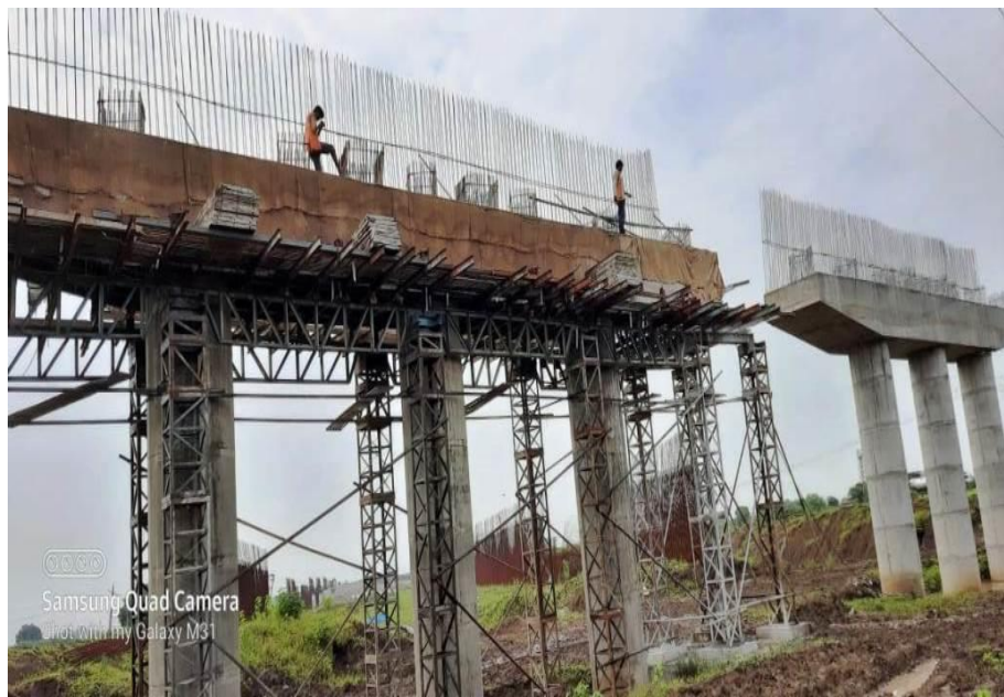
323+074 Pier cap curing work Interchange
