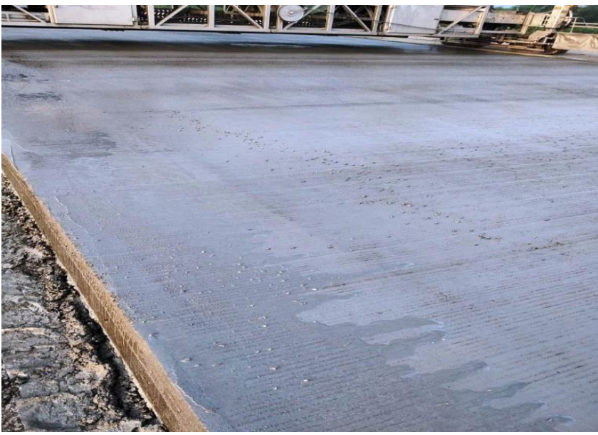
339+942 to 340+320 Texturing & curing at PQC LHS
