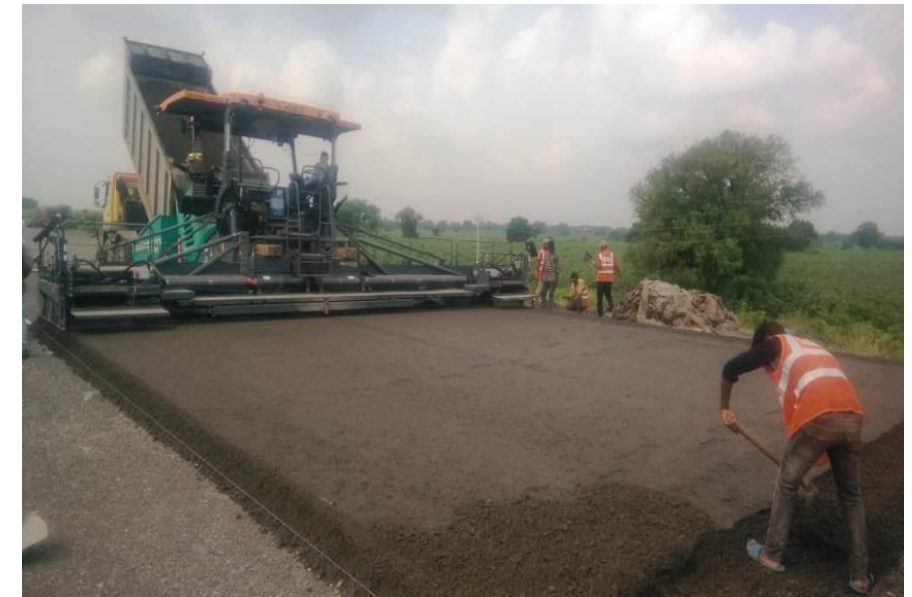
332+190 to 332+390 DLC Laying Work LHS
