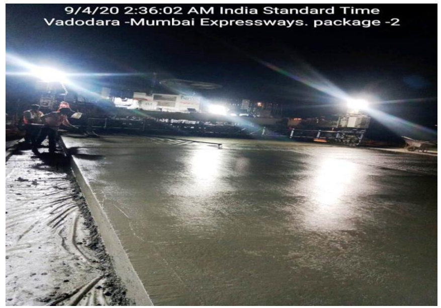
339+775 TO 340+020 PQC Laying work RHS
