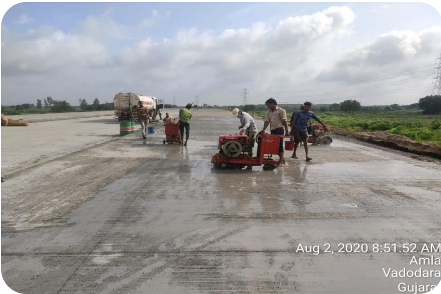
340+100 Initial Cutting work of PQC RHS
