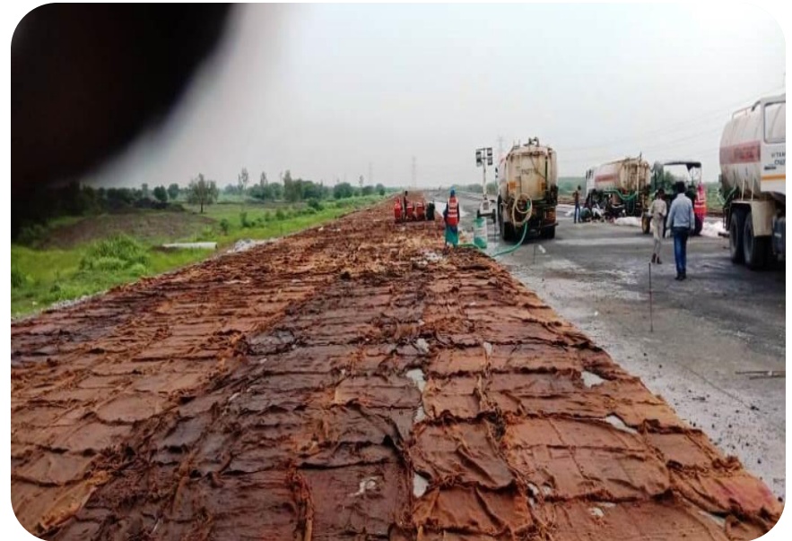
340+000 CURING WORK OF PQC LHS
