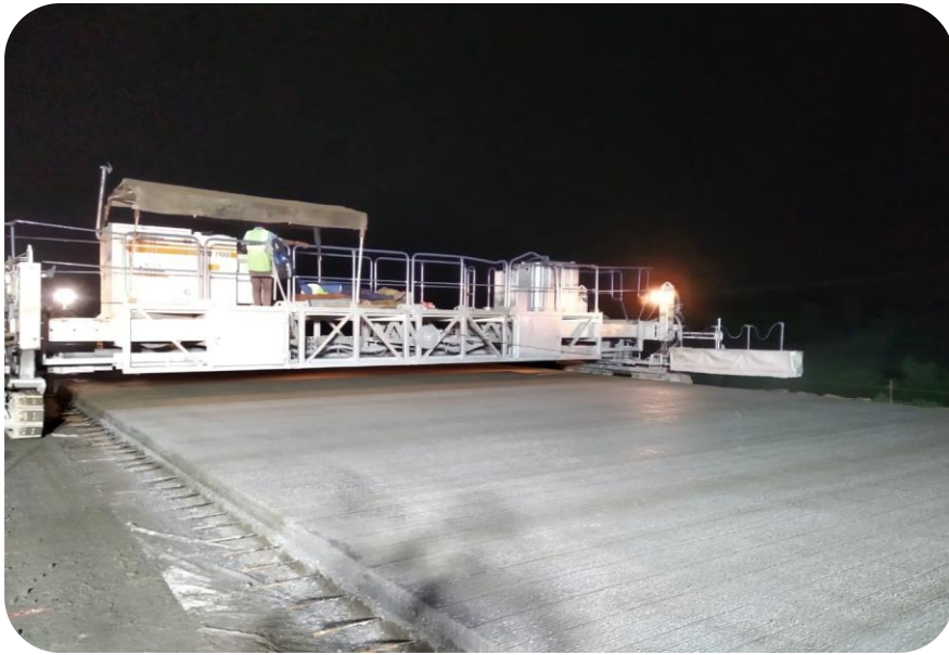
340+300 PQC Laying Completed LHS
