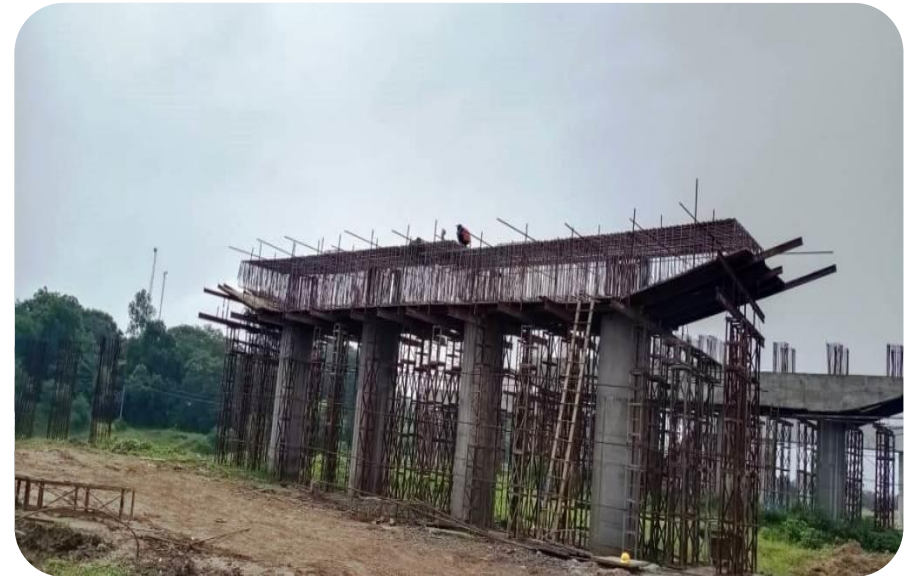
353+666 Pier Cap Interchange
