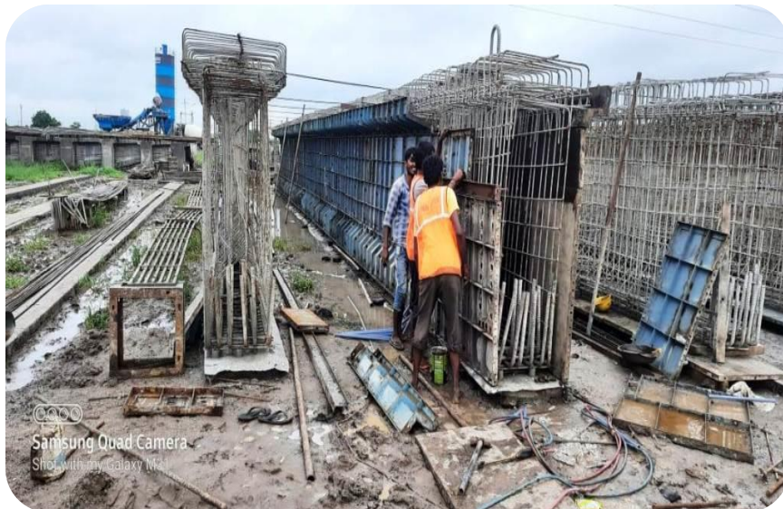
323+074 RCC Girder Shuttering work Interchange
