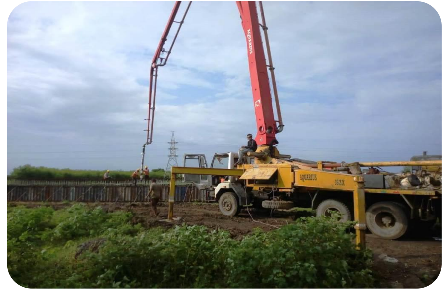
331+840 RHS wall concrete pouring work Box Culvert
