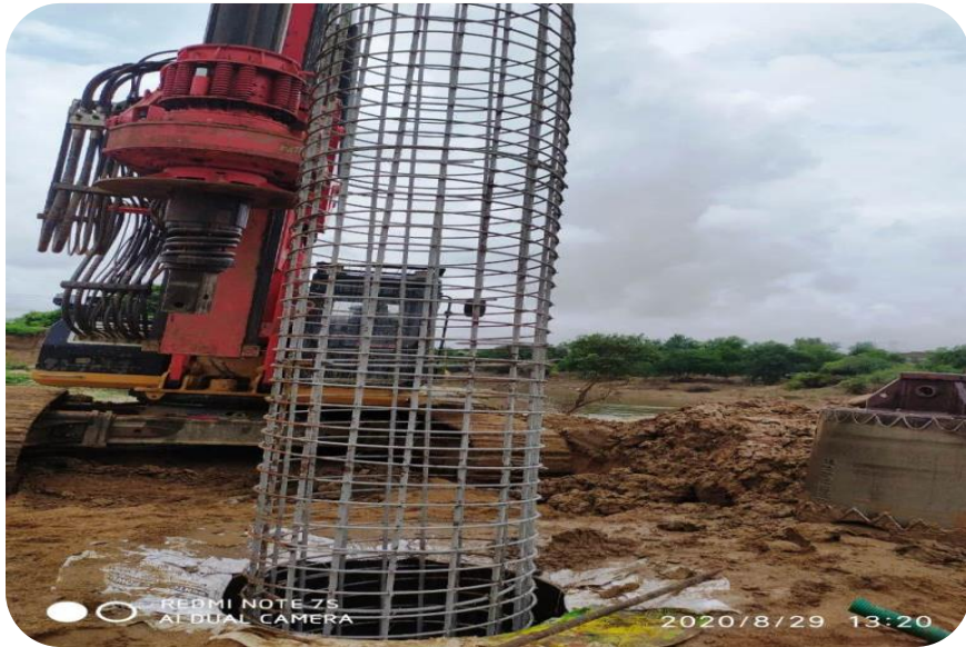
336+810 Bottom cage Lowering MJB
