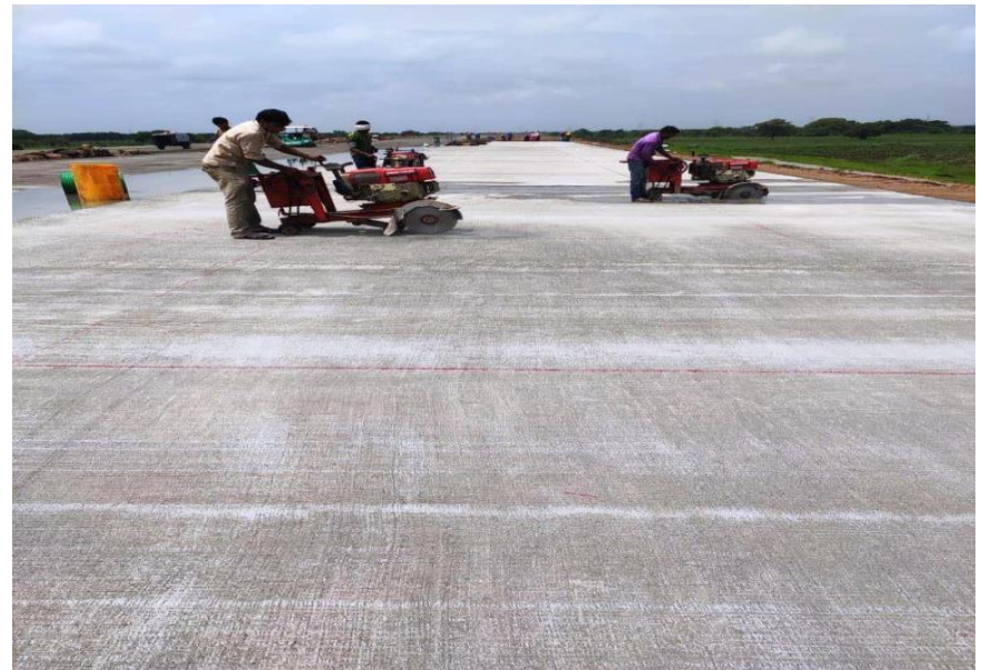
339+000 INITIAL CUTTING WORK OF PQC
