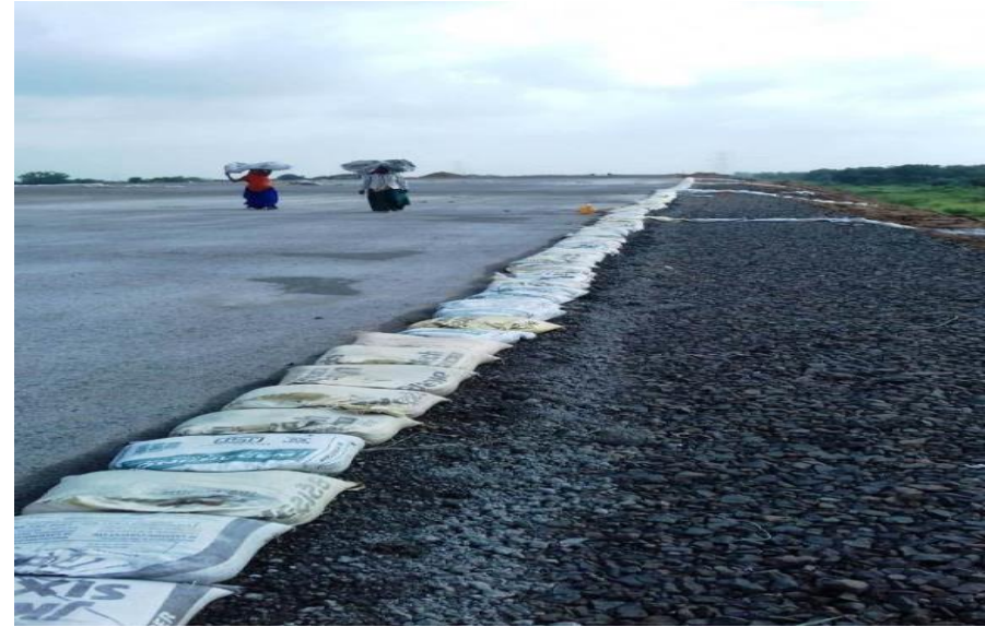
335+040 TEMPORARY DRAIN WORKS WITH SOIL BAG RHS
