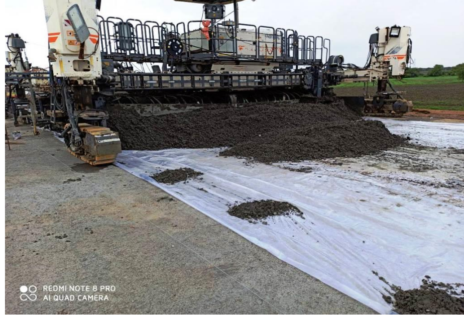
339+090 TO 339+220 PQC LAYING IN PROGRESS LHS
