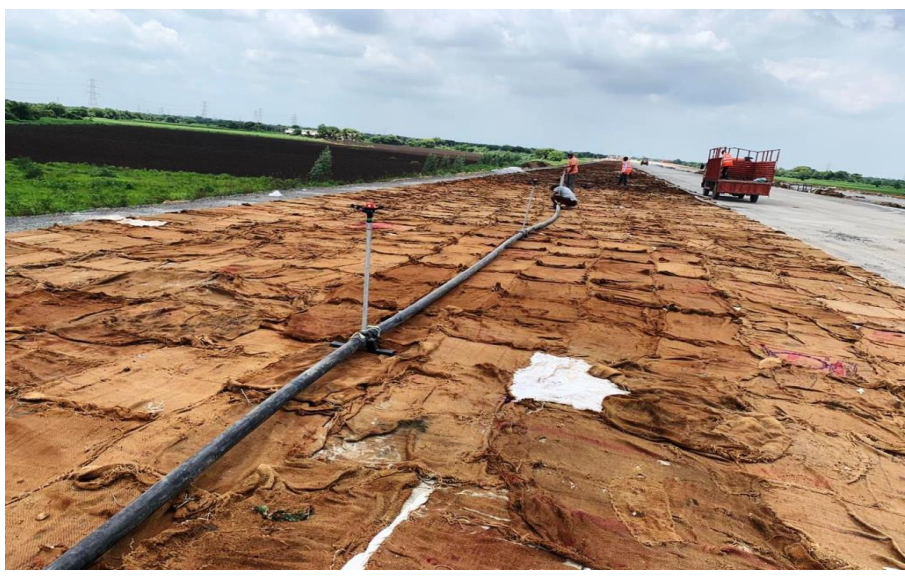
339 PVC PIPE SPRINKLER INSTALLED AT PQC SITE FOR CURING
