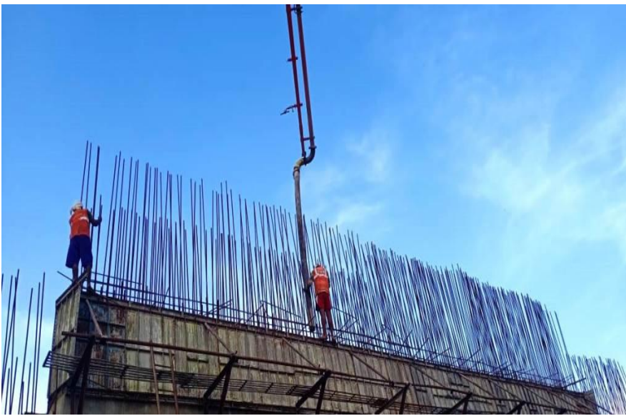
353+340 TO 353+360 WALL CONCRETE POURING RETAINING WALL
