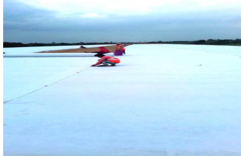
329+440 TO 329+680 GEO TEXTILE LAYING WORK
