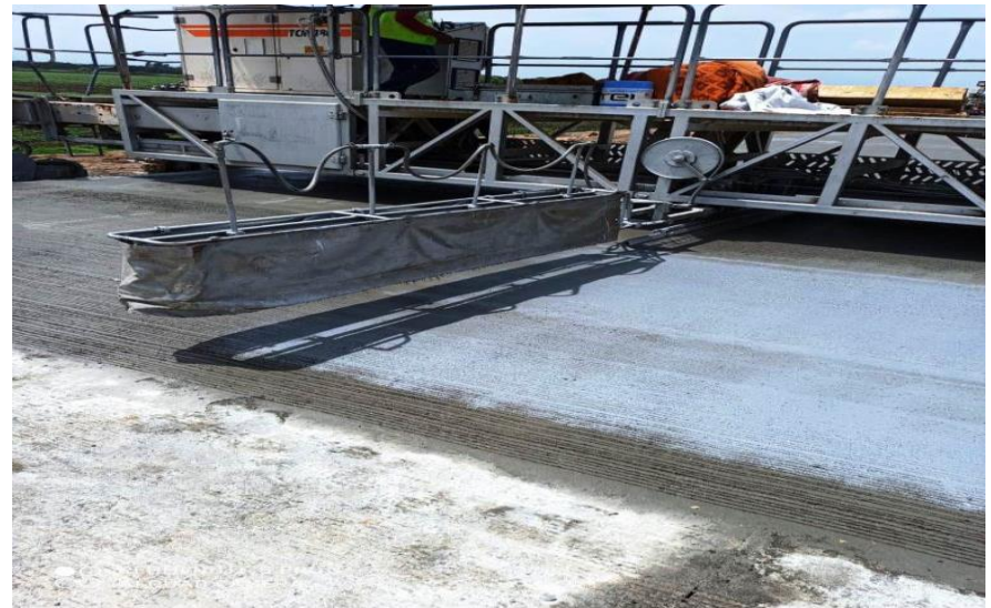
339+090 TO 339+220 CURING COMPOUND APPLIED LHS
