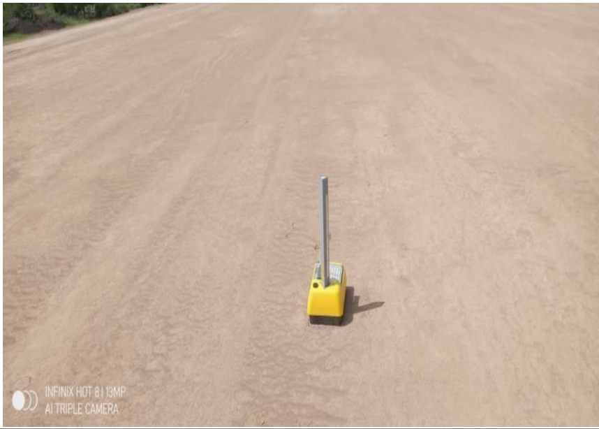
FDD CHECKING OF EMBANKMENT TOP AT CH 329+550 TO 680 BHS
