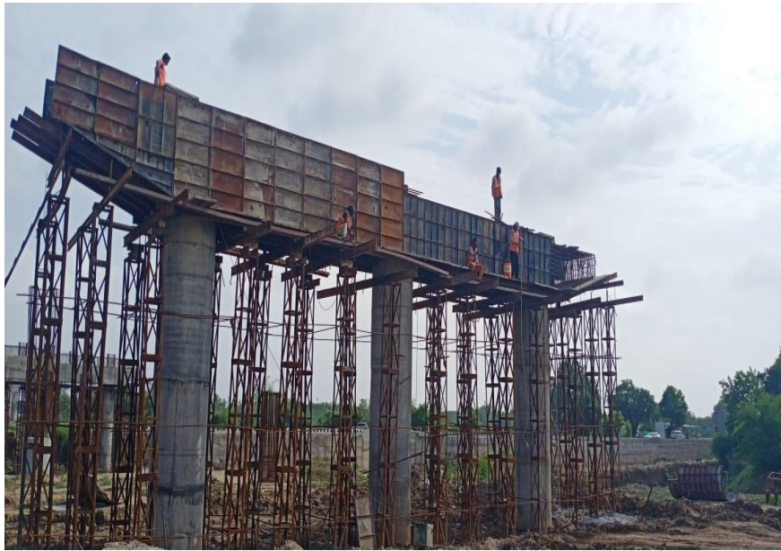
353+666 PIER CAP SHUTTERING WORK IN PROGRESS
