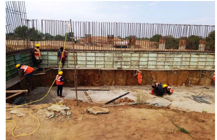
336+810 MJB RHS WALL LIFT SUTURING WORK IN PROGRESS
