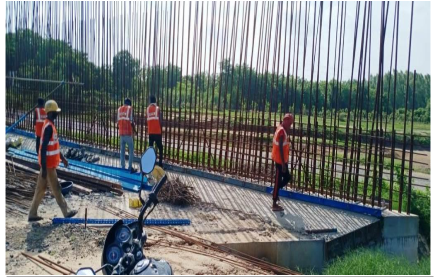
351+810 LVUP WALL STEEL BINDING & SHUTTERING WORK IN PROGRESS
