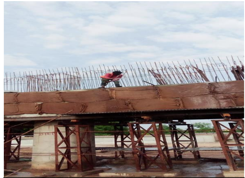
CURING WORK IN PROGRESS AT CH 354+636 MNB CAP
