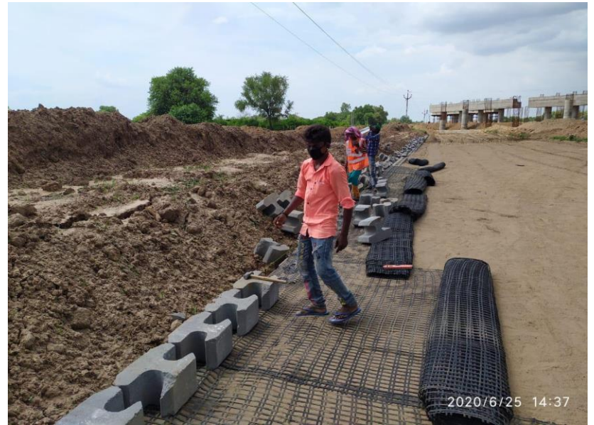
344+383 RE WALL GEOTEXTILE LAYING IN PROGRESS
