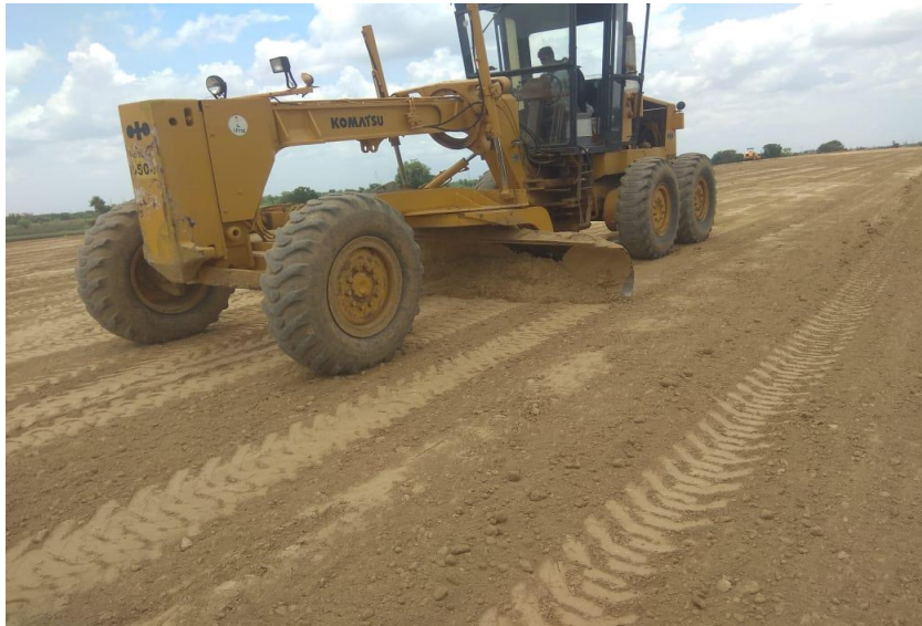
329+410 TO 329+550 EMBANKMENT FINISHING WORK PROGRESS
