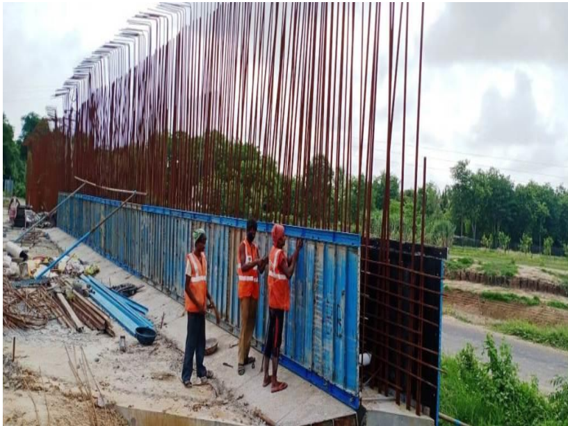
351+810 LVUP WALL SHUTTERING WORK IN PROGRESS
