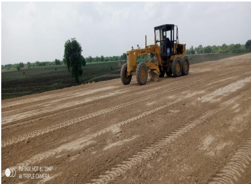
SUBGRADE TOP PREPARATION 329+550 TO 329+680
