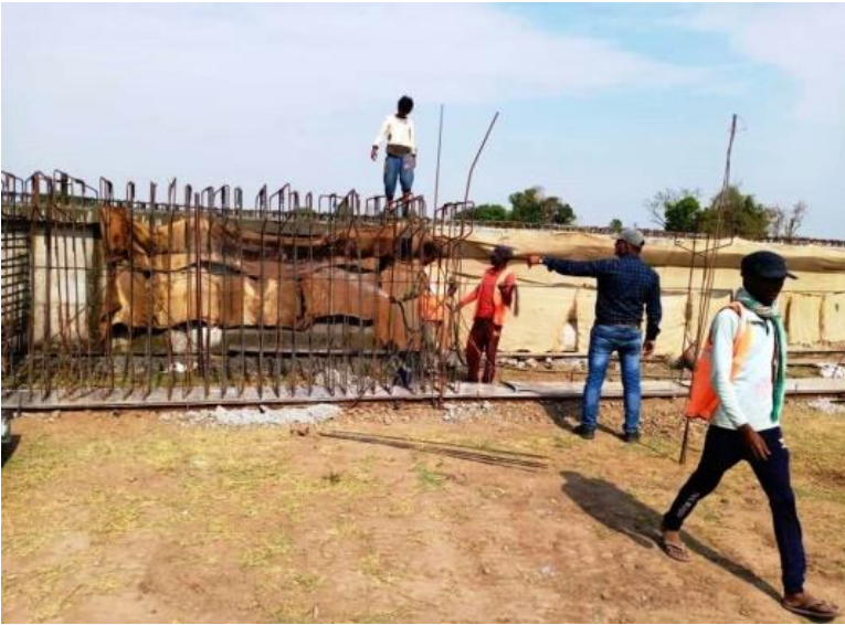
CURING WORK OF GIRDER AT INTERCHANGE CH 353+666
