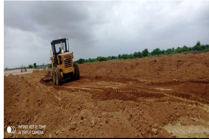
EMBANKMENT GRADING WORK AT CH 329+110 TO 329+270
