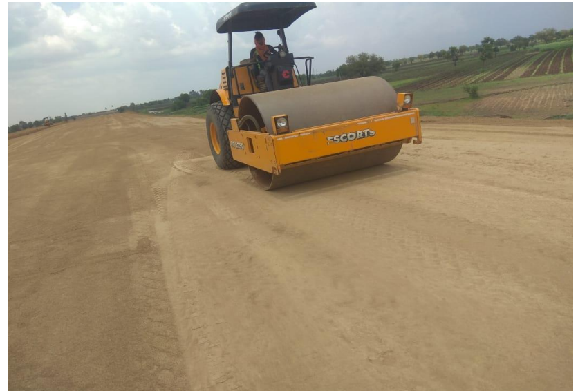
329+410 TO 329+550 EMBANKMENT ROLLING WORK PROGRESS
