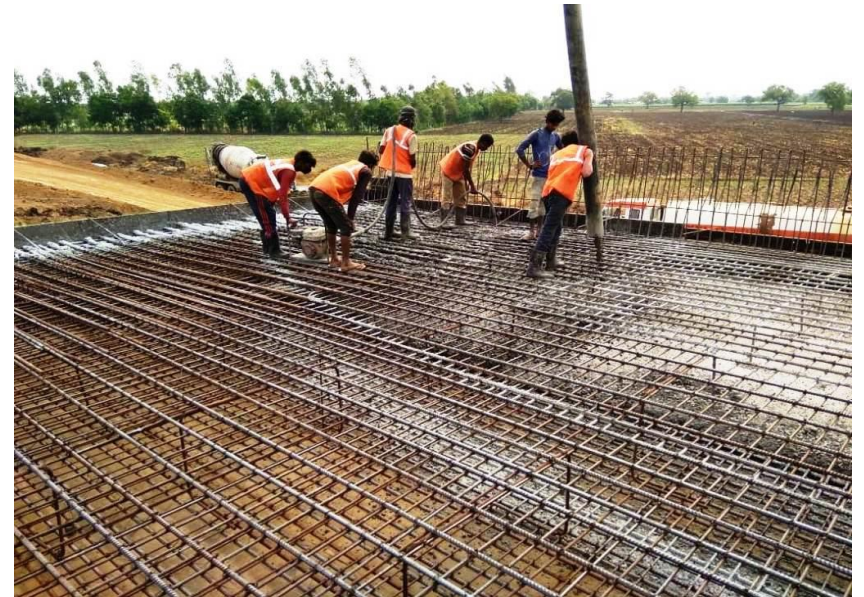
327+575 CUP SLAB CONCRETE POURING WORK IN PROGRESS
