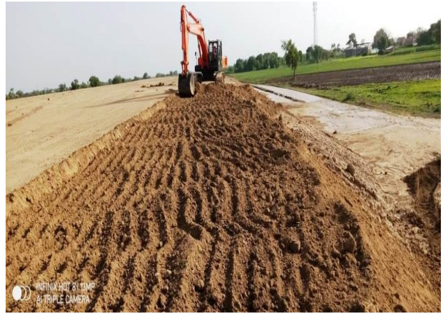
RAIN CUT REPAIRING AT CH 330+040 TO 330+230 LHS
