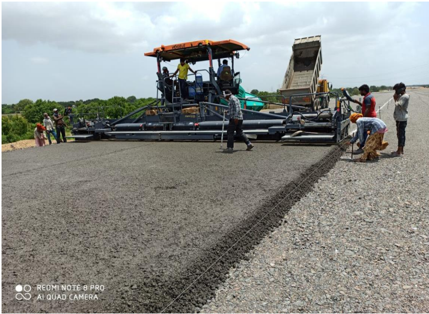
DLC LAYING WORK IN PROGRESS AT CH. 335+580 LHS
