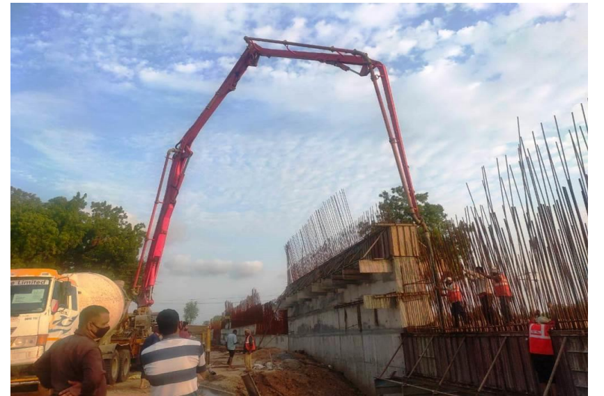
RETAINING WALL CONCRETE POURING IN PROGRESS FROM CH 353+440 TO 353+460
