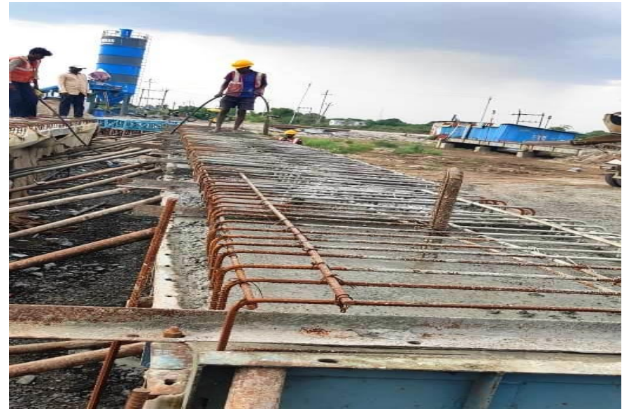
323+074 INTERCHANGE GIRDER CONCRETE POURING COMPLETED
