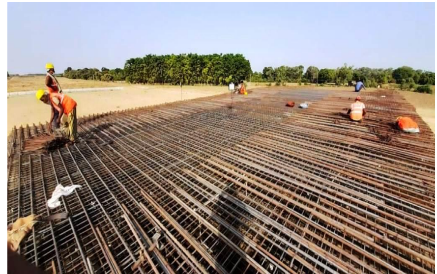
348+978 CUP RHS SLAB REINFORCEMENT BINDING WORK IN PROGRESS
