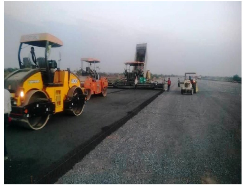
DLC LAYING IN PROGRESS AT CH 339+160 to 339+410 RHS
