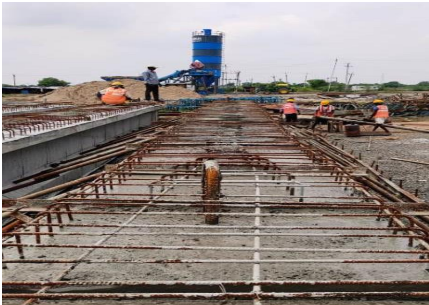
323+074 INTERCHANGE RCC GIRDER CONCRETE POURING IN PROGRESS
