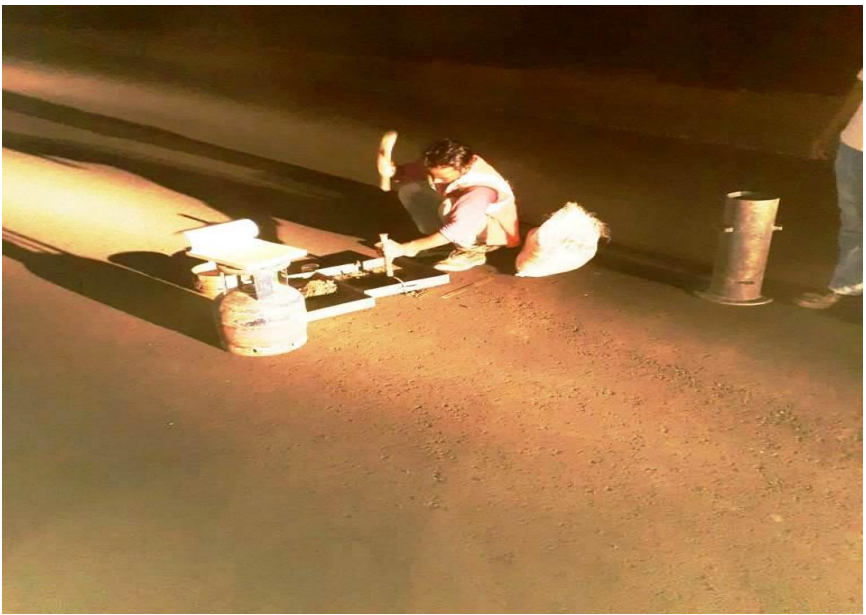
FDD CHECKING OF DLC AT CH 339+040 to 339+170 LHS
