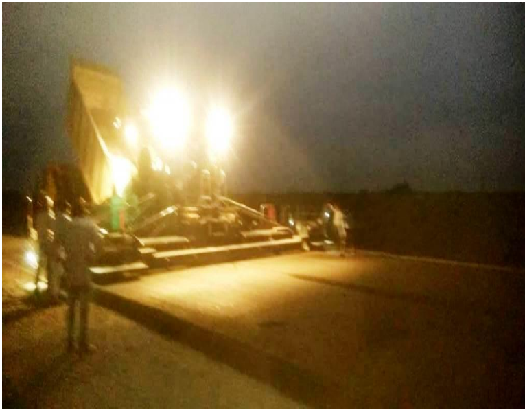
DLC LAYING IN PROGRESS AT CH 339+030 TO 339+170 LHS
