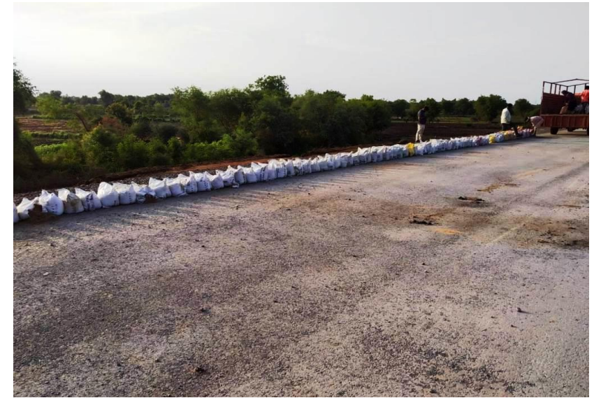
SLOPE PROTECTION WORK IN PROGRESS AT CH-334+900 TO 335+000 LHS
