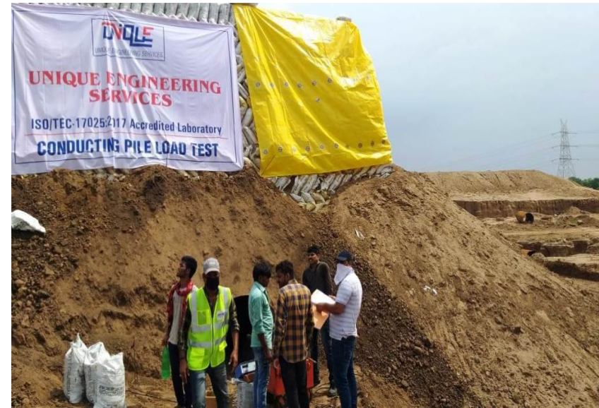
336+810 MJB PILE LOAD TESTING
