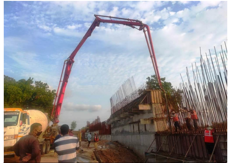
RETAINING WALL CONCRETE POURING IN PROGRESS FROM CH 353+440 TO 353+460
