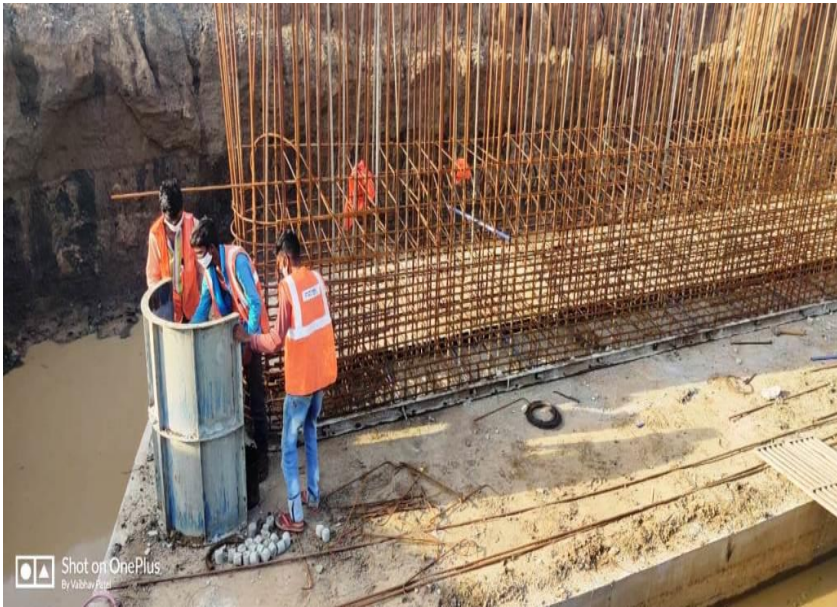
324+193 SHUTTERING WORK IN PROGRESS OF MNB PIER SHAFT
