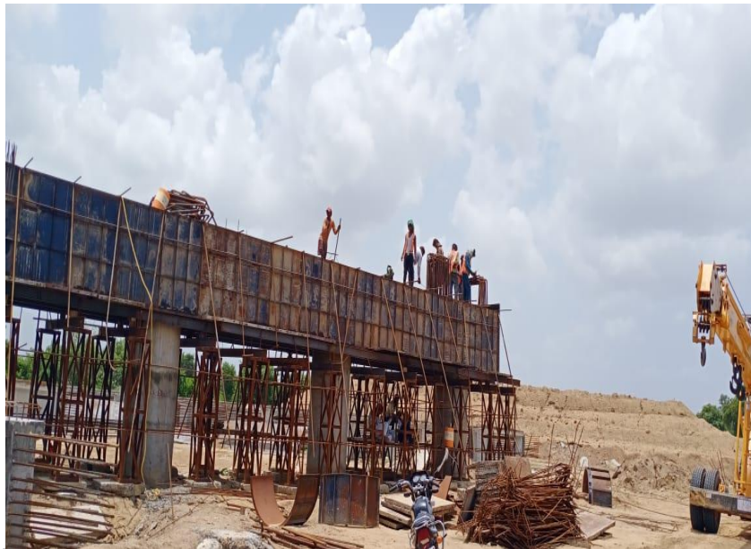
354+636 MNB PILE CAP STEEL BINDING WORK IN PROGRESS
