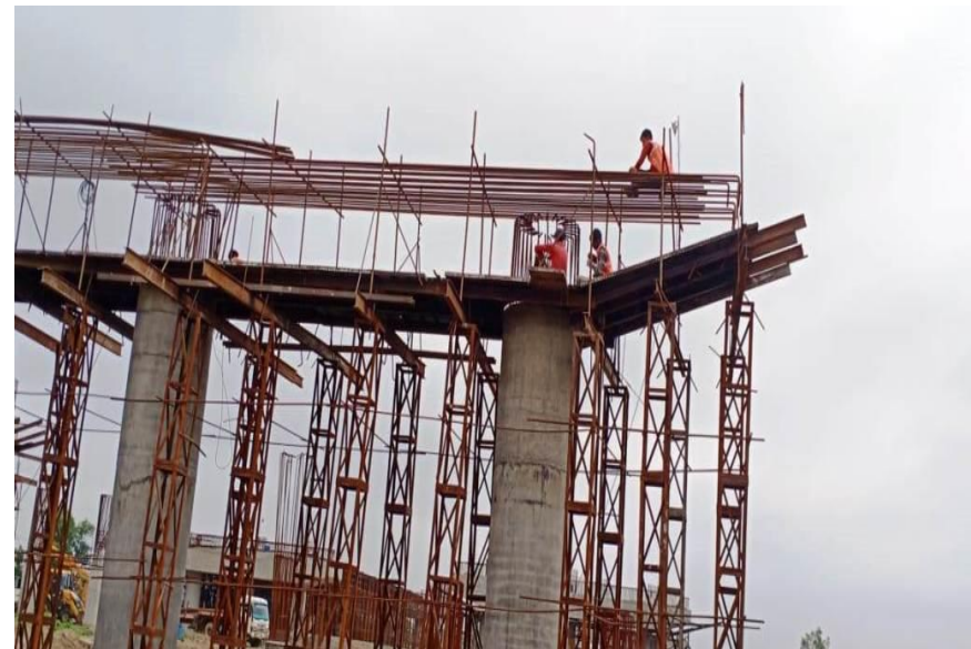
353+666 INTERCHANGE PIER CAP STEEL BINDING IN PROGRESS
