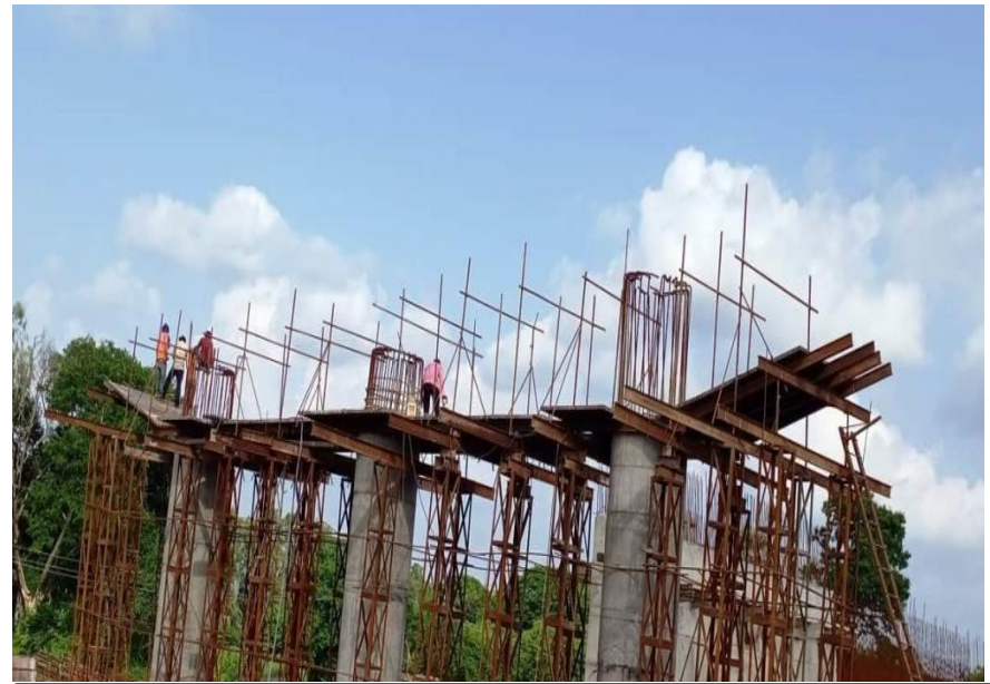
353+666 IC RA1 PIER CAP STEEL PLACING WORK IN PROGRESS
