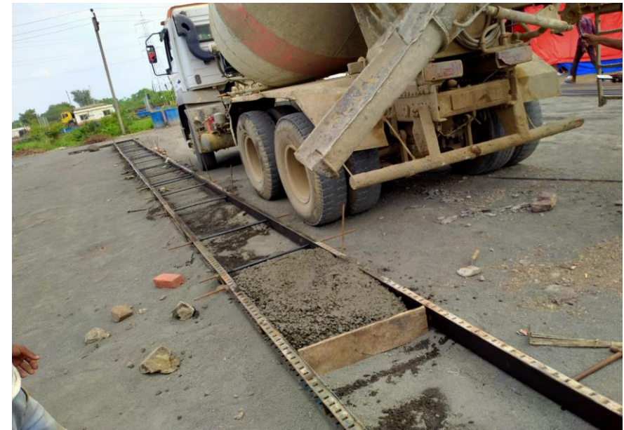
350+201 PREPARATION OF PCC BED FOR RCC GIRDER
