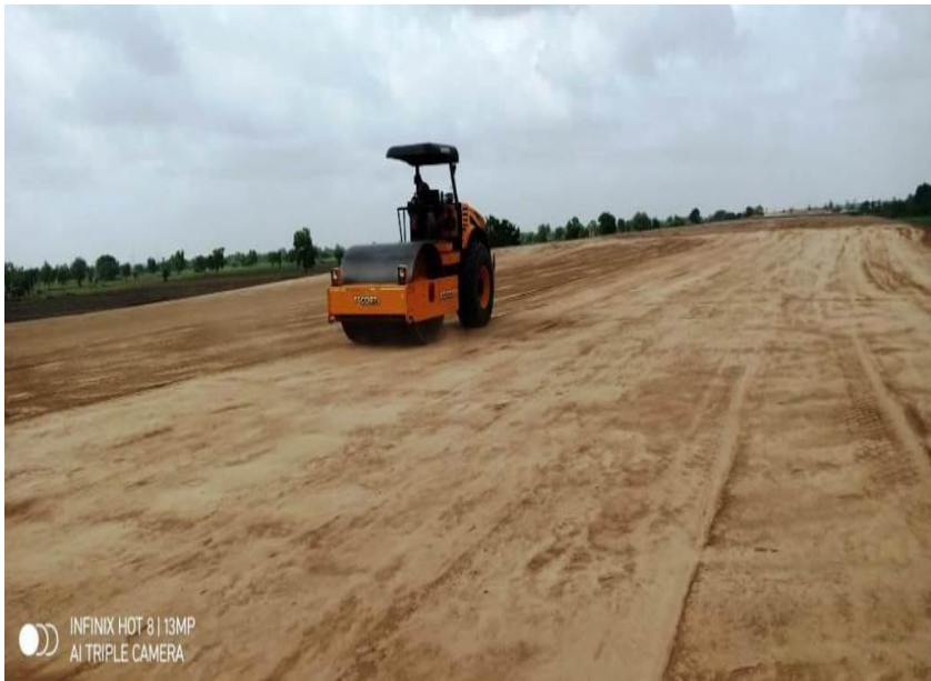
EMBANKMENT ROLLING WORK AT CH 330+180 TO 330+230
