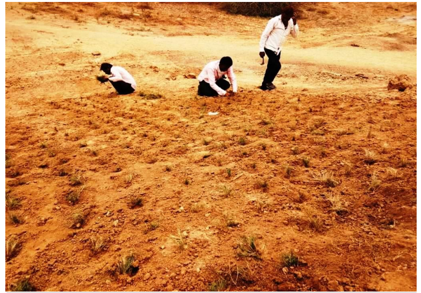
TURFING WORK IN PROGRESS AT CH 345+800 TO 345+940 LHS
