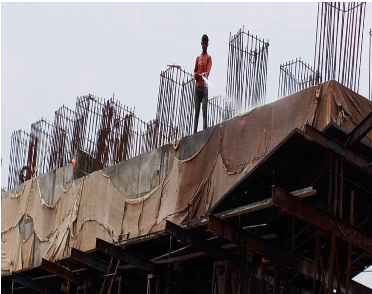
CURING OF PIER CAP WORK AT CH 353+666 INTERCHANGE
