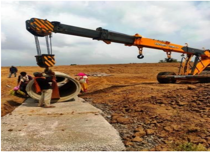
HPC PIPE LAYING WORK IN PROGRESS 349+668
