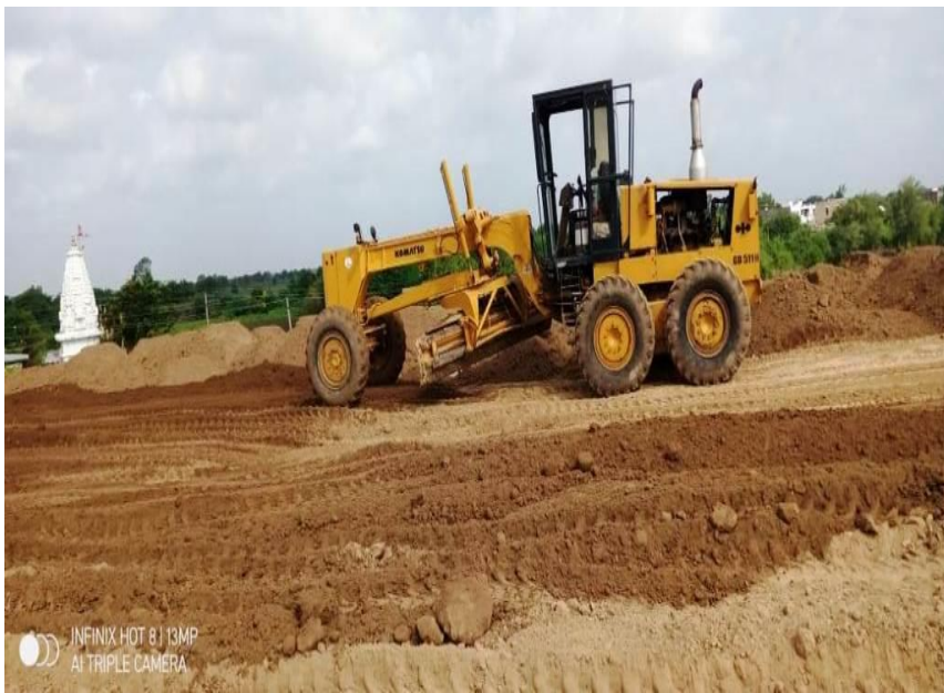
EMBANKMENT LAYER GRADING WORK AT CH 329+410 TO 329+550
