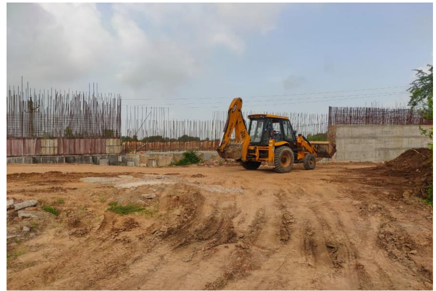
RETAINING WALL BACKFILLING IN PROGRESS AT CH 353+470 TO 353+490
