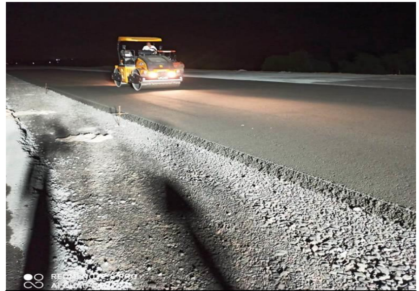
DLC LAYING FINISHING ROLLER WORK AT CH 335+580 TO 335+780 RHS
