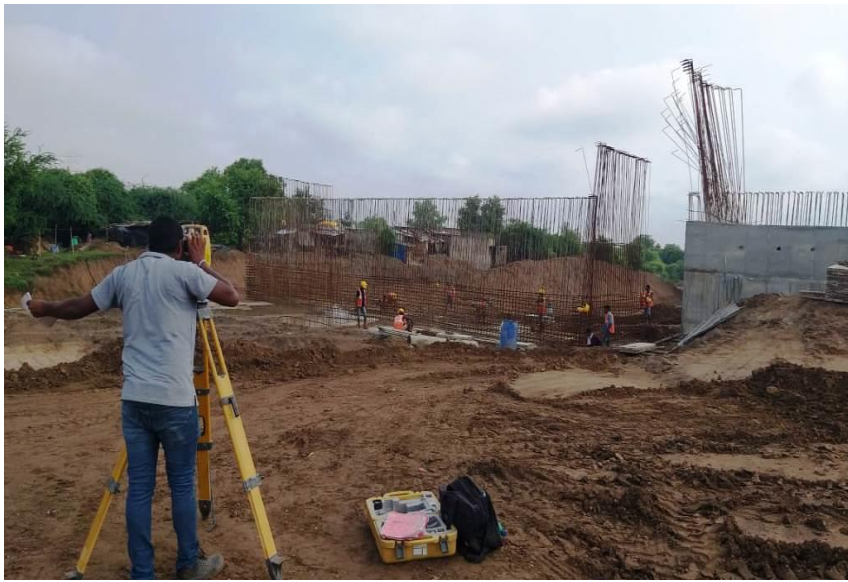
336+810 MJB LHS POINT MARKING AND STARTER FIXING WORK IN PROGRESS
