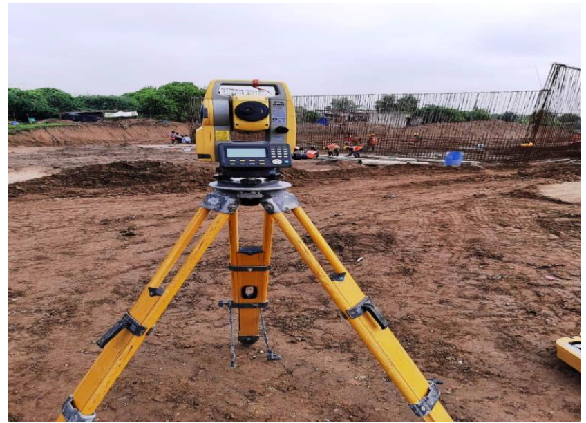
336+800 LA2 WALL LAYOUT MARKING WORK
