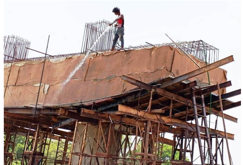
CURING WORK OF PIER CAP AT INTERCHANGE CH 353+666
