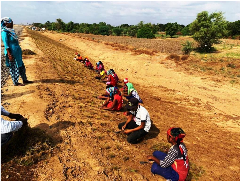
TURFING WORK IN PROGRESS AT CH 345+150 TO 345+400 LHS
