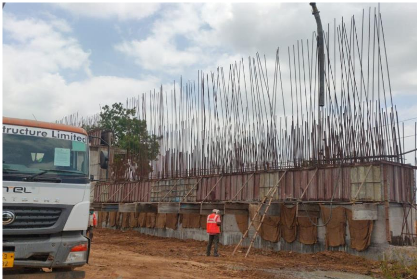
353+450 to 353+470 RETAINING WALL CONCRETE POURING PROGRESS
