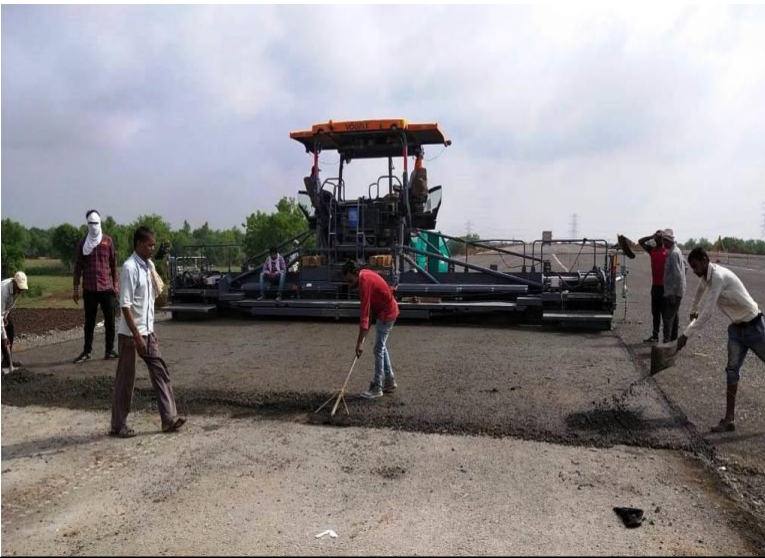
DLC LAYING WORK IN PROGRESS AT CH 335+060 TO 335+120 LHS
