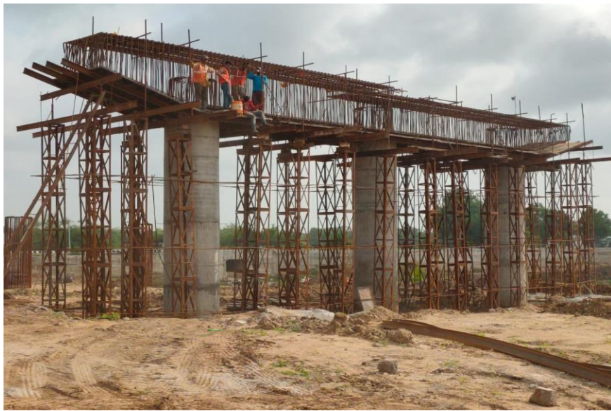
353+666 INTERCHANGE PIER CAP STEEL BINDING WORK
