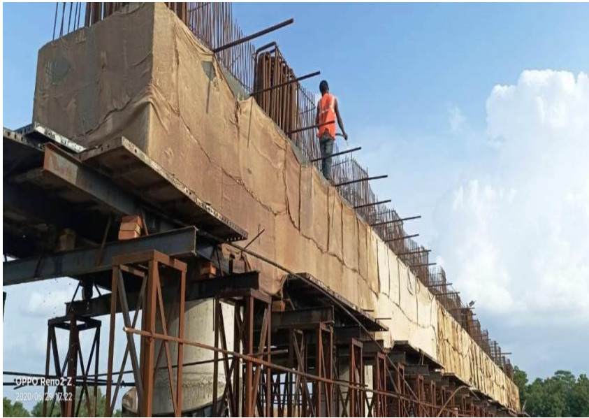
354+636 MNB PIER CAP CURING IN PROGRESS
