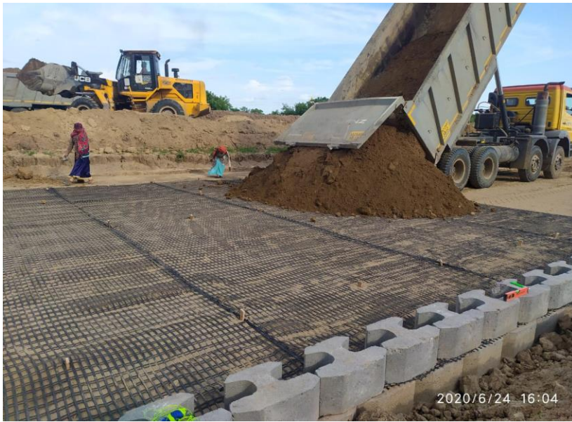
344+383 RE WALL BACKFILLING WORK IN PROGRESS
