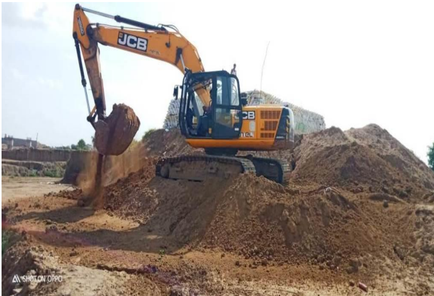
336+810 MJB PILE LOAD TESTING PREPARATION WORK IN PROGRESS
