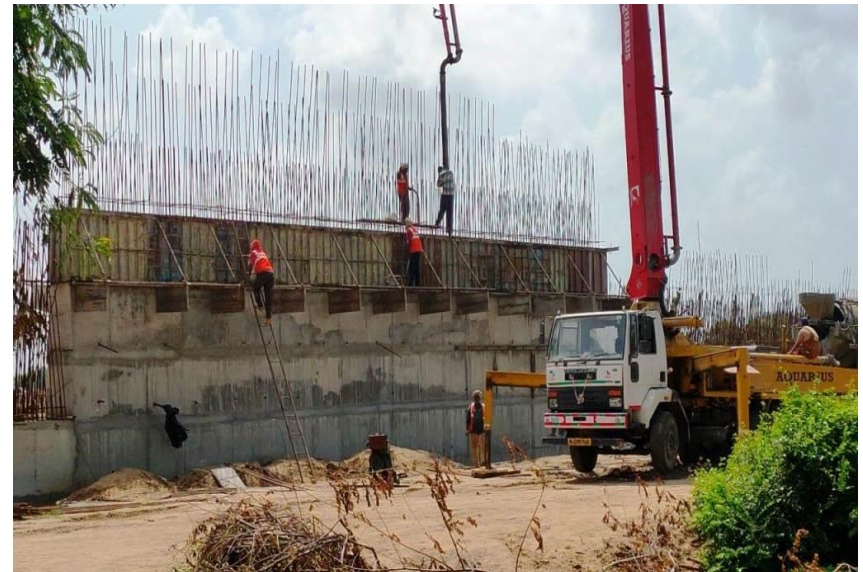
RETAINING WALL 353+440 LIFT CONCRETE POURING IN PROGRESS
