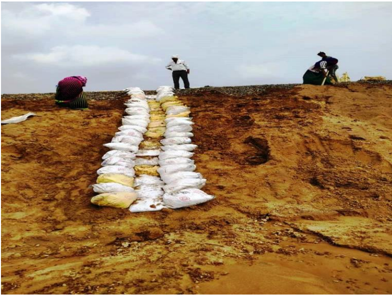
RAIN CUT PROTECTION WORK AT CH 334+620 LHS
