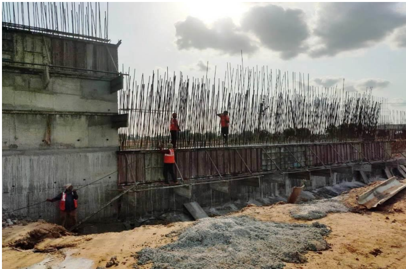
RETAINING WALL REINFORCEMENT & SHUTTERING WORK AT CH 353+420 TO 353+440,
