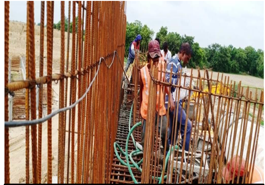
354+636 MNB ABUTMENT CAP CONCRETE POURING WORK
