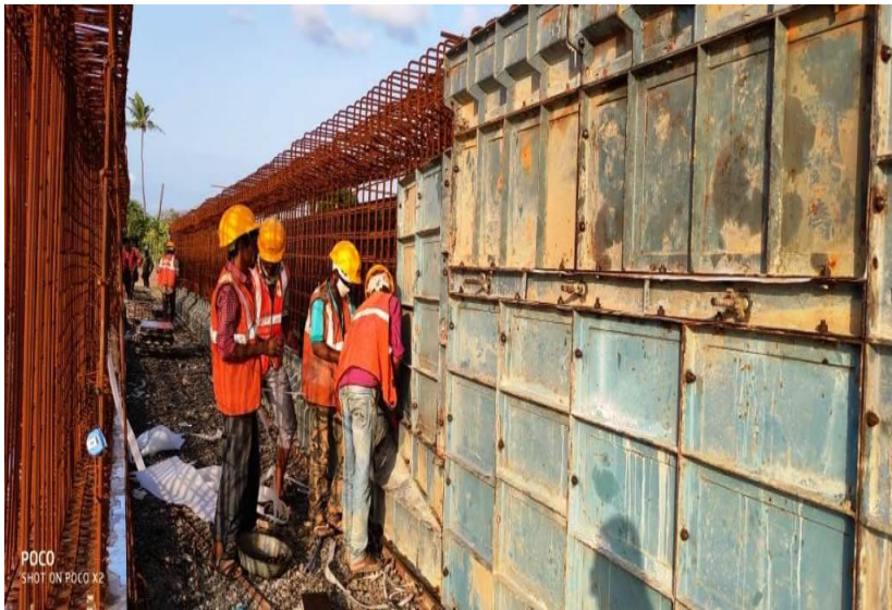
330+640 MNB PSC GIRDER SHUTTERING WORK IN PROGRESS
