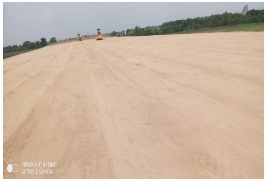
EMBANKMENT TOP ROLLING WORK IN PROGRESS AT CH.329+550 TO 329+700 BHS
