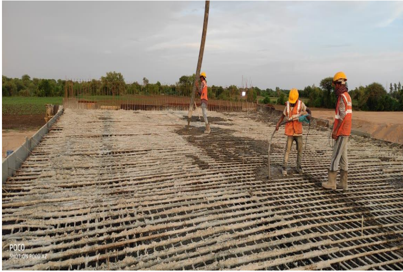
328+175 CUP LHS TOP SLAB & TOP HAUNCH CONCRETE POURING IN PROGRESS
