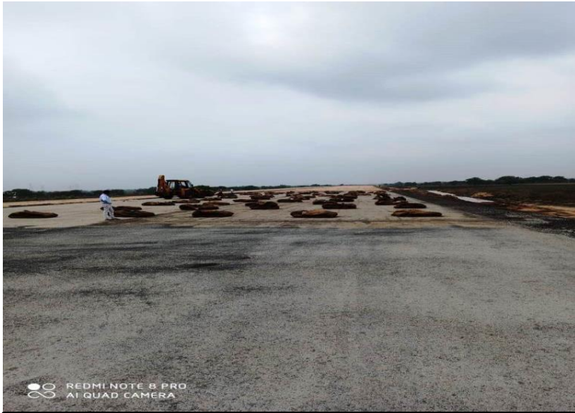
339+500 HESSIAN CLOTHES FOLDING IN PROGRESS
