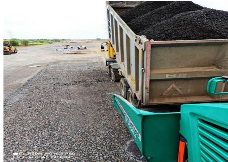
DLC LAYING WORK PROGRESS AT CH 335+580 TO 335+700
