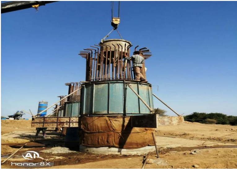
336 +810 MJB CONCRETE POURING WORK IS IN PROGRESS
