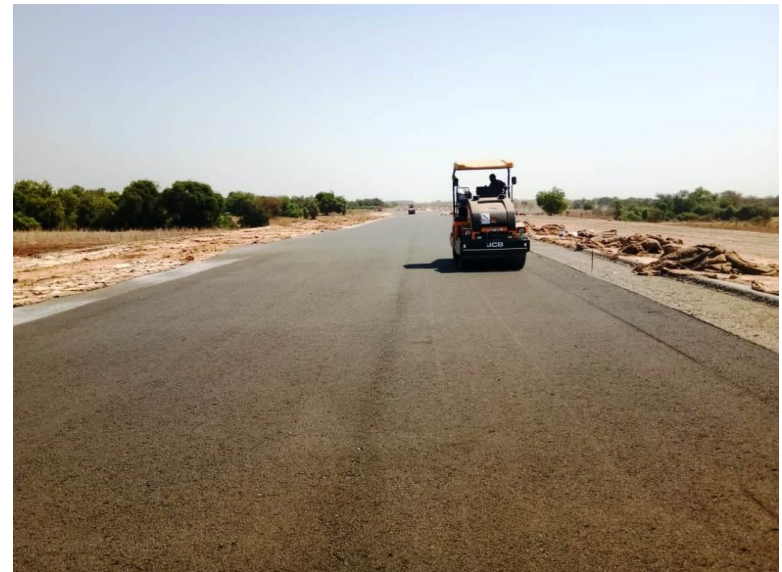
DLC LAYING COMPLETED AT CH 345+770 TO 346+030 LHS
