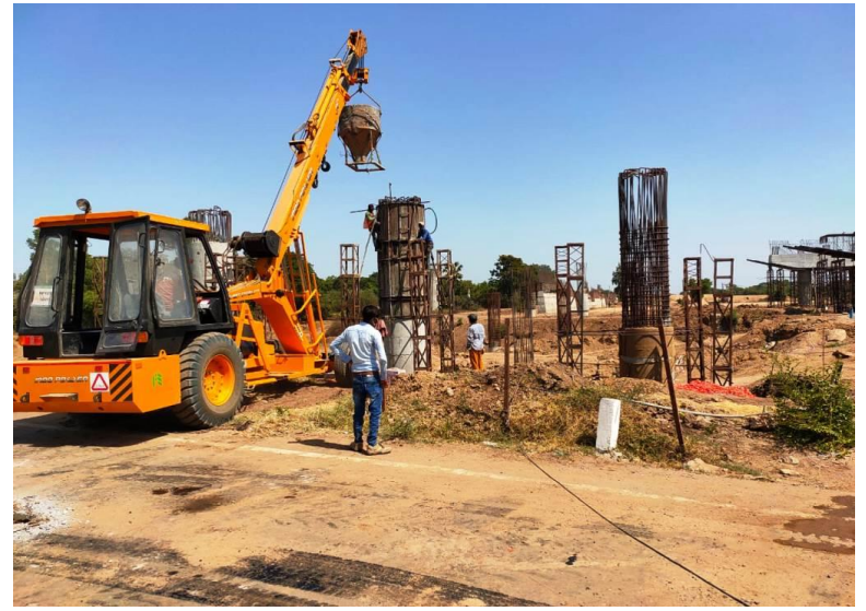
353+666 INTERCHANGE FINAL LIFT PIER CONCRETE POURING IN PROGRESS
