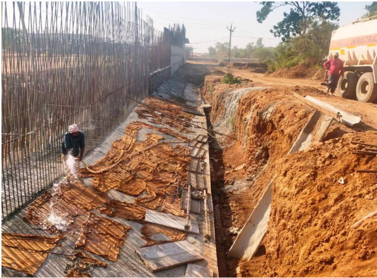
353+440 TO 353+460. RETAINING WALL RAFT & WALL CURING WORK PROGRESS
