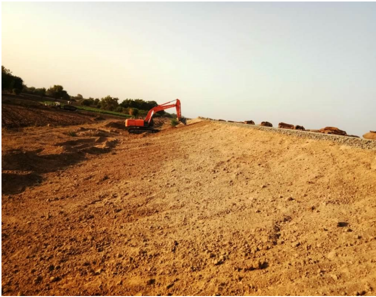
SLOP CUTTING WORK IN PROGRESS 346+300
