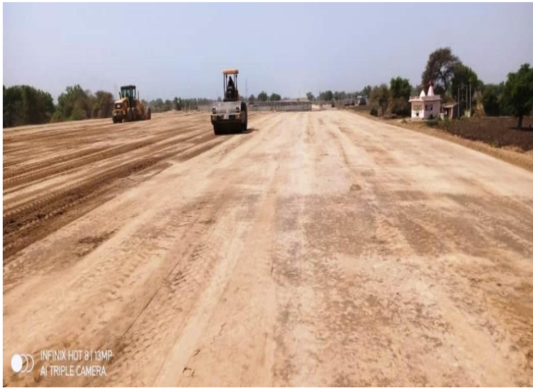
EMB FINISHING AND ROLLING AT 325+810 TO 326+010 BHS
