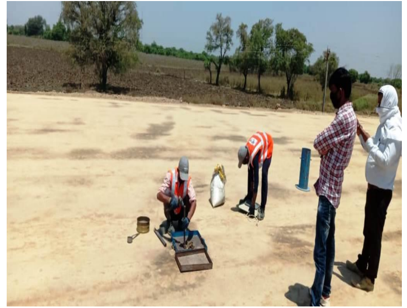
FDD CHECKING OF SUBGRADE FROM 332+300 TO 332+ 400
