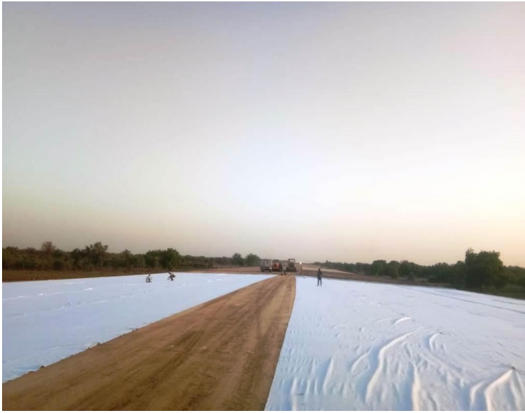
GEOTEXTILE LAYING WORK IN PROGRESS
