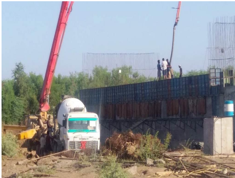
337+874 MNB CONCRETE POURING WORK IS IN PROGRESS
