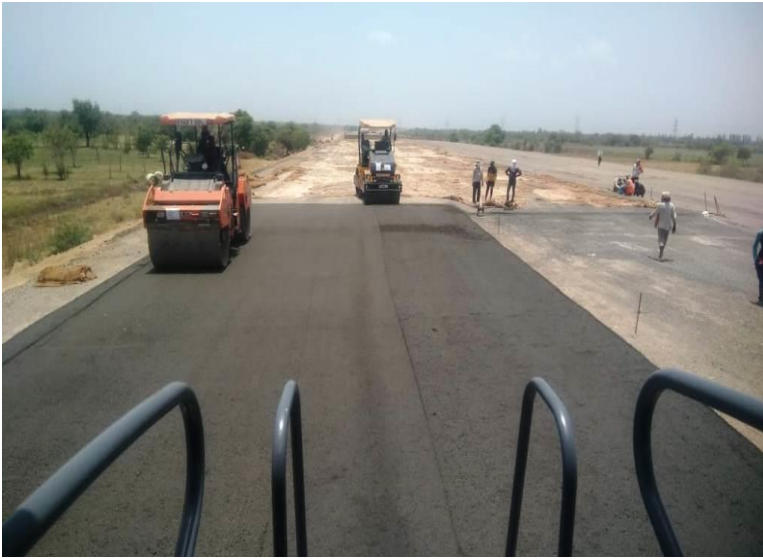
DLC LAYING WORK IS IN PROGRESS AT CH 338+750 to 338+880 RHS
