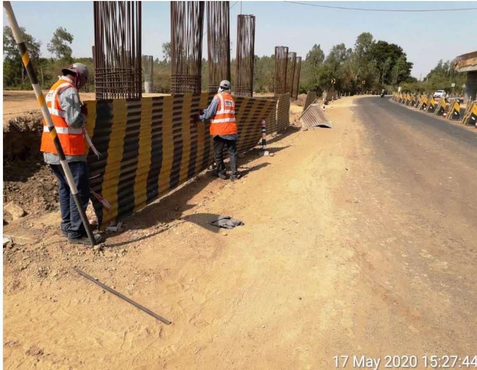
HARD BARRICADING SIGN BOARD INSTALLED AT CH. 353
