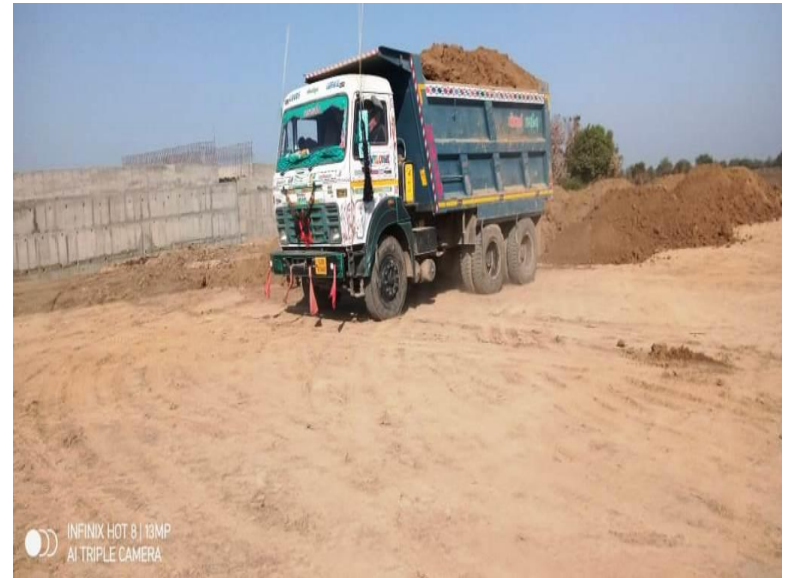
324+920 TO 970 EMB BHS DUMPING WORK
