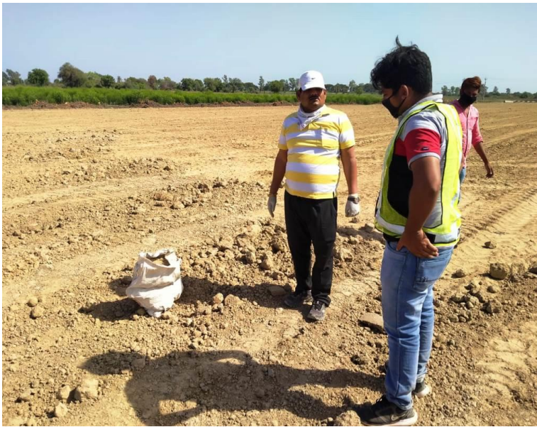
JOINT SAMPLE AT CH-331+450 TO 331+690
