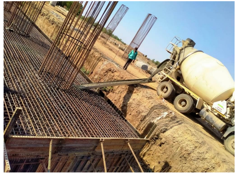
344+383 FLY OVER PILE CAP CONCRETE POURING WORK IS IN PROGRESS
