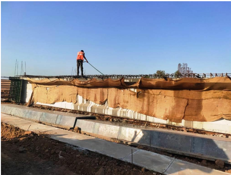
353+666 INTERCHANGE GIRDER CURING WORK IN PROGRESS
