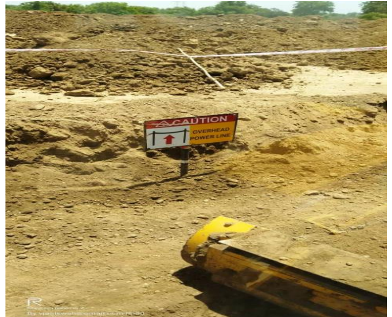
"OVERHEAD POWER LINE" SIGN BOARD REMOVED & REINSTALLED AT CH 324+900
