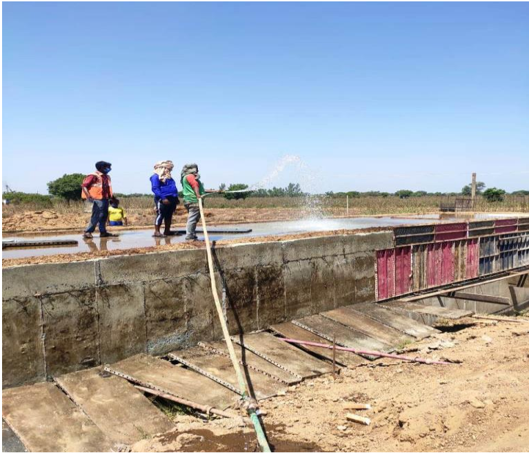
CURING AT 324+987 BC SLAB
