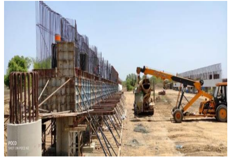
330+640 MNB PIER CAP CONCRETE POURING IN PROGRESS
