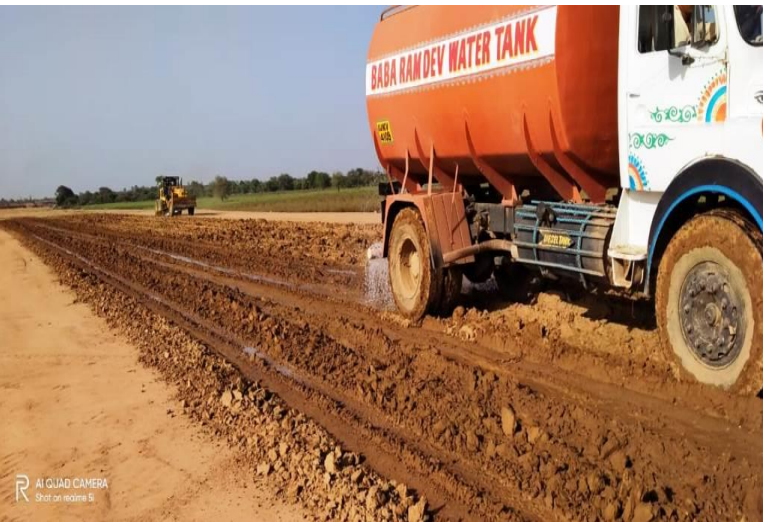
MIXING AND WATERING SIMULTANEOUSLY AT CH.328+400 TO 328+500
