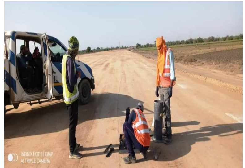
SUB GRADE CHECKING FROM 328+300 TO 400 BHS
