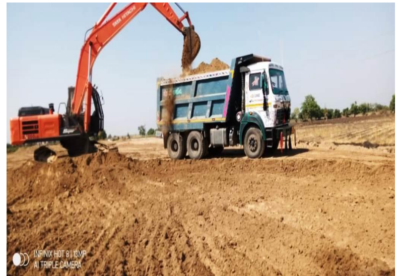
RECTIFICATION WORK AT CH 325+650 TO 325+740
