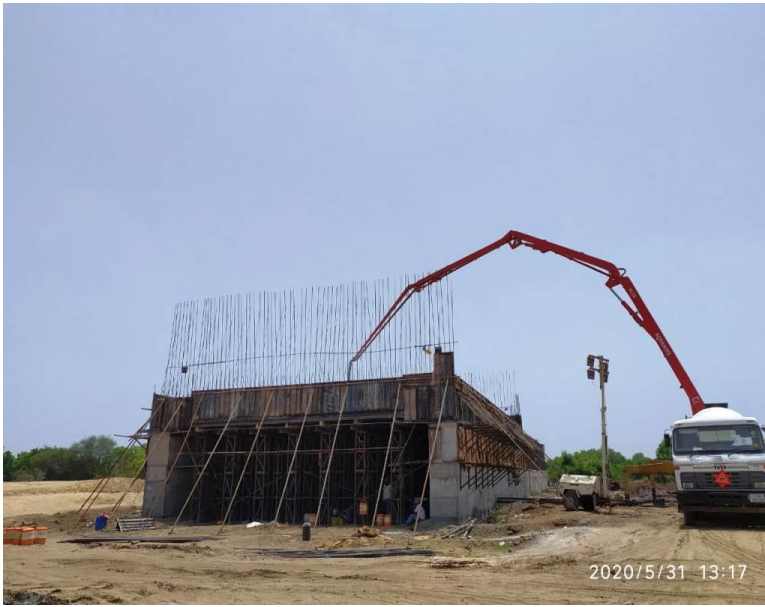
352+700 CUP RHS SLAB CONCRETE POURING IN PROGRESS-
