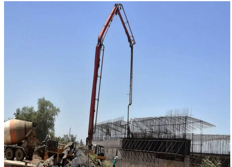
351+284 VUP RHS WALL LIFT CONCRETE POURING IN PROGRESS
