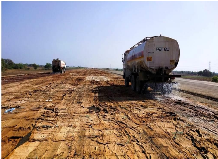
DLC CURING AT 338+600 TO 338+870 LHS
