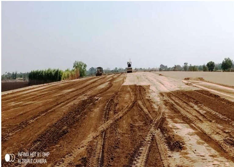
327+940 TO 328+150 RHS FINISHING AND ROLLING WORK
