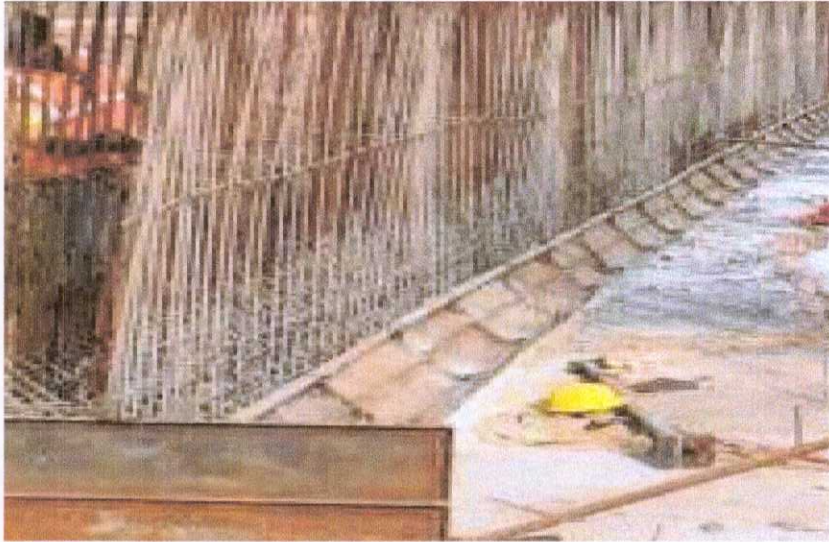
351+009 BOX CULVERT PROTECTION OF REINFORCEMENT BY CEMENT SLURRY.
