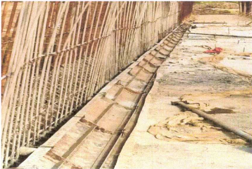
347+922 CUP PROTECTION OF REINFORCEMENT BY CEMENT SLURRY.
