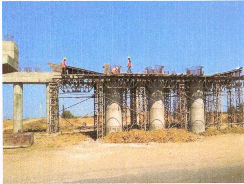
323+074 INTERCHANGE PIER CAP SHUTTERING WORK IS IN PROGRESS
