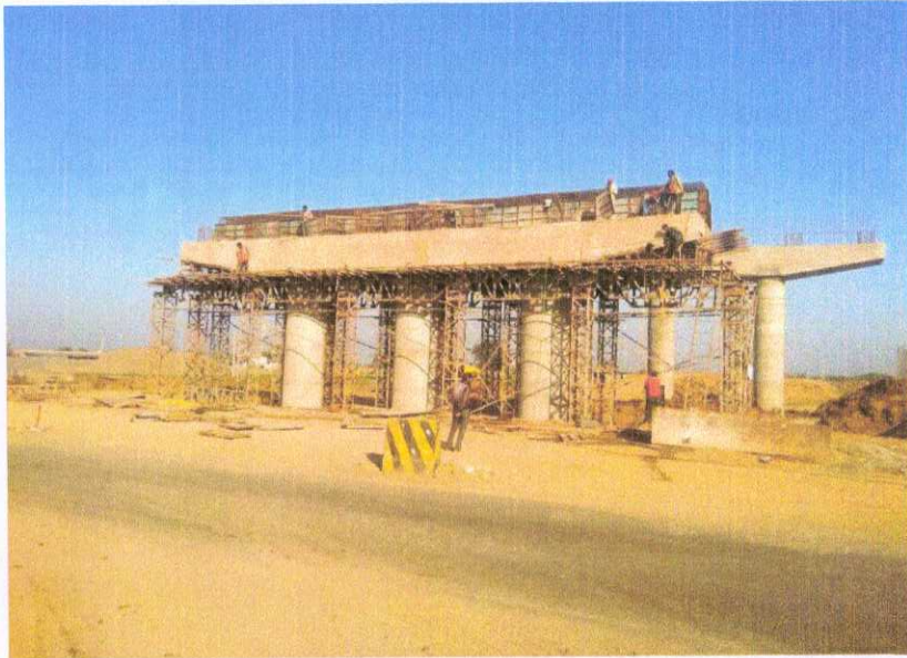
323+074 LHS PIER CAP SHUTTERING WORK IN PROGRESS
