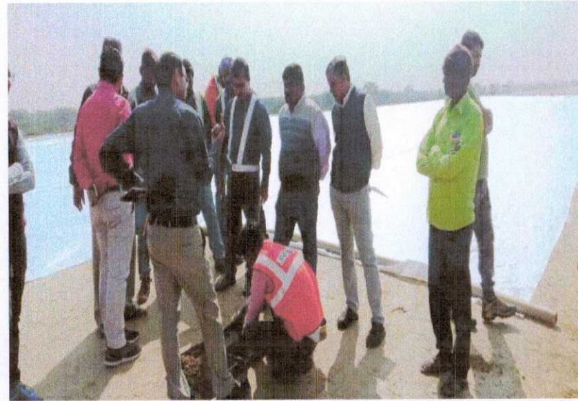
SG TESTING AT CH 338+050 TO 338+100
