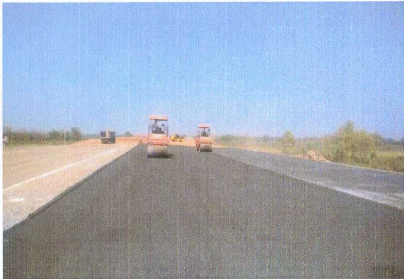
DLC LAYING COMPLETED AT CH. 332+970 to 333+090 RHS
