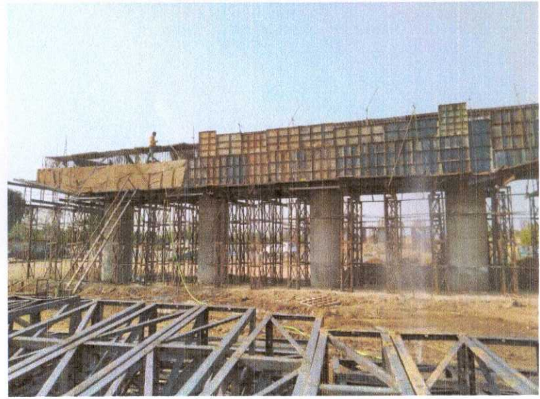
353+666 IC LP3 PIER CAP CURING WORK IS IN PROGRESS
