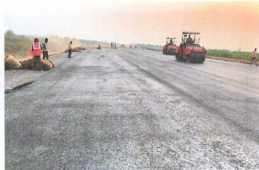
ROLLING AND HESSIAN CLOTH SPREADING WORK IS IN PROGRESS AT DLC
