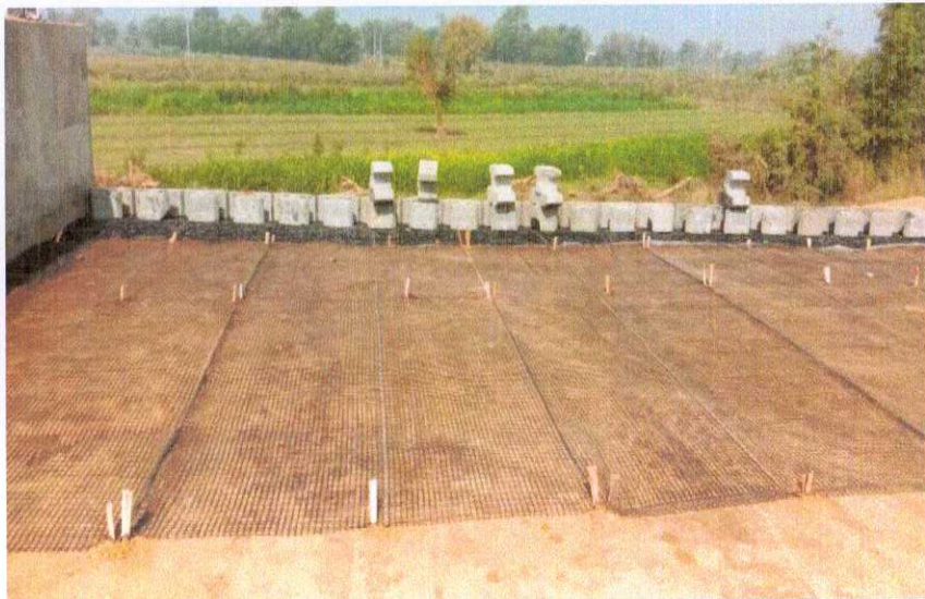
334+868 CUP RE WALL BLOCK ERRECTION AND GEOGRID LAYING IN PROGRESS
