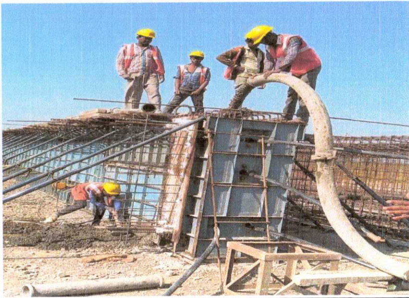
330+640 MNB GIRDER CASTING IN PROGRESS
