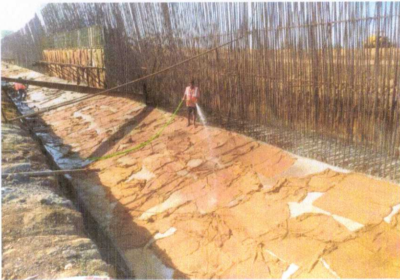
353+265 TO 353+285 RHS RETAINING WALL RAFT CURRING
