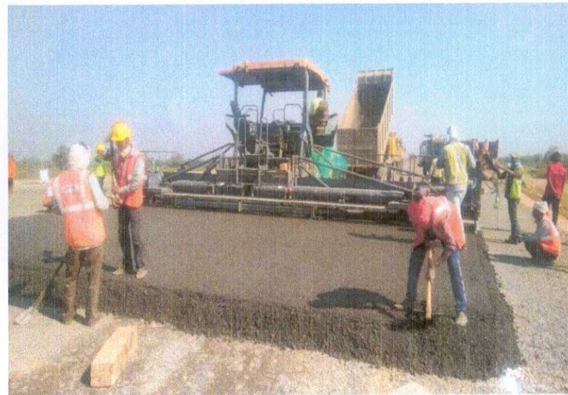
DLC LAYING IN PROGRESS AT CH. 332+970 TO 333+090 RHS
