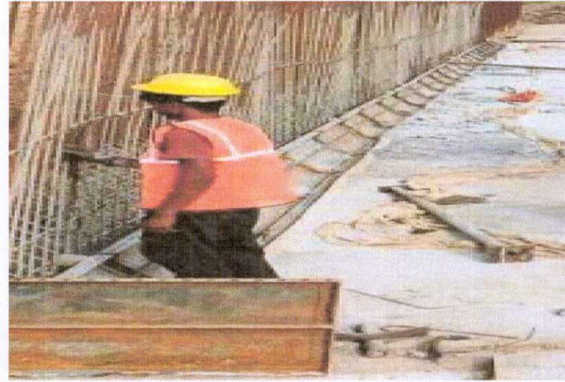
347+922 CUP PROTECTION OF REINFORCEMENT BY CEMENT SLURRY.
