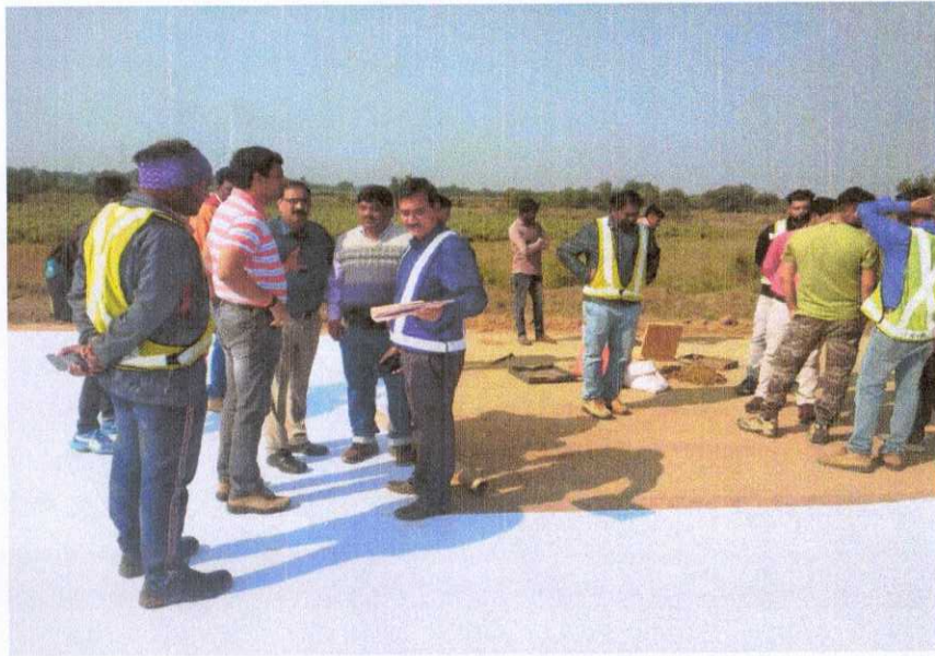
SG TESTING AT CH 338+050 TO 338+100
