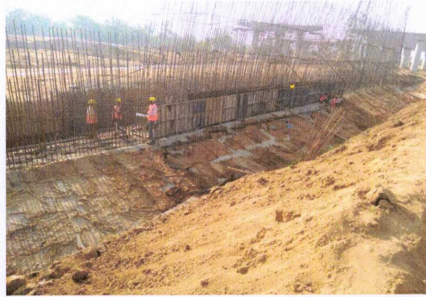
RETAINING WALL SHUTTERING WORK IN PROGRESS AT CH NO 323+172 TO 323+192 LHS
