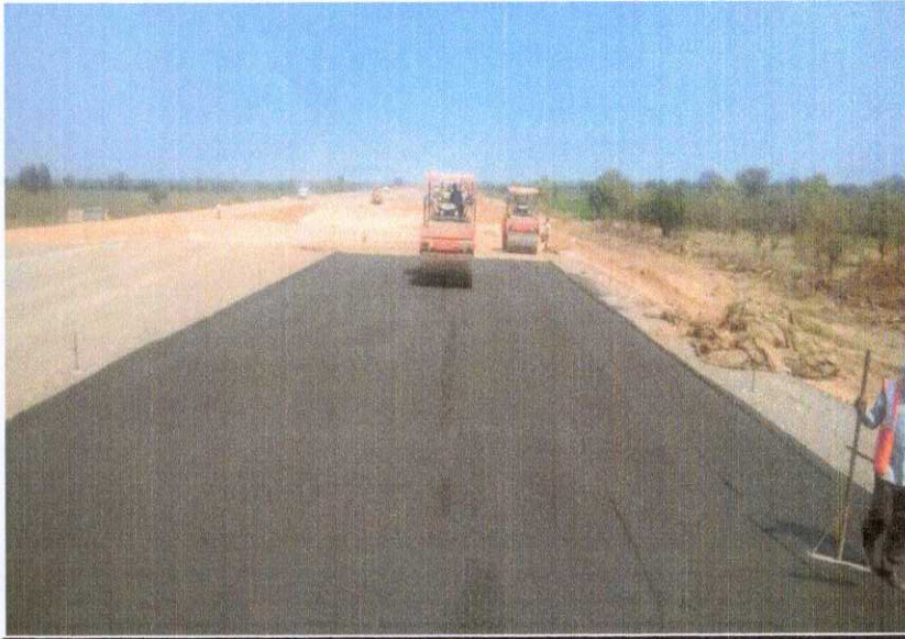
DLC LAYING WORK IS IN PROGRESS AT CH. 332+720 TO 332+850 RHS
