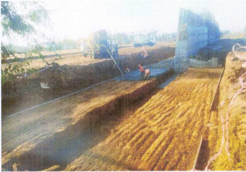
RETAINING WALL RHS PCC WORK IS IN PROGRESS AT CH. 353+490 TO 353+510
