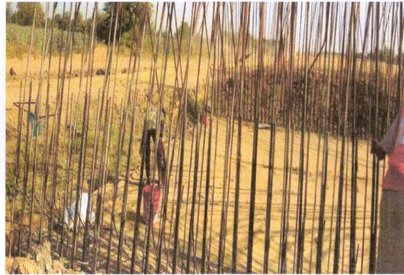
347+922 CUP PROTECTION OF REINFORCEMENT BY CEMENT SLURRY.
