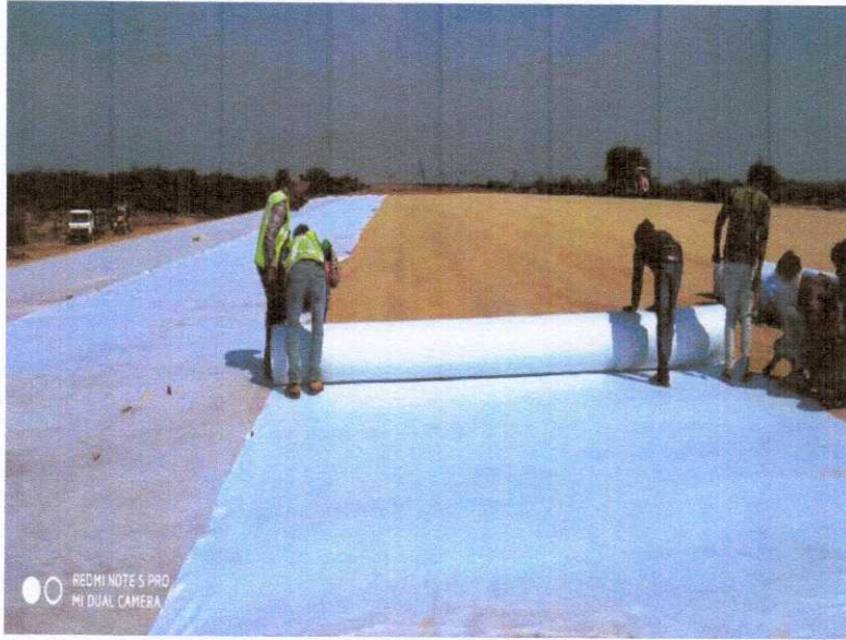
GEO TEXTILE LAYING WORK IS IN PROGRESS
