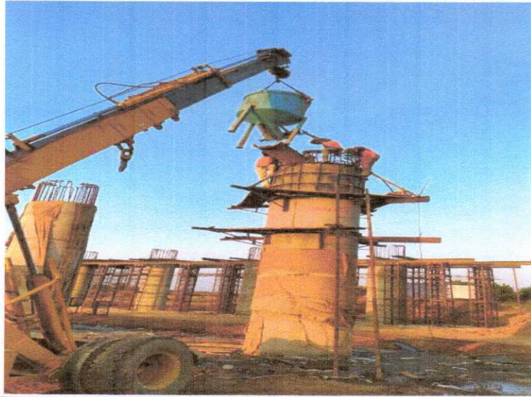
344+383 FLYOVER PIER LIFT CONCRETE POURING WORK IS IN PROGRESS
