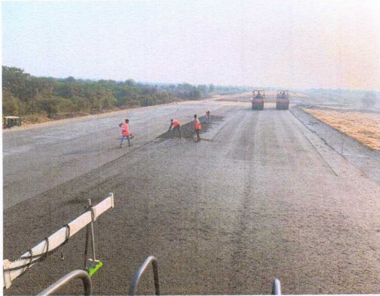
DLC LAYING WORK IS IN PROGRESS AT 338
