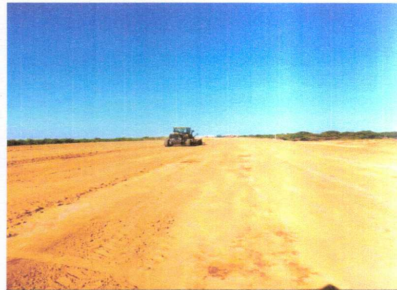
EMBANKMENT LAYER TOP IS IN PROGRESS AT CHAINAGE 337+620 TO 337+800.
