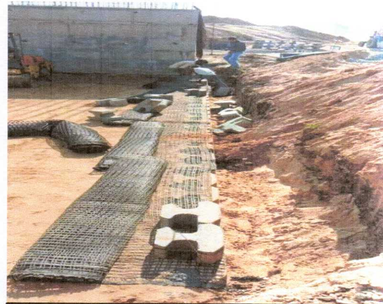
334+280 CUP LHS RE WALL GEOGRID LAYING IN PROGRESS
