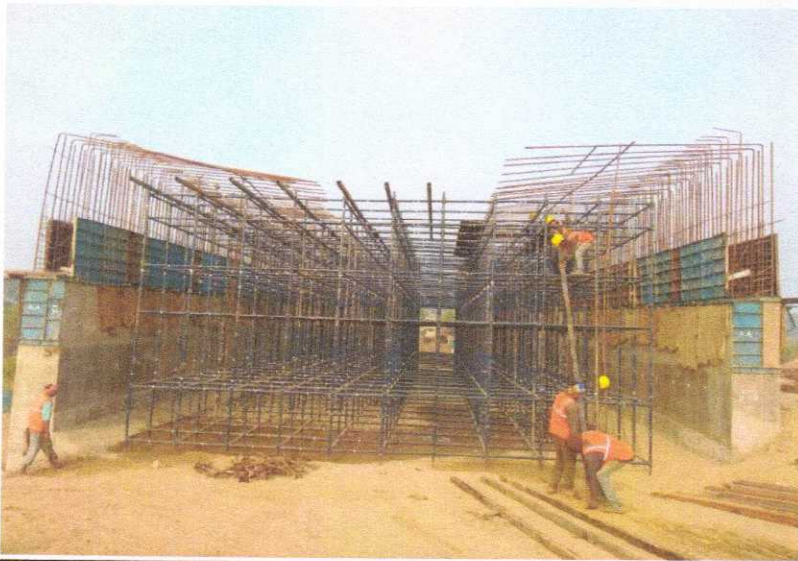
337+022 LVUP SCAFFOLDING WORK FOR LVUP SLAB IS IN PROGRESS
