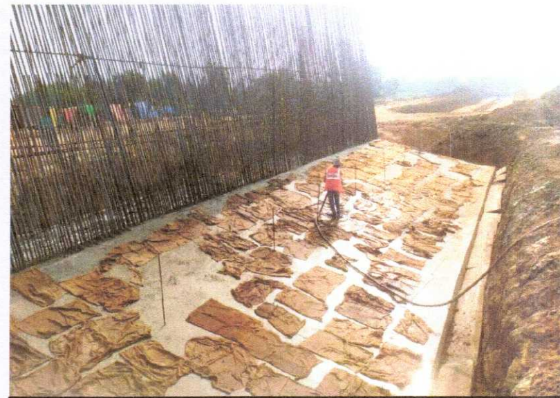
RETAINING WALL 353+320 TO 340 RHS RAFT CURING WORK
