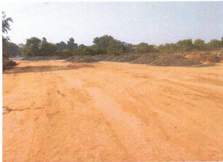
GSB DUMPING AT 353+650 INTERCHANGE DIVERSION
