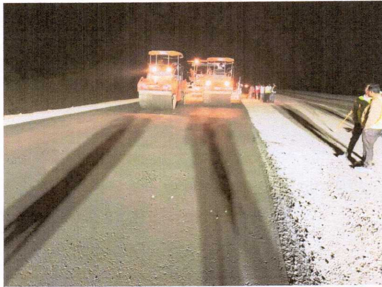
DLC LAYING WORK IS IN PROGRESS FROM 337+960 TO 338+060
