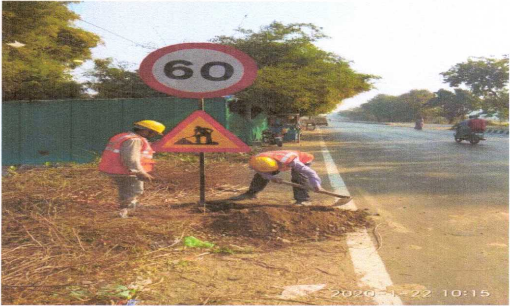
ADVANCE INFORMATORY SIGN BOARDS INSTALLATION AT 353+666 DIVERSION
