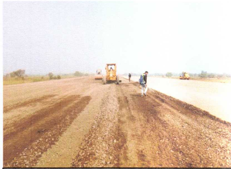
GSB BED PREPARATION WORK IS IN PROGRESS FROM 337+950 TO 338+050 LHS
