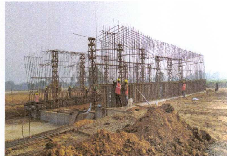
347+108 CUP 01ST LIFT WALL STEEL BINDING AND SHUTTERING WORK IN PROGRESS
