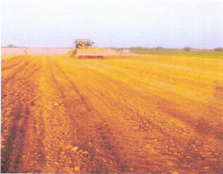
PREPARING EMB TOP AT CH. 332+950 TO 333+150
