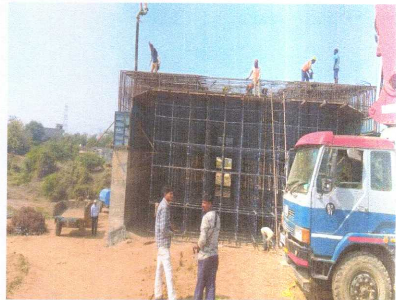
337+022 LVUP CONCRETE POURING WORK IS IN PROGRESS
