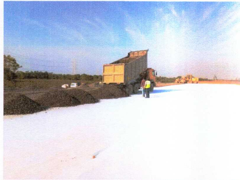
GSB DUMPING WORK IS IN PROGRESS
