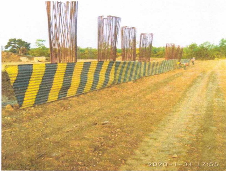
TIN SHEET BARRICADING AT 353+666 DIVERSION
