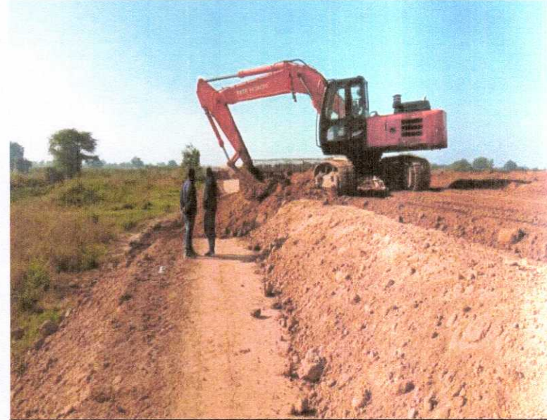
340+500 TO 800 PREPARATION OF SLOP WORK IN PROGRESS
