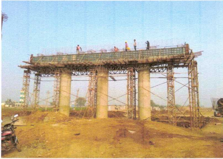
323+074 INTERCHANGE LHS PIER CAP CONCRETE POURING IS IN PROGRESS
