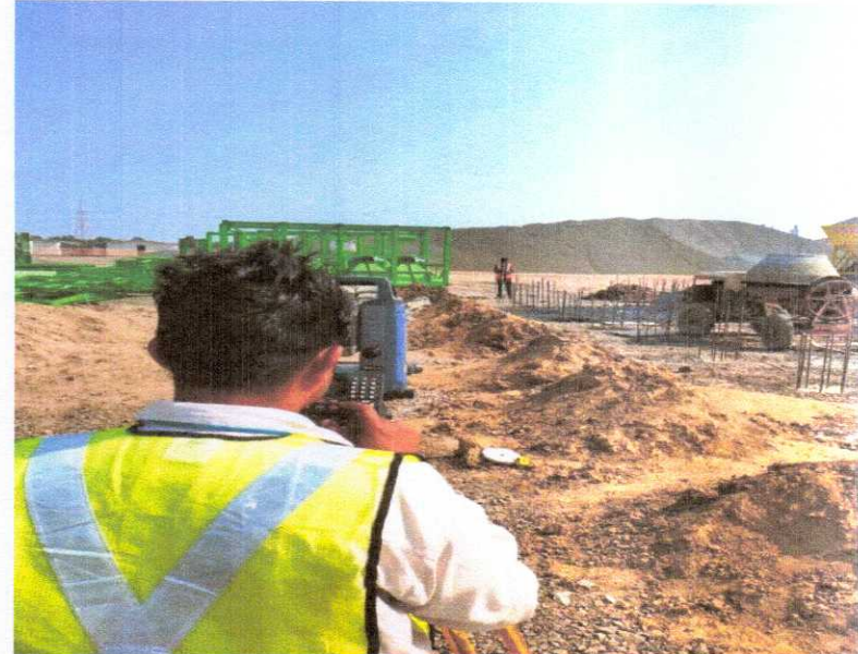
ERECTION OF PQC CONCRETE PLANT IN PROGRESS
