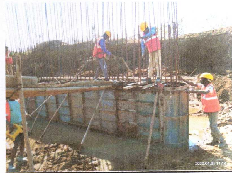
324+193 MNB PIER LIFT CONCRETE POURING IN PROGRESS
