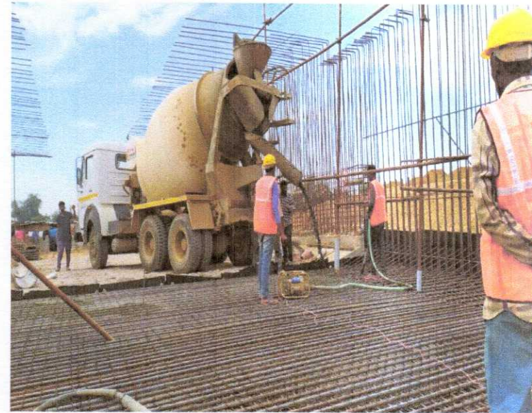
345+653 CUP RHS RAFT CONCRETE POURING IN PROGRESS
