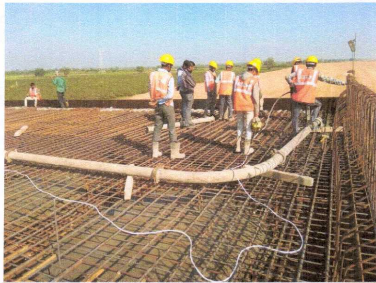
323+720 CUP LHS SLAB CONCRETE WORK IN PROGRESS
