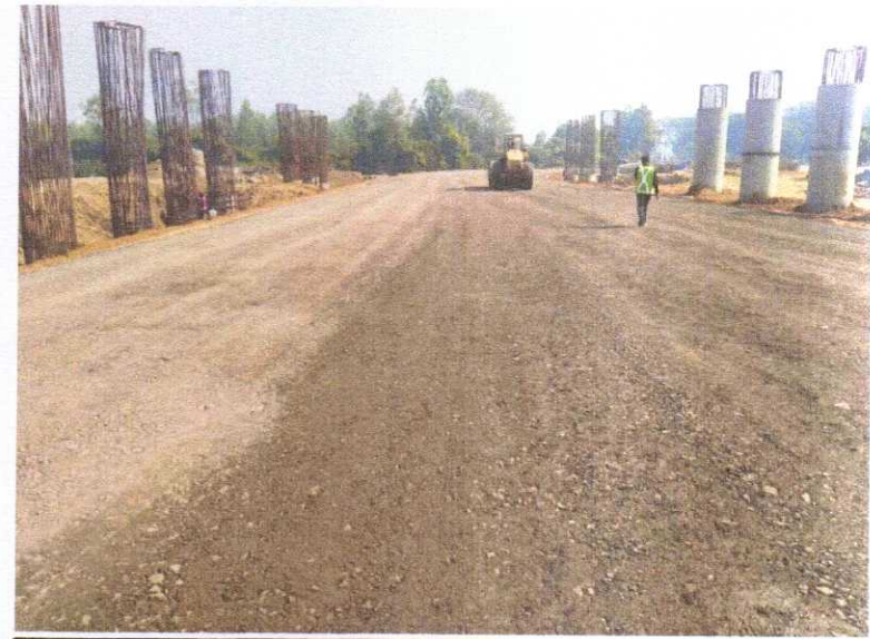
GSB TOP IN PROGRESS AT CH- 353+666 FORDIVERSION ROAD INTERCHANGE LOCATION
