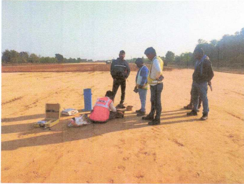
FDD CHECKING AT 354+360 TO 354+460 EMB LAYER BHS
