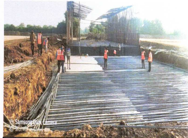
352+700 CUP BHS RAFT REINFORCEMENT CUTTING AND BINDING WORK IN PROGRESS
