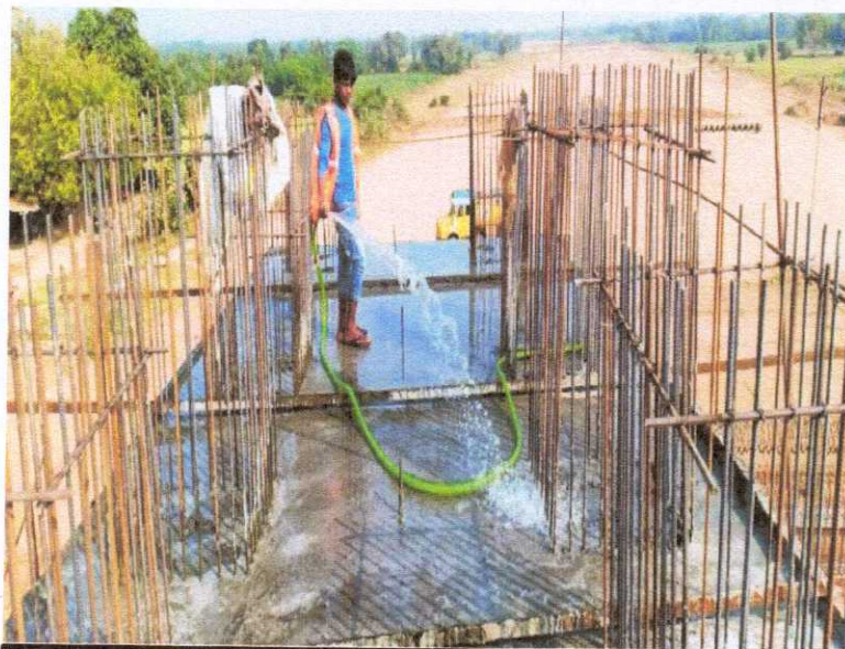
349+441 VOP PIER CAP CURING WORK IN PROGRESS
