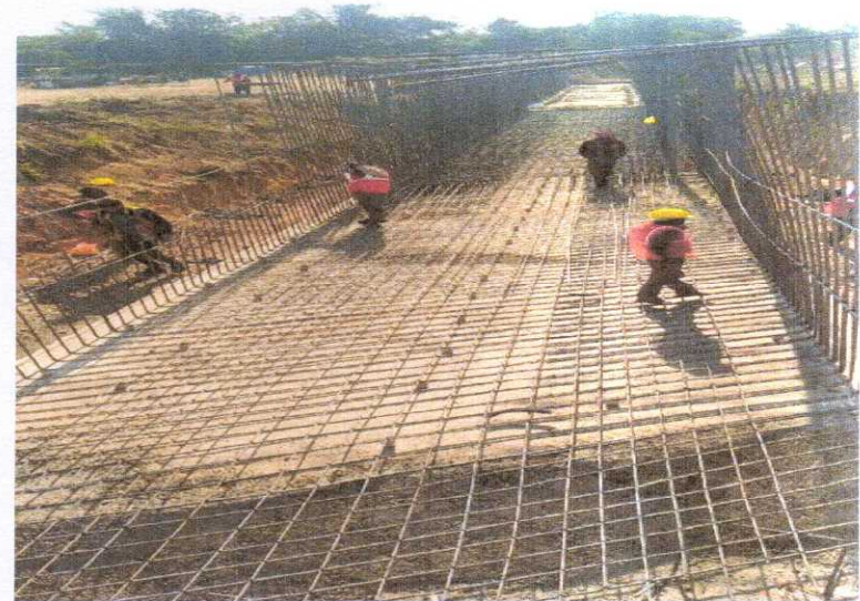
332+659 BOX CULVERT LHS RAFT STEEL BINDING WORK IS IN PROGRESS
