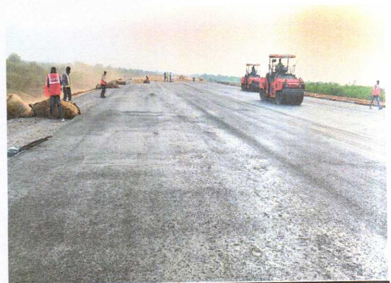
ROLLING AND HESSIAN CLOTH SPREADING WORK IS IN PROGRESS AT DLC
