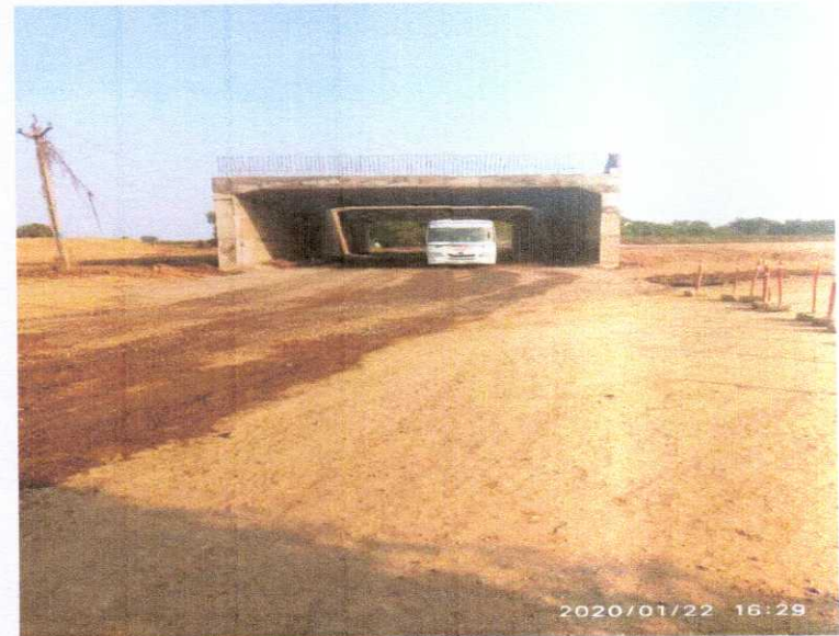
325+769 LVUP DIVERSION CLOSED & TRAFFIC PERMITTED
