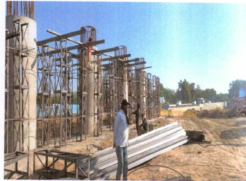
353+666 INTERCHANGE STAGING FOR PIER CAP IN PROGRESS
