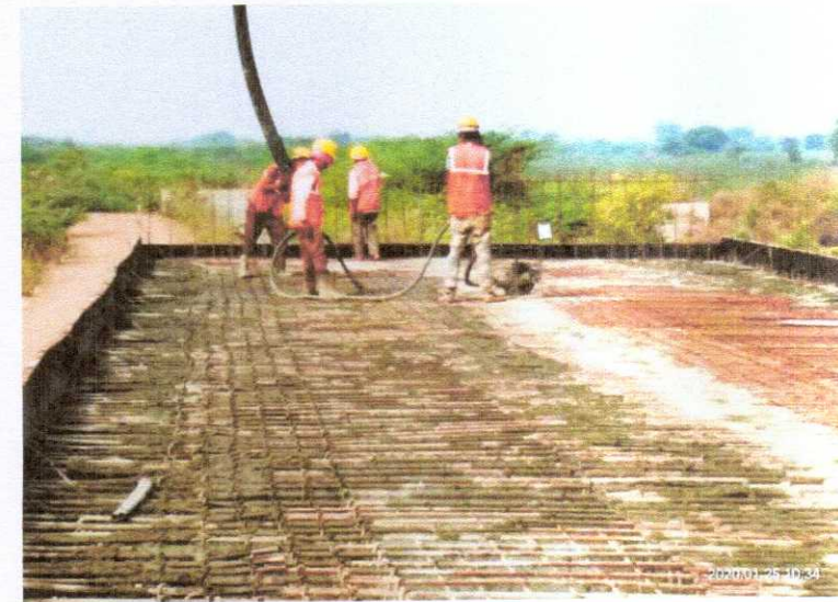
324+236 BOX CULVERT SLAB CONCRETE POURING WORK IS IN PROGRESS
