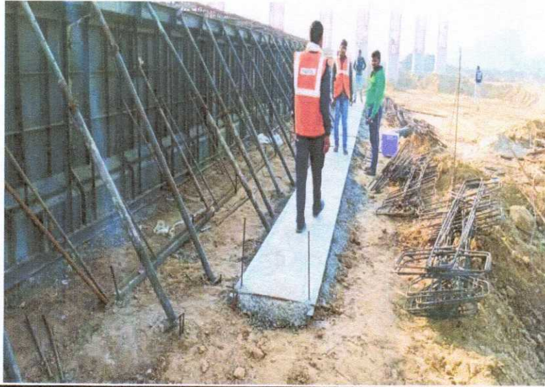
354+636 MNB GIRDER STEEL MAKING & BINDING WORK IS IN PROGRESS
