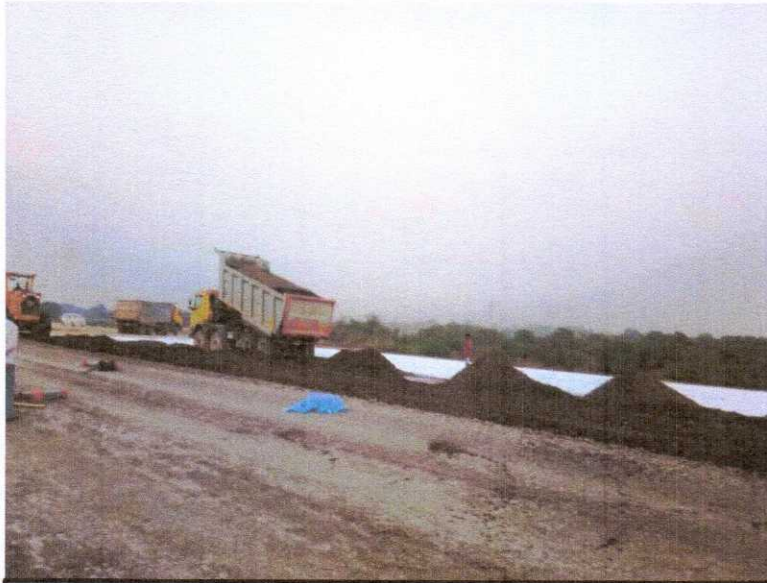
GSB DUMPING WORK IS IN PROGRESS AT 337+960 TO 338+050 RHS
