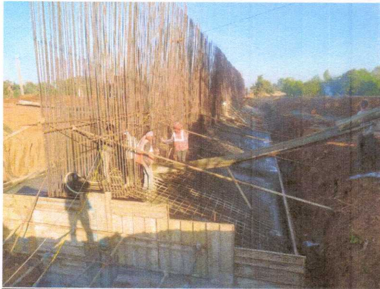
353+490 TO 510 RHS RAFT RETAINING WALL CONCRETE POURING IN PROGRESS
