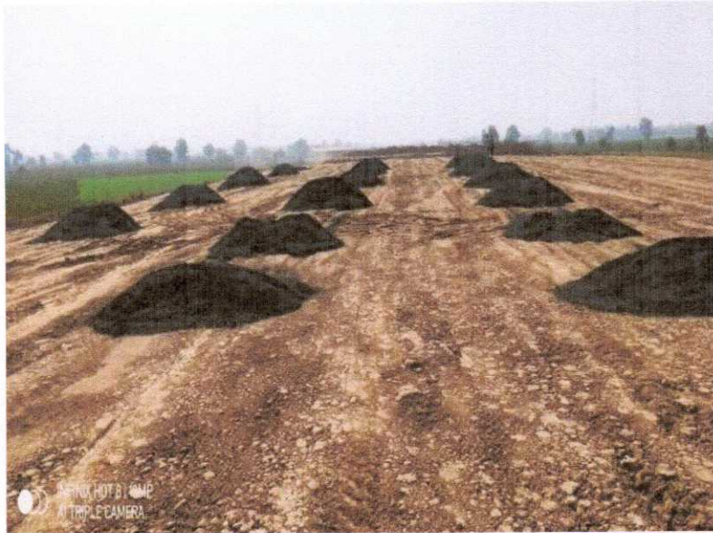
CPR SLAG UNLOADING AT KM 327+610-700
