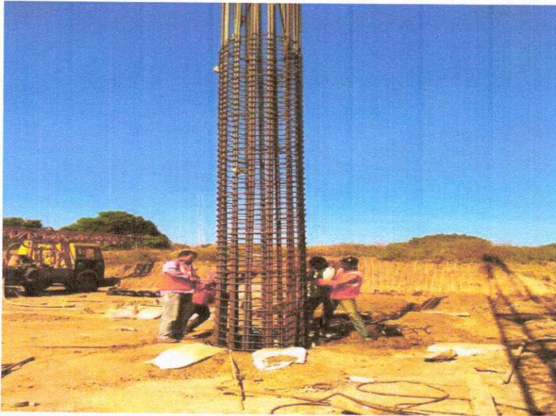
336+810 MJB MIDDLE AND BOTTOM CAGE LAP JOINT COMPLETED
