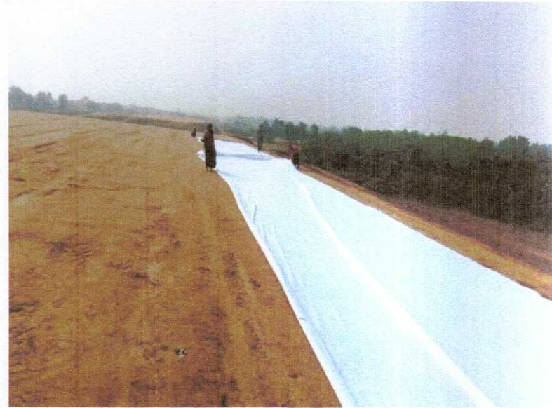
GEO TEXTILE LAYING WORK IS IN PROGRESS
