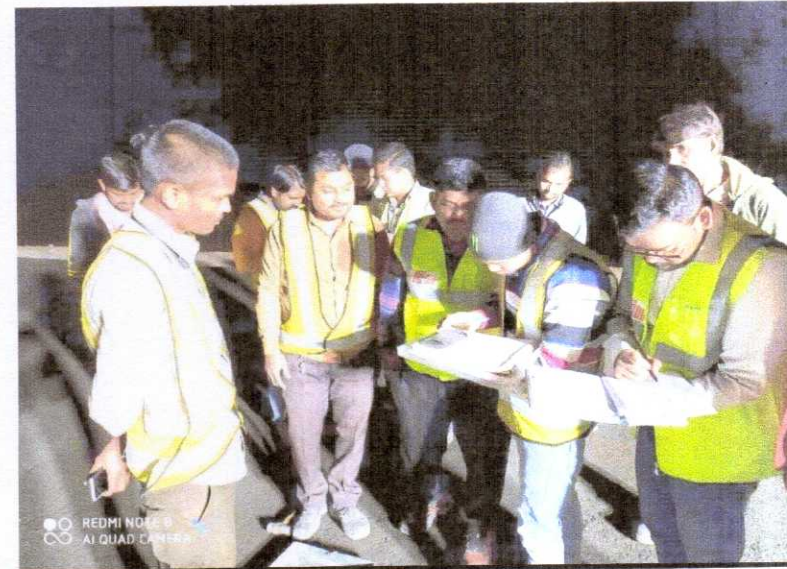
FDD TEST OF DLC FROM CH. 337+960 TO 338+060 AFTER LAYING & ROLLING
