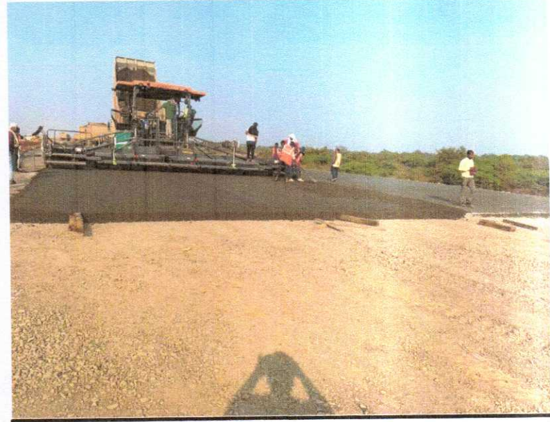
DLC LAYING WORK IS IN PROGRESS AT 338
