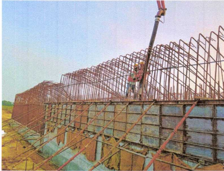
327+575 CUP CONCRETE POURING WORK IS IN PROGRESS
