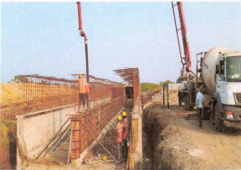
324+236 BOX CULVERT LHS MIDDLE WALL CONCRETE POURING IN PROGRESS
