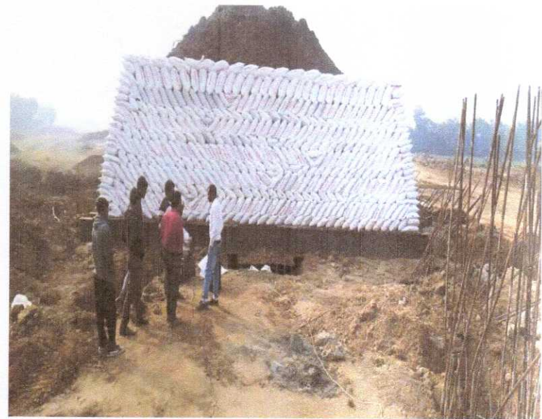
354+636 MNB INITIAL PILE LOAD TESTING
