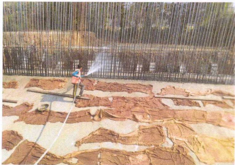
RETAINING WALL 353+490 TO 510 RHS RAFT CONCRETE POURING IS IN PROGRESS
