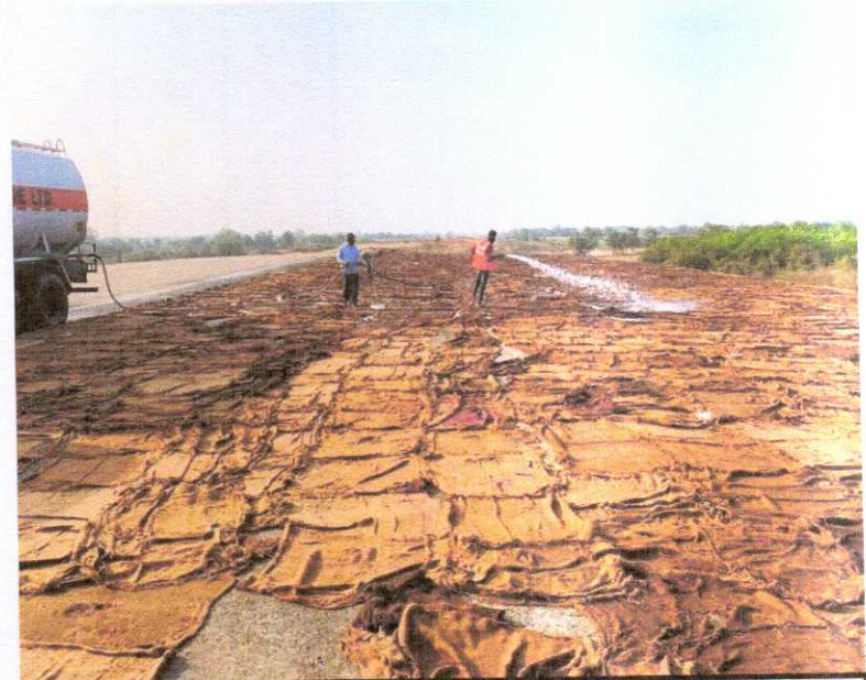
DLC CURING WORK IS IN PROGRESS
