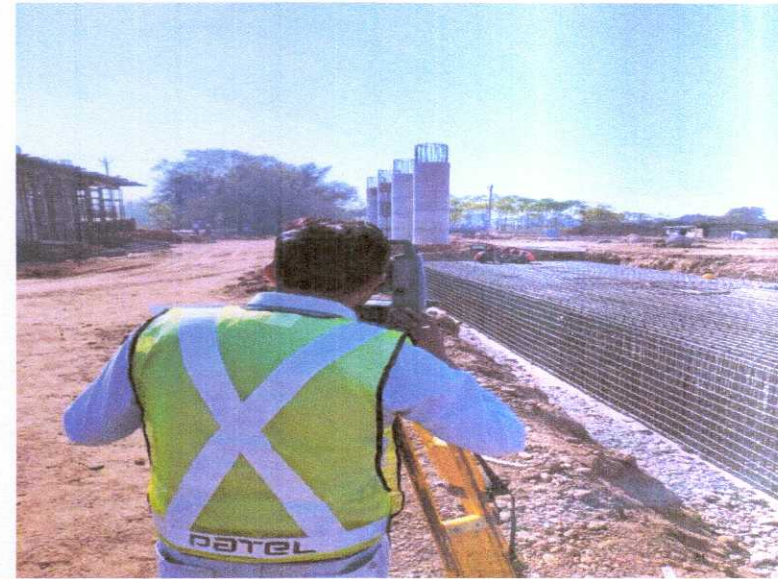
344+383 LAYOUT MARKING OF PEIR POINTS ON PILE CAP STEEL TOP
