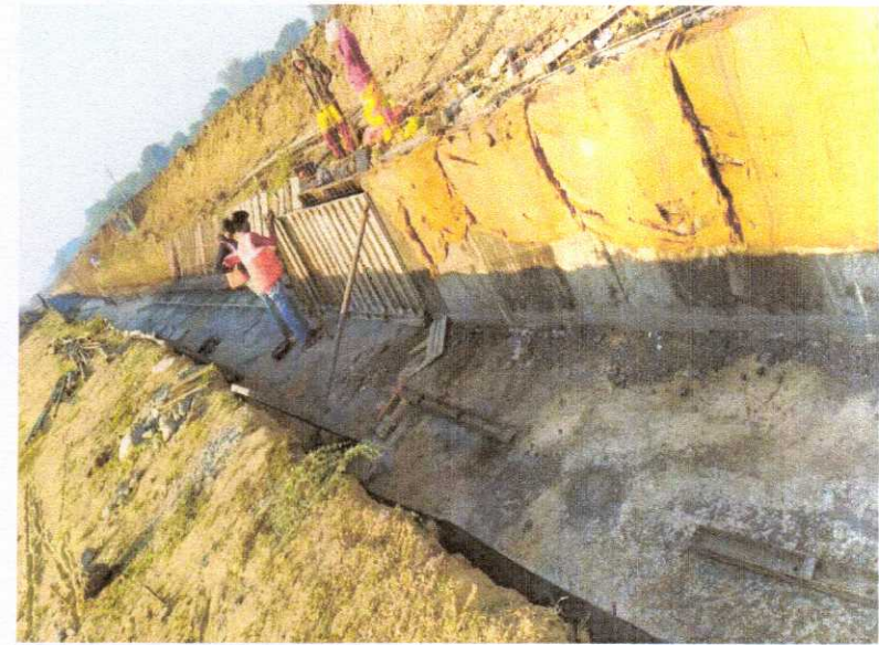
TOE WALL 347+050 WALL SHUTTERING WORK IN PROGRESS
