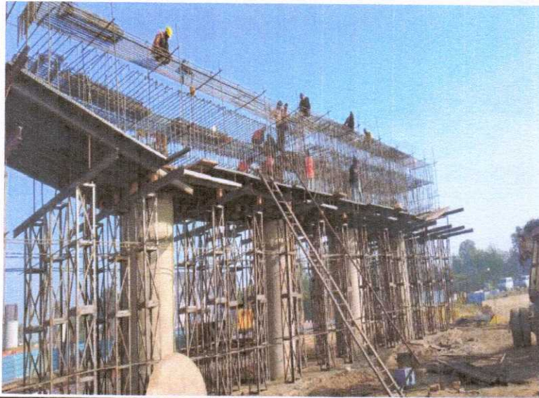
353+666 INTERCHANGE SHUTTERING WORK FOR PIER CAP WORK IS IN PROGRESS
