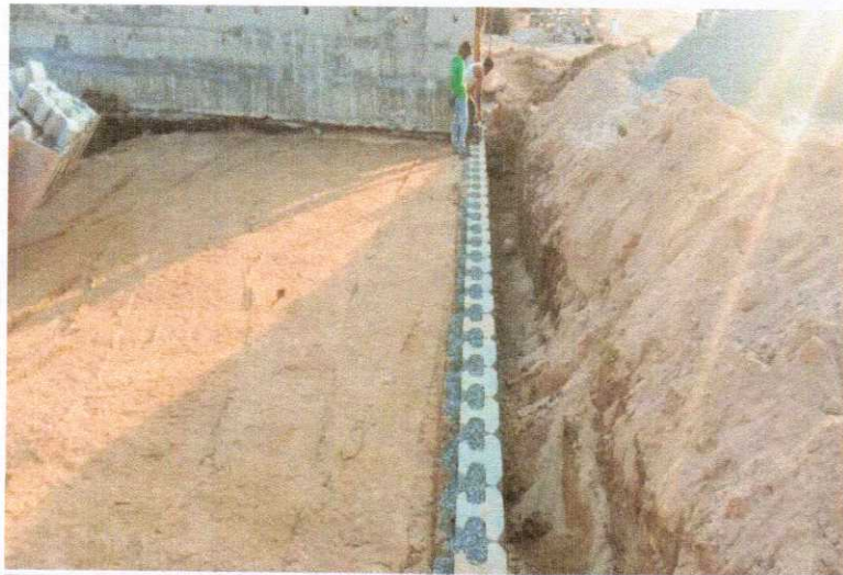
334+280 CUP RE WALL LHS SIDE BLOCK ERECTION WORK IS IN PROGRESS
