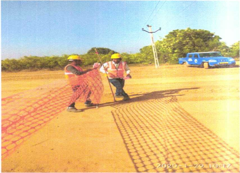
OVERHEAD POWER LINE WARNING BARRIER INSTALLATION AT 355
