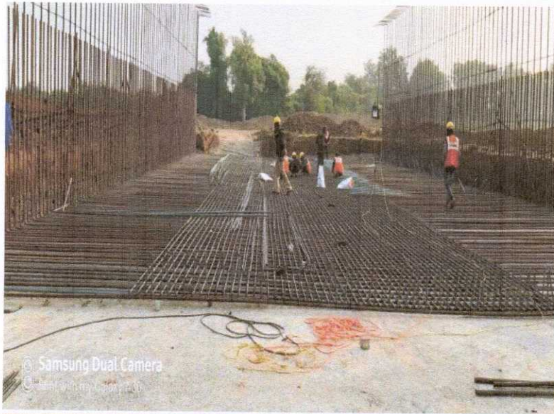
352+700 CUP REINFORCEMENT CUTTING AND BINDING WORK IS IN PROGRESS
