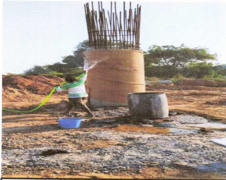
354+636 MNB PIER SHAFT CURING WORK
