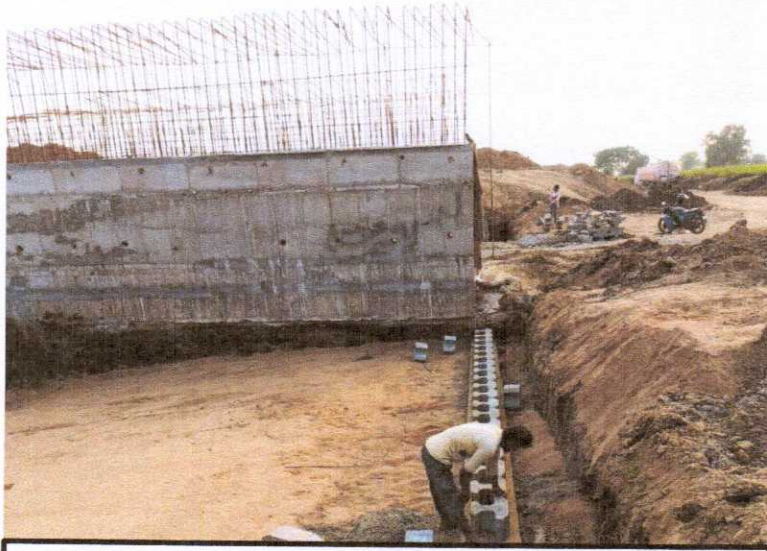
334+280 CUP LHS RE WALL BLOCKS ERECTION WORK IS IN PROGRESS
