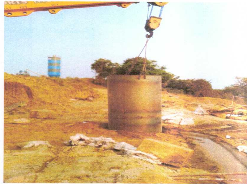
336+810 MJB LINER PUNCHING IN PROGRESS
