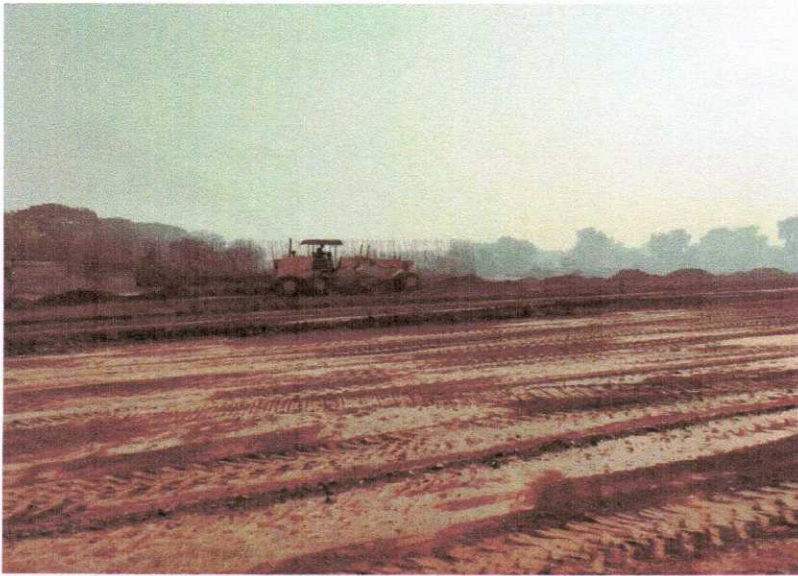
GRADING WORK IS IN PROGRESS AT 353+250 TO 353+350
