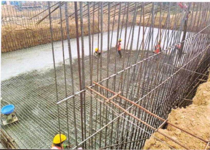
332+621.5 CUP RHS RAFT CONCRETE POURING IN PROGRESS
