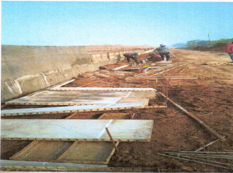
354+850 TOE WALL SHUTTERING WORK IN PROGRESS
