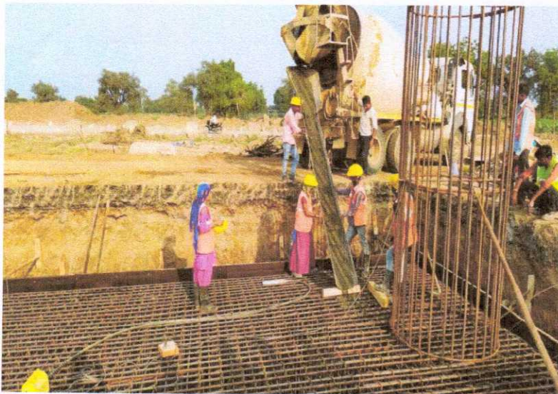
344+383 FLYOVER PILE CAP CONCRETE POURING IS IN PROGRESS
