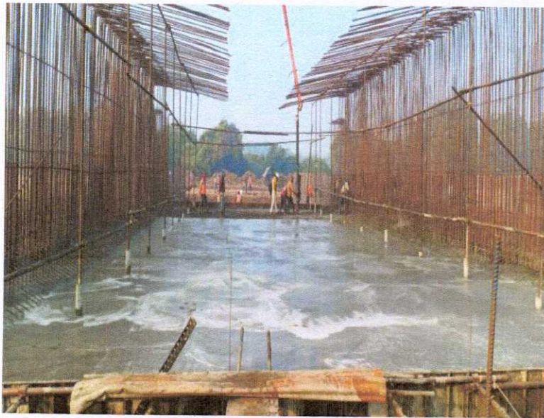
352+700 CUP RAFT CONCRETE POURING IS IN PROGRESS
