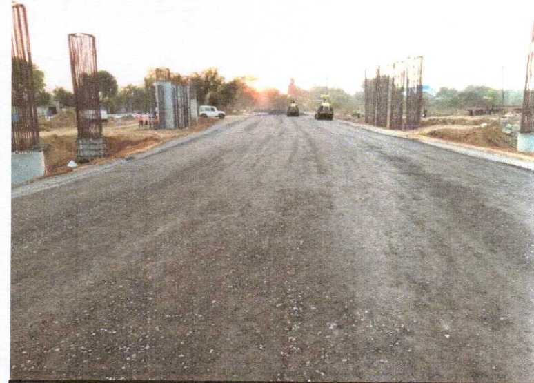
WMM WORK IS IN PROGRESS INTERCHANGE DIVERSION 353+661
