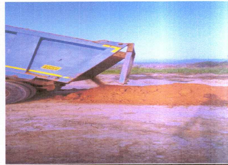
SOIL DUMPING WORK IS IN PROGRESS
