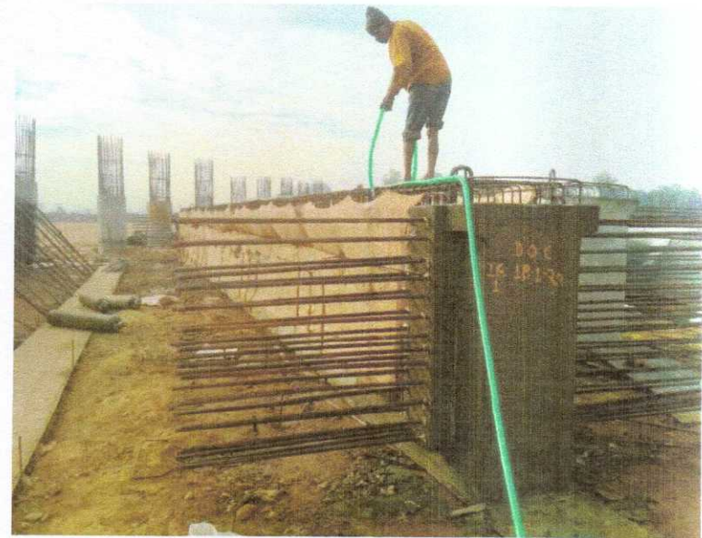
354+636 MNB GIRDER CURING WORK IS IN PROGRESS
