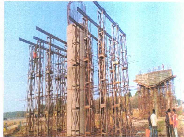
349+441 VOP PIER CAP STAGING WORK IN PROGRESS
