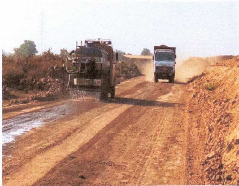
WATERING ON ROAD AT KM 329+500 TO 330+400
