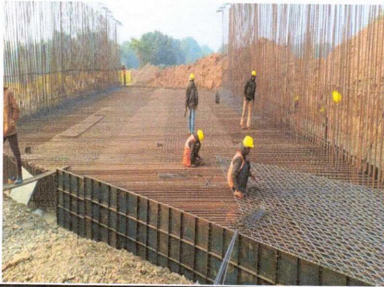
351+800 LVUP LINK BAR BINDING AND SHUTTERING WORK IS IN PROGRESS
