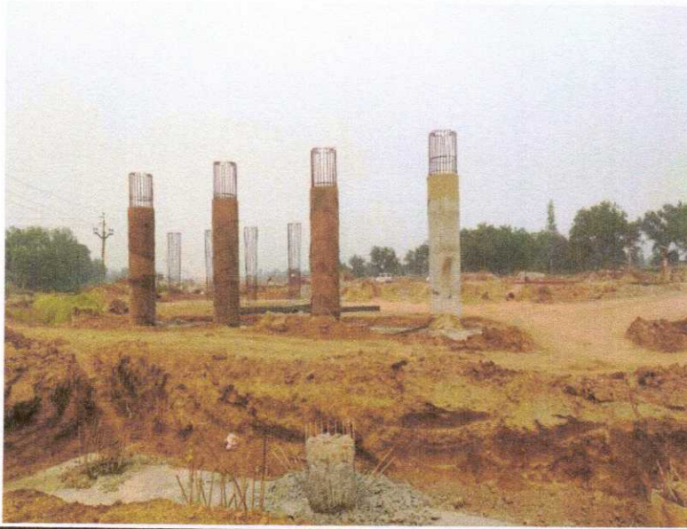
344+383 FLY OVER CURING WORK IS IN PROGRESS
