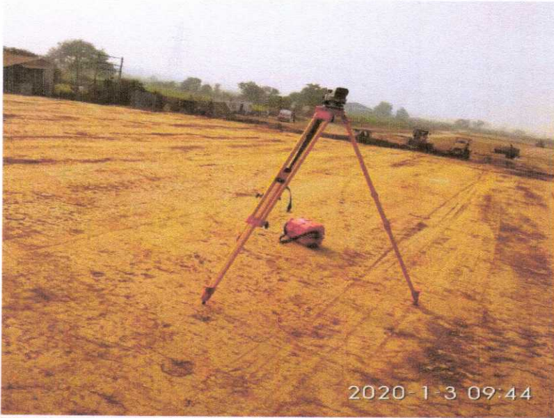
A NEW AUTO LEVEL FOR PREPARATION OF EMBANKMENT TOP
