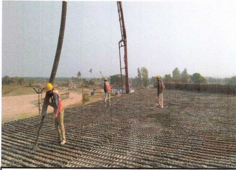
330+402 VUP SLAB AND TOP HAUNCH CONCRETE POURING IS IN PROGRESS
