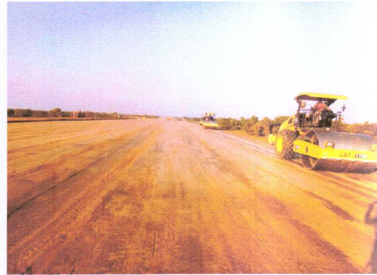
ROLLING WORK IN PROGRESS RHS ON SG TOP FROM 335+460 TO 335+590
