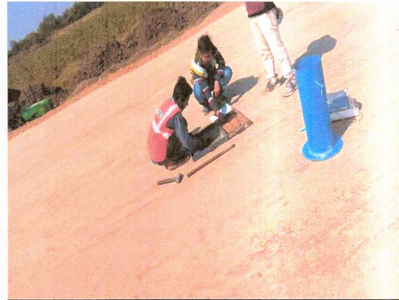
FDD TESTING WORK IN PROGRESS FROM CH338+200 TO 400
