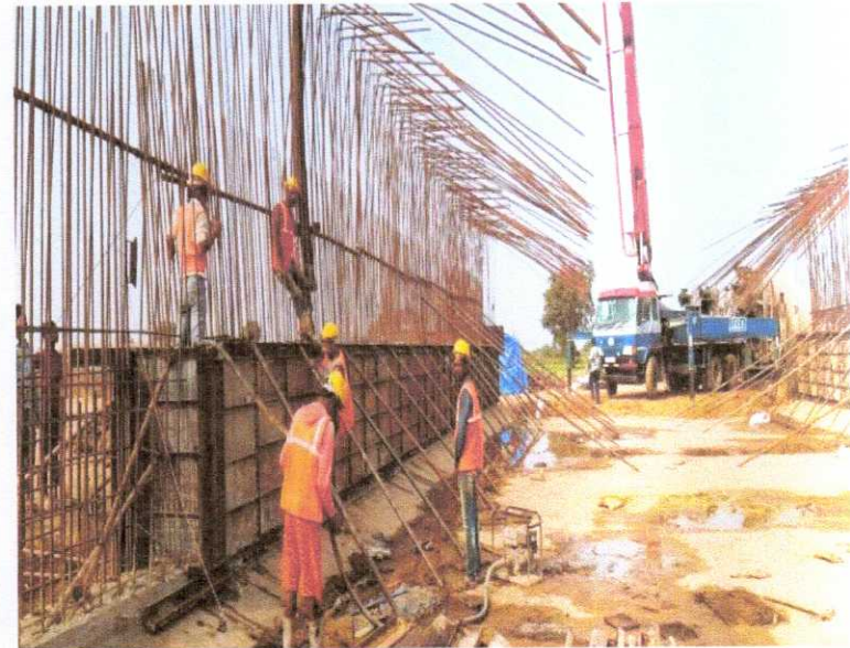
327+575 CUP WALL LIFT CONCRETE POURING IN PROGRESS
