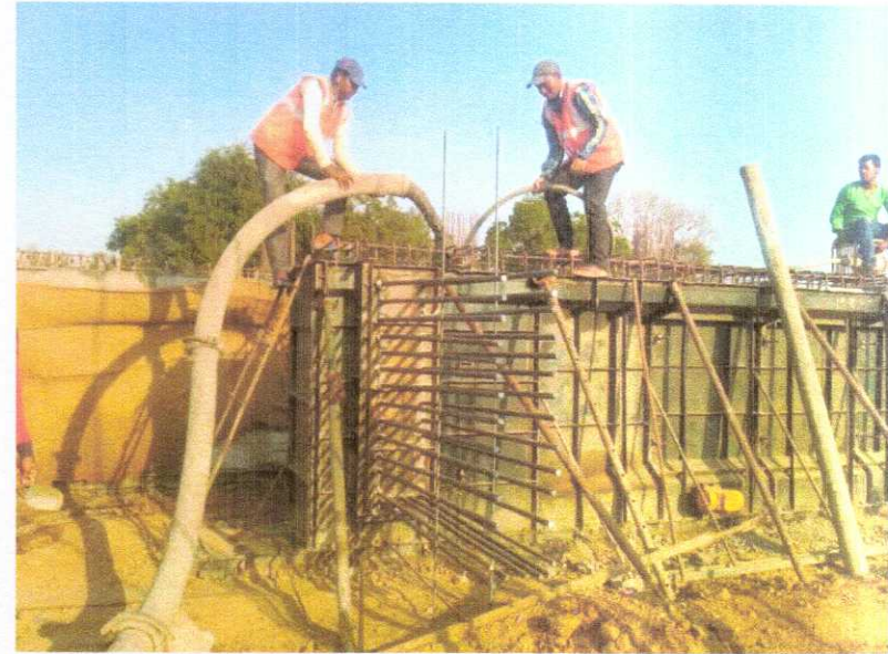
354+636 MNB GIRDER CONCRETE POURING IN PROGRESS
