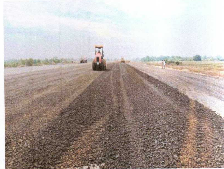
GSB TOP LAYING IN PROGRESS AT CH- 337+630 TO 760 LHS
