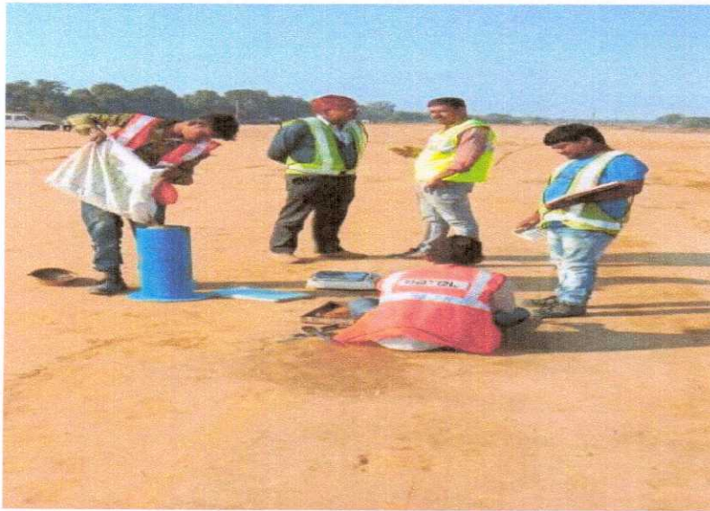
CHECKING OF EMB. LAYER FROM CH 354+000 TO 354+100
