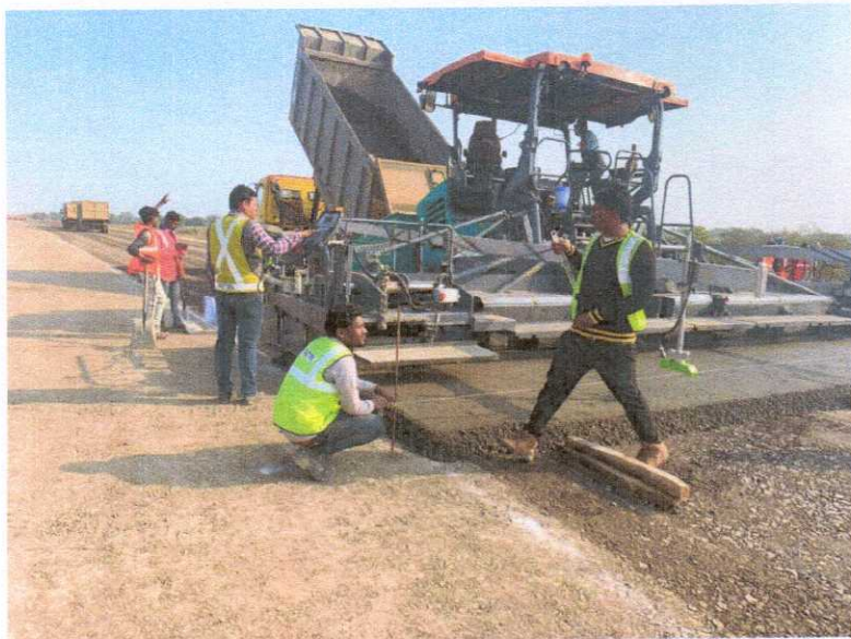
DLC LAYING WORK IS IN PROGRESS
