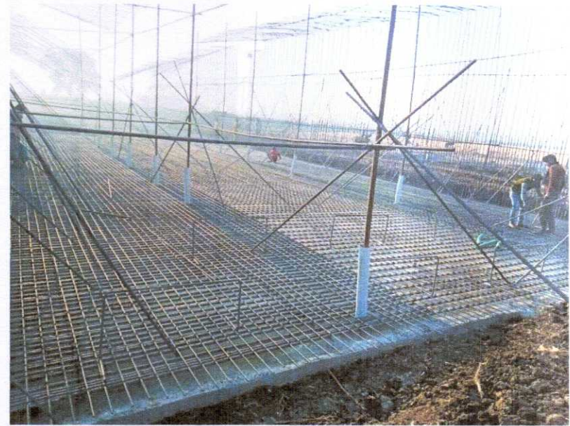
331+425 CUP LHS RAFT STEEL BINDING WORK IS IN PROGRESS
