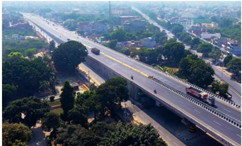
The Zirakhpur-Bathinda stretch of NH-64 is well equipped with a three-grade separator flyover bridge, four underpasses, one rail over-bridge, seven minor bridges over river and 38 culverts, among others.
